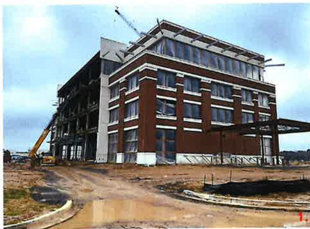
Progress as of 2-22-2021.
