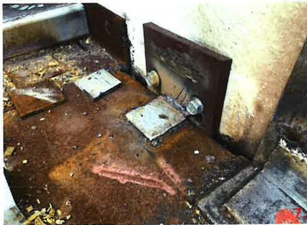
Panel 104-1 has been modified with FM 02-1. HD screw-in anchors were installed instead of epoxy threaded rods at these two connections.
