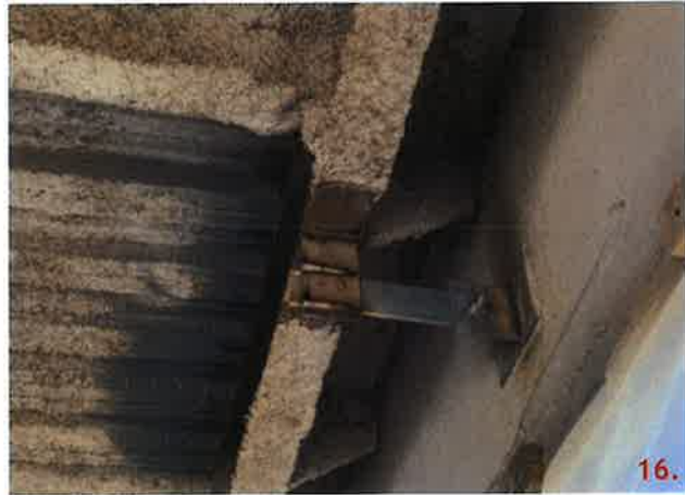
Panel 217B-1 and 203B-2 have been modified with FM-11.1. This detail requires the use of a L4x4x3/8 to be welded to the structural steel. This connection has a 6x8x3/8 plate instead.
