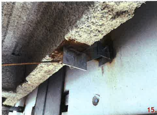
Panel 217B-1 and 203B-2 have been modified with FM-11.1. This detail requires the use of a L4x4x3/8 to be welded to the structural steel. This connection has a 6x8x3/8 plate instead.
