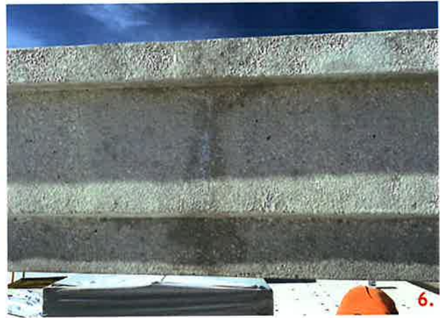
Panel 105-1 has another location that is not reinforced.
