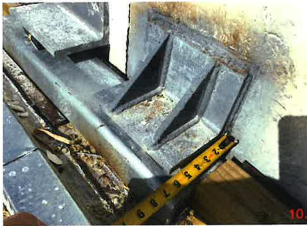
Panel 122-1, at connection point 22 the embedded angle was installed too high but not 4" high. The bottom leg of the angle was cut off and a new L6x6 angle with gussets was welded to the embedded angle all around. A field modification was not provided for this connection.
