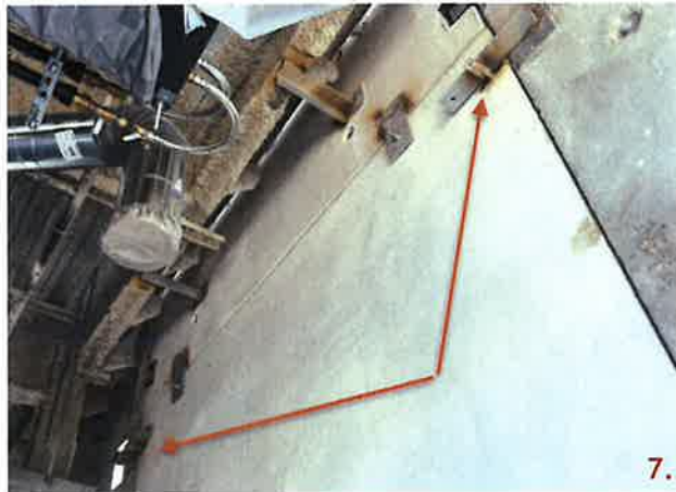
Panel 242 between grid lines 5 and 6 at elevation 16'-0" has two connections with angles welded to the plate and the 6" PSA strap.
