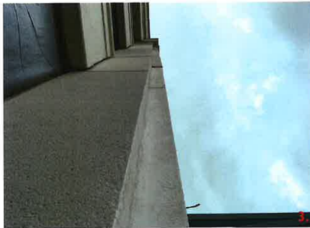
Panel 107 at grid line G is approximately 1/4" out of plumb over a span of 6'. This indicates that panel 107 is installed too far away from the building to achieve proper alignment with the panel above.
