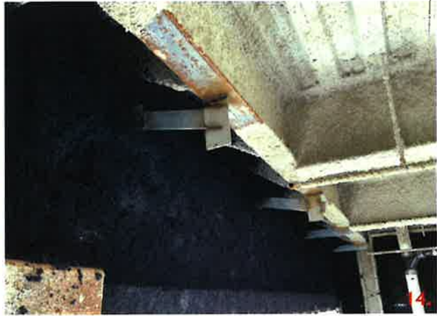
Panel 114 has two connections detailed 11 that have been modified similar to FM 11-1. Instead of using a L4x4x3/8x1'-7" a PL3/8x6x8" was used.
