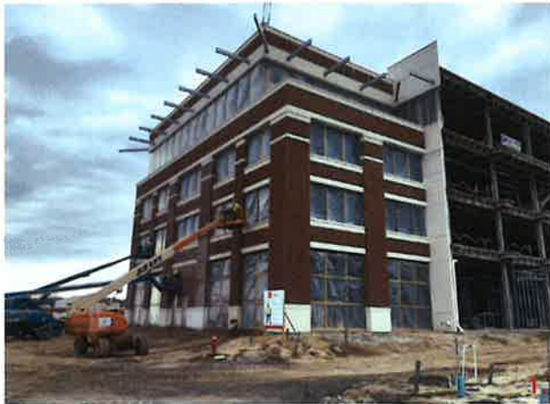
Progress as of 1/19/2021.
