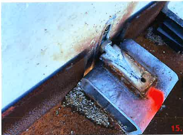
Panel 104-2 has a connection point detailed 02 that has a HSS6x3x3/8 6" length below the PSA strap.
