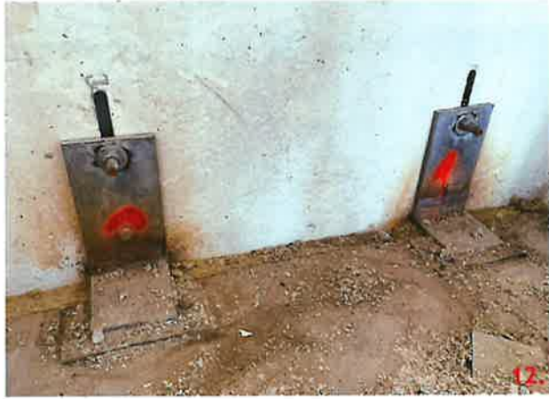
Panel 112-1 has been field modified at connection point detailed 10.
