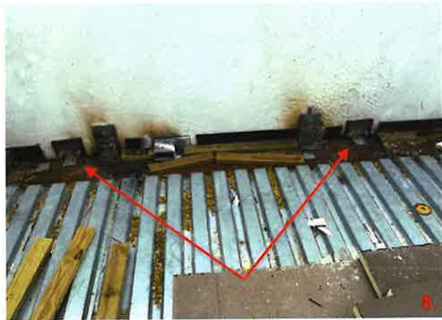
Panel 104-1 has been modified with FM 02-1. HD screw-in anchors were installed instead of epoxy threaded rods at these two connections.
