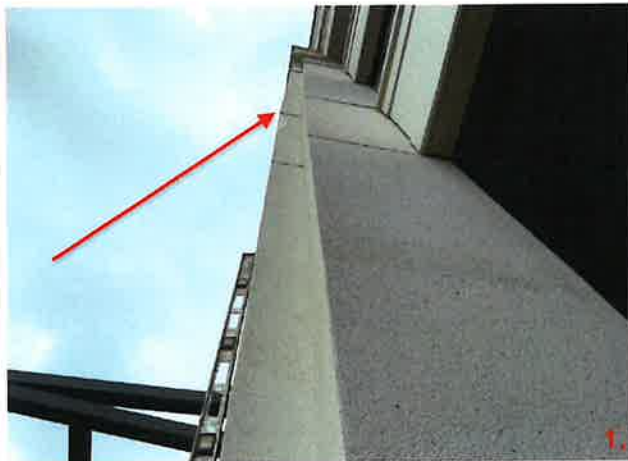
Panel 107 at grid line D is approximately 1" out of plumb over a span of 6'. It appears that adjusting panel 107 at the top will produce proper alignment of the panels.
