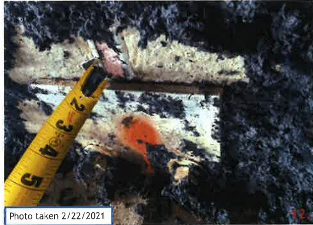
Panel 215-1 has two connection points that have been field modified similar to FM-10.1. A 6" PSA strap was used at this connection instead of a 3/8x3x5 plate. The plates attached to the panel are 1/2" thick. FM10.1 requires 3/4" plates.
