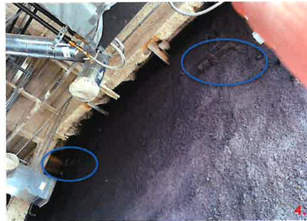
Panel 243 near grid line 4 at elevation 16'-0" has an angle welded to the plate and the 6" PSA strap.
