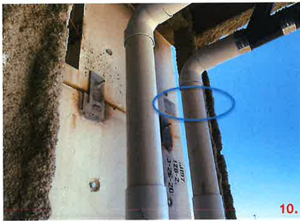
Panel 103-1 & 129-1 are not connected to the structural steel as detailed on 28.
