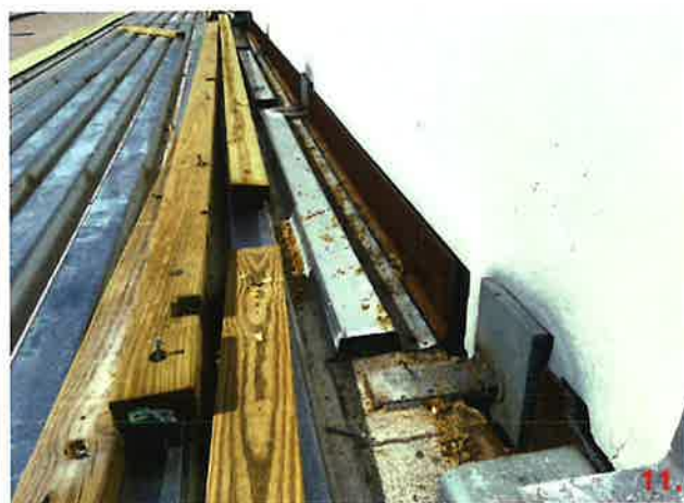
Panels 123-2, 124-2, 125-1 and 126-1 have modifications at the 07 and 02 connections. It does not appear that these connections needed a modification as the threaded rod is screwed into the PSA clip at an elevation that would have permitted the 3/4" diameter smooth rod and 6" PSA strap to be welded to the perimeter angle.
