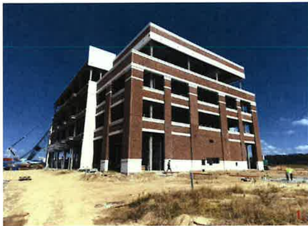
Progress as of 10/7/2020.
