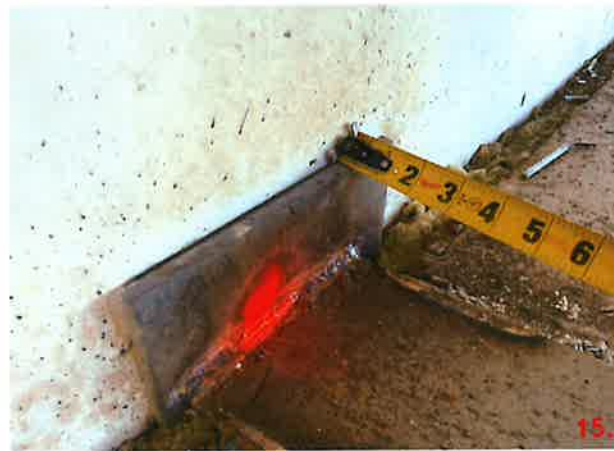
Panel 117-1 and 116-2 have two connection points detailed 10 that have been field modified using FM 10.2. The field modification requires a 3/4" thick vertical plate and a 1/2" thick plate was used.
