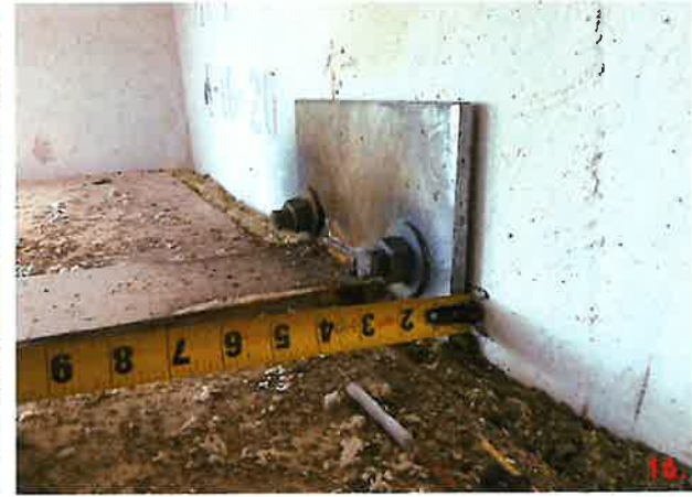
Panel 117-1 and 116-2 have two connection points detailed 9 that have been field modified using FM 9.2. The field modification requires a 3/4" thick vertical plate and a 1/2" thick plate was used.
