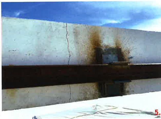
Panel 105-1 has another location that is not reinforced.
