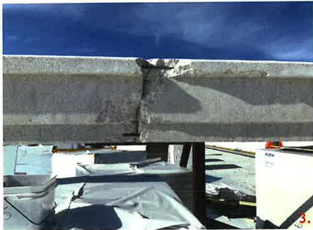
Panel 105-1 is cracked in two locations. One of the locations has been reinforced with L6x6 angle and 3/4x4" HD screw anchors.
