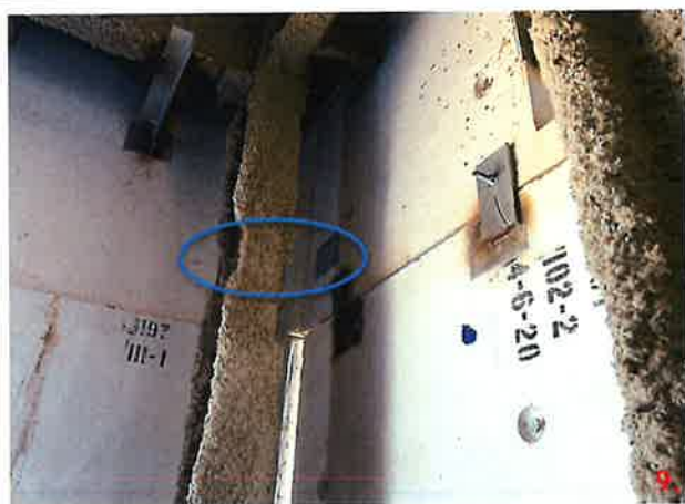
Panel 103-1 & 129-1 are not connected to the structural steel as detailed on 28.
