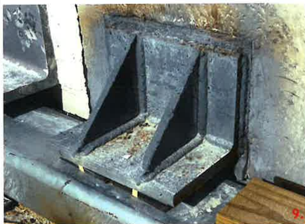
Panel 122-1, at connection point 22 the embedded angle was installed too high but not 4" high. The bottom leg of the angle was cut off and a new L6x6 angle with gussets was welded to the embedded angle all around. A field modification was not provided for this connection.
