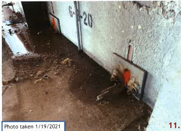
Panel 215-1 has two connection points that have been field modified similar to FM-10.1. A 6" PSA strap was used at this connection instead of a 3/8x3x5 plate. The plates attached to the panel are 1/2" thick. FM10.1 requires 3/4" plates.
