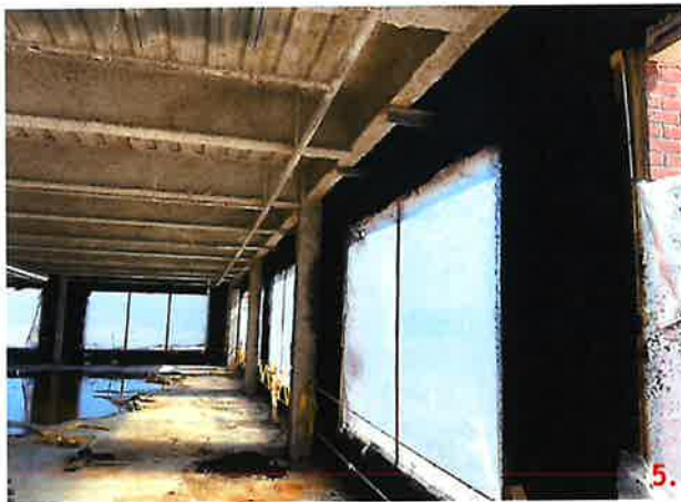
Panel 248-4, 203A-2, 217-4, 217-6, 222-2, 217-5, 217-3, 249-2 & 203B-2 connection points detailed 11 do not have 3/8x6x6 plates with slotted holes welded to the embedded plate.
