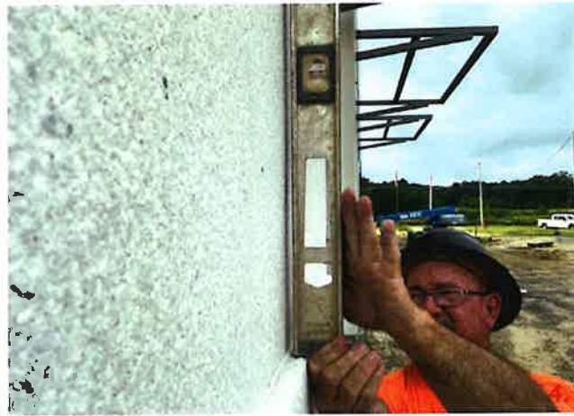
Panel 107 at grid line G is approximately 1/4" out of plumb over a span of 6'. This indicates that panel 107 is installed too far away from the building to achieve proper alignment with the panel above.
