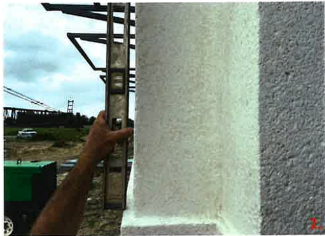
Panel 107 at grid line D is approximately 1" out of plumb over a span of 6'. It appears that adjusting panel 107 at the top will produce proper alignment of the panels.
