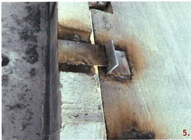
On panels 239 and 240 below elevation 20'-0" between grid lines 4 and 5, plates and angles were used as spacers to achieve the desired placement of the panels.
