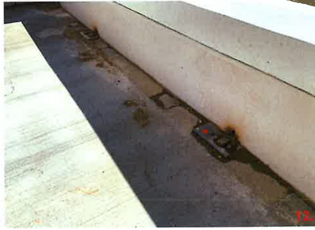
Panel 207-2 is connected to the slab at two connections with a PSA strap that is welded to plate 1/2"x6"x12". This plate is anchored to the slab with (2) 5/8" anchors. These anchors are approximately 4" from the edge of the slab.
