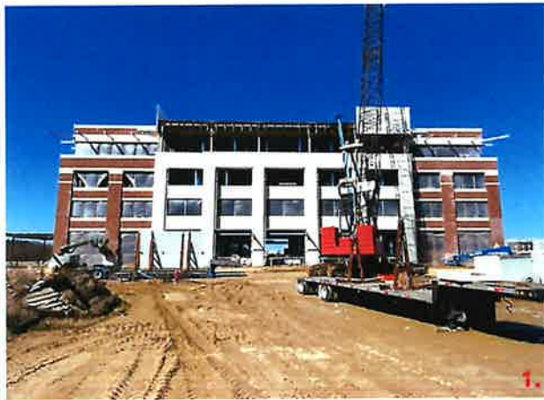
Progress as of 2-23-2021.
