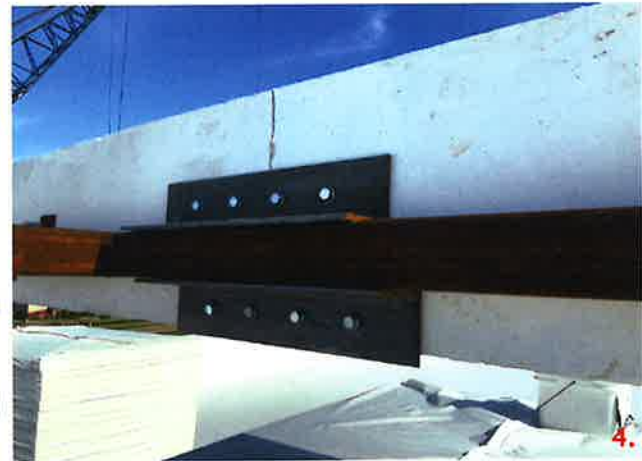
Panel 105-1 is cracked in two locations. One of the locations has been reinforced with L6x6 angle and 3/4x4" HD screw anchors.
