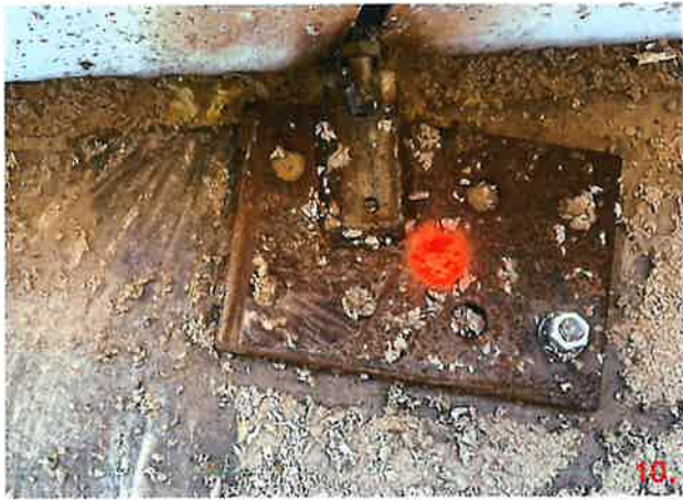
Panel 109-13 and 109-10 have two connection points detailed 10 that have been field modified. The PSA strap is welded to a plate 1/2x7x10 that is welded to the embed on one side and anchored to the slab on the other side. FM 10.4 and FM 10.3 could have been used for these connections.
