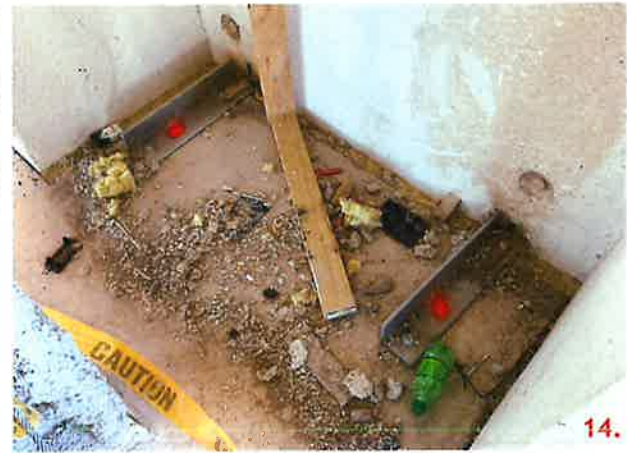
Panel 112-6 and 112-9 have been field modified. A section of the slab has been cut off. A L4x4x3/8 19" length is welded to the remainder of the embeds and a 5/8 anchor is installed in the slab approximately 16" from the edge. The PSA strap is welded to the 1/2x6x12 plate. A FM was not provided for these connections.
