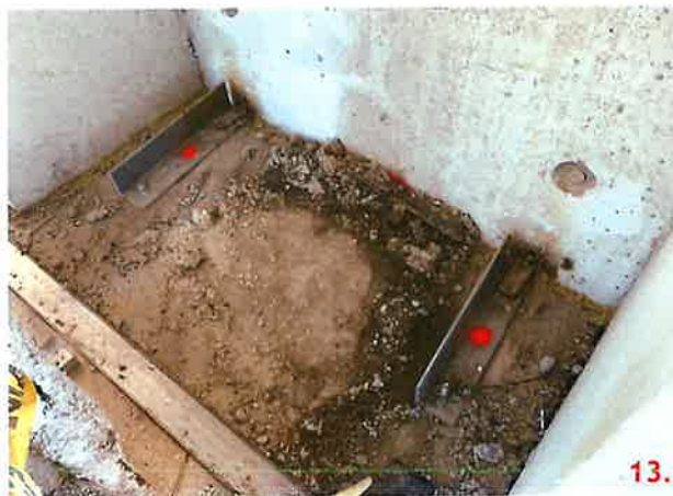
Panel 112-6 and 112-9 have been field modified. A section of the slab has been cut off. A L4x4x3/8 19" length is welded to the remainder of the embeds and a 5/8 anchor is installed in the slab approximately 16" from the edge. The PSA strap is welded to the 1/2x6x12 plate. A FM was not provided for these connections.
