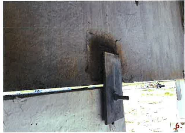
On panels 239 and 240 below elevation 20'-0" between grid lines 4 and 5, plates and angles were used as spacers to achieve the desired placement of the panels.
