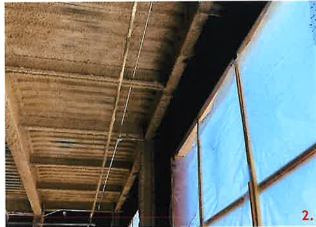
Panel 248-1, 203A-3, 217-2, 245, 244, 245-1, 217-1, 203B-1 & 249-4 connection points detailed 11 do not have 3/8x6x6 plates with slotted holes welded to the embedded plate.
