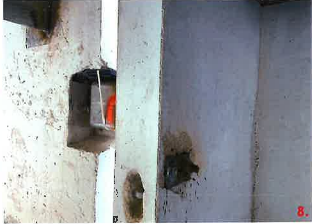
Panel 118-2 connection point detailed 18 has been field modified. The HSS6x3x3/8 has been welded to a plate 3/8x4x11.5. The plate is welded to the embed plate of panel 117-1 with a 1/4" fillet weld 4" length on three sides. The 3/8x4x11.5 plate is bolted through panel 117-1 with two 3/4 threaded rods with a 3x4x3/8 plate backer along with washers and nuts.
