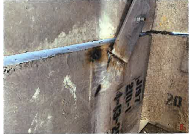
Panel connections of 210 and 219 at elevation 22'-0" at grid line 7 are skewed.
