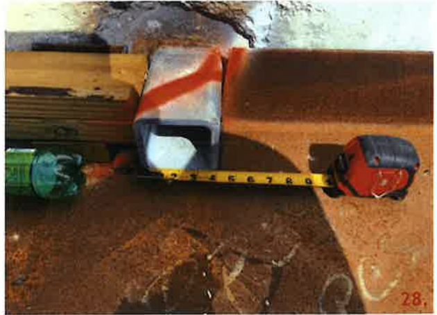
Panel 130-2, 230-1 and 231-2 have a load bearing point that has been field modified using FM-01.2. A HSS4x4x3/8 6" length was used instead of a HSS6x3x3/8 3.5" length.
