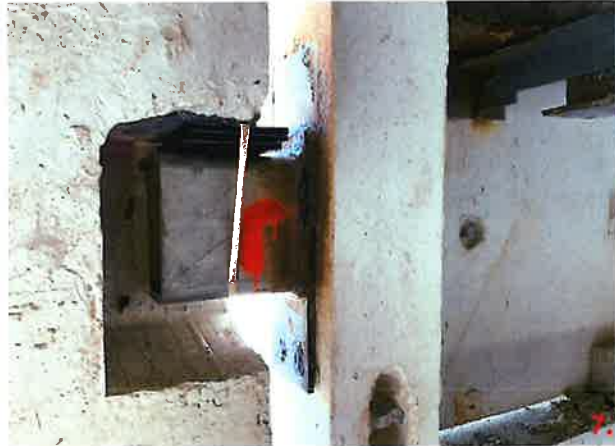
Panel 118-2 connection point detailed 18 has been field modified. The HSS6x3x3/8 has been welded to a plate 3/8x4x11.5. The plate is welded to the embed plate of panel 117-1 with a 1/4" fillet weld 4" length on three sides. The 3/8x4x11.5 plate is bolted through panel 117-1 with two 3/4 threaded rods with a 3x4x3/8 plate backer along with washers and nuts.
