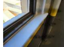
Wall at Top of West Bleachers From South to North Photo 21
