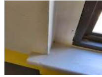
Wall at Top of West Bleachers From South to North Photo 14
