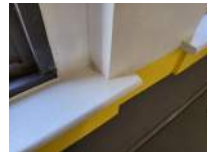
Wall at Top of West Bleachers From South to North Photo 26
