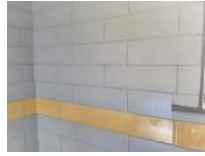
Men's Restroom 22 Darryl Dilmore Aug 30, 2022 9:55 AM
