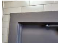
Women's Restroom Photo 10 Darryl Dilmore Aug 30, 2022 9:33 AM
