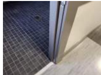
Women's Restroom Photo 2 Darryl Dilmore Aug 30, 2022 9:32 AM
