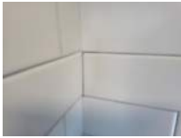
Men's Restroom 26 Darryl Dilmore Aug 30, 2022 9:56 AM
