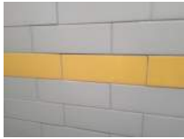
Women's Restroom Photo 21 Darryl Dilmore Aug 30, 2022 9:35 AM
