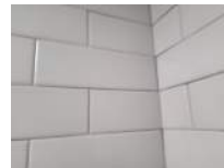
Women's Restroom Photo 9 Darryl Dilmore Aug 30, 2022 9:33 AM
