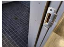
Women's Restroom Photo 3 Darryl Dilmore Aug 30, 2022 9:32 AM
