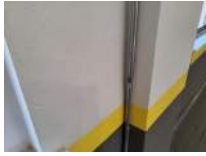
Wall at Top of West Bleachers From South to North Photo 12
