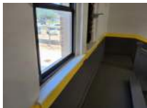
Wall at Top of West Bleachers From South to North Photo 30
