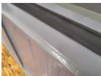
West Bleachers Photo 32 Darryl Dilmore Aug 30, 2022 11:03 AM
