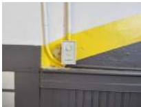
North Wall Photo 10
