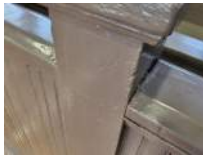
West Bleachers Photo 9 Darryl Dilmore Aug 30, 2022 11:00 AM
