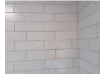
Men's Restroom 24 Darryl Dilmore Aug 30, 2022 9:56 AM
