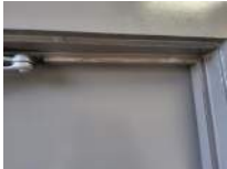
Men's Restroom 5 Darryl Dilmore Aug 30, 2022 9:53 AM
