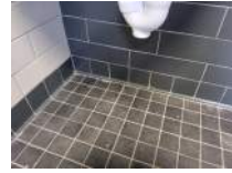
Women's Restroom Photo 20 Darryl Dilmore Aug 30, 2022 9:35 AM
