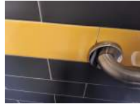
Women's Restroom Photo 17 Darryl Dilmore Aug 30, 2022 9:34 AM
