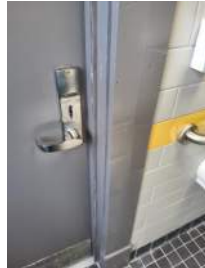
Men's Restroom 7 Darryl Dilmore Aug 30, 2022 9:54 AM
