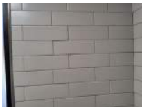
Women's Restroom Photo 6 Darryl Dilmore Aug 30, 2022 9:32 AM
