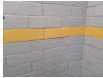
Women's Restroom Photo 22 Darryl Dilmore Aug 30, 2022 9:35 AM
