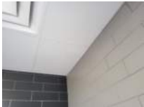
Men's Restroom 30 Darryl Dilmore Aug 30, 2022 9:56 AM
