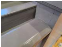
West Bleachers Photo 6 Darryl Dilmore Aug 30, 2022 11:00 AM
