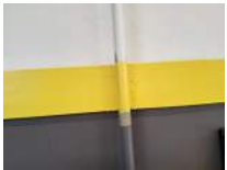
North Wall Photo 3
