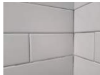
Women's Restroom Photo 8 Darryl Dilmore Aug 30, 2022 9:33 AM
