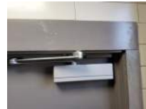
Women's Restroom Photo 11 Darryl Dilmore Aug 30, 2022 9:33 AM
