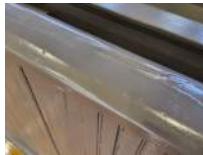
West Bleachers Photo 11 Darryl Dilmore Aug 30, 2022 11:00 AM
