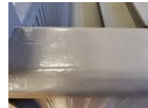
West Bleachers Photo 19 Darryl Dilmore Aug 30, 2022 11:01 AM
