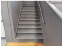
Bleacher Access Stairs Photo 1
