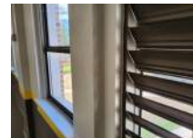
Wall at Top of West Bleachers From South to North Photo 35
