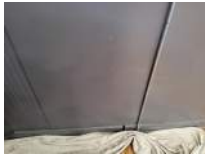
South Wall Photo 4 Darryl Dilmore Aug 30, 2022 11:32 AM
