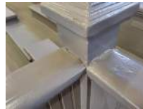
West Bleachers Photo 17 Darryl Dilmore Aug 30, 2022 11:01 AM
