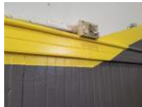
South Wall at West Bleachers 5 Darryl Dilmore Aug 30, 2022 11:05 AM
