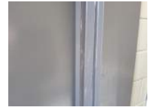
Men's Restroom 4 Darryl Dilmore Aug 30, 2022 9:53 AM
