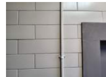
Women's Restroom Photo 14 Darryl Dilmore Aug 30, 2022 9:34 AM
