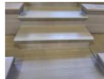
Treads & Risers Working From North to South Photo 5
