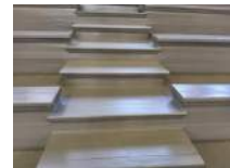
Treads & Risers Working From North to South Photo 6
