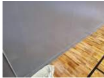
South Wall Photo 5 Darryl Dilmore Aug 30, 2022 11:33 AM
