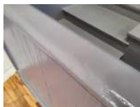
West Bleachers Photo 34 Darryl Dilmore Aug 30, 2022 11:03 AM
