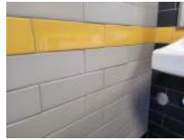
Women's Restroom Photo 23 Darryl Dilmore Aug 30, 2022 9:35 AM
