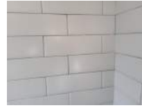
Men's Restroom 23 Darryl Dilmore Aug 30, 2022 9:56 AM
