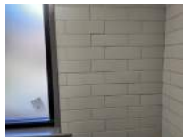
Women's Restroom Photo 7 Darryl Dilmore Aug 30, 2022 9:33 AM
