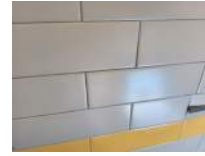
Men's Restroom 25 Darryl Dilmore Aug 30, 2022 9:56 AM
