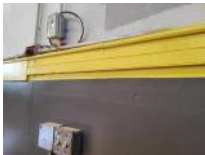
South Wall at West Bleachers 4 Darryl Dilmore Aug 30, 2022 11:05 AM
