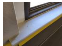
Wall at Top of West Bleachers From South to North Photo 10 Darryl Dilmore Aug 30, 2022 11:09 AM
