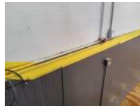
South Wall Photo 1 Darryl Dilmore Aug 30, 2022 11:32 AM
