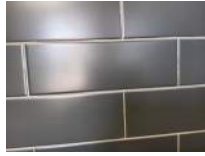
Women's Restroom Photo 16 Darryl Dilmore Aug 30, 2022 9:34 AM
