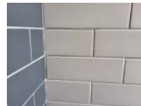
Women's Restroom Photo 13 Darryl Dilmore Aug 30, 2022 9:33 AM
