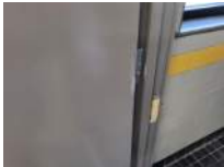
Women's Restroom Photo 1 Darryl Dilmore Aug 30, 2022 9:32 AM
