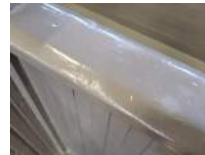
West Bleachers Photo 18 Darryl Dilmore Aug 30, 2022 11:01 AM
