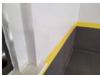
Wall at Top of West Bleachers From South to North Photo 36
