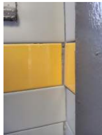
Men's Restroom 11 Darryl Dilmore Aug 30, 2022 9:54 AM
