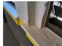
Wall at Top of West Bleachers From South to North Photo 34
