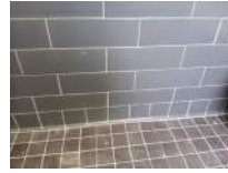
Women's Restroom Photo 19 Darryl Dilmore Aug 30, 2022 9:35 AM
