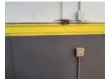
South Wall Photo 2 Darryl Dilmore Aug 30, 2022 11:32 AM
