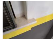
Wall at Top of West Bleachers From South to North Photo 5 Darryl Dilmore Aug 30, 2022 11:09 AM
