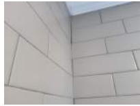
Men's Restroom 27 Darryl Dilmore Aug 30, 2022 9:56 AM
