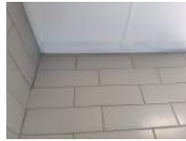
Men's Restroom 28 Darryl Dilmore Aug 30, 2022 9:56 AM
