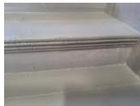
Treads & Risers Working From North to South Photo 2
