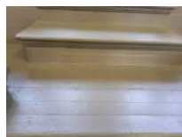
Treads & Risers Working From North to South Photo 9
