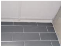
Women's Restroom Photo 24
