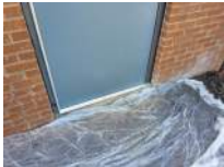
Door at Exterior Stair Photo 1
