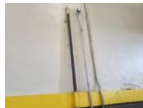
North Wall Photo 8 Darryl Dilmore Aug 30, 2022 11:25 AM
