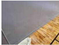
South Wall Photo 5 Darryl Dilmore Aug 30, 2022 11:33 AM
