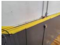
South Wall Photo 1
