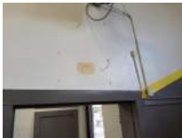
North Wall Photo 9
