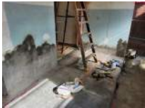
MS Auditorium Interior Access From Ramp Photo 3
