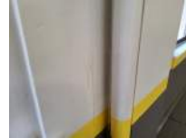
Wall at Top of West Bleachers From South to North Photo 22
