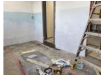
MS Auditorium Interior Access From Ramp Photo 2
