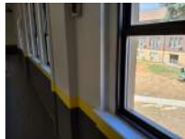
Wall at Top of West Bleachers From South to North Photo 25
