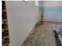
MS Auditorium Interior Access From Ramp Photo 1
