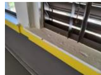
Wall at Top of West Bleachers From South to North Photo 33
