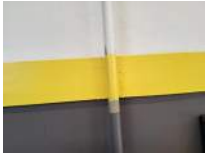
North Wall Photo 3
