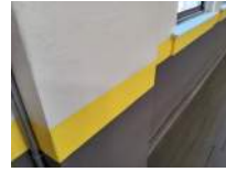
Wall at Top of West Bleachers From South to North Photo 15
