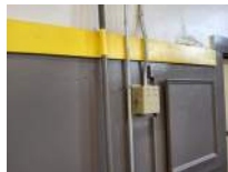
North Wall Photo 7 Darryl Dilmore Aug 30, 2022 11:25 AM
