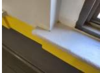
Wall at Top of West Bleachers From South to North Photo 18
