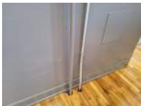
North Wall Photo 6 Darryl Dilmore Aug 30, 2022 11:25 AM
