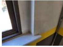
Wall at Top of West Bleachers From South to North Photo 13
