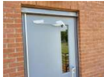
Door at Exterior Stair Photo 3
