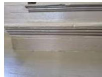
Treads & Risers Working From North to South Photo 4
