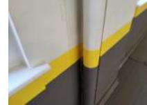
Wall at Top of West Bleachers From South to North Photo 23
