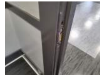
Mech Closet 5 Darryl Dilmore Aug 30, 2022 9:46 AM
