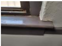
Mech Closet 14 Darryl Dilmore Aug 30, 2022 9:47 AM
