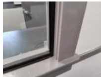
Women's Restroom Photo 28
