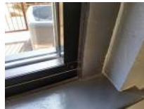
Lobby 33 Darryl Dilmore Aug 30, 2022 9:50 AM
