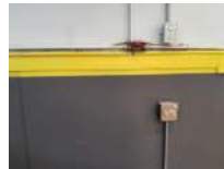
South Wall Photo 2
