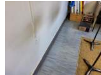
MS Auditorium Lobby Storage Photo 8 Darryl Dilmore Aug 30, 2022 12:05 PM
