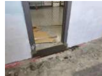
MS Auditorium Interior Access From Ramp Photo 5
