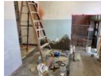
MS Auditorium Interior Access From Ramp Photo 4
