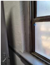
Mech Closet 20 Darryl Dilmore Aug 30, 2022 9:47 AM
