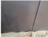
South Wall Photo 4 Darryl Dilmore Aug 30, 2022 11:32 AM
