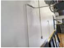
North Wall Photo 2
