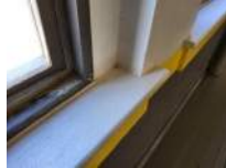
Wall at Top of West Bleachers From South to North Photo 19
