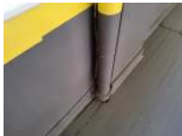
Wall at Top of West Bleachers From South to North Photo 24
