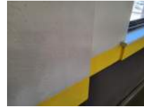
Wall at Top of West Bleachers From South to North Photo 16
