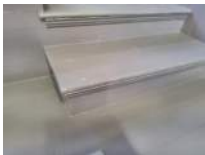
Treads & Risers Working From North to South Photo 1
