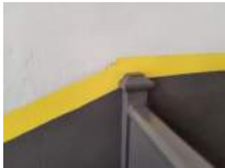
South Wall Photo 6
