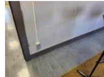
MS Auditorium Lobby Storage Photo 7 Darryl Dilmore Aug 30, 2022 12:05 PM
