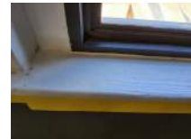
Wall at Top of West Bleachers From South to North Photo 29
