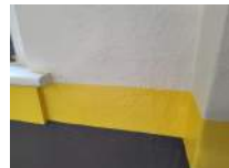
Wall at Top of West Bleachers From South to North Photo 32
