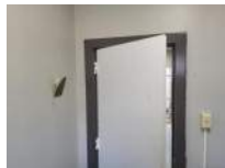
MS Auditorium Lobby Storage Photo 11 Darryl Dilmore Aug 30, 2022 12:05 PM
