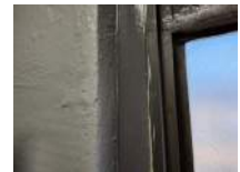
Mech Closet 19 Darryl Dilmore Aug 30, 2022 9:47 AM
