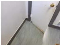
MS Auditorium Lobby Storage Photo 10 Darryl Dilmore Aug 30, 2022 12:05 PM
