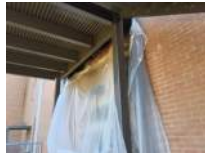
Exterior Stair Photo 8
