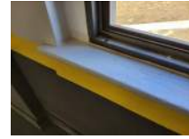
Wall at Top of West Bleachers From South to North Photo 17
