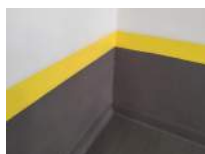
Wall at Top of West Bleachers From South to North Photo 37
