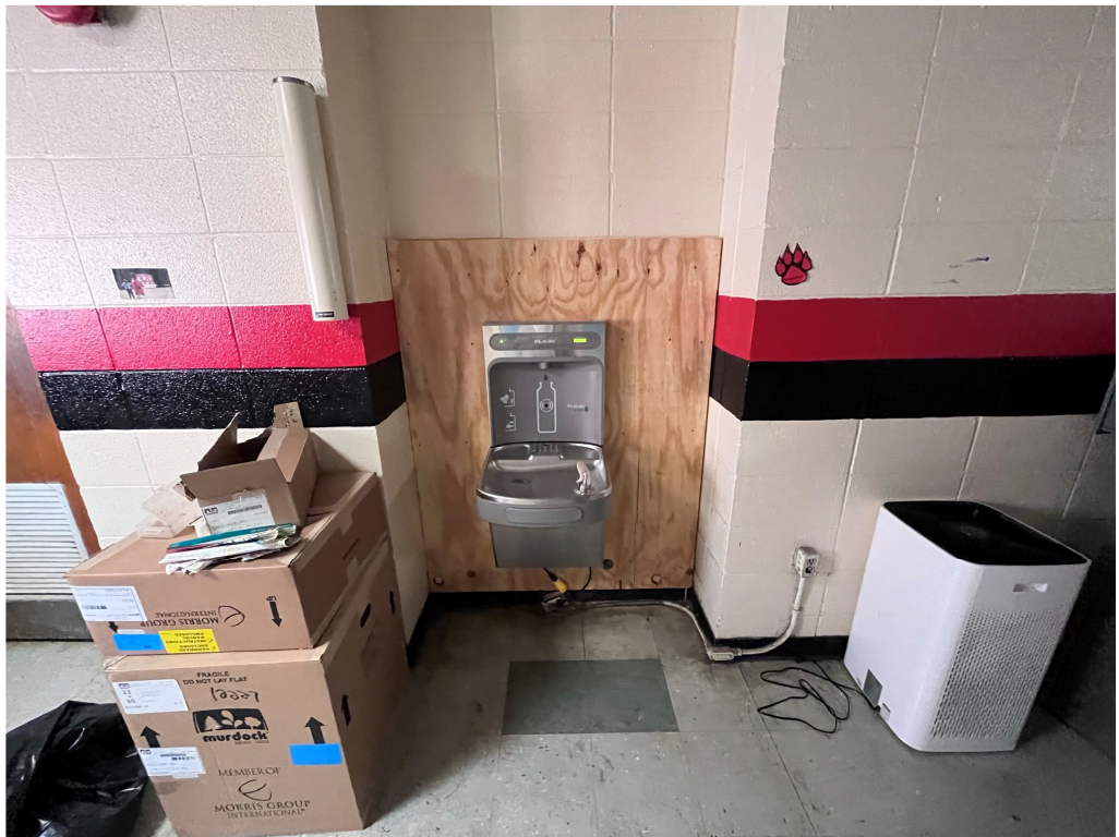
Figure 4 – New Fountain Work at Leflore County
