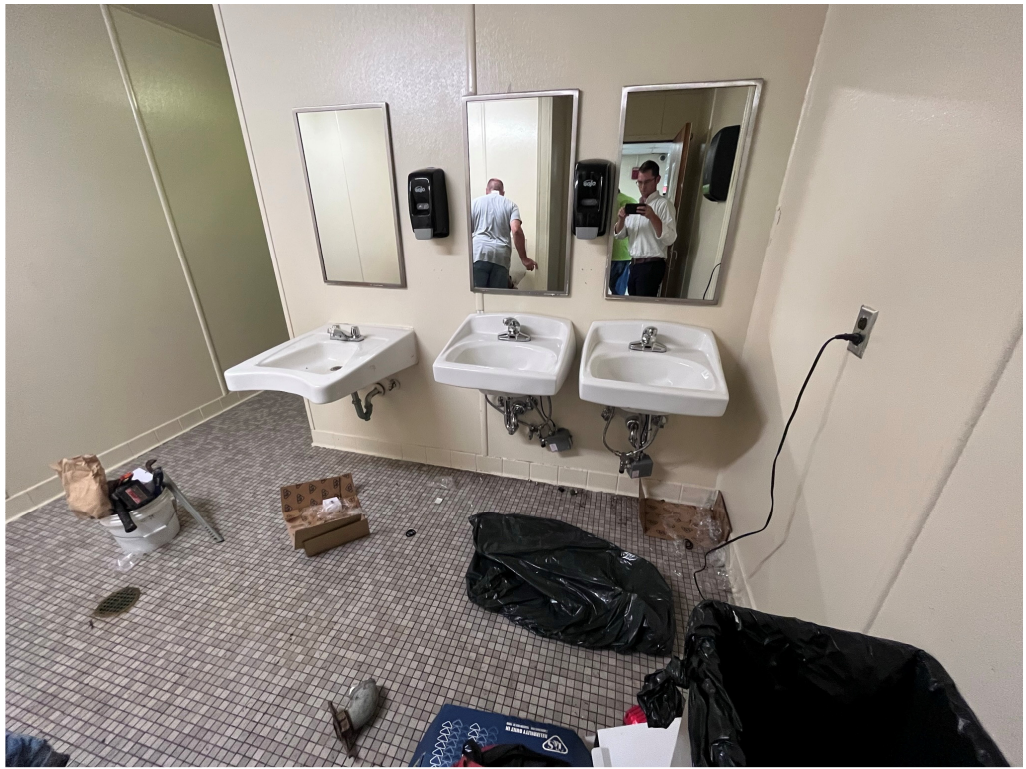
Figure 1 – Contractor on site at Leflore County
