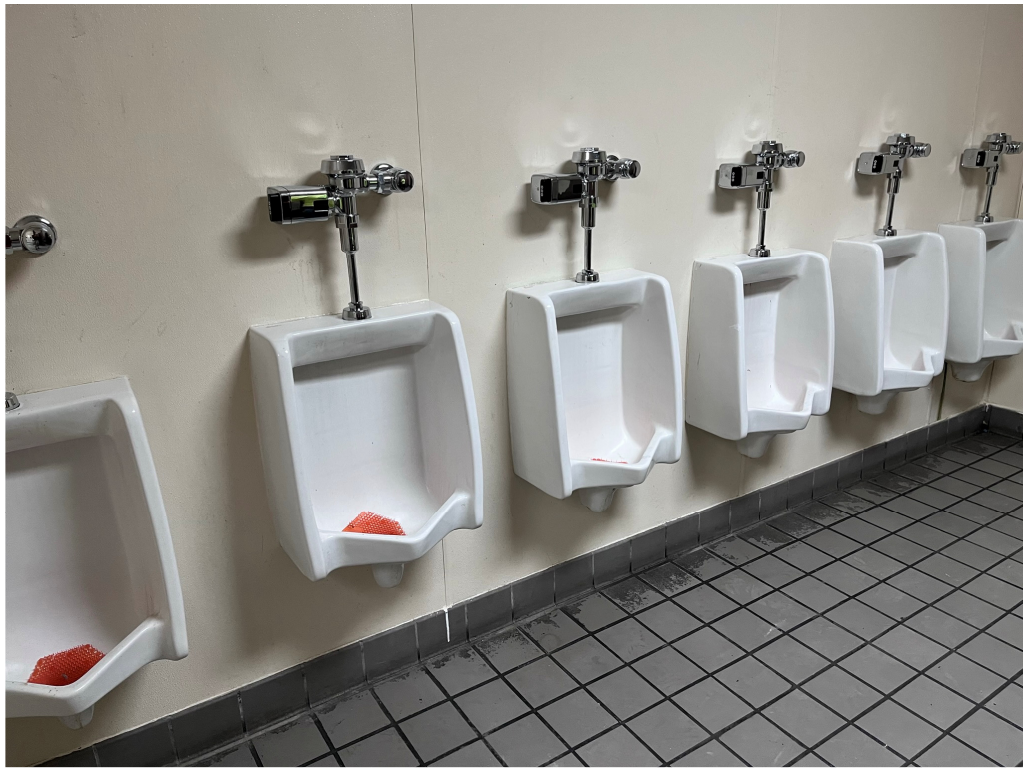
Figure 5 – Flush Valves Changed out at Leflore County
