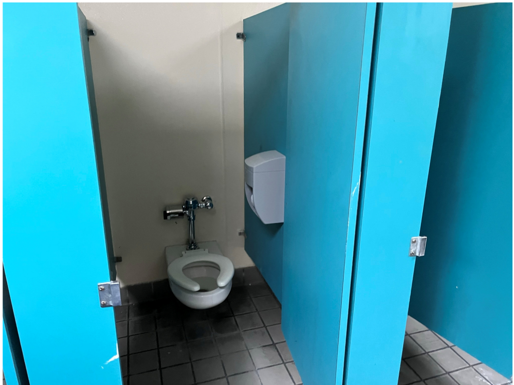
Figure 6 – Flush Valves Changed out at Leflore County
