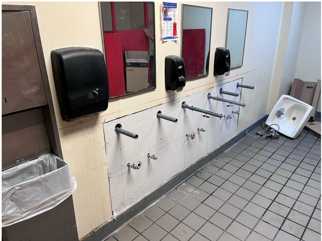
Figure 4 – New Lavatory Work at Leflore County
