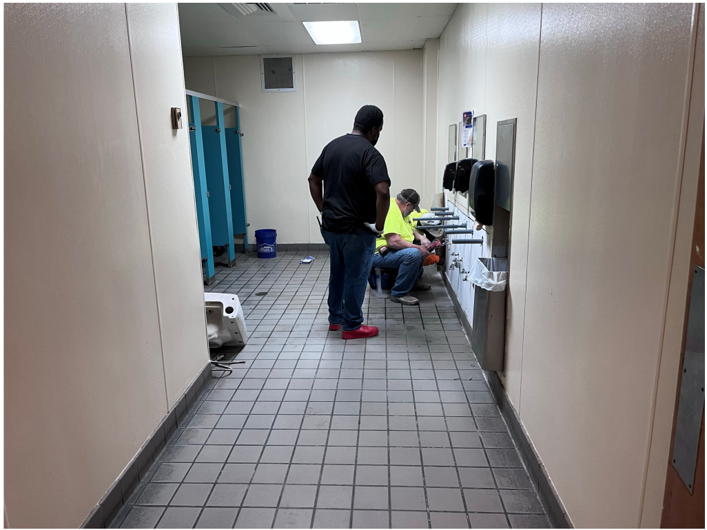
Figure 3 – New Lavatory Work at Leflore County
