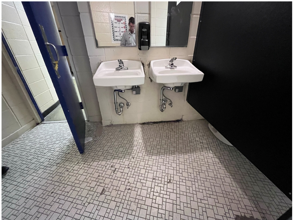
Figure 4 – New work still requires Pipe Padding
