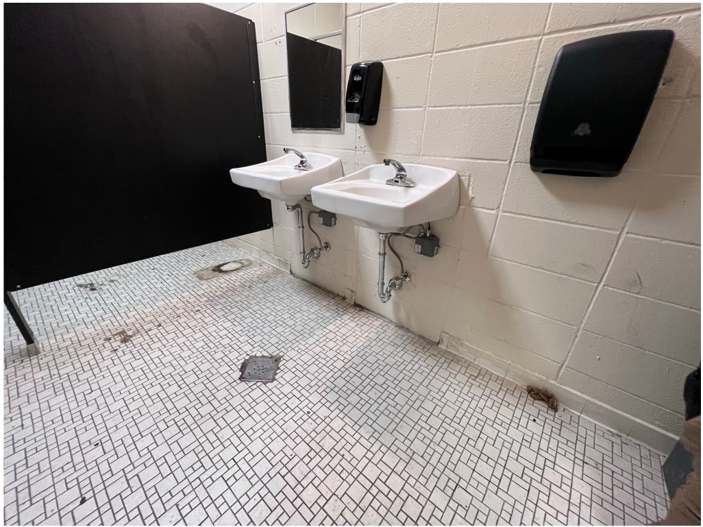
Figure 1 – Work at East Elementary is ongoing
