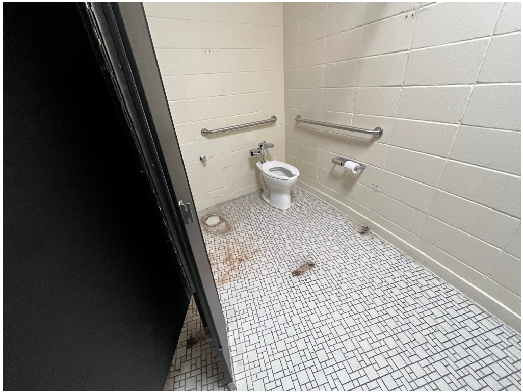
Figure 5 – New ADA Sized Toilet
