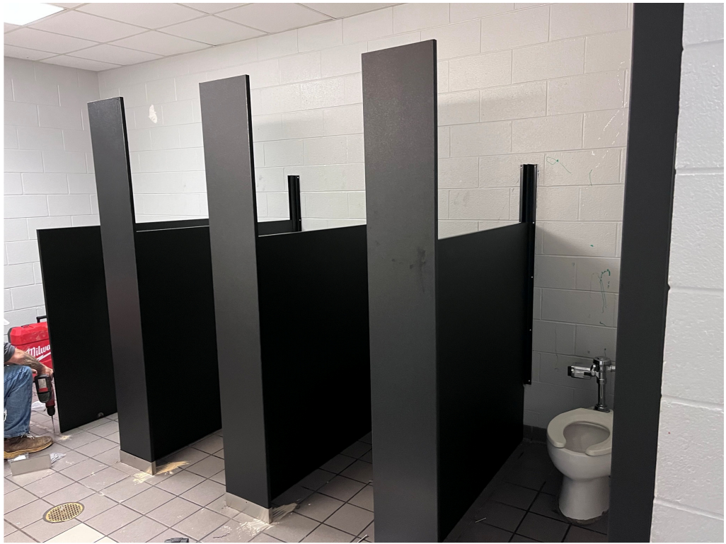
Figure 11 – Partition installation, starting at Greenwood Middle
