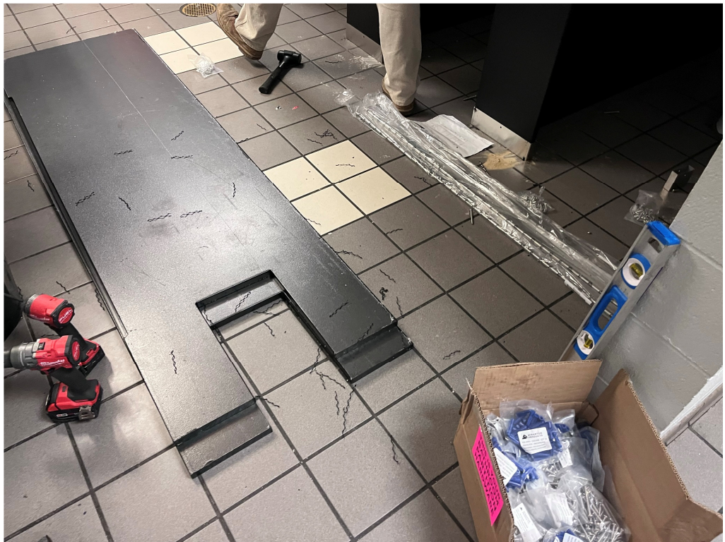
Figure 12 – Partition installation, starting at Greenwood Middle
