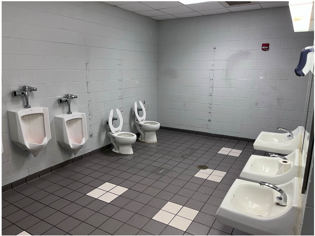
Figure 9 – Partitions removed at Greenwood Middle
