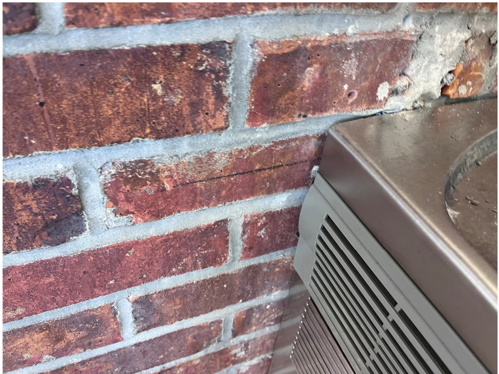
Figure 6 – Remove any construction markings
