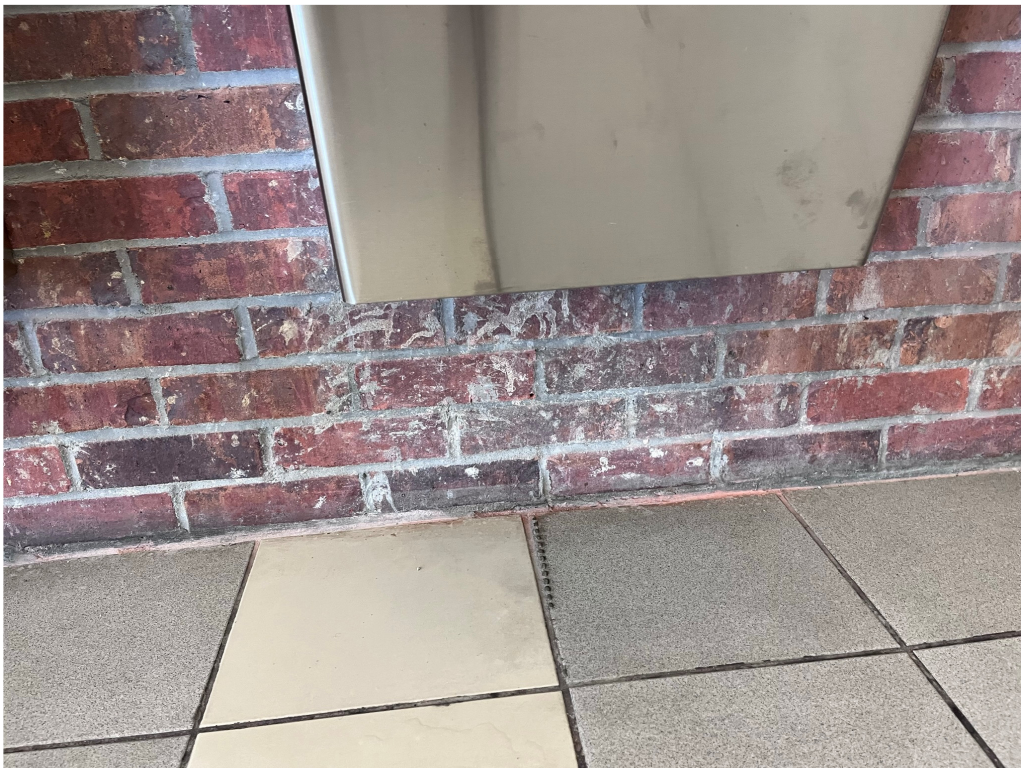
Figure 8 – Masonry dust from installation needs to be removed from brick face
