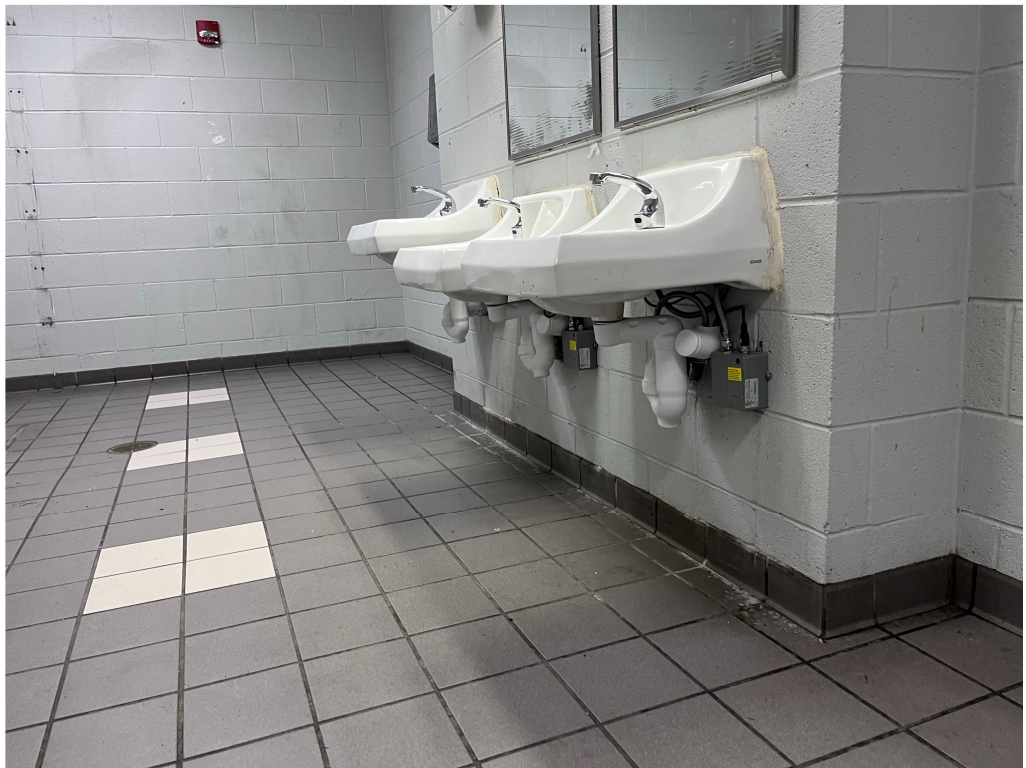
Figure 10 – Insulation Installed at Greenwood Middle
