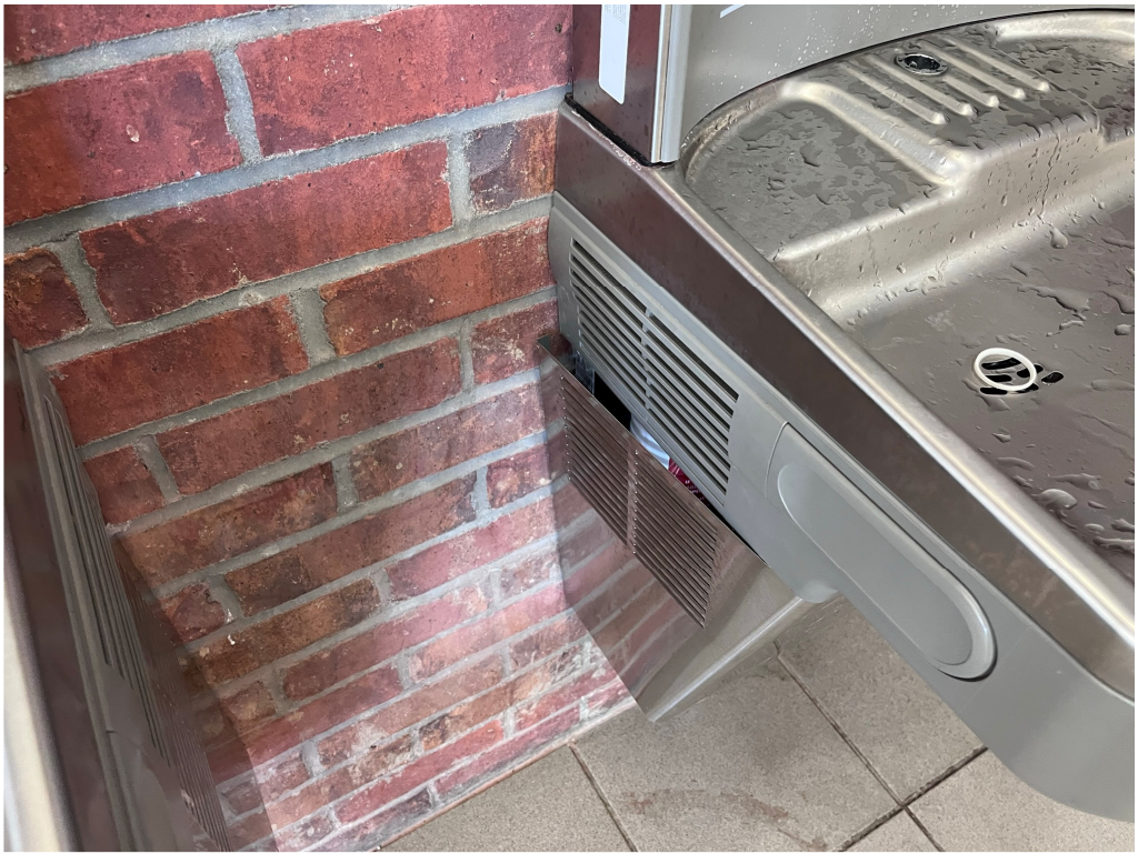
Figure 7 – Ensure that covers are fully secured
