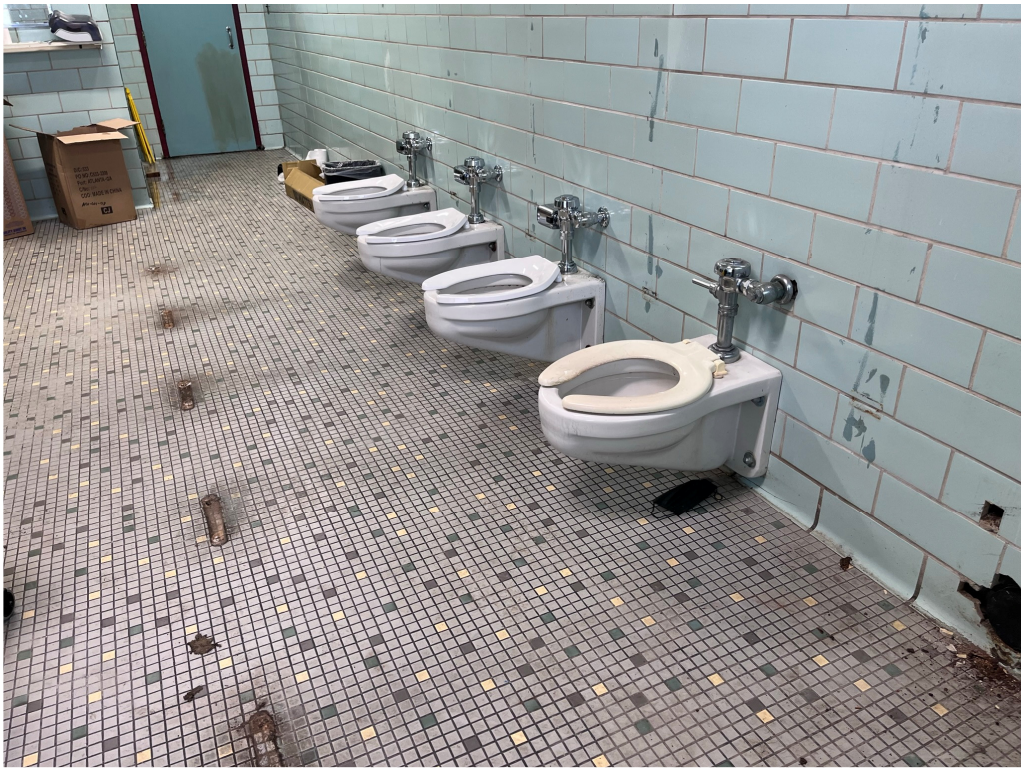
Figure 7 – GHS Plumbing work and Partition Demo
