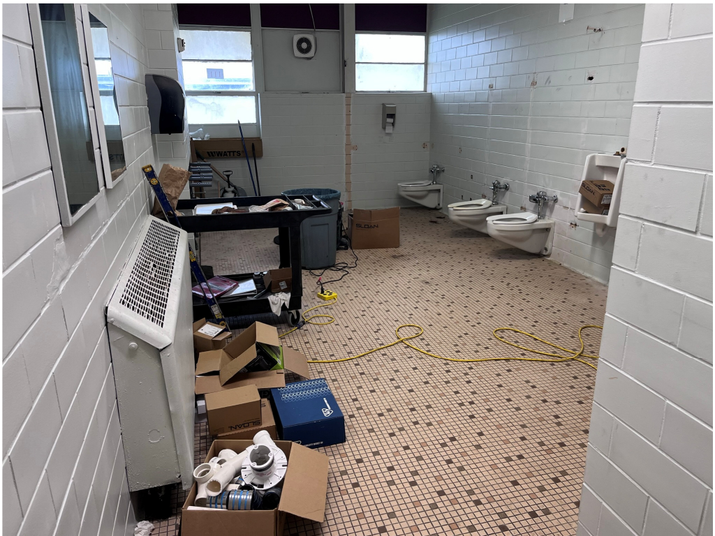
Figure 2 – GHS work is ongoing
