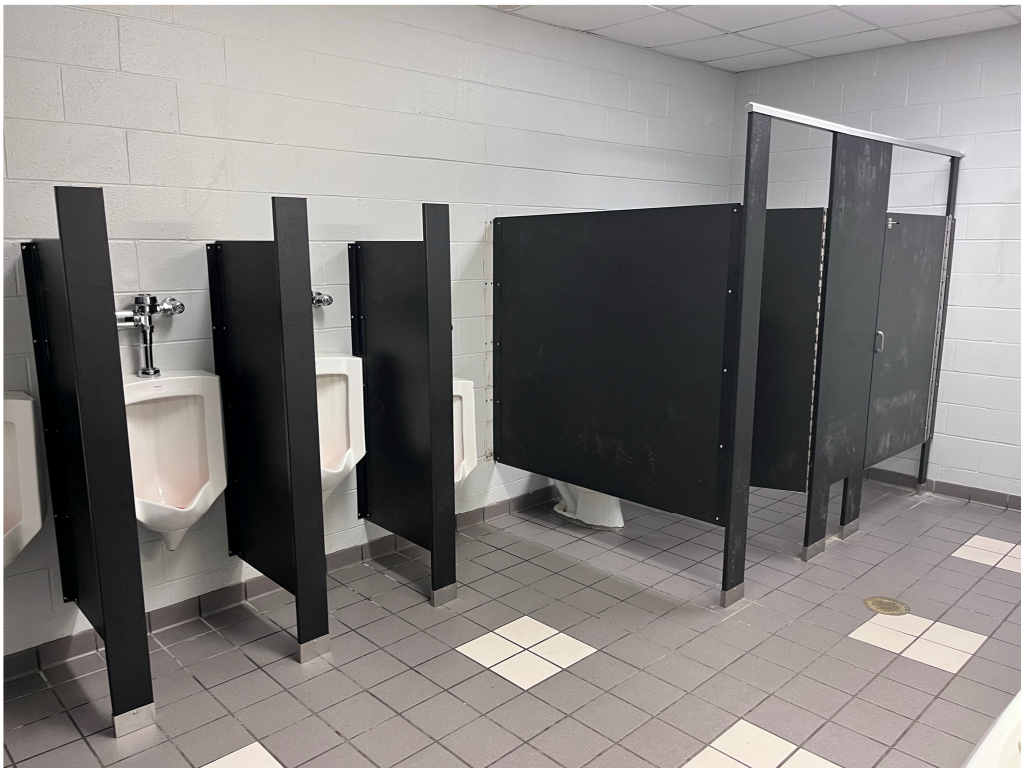
Figure 8 – GMS Partitions Installed
