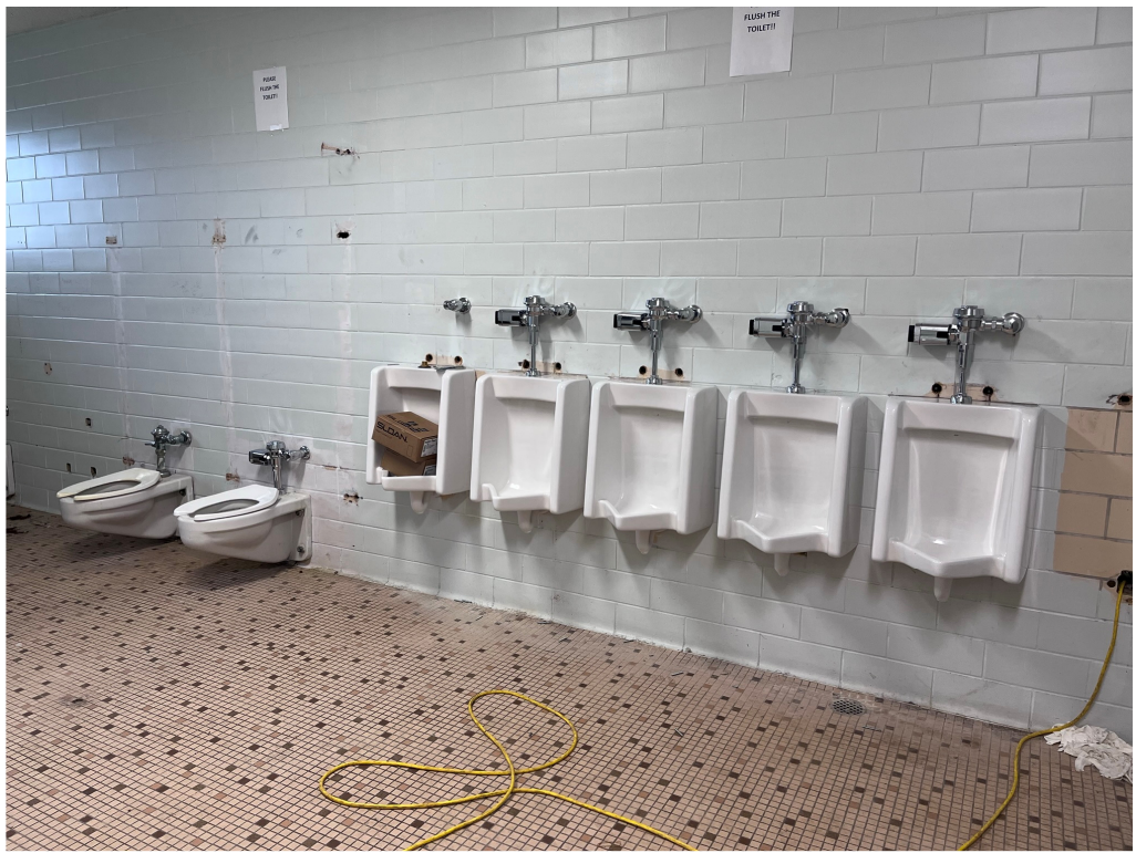
Figure 3 – GHS New Valve Install
