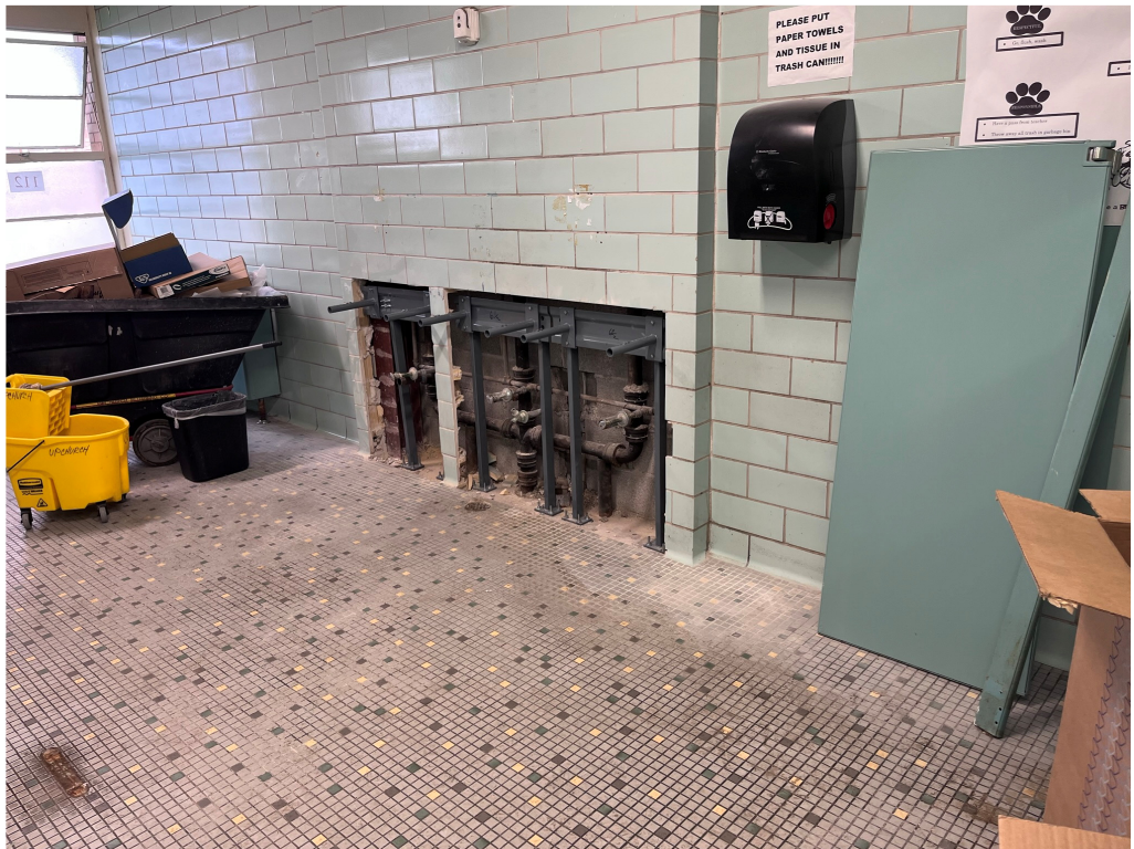
Figure 6 – GHS Plumbing work and Wall Demo
