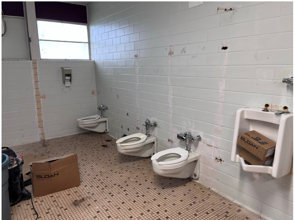
Figure 4 – GHS Plumbing Demo
