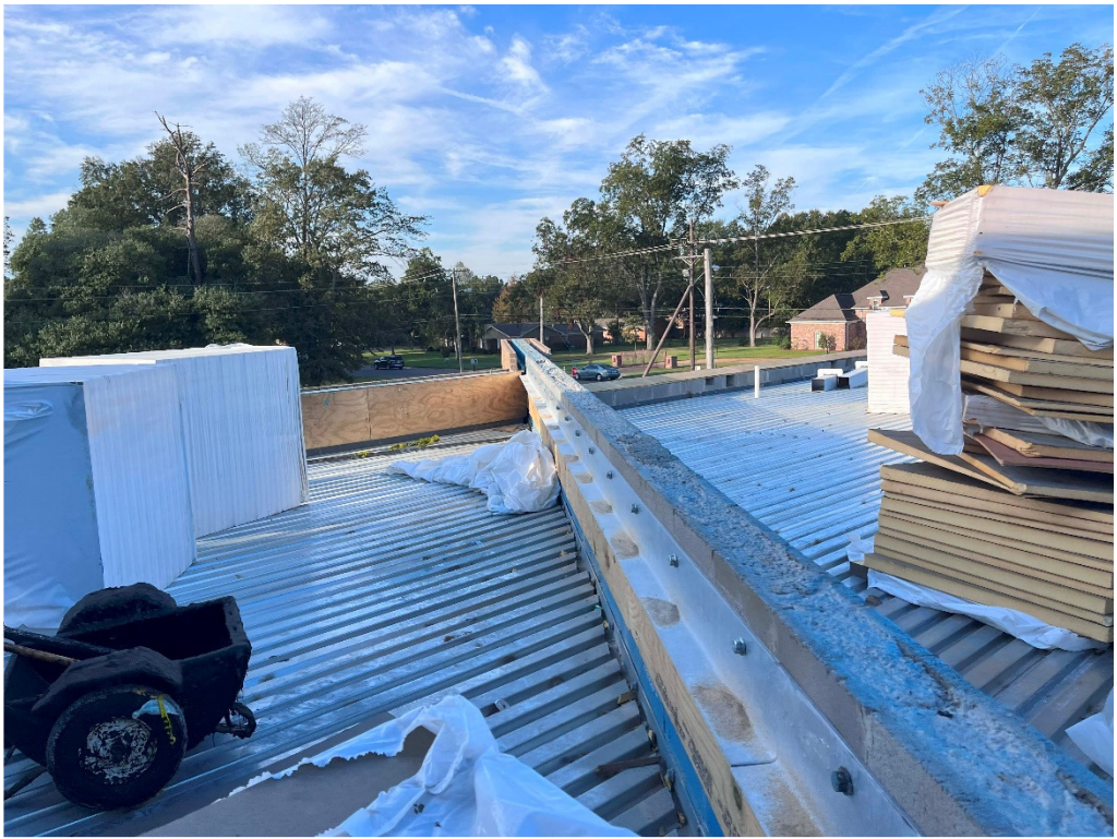
Figure 15 – GHS: roof top progress
