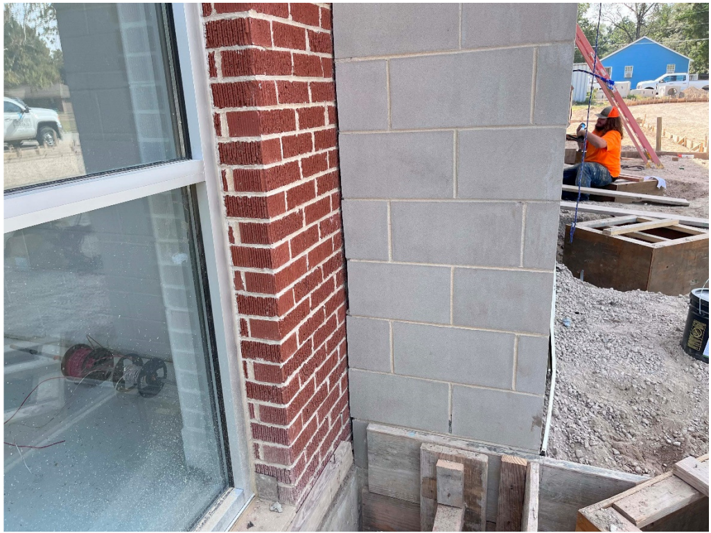
Figure 31 – TEHS: Joints Awaiting Sealant Installation
