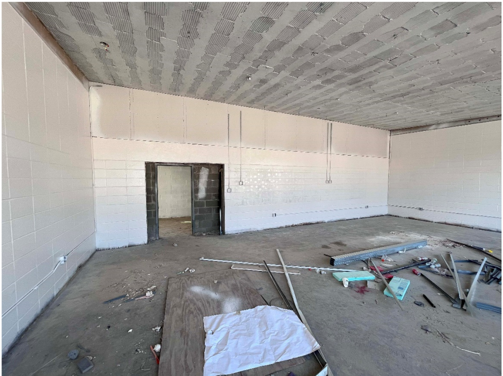
Figure 20 – GHS: Typical north classroom progress
