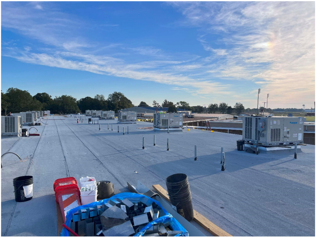
Figure 7 – GHS: diagonal hall roof progress
