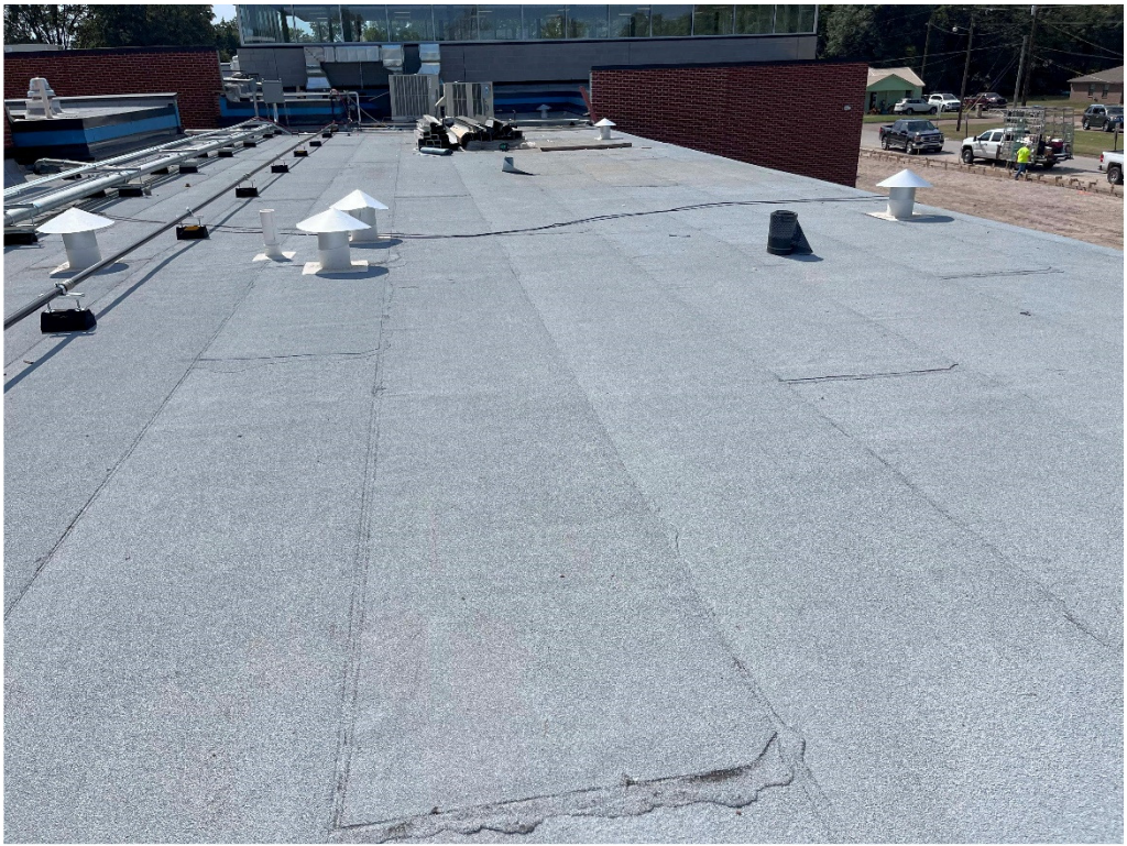
Figure 45 – TEHS: roof progress noted
