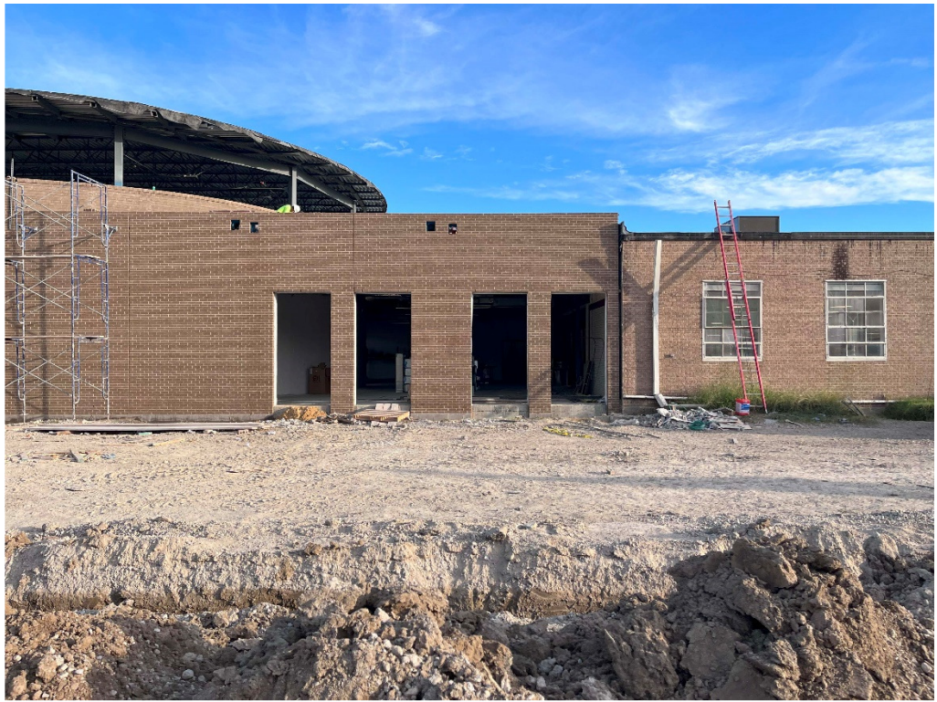
Figure 1 – GHS: new brick installation
