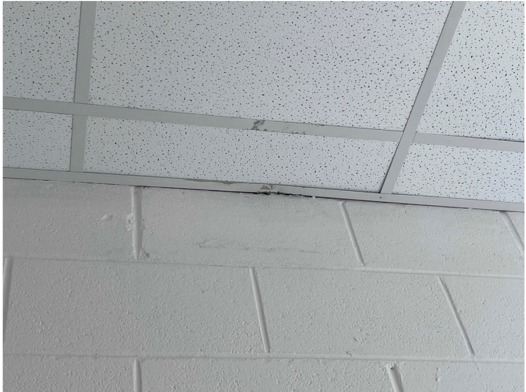
Figure 35 – TEHS: contractor is reminded to that all new ceiling installation shall be new and without deformation or discoloring
