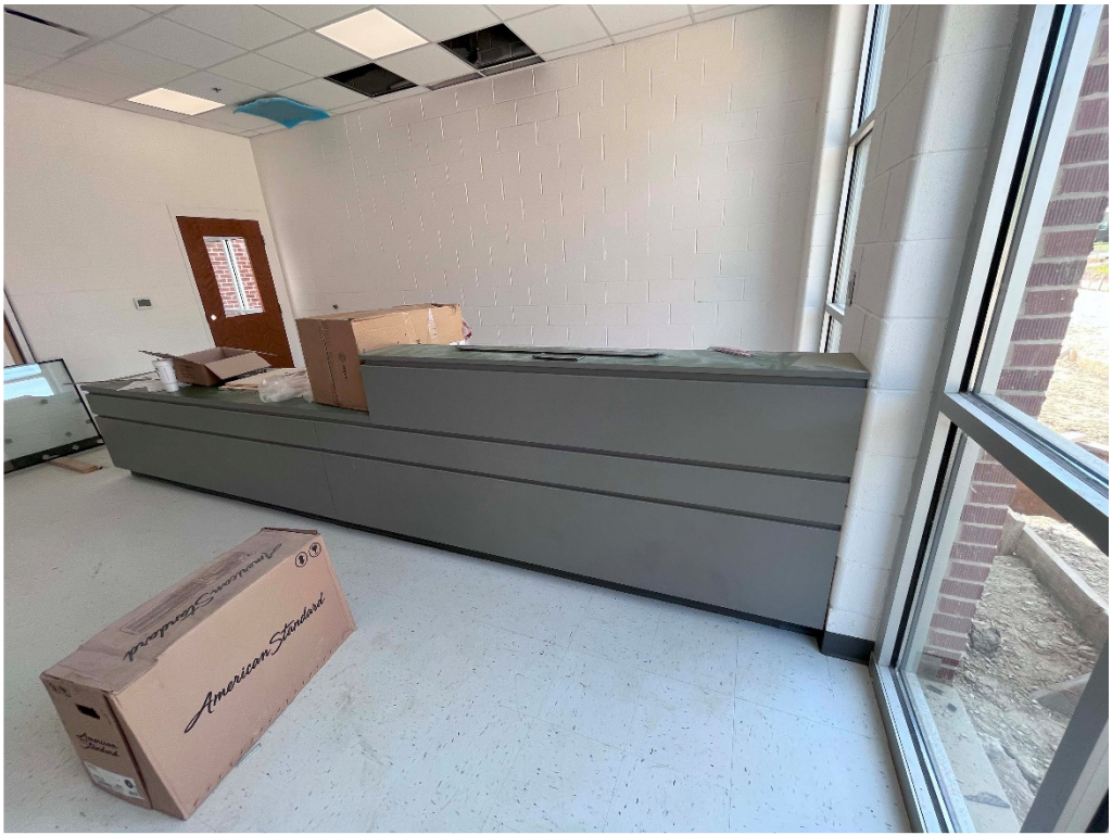
Figure 33 – TEHS: millwork installed
