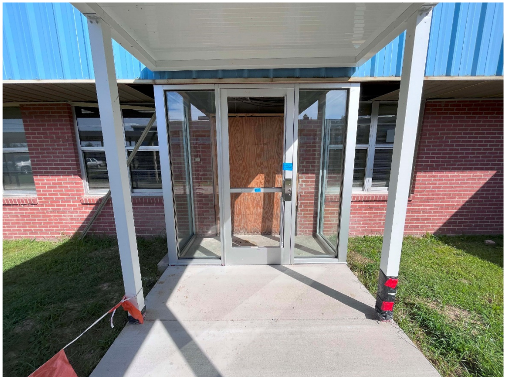
Figure 26 – Merrit Middle: progress at Merrit Middle Entry
