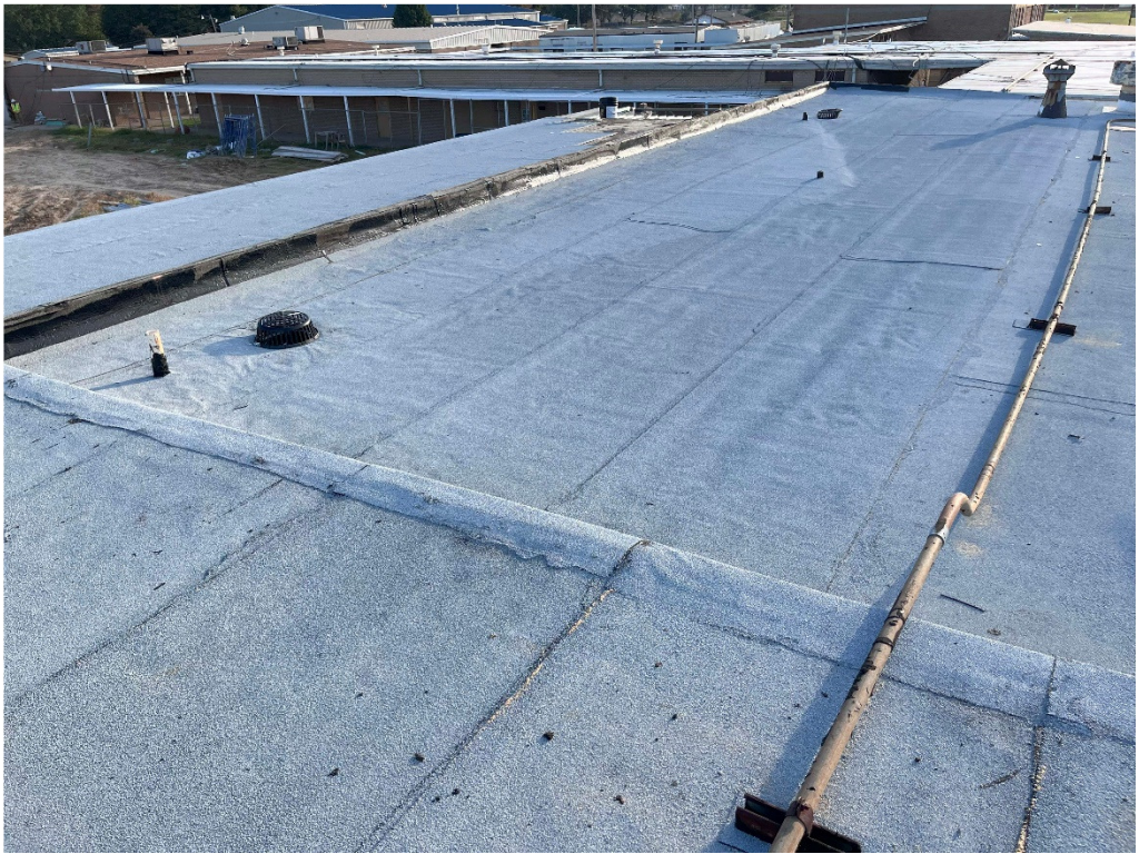
Figure 4 – GHS: progress at cafeteria roof
