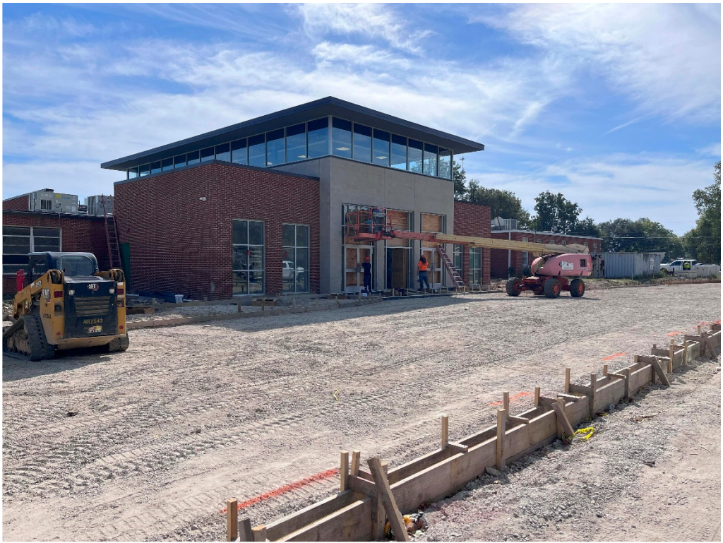
Figure 27 – TEHS: progress at front entry; glass install in progress
