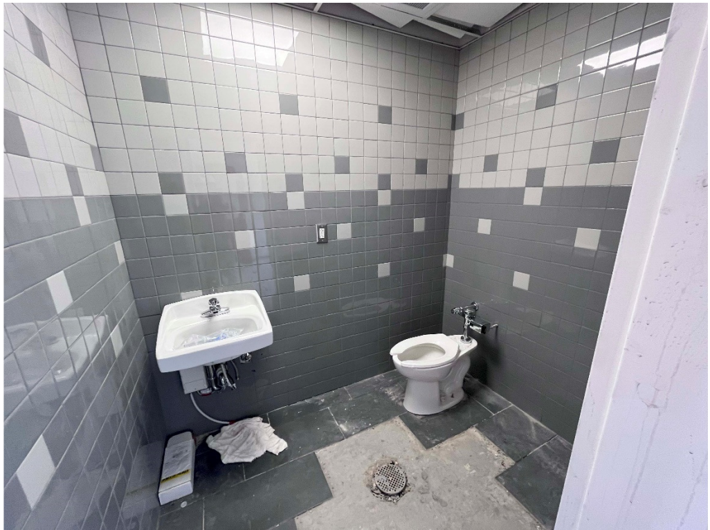
Figure 37 – TEHS: progress at toilets rooms noted
