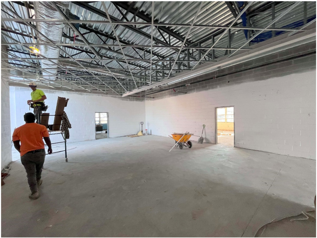
Figure 19 – GHS: NE end of diagonal hall
