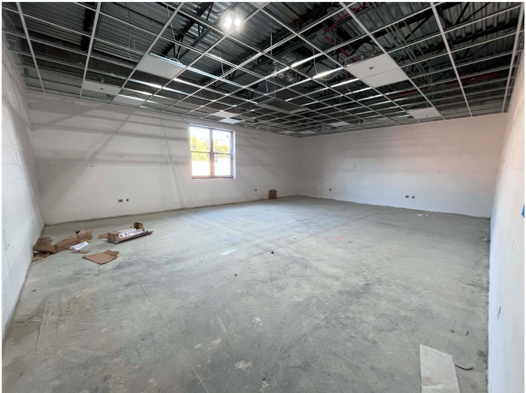
Figure 18 – GHS: typical classroom at diagonal hall progress
