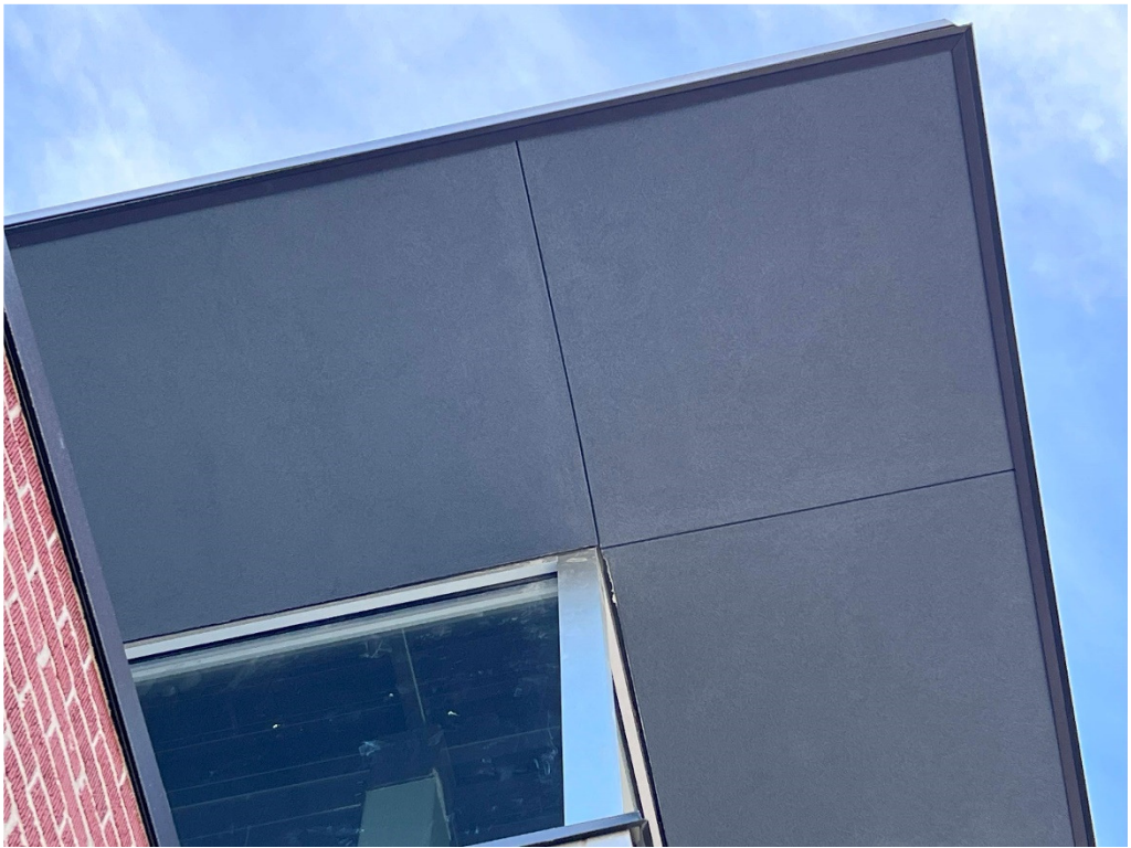
Figure 28 – TEHS: stucco installed
