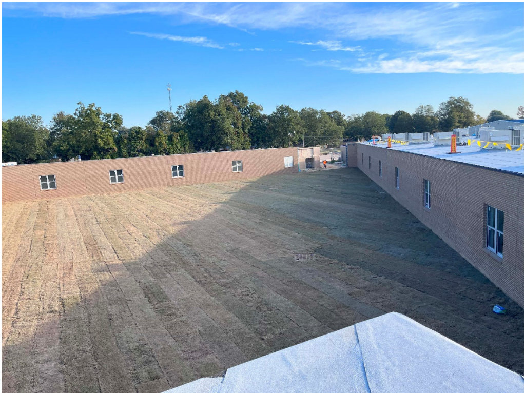
Figure 11 – GHS: NW exterior courtyard progress
