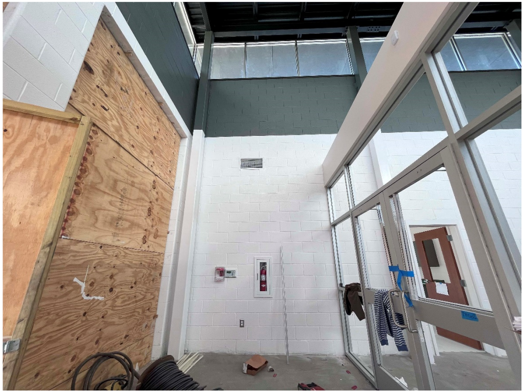
Figure 32 – TEHS: secure vestibule progress
