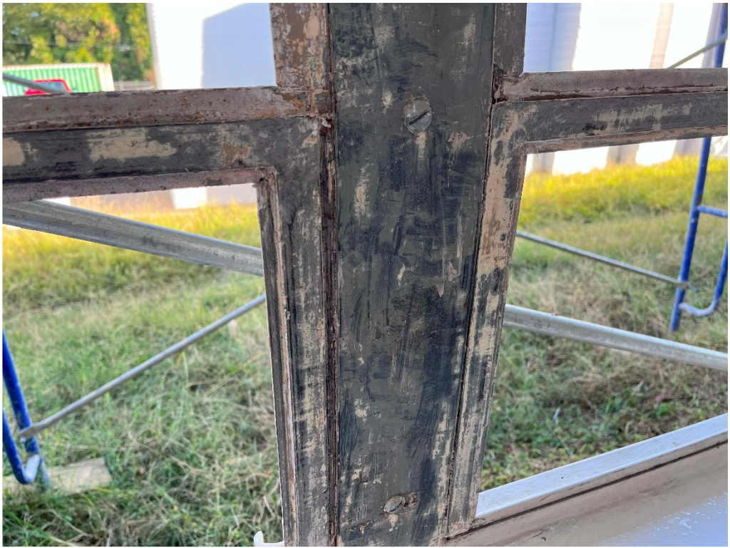
Figure 21 – GHS: progress at window restoration at north hall
