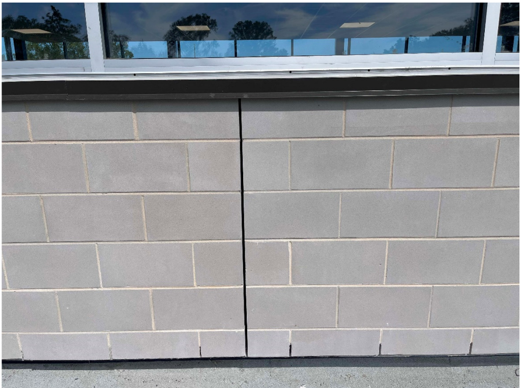
Figure 48 – TEHS: Joints Awaiting Sealant Installation
