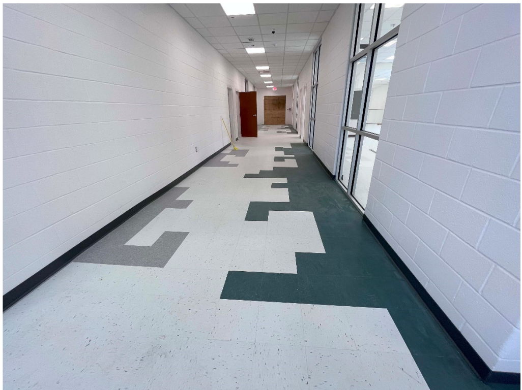
Figure 40 – TEHS: VCT progress noted at corridors
