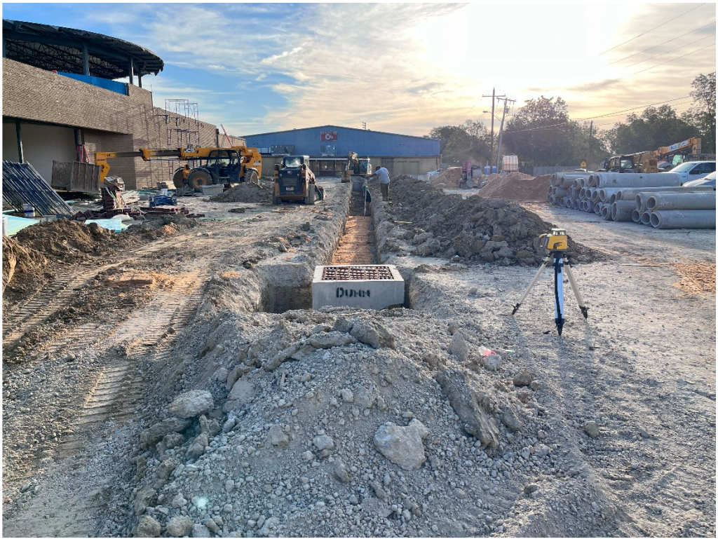
Figure 3 – GHS: subdrainage work at parking
