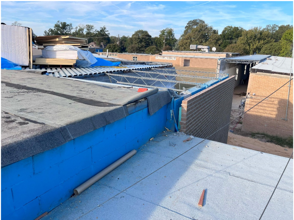
Figure 10 – GHS: roof progress at NE campus corner
