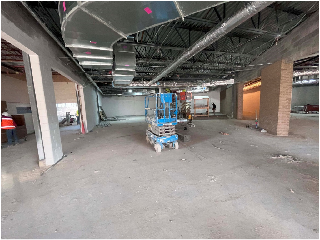
Figure 17 – GHS: front lobby, where discussed lowered ceiling may be required
