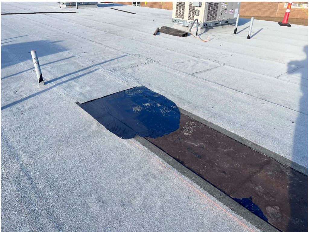
Figure 8 – GHS: roof progress to NE campus corner
