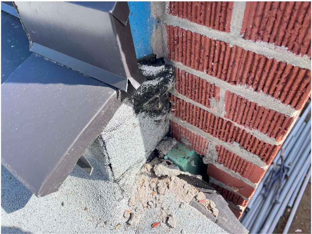
Figure 44 – TEHS: provide flashing and sealants over open wall cavity
