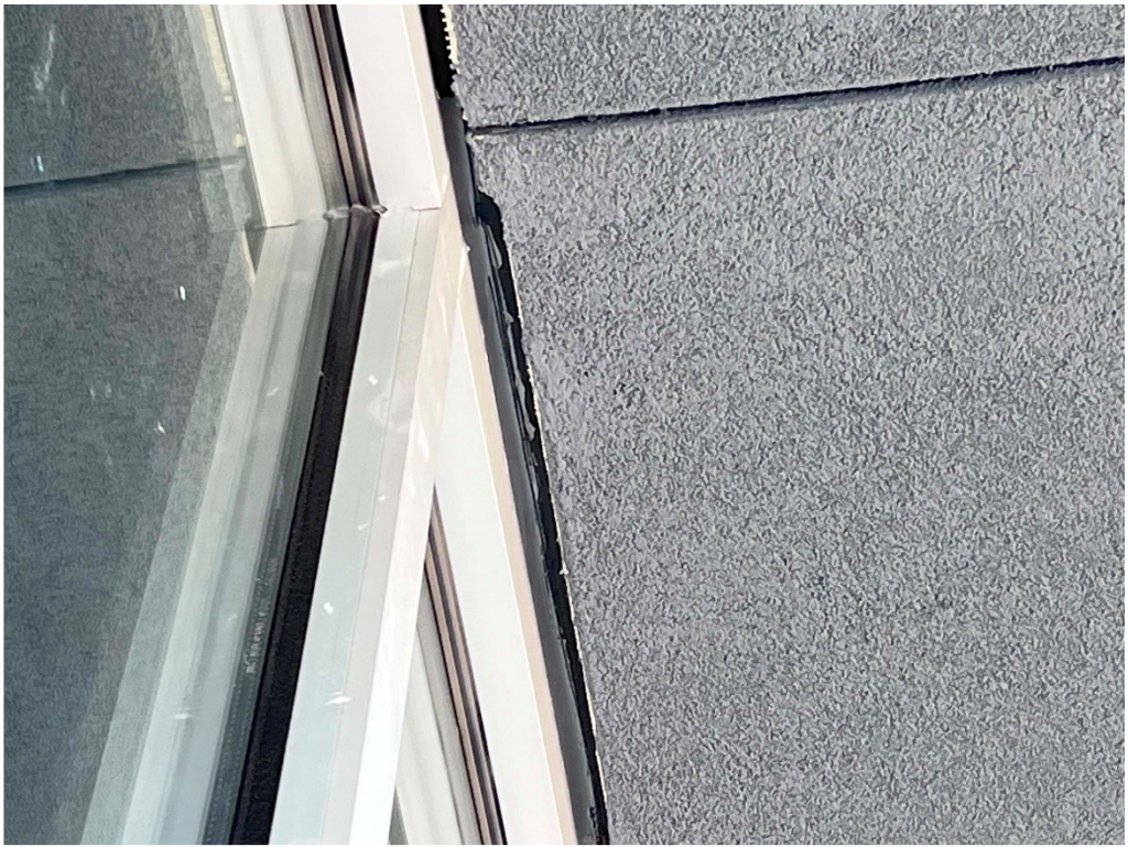
Figure 29 – TEHS: Joints Awaiting Sealant Installation
