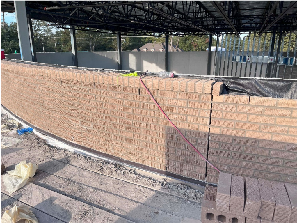
Figure 12 – GHS: Brick work at roof top
