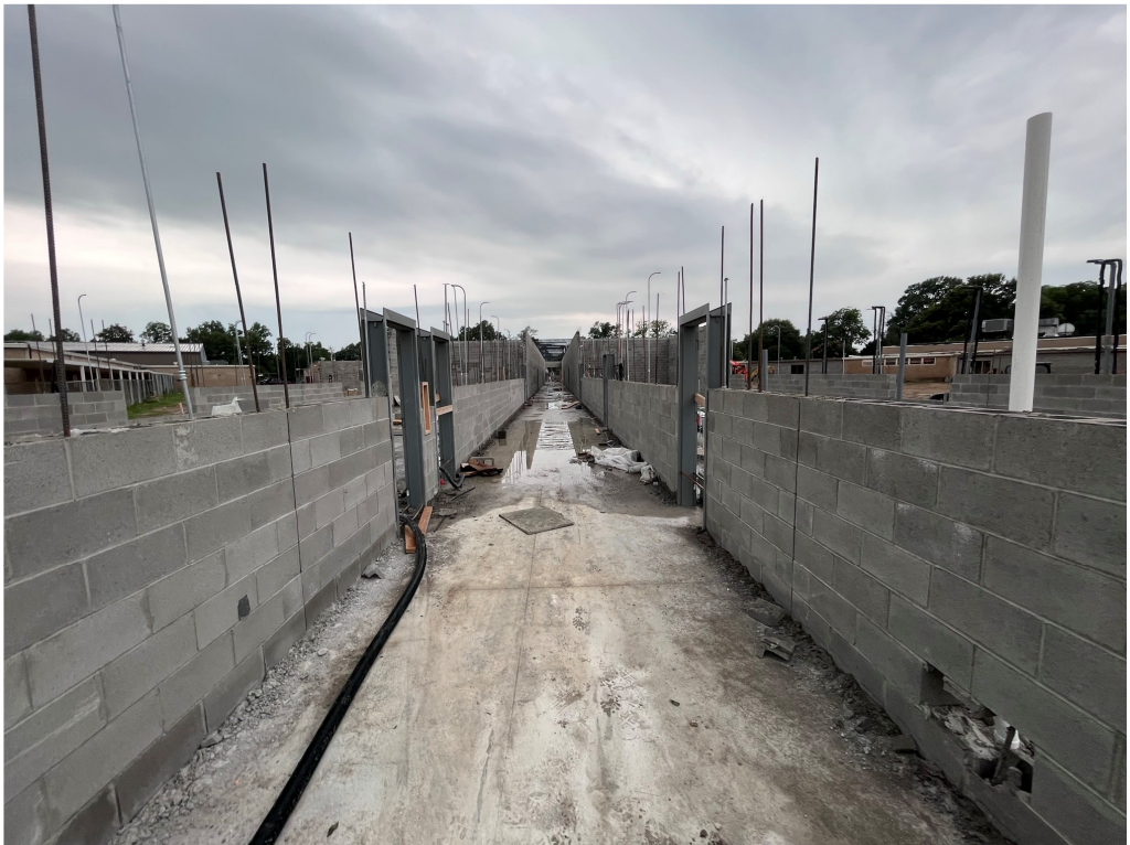
Figure 8 – GHS NE Hall Looking SW
