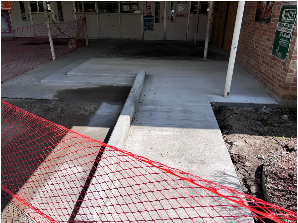
Figure 20 – AW James Concrete for Secure Vestibule
