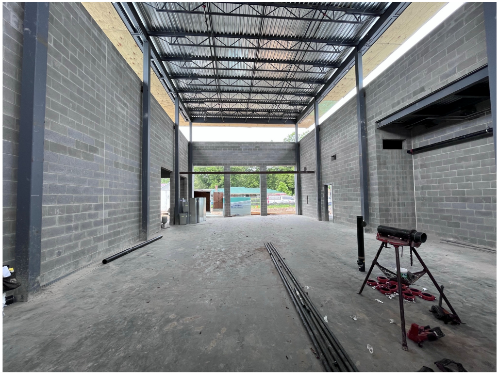
Figure 15 – TEHS Progress at Lobby
