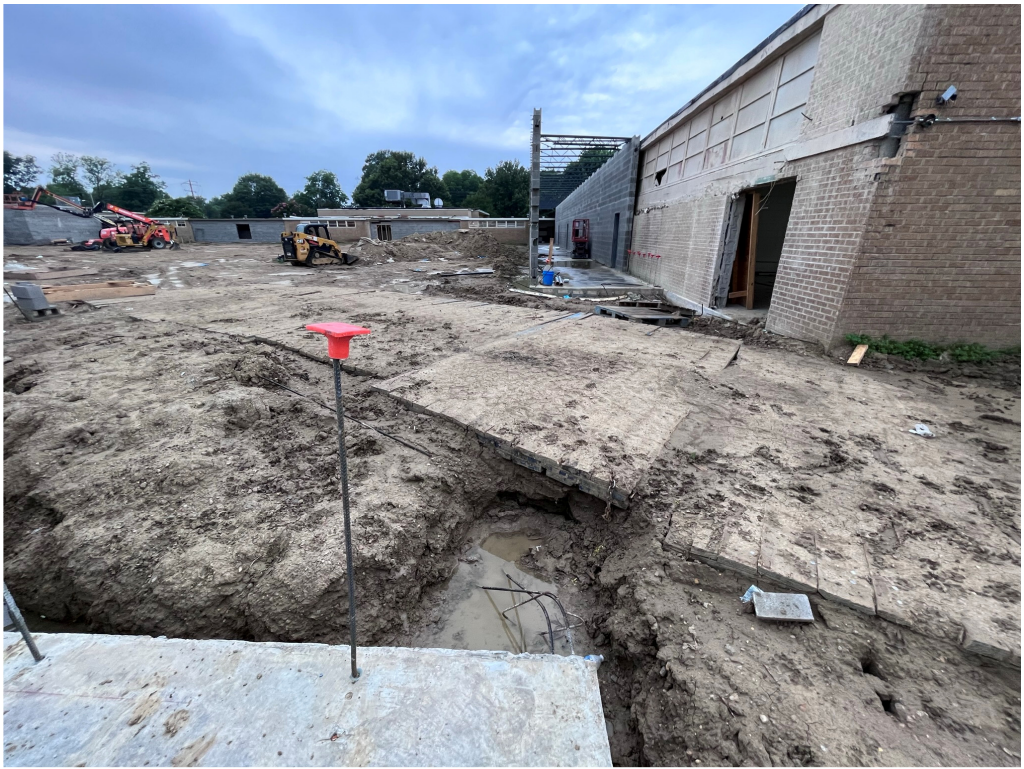
Figure 11 – GHS Construction Mats for Heavy Equipment are Temporary
