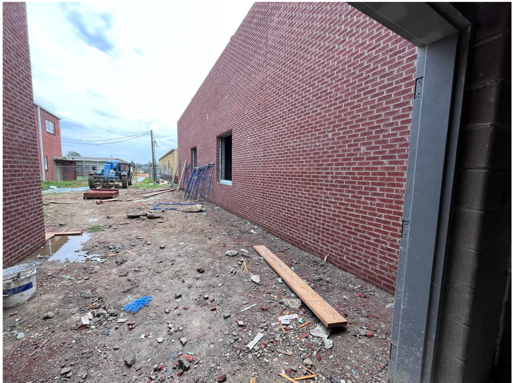
Figure 16 – TEHS Brick work @ Addition Rear
