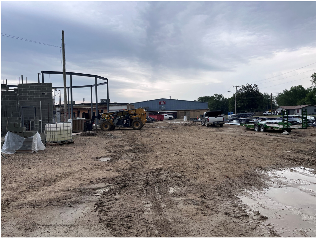
Figure 1 – GHS SW Exterior and Parking
