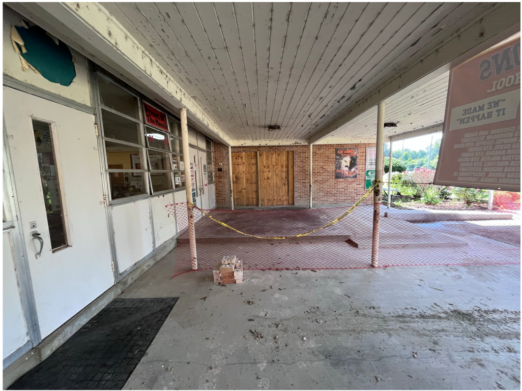
Figure 21 – AW James Concrete for Secure Vestibule
