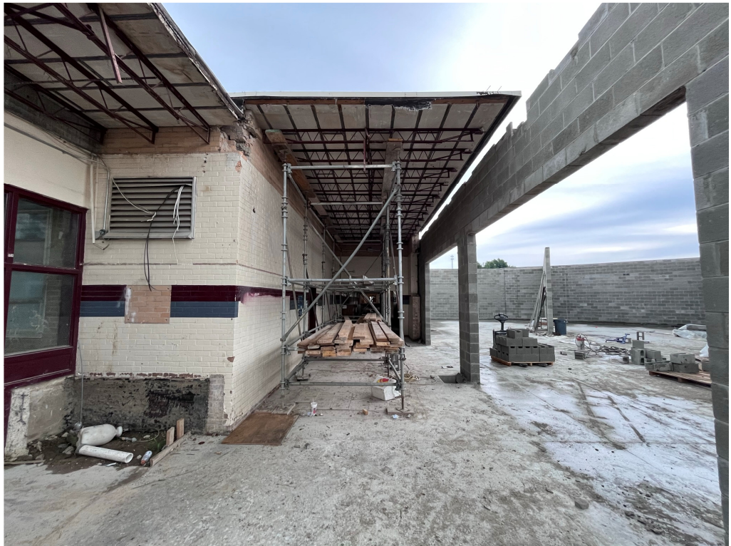
Figure 4 – GHS SW Lobby at Existing Admin Connection to New
