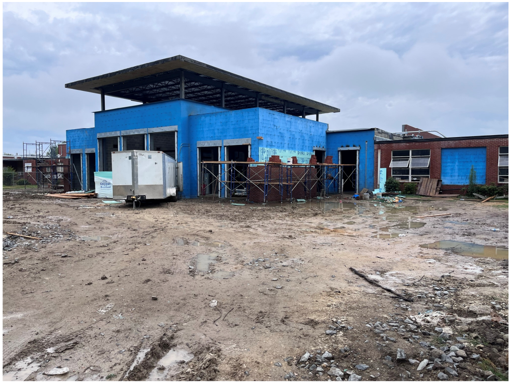
Figure 13 – TEHS Front of Site
