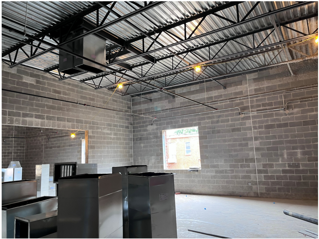
Figure 17 – TEHS HVAC Roof Ducting Set in Place
