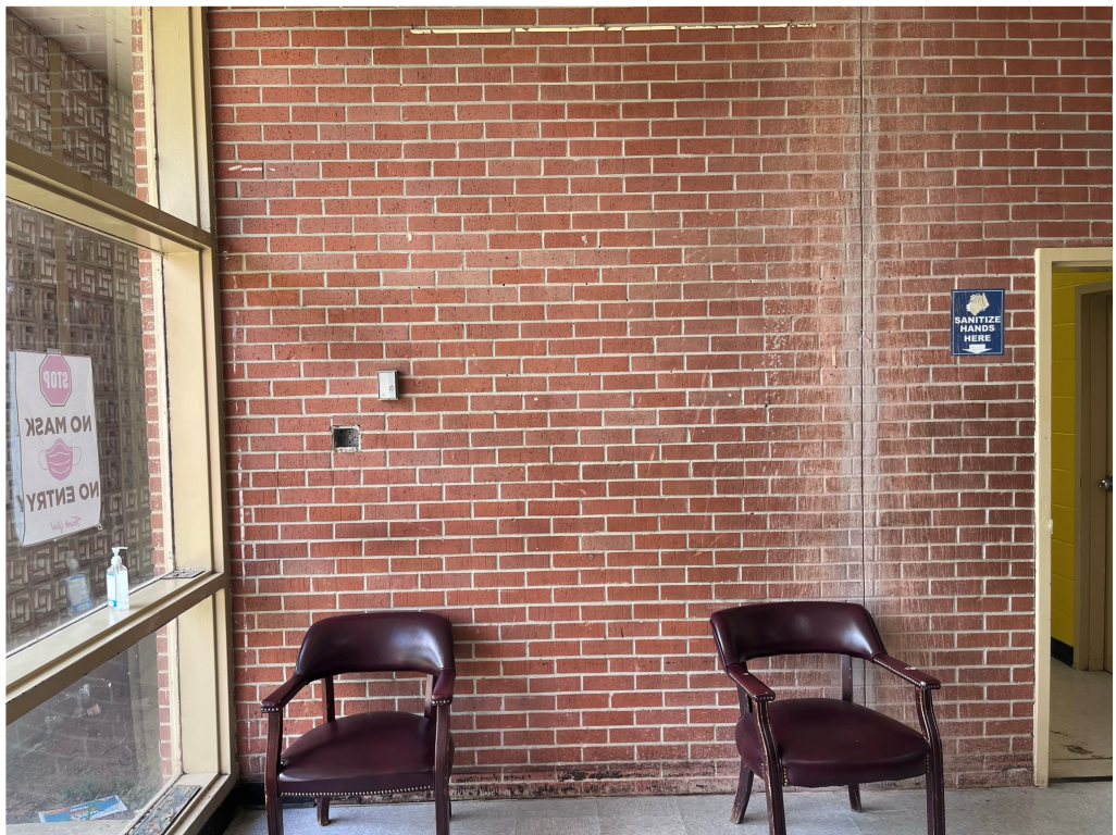
Figure 24 – RMS Demo Started at Secure Vestibule Interior
