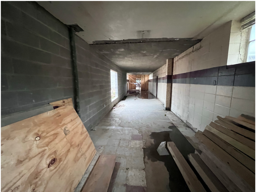
Figure 12 – GHS West Existing Hall Progress
