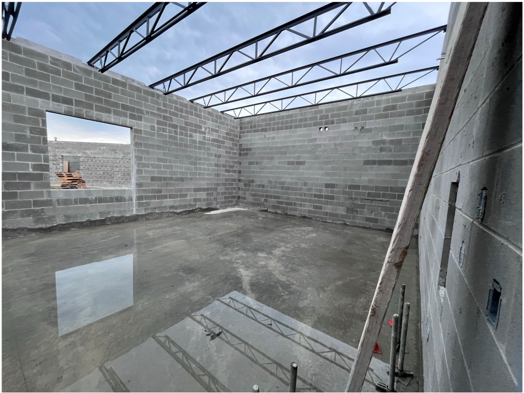
Figure 6 – GHS Steel Supports Set in Classrooms
