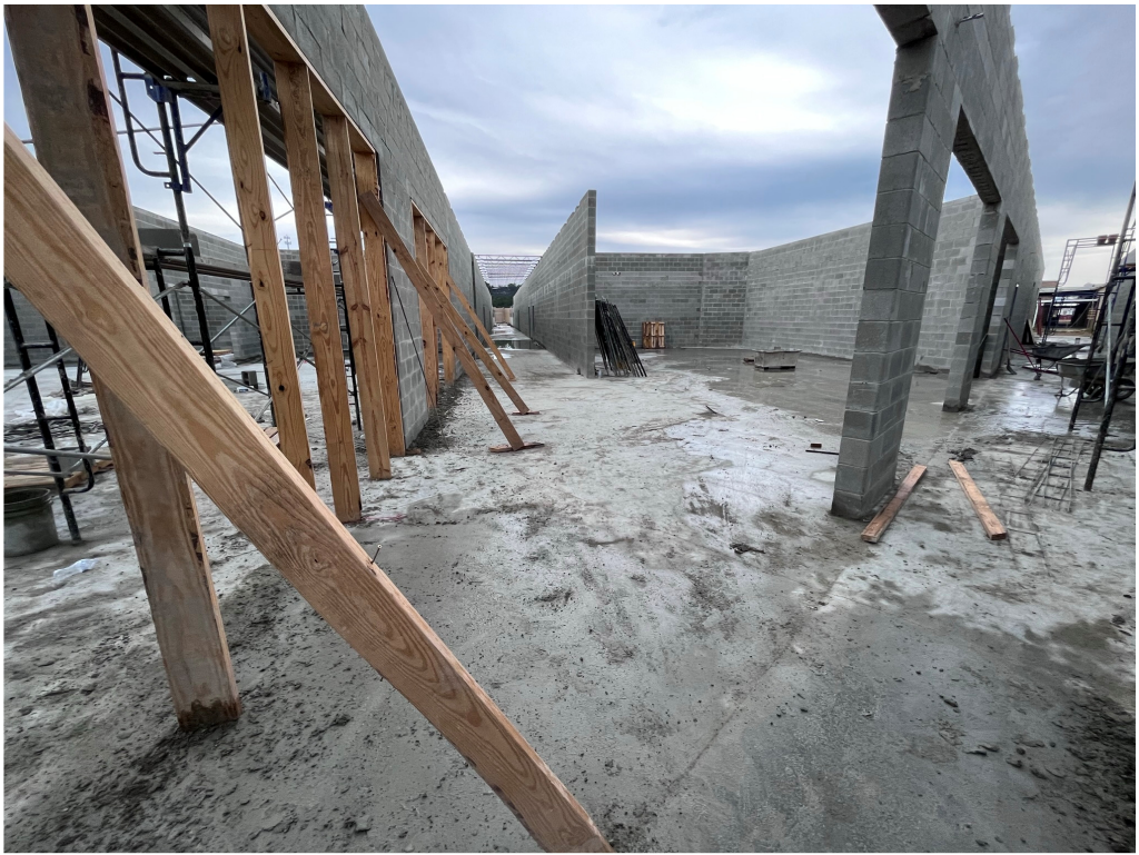
Figure 5 – GHS SW Lobby Looking NE
