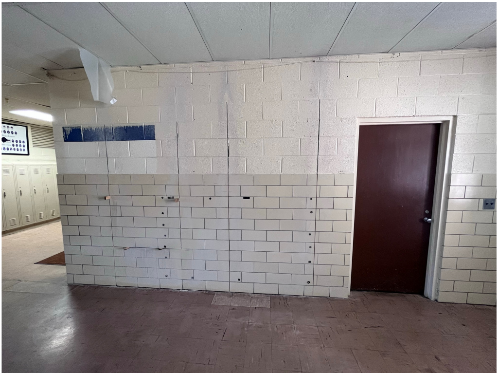
Figure 19 – Drew Hunter Demo Work Started for Secure Vestibules
