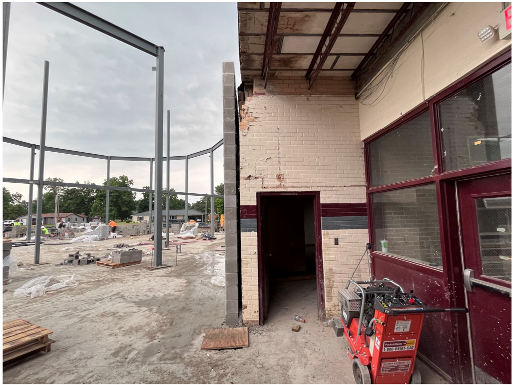
Figure 3 – GHS SW Lobby at Existing Admin Connection to New
