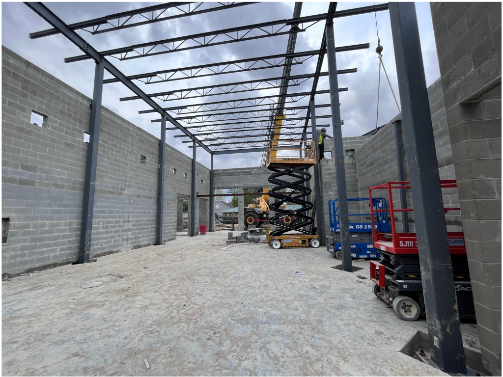
Figure 8 – TEHS Steel Setting
