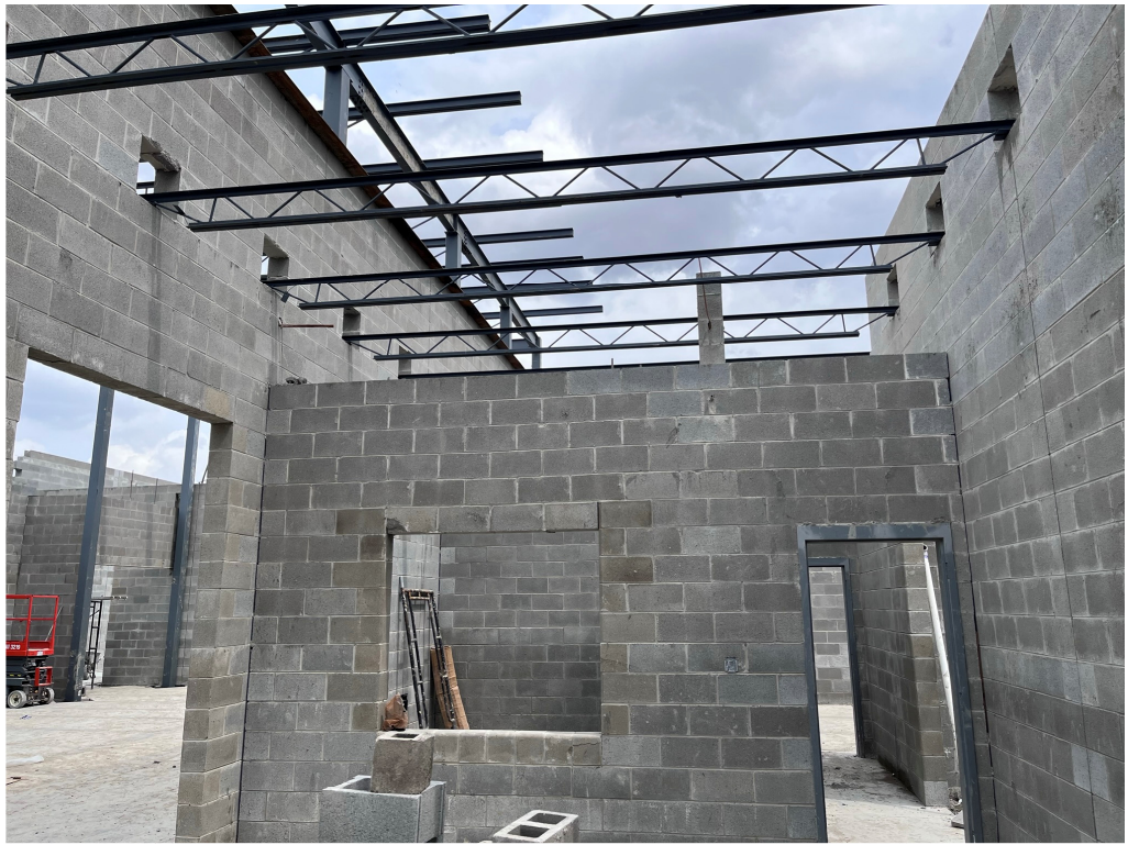
Figure 3 – TEHS Steel Setting
