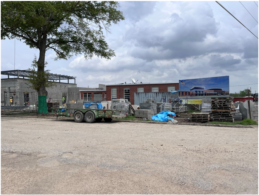
Figure 1 – TEHS Front of Site
