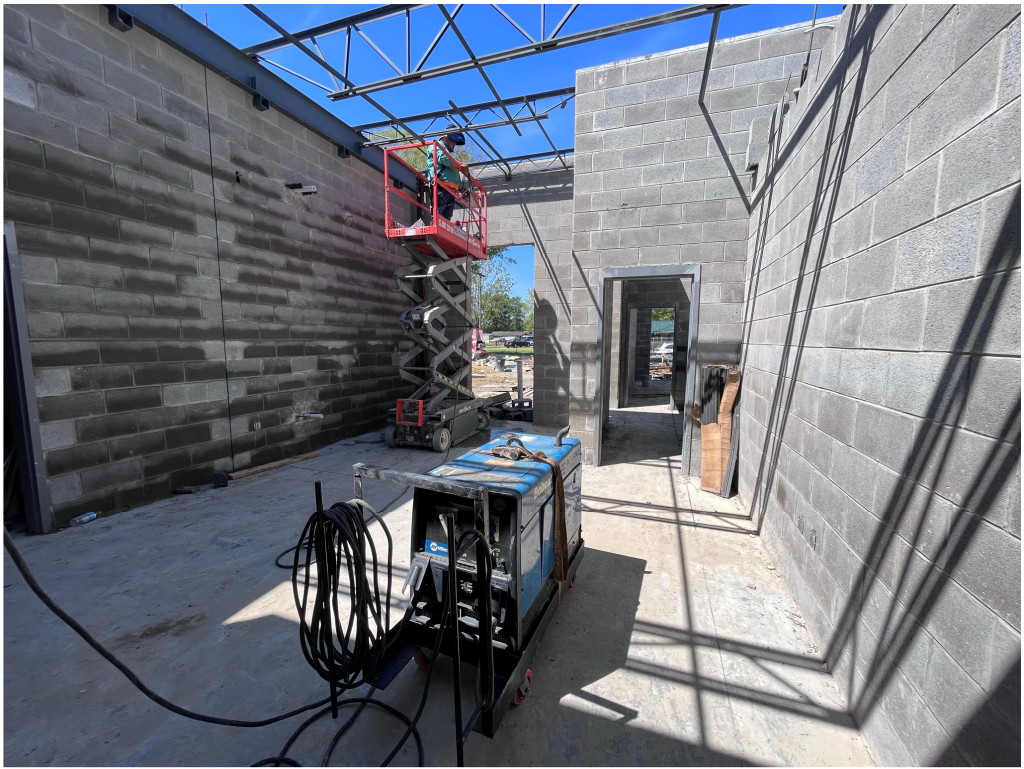
Figure 7 – TEHS Steel Setting
