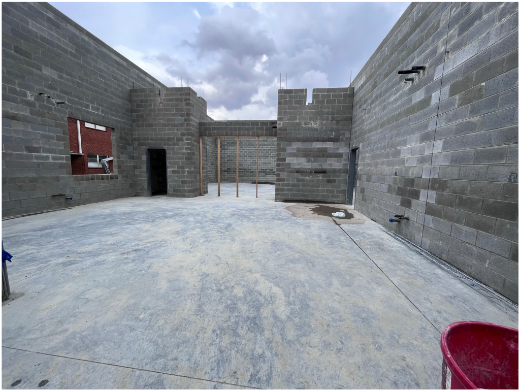
Figure 6 – TEHS Steel Setting
