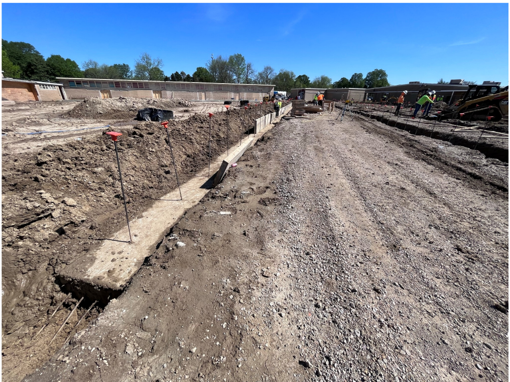
Figure 18 – Footing Forms Installation is ongoing
