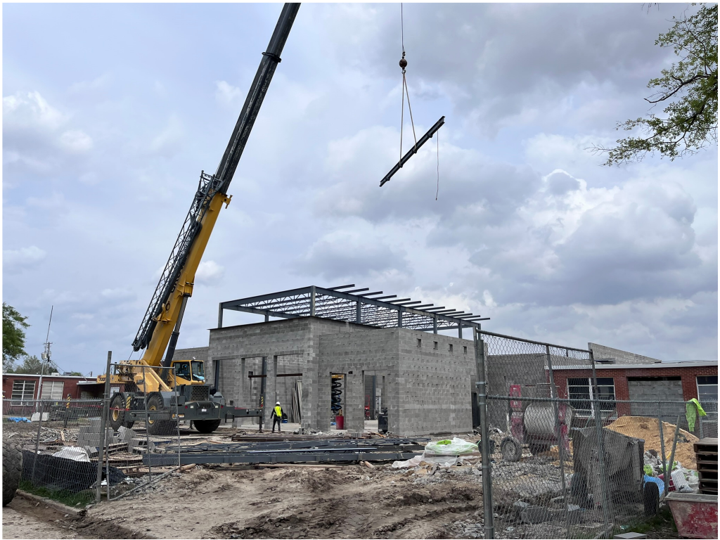
Figure 2 – TEHS Steel Setting
