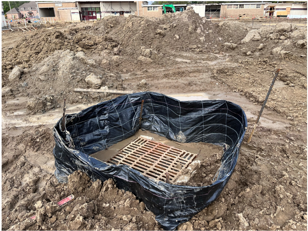
Figure 14 – Silt Fencing in Use
