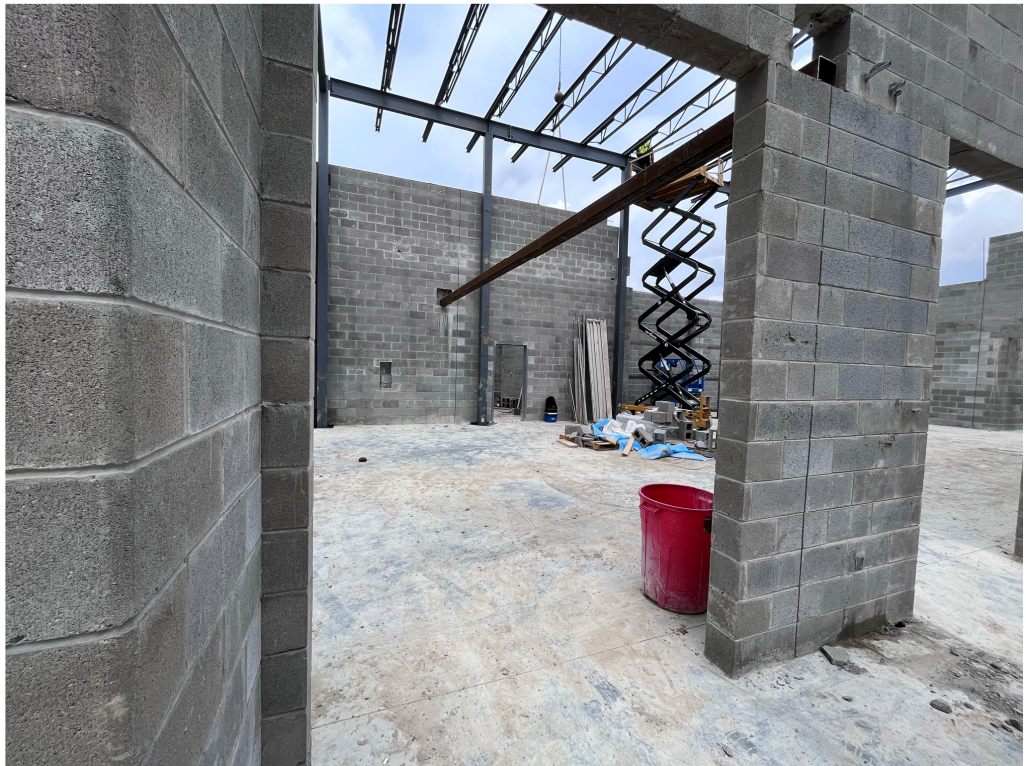
Figure 4 – TEHS Steel Setting
