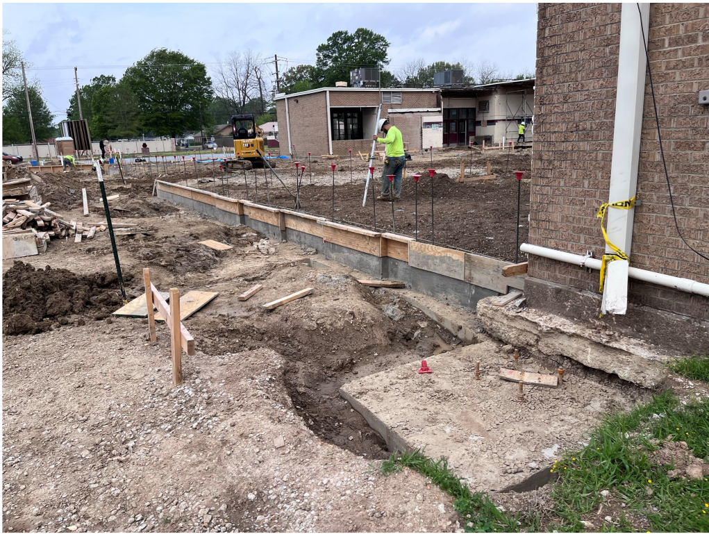
Figure 9 – Foundation work near cafeteria at Gentry
