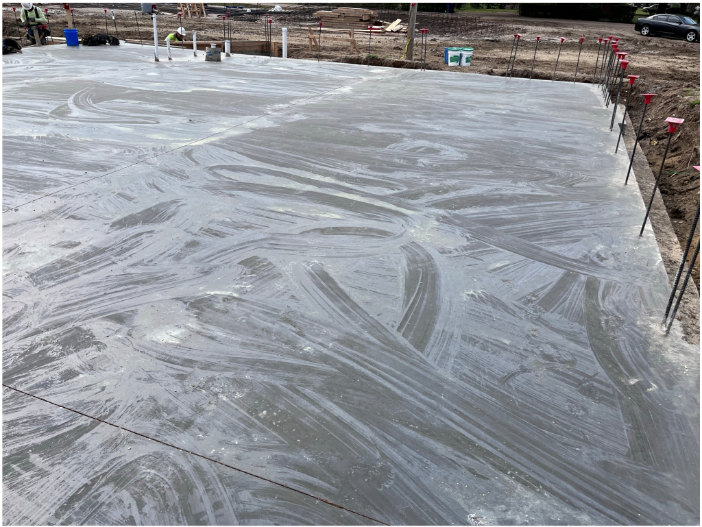
Figure 11 – New Slab at Admin at Gentry
