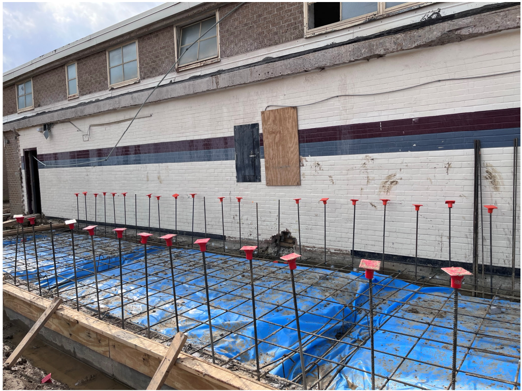
Figure 13 – Typical Foundation Prep
