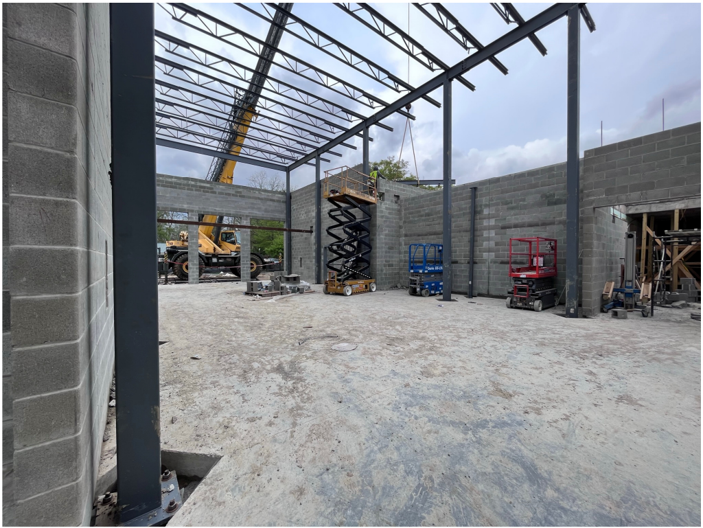
Figure 5 – TEHS Steel Setting
