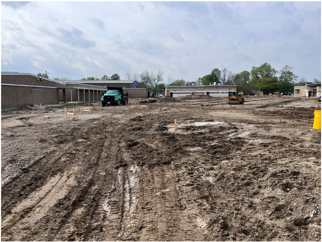
Figure 15 – Gentry Work Yard
