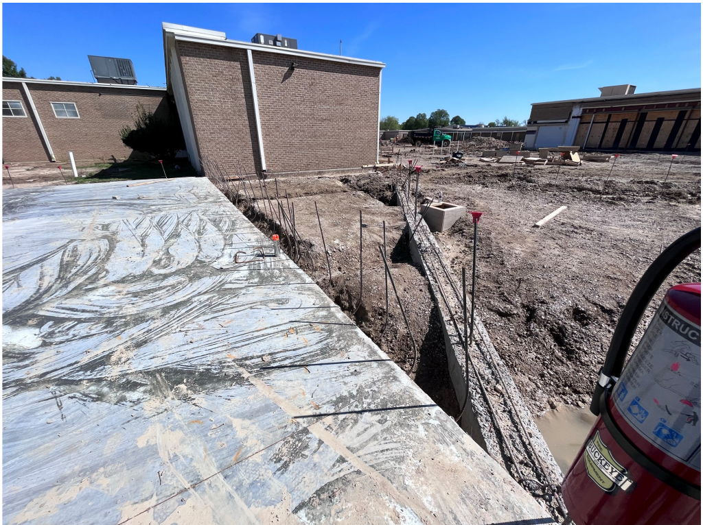
Figure 17 – Continued Foundation Work at Gentry
