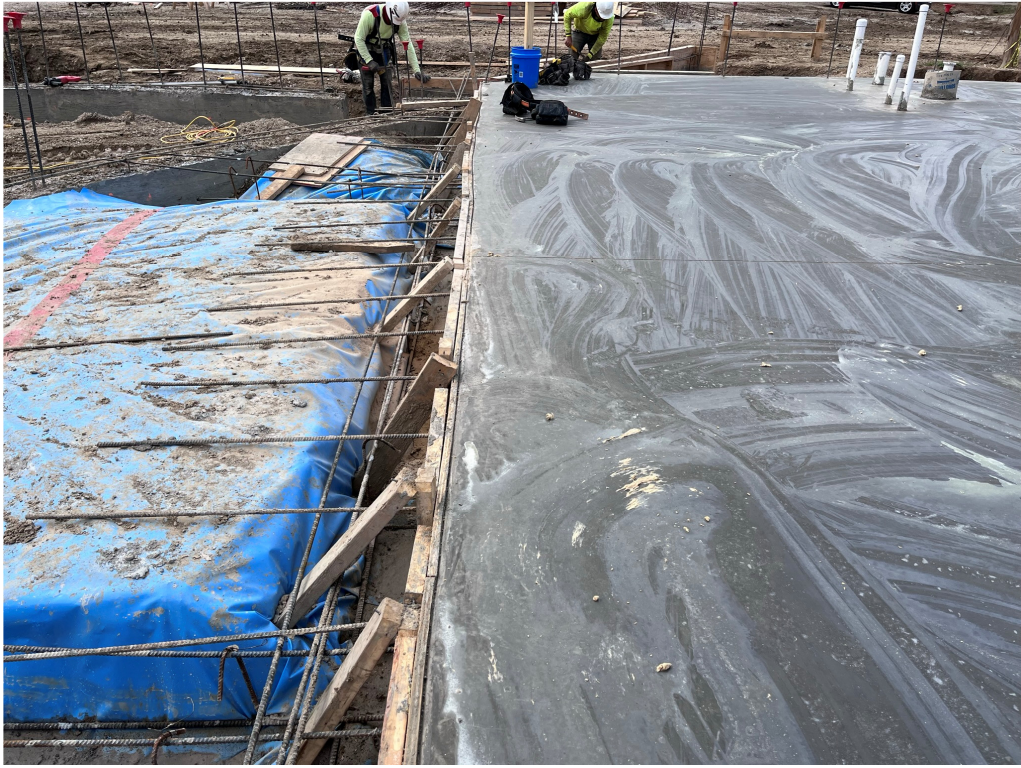
Figure 10 – New Slab at Admin at Gentry
