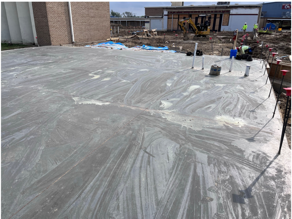
Figure 12 – New Slab at Admin at Gentry
