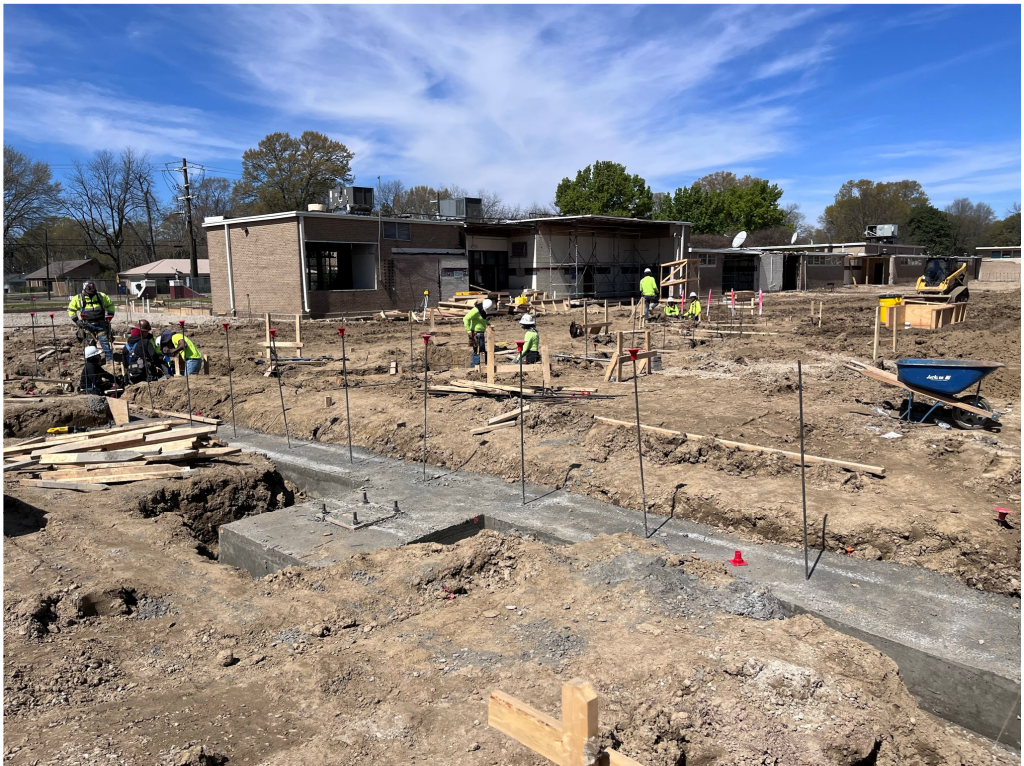
Figure 10 – GHS Concrete Footings Poured
