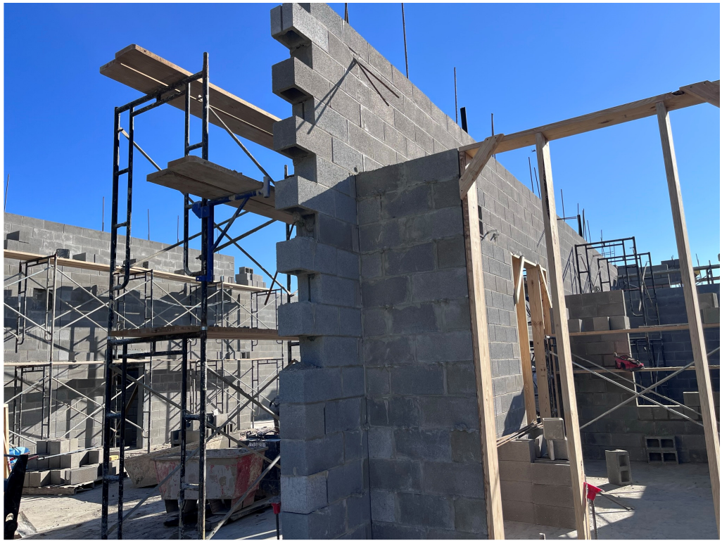
Figure 3 – THES Masonry is Ongoing
