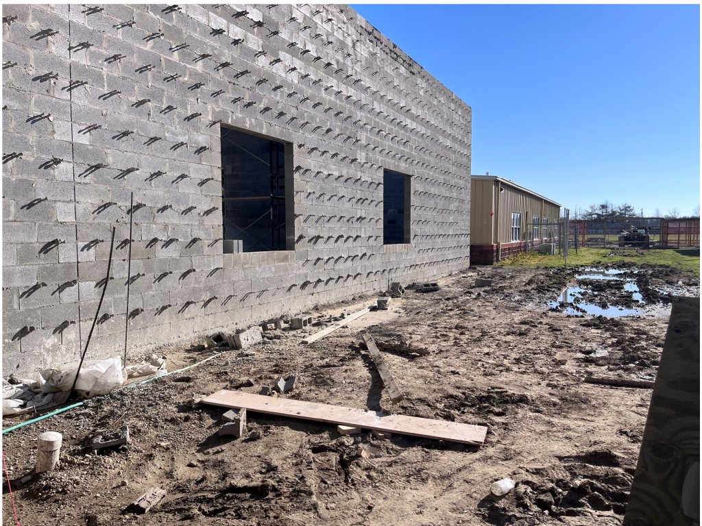
Figure 8 – THES Southern Wall at STEM Class Room Addition
