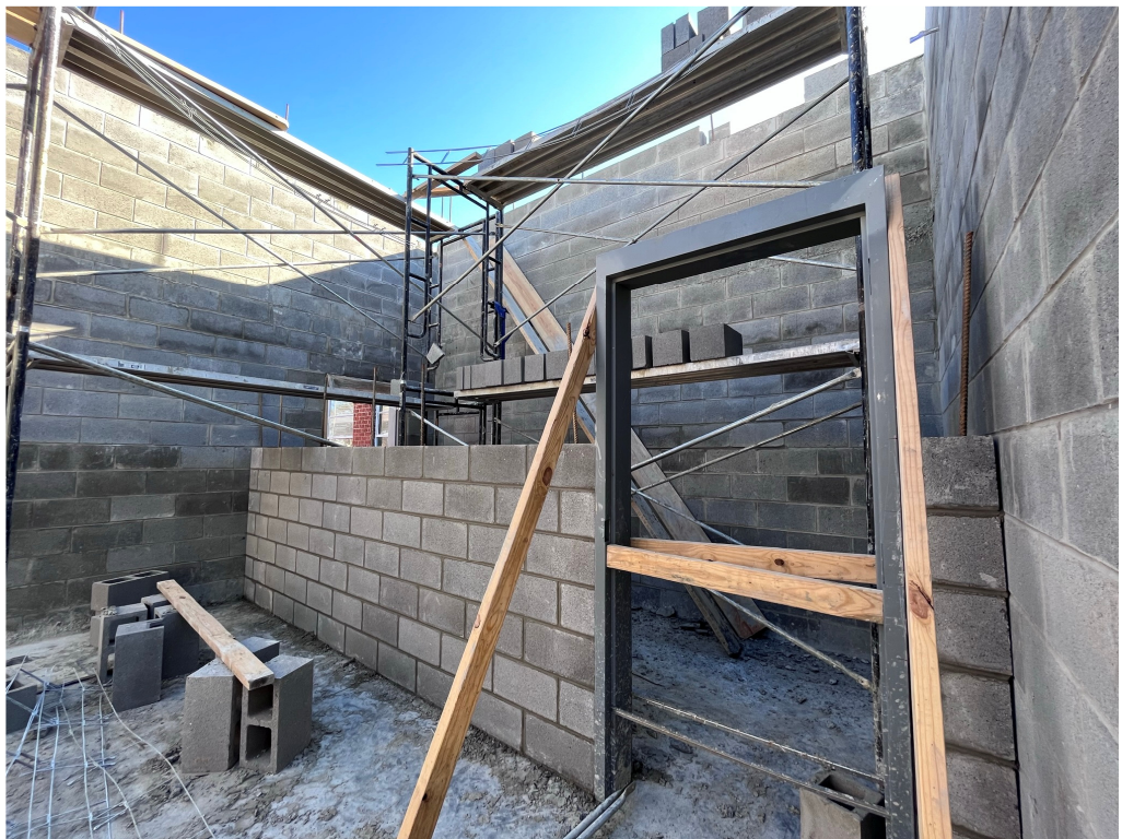
Figure 6 – THES Conference Room Wall
