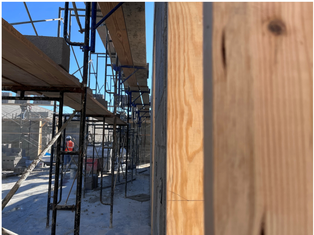
Figure 4 – THES Masonry Appears Straight and in Good Condition
