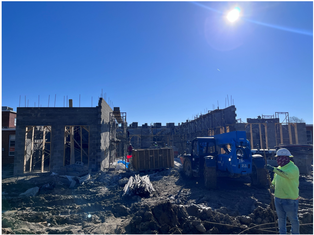
Figure 1 – THES Building Frontage Progress
