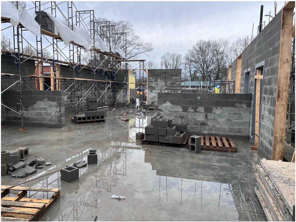
Figure 35 – TEHS Block Work
