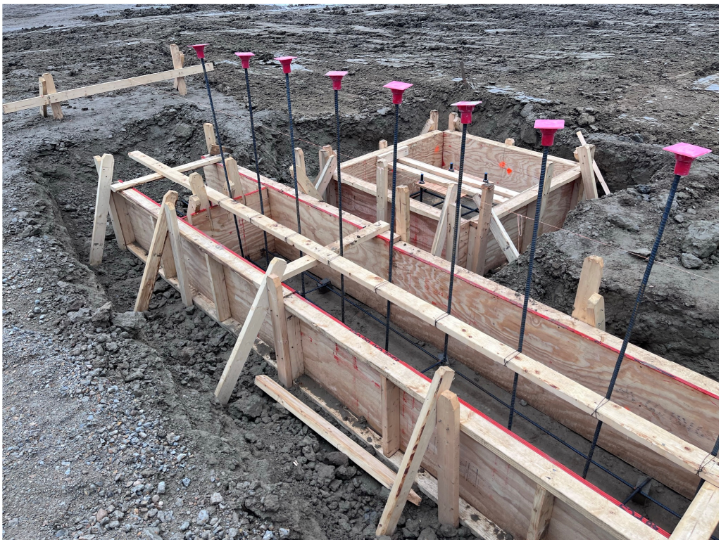
Figure 12 – GHS Rebar Install at Formwork
