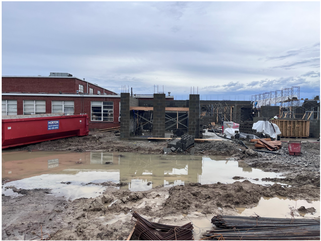
Figure 23 – TEHS Lay Down Yard at Front
