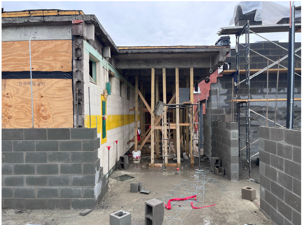
Figure 28 – TEHS Tie In at Existing Hallway
