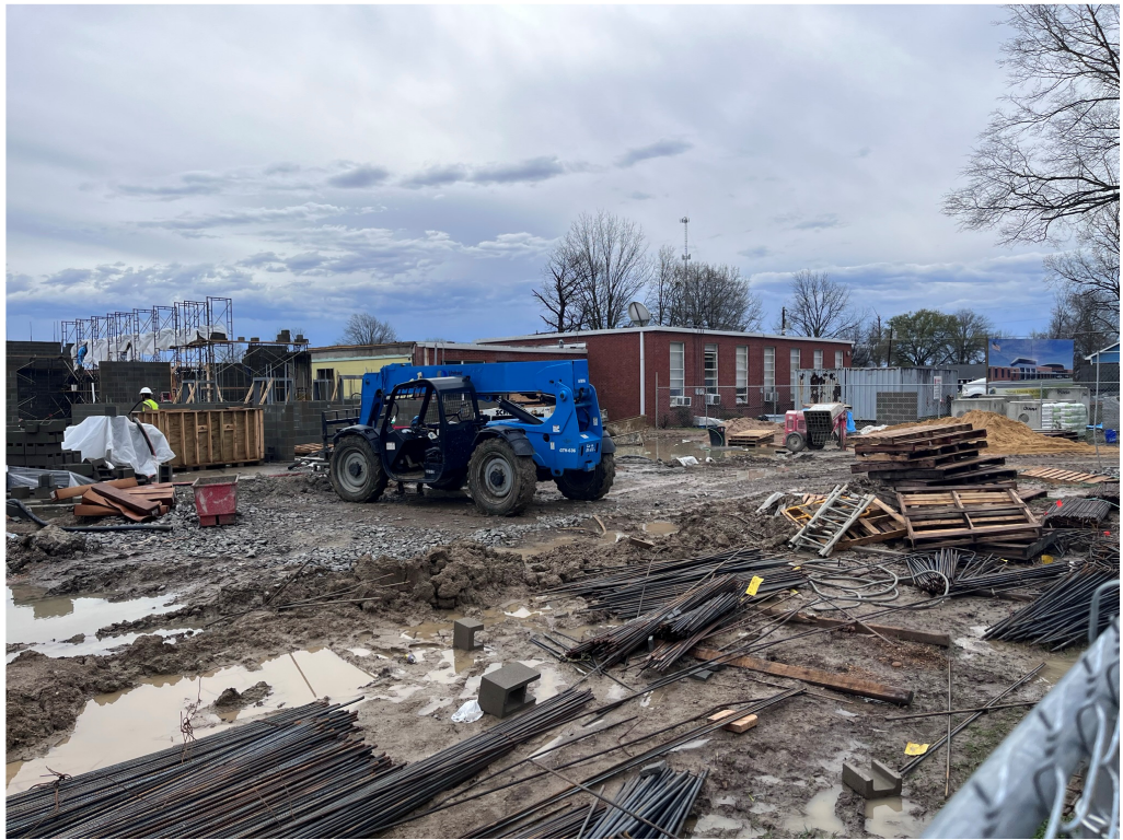
Figure 24 – TEHS Lay Down Yard at Front
