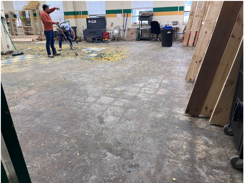
Figure 38 – TEHS Media Center Flooring Demo
