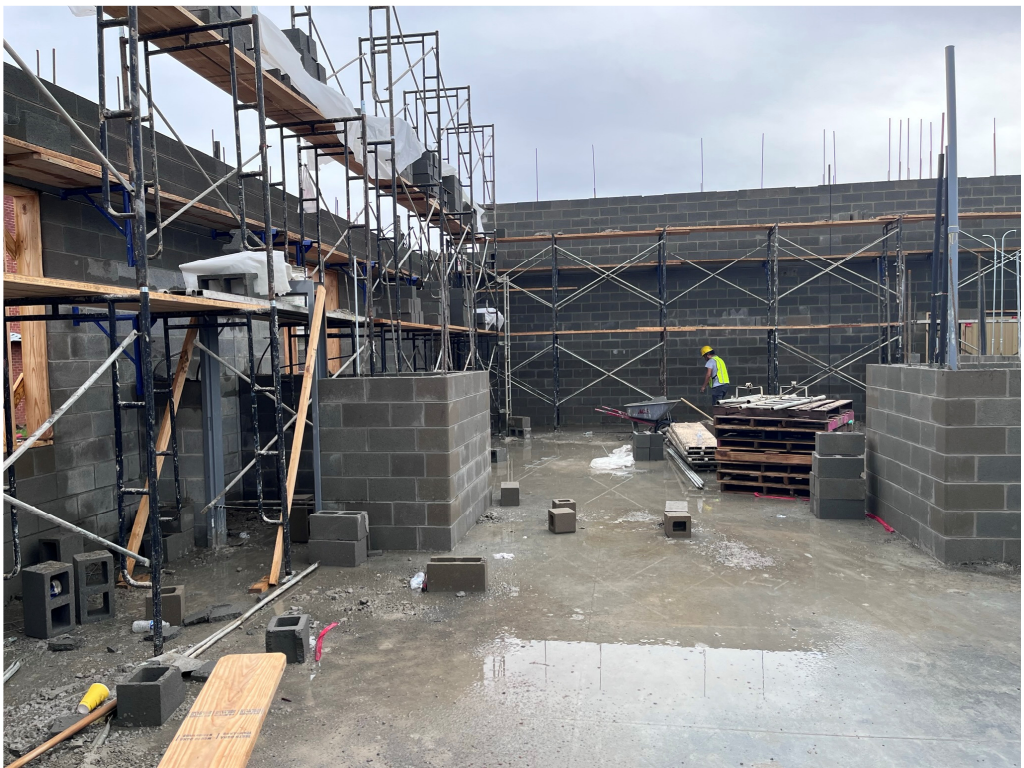
Figure 32 – TEHS Block Work
