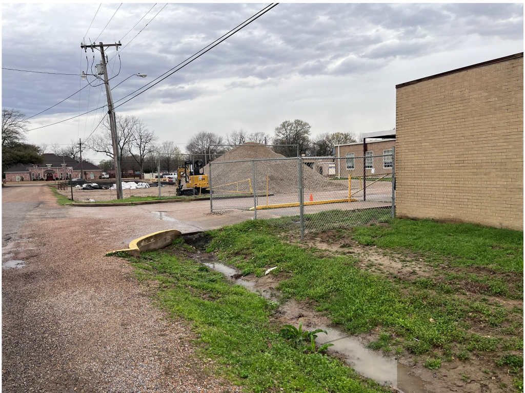
Figure 2 – GHS Temp Fencing and Gate at Gym
