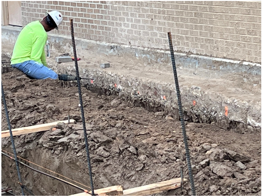
Figure 18 – GHS Foundation work and Rebar Tie In at North Building
