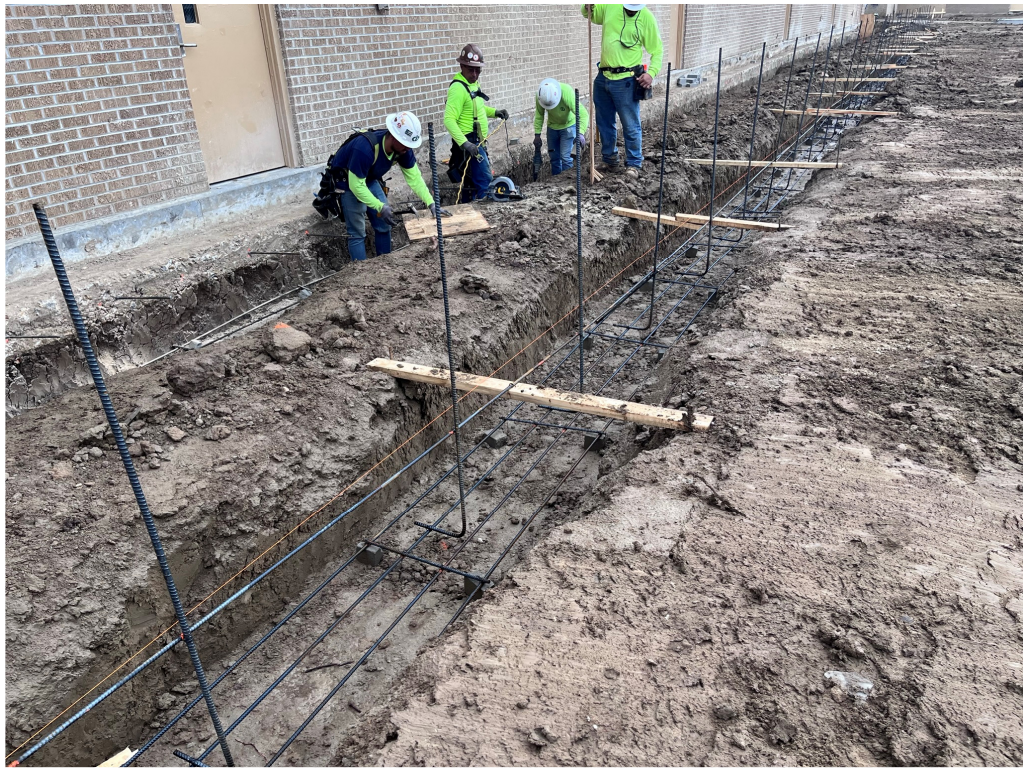
Figure 17 – GHS Foundation work and Rebar Tie In at North Building
