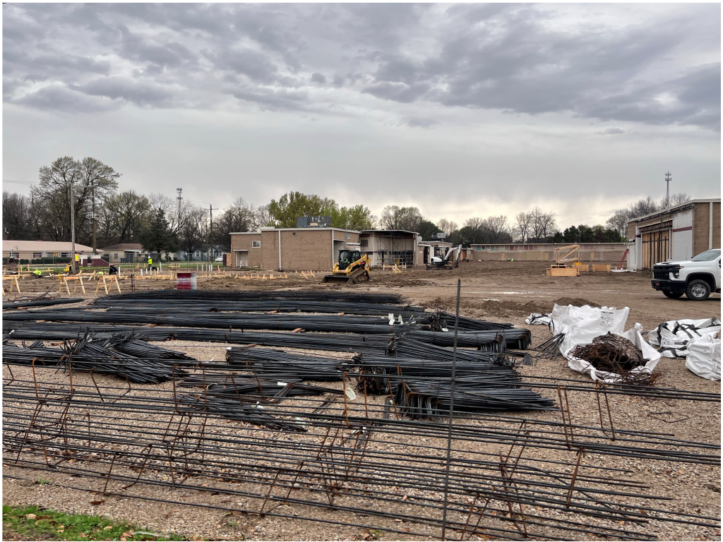
Figure 4 – GHS Lay Down Yard on Southwest Corner
