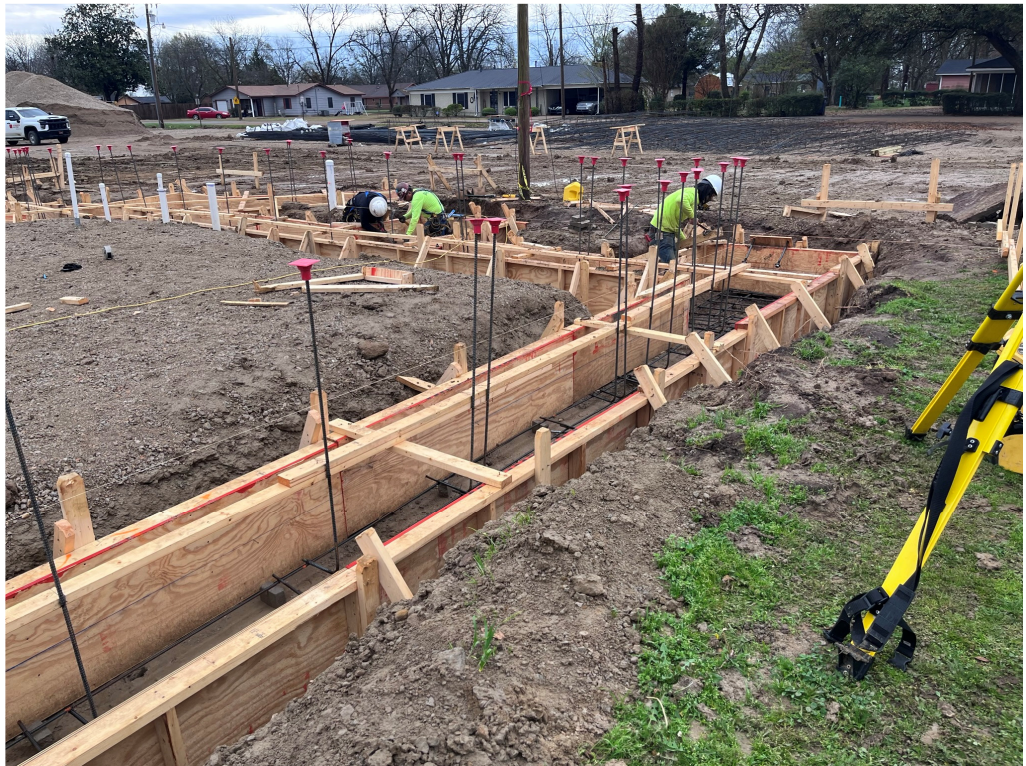
Figure 6 – GHS Formwork
