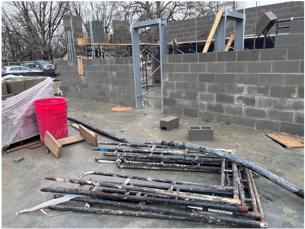
Figure 27 – TEHS Metal Door Frames Installed
