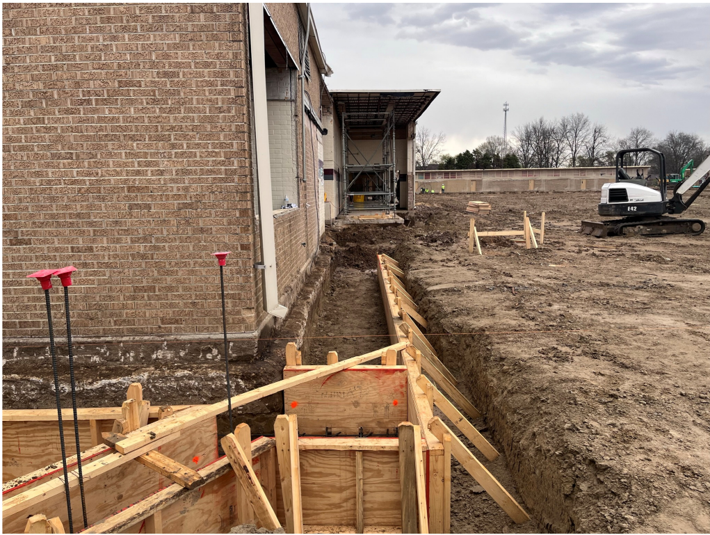
Figure 15 – GHS Foundation Formwork @ Southwest Corner
