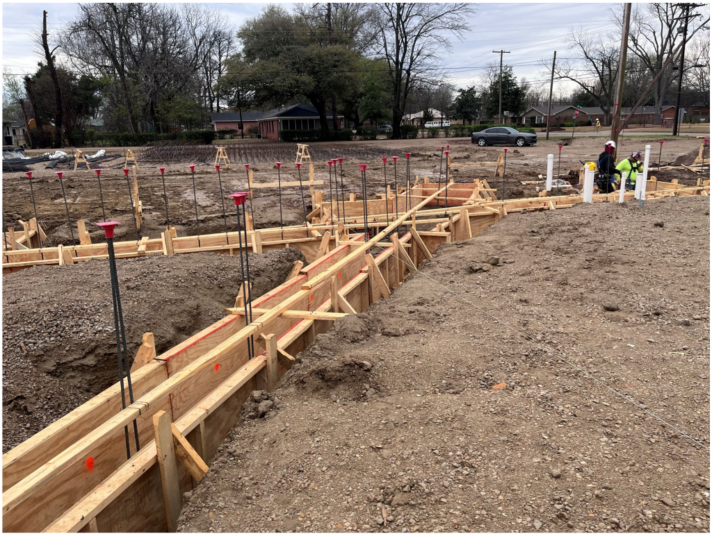
Figure 11 – GHS Forming at Diagonal Wall
