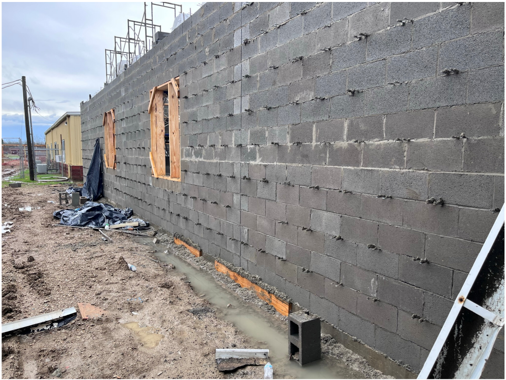
Figure 29 – TEHS Exterior Block and Brick Ties
