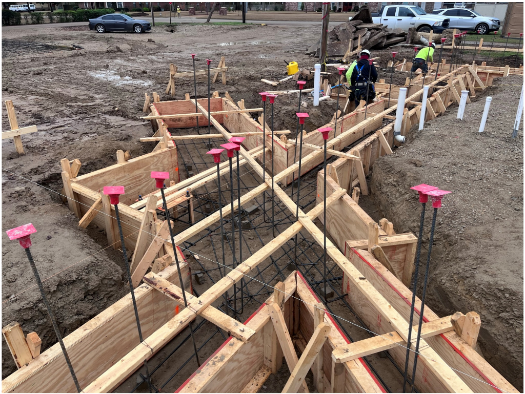
Figure 13 – GHS Rebar Install at Formwork
