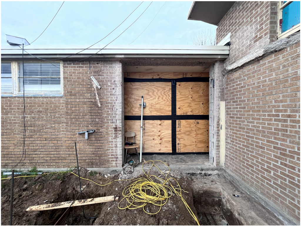
Figure 19 – GHS Foundation work and Rebar Tie In at North Building
