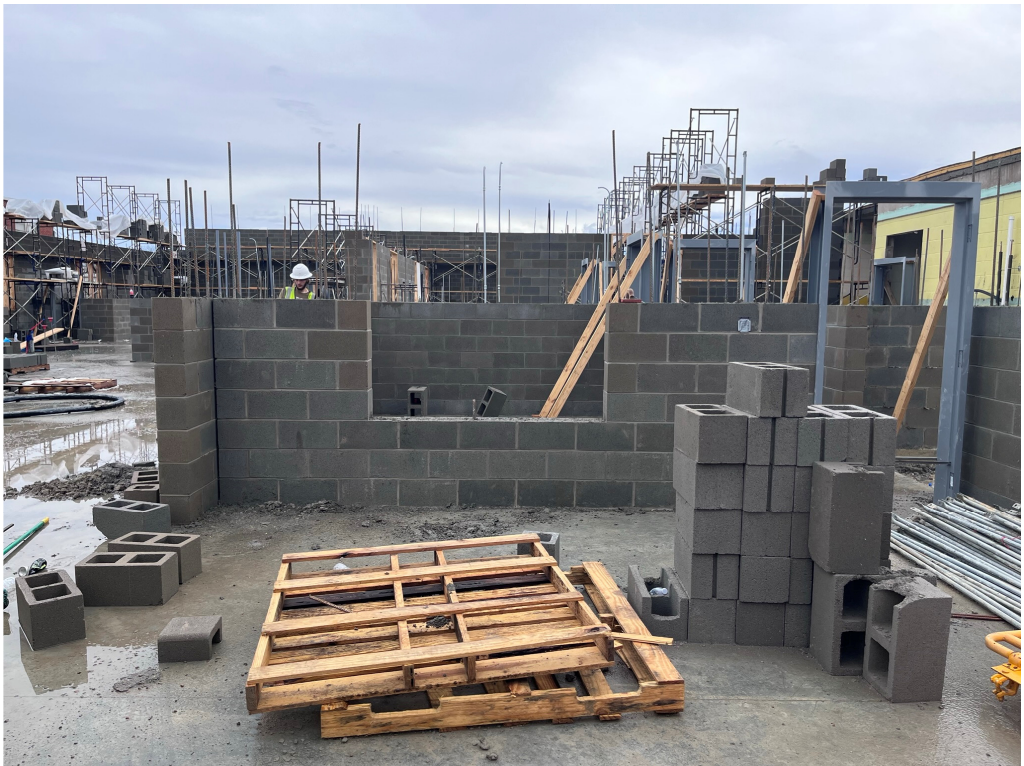
Figure 25 – TEHS Block Work at Reception
