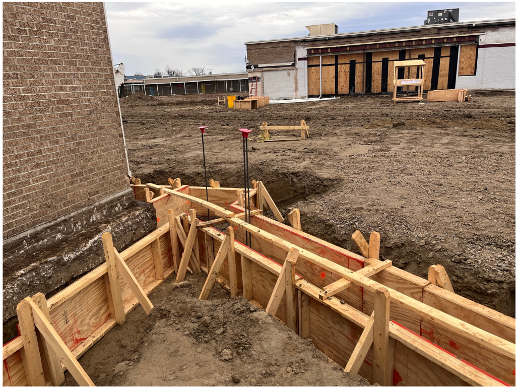
Figure 10 – GHS Forming at Diagonal Wall
