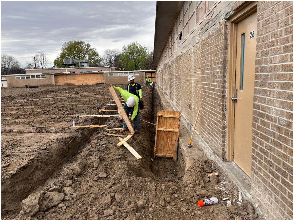
Figure 20 – GHS Foundation work and Rebar Tie In at North Building
