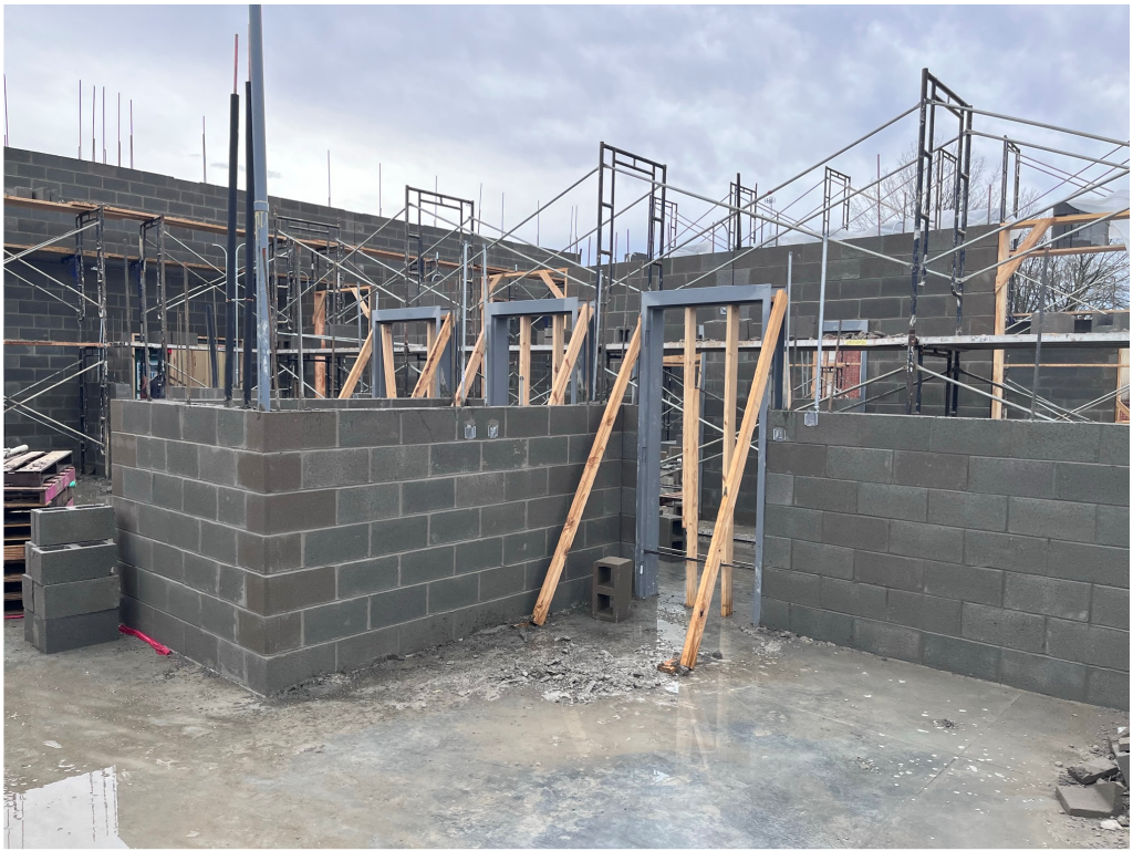
Figure 33 – TEHS Block Work
