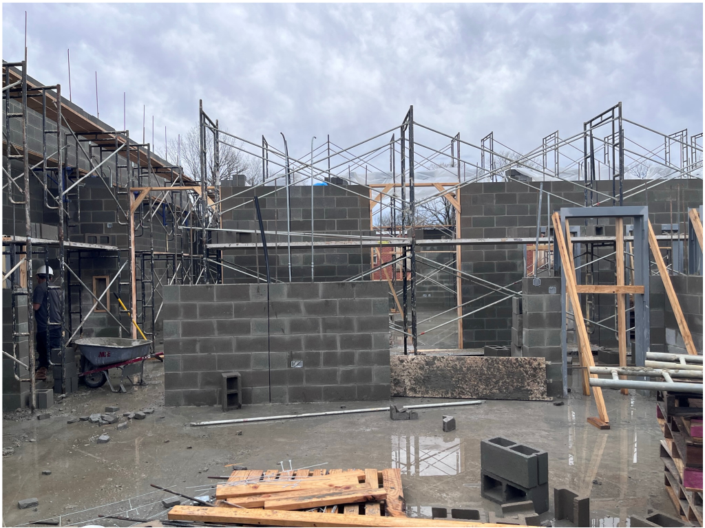
Figure 34 – TEHS Block Work
