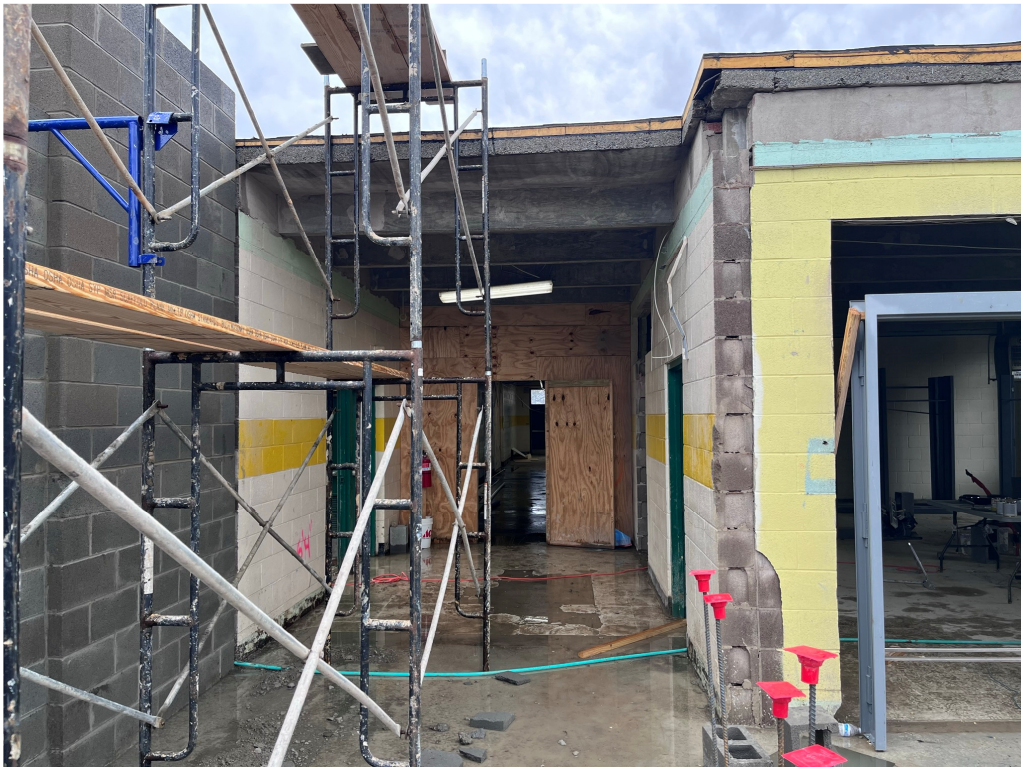
Figure 36 – TEHS Block Work
