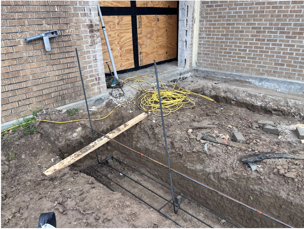
Figure 16 – GHS Foundation work and Rebar Tie In at North Building
