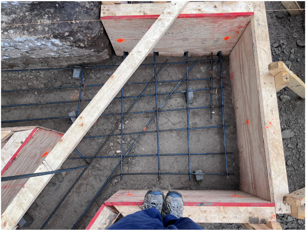
Figure 14 – GHS Rebar Install at Formwork
