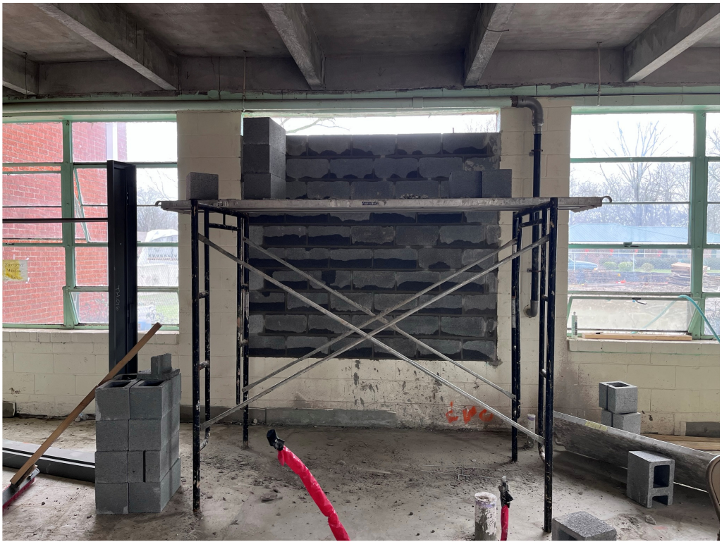
Figure 37 – TEHS Blocking at Windows
