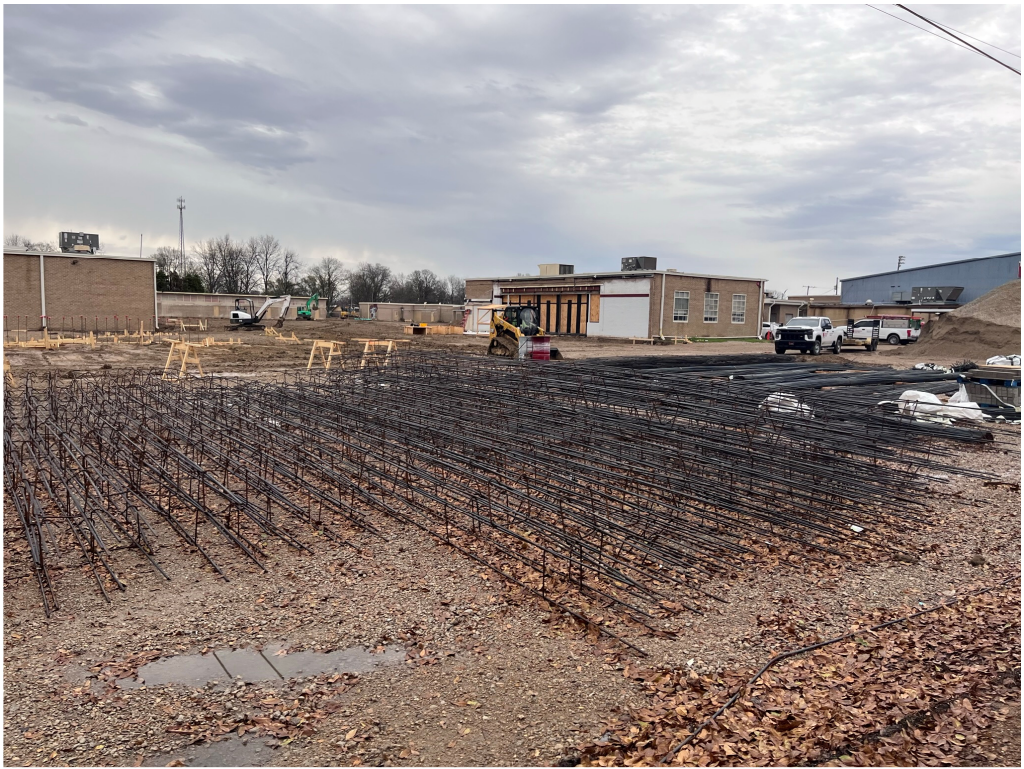
Figure 3 – GHS Lay Down Yard on Southwest Corner
