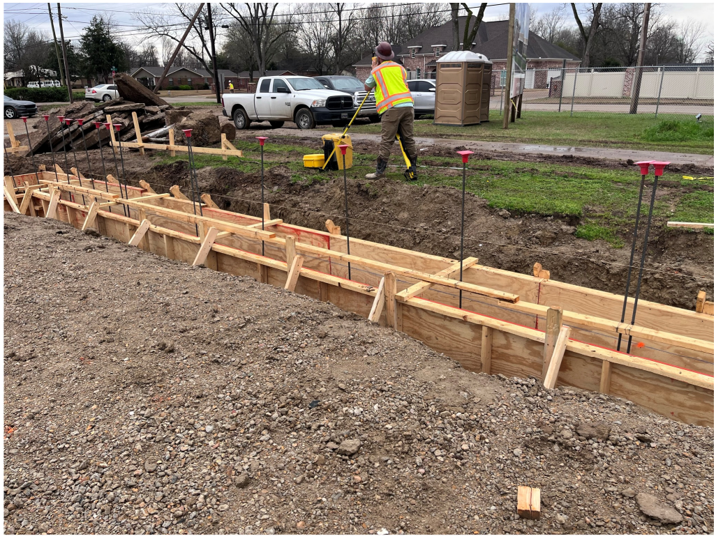
Figure 9 – GHS Worker Surveying
