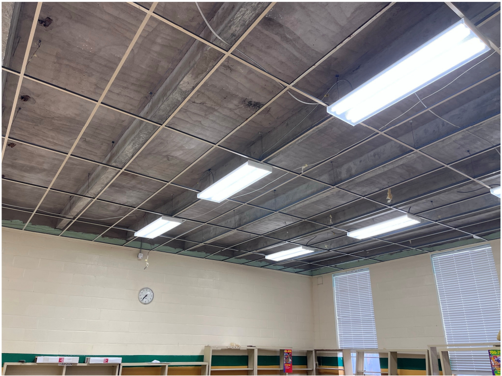
Figure 40 – TEHS Media Center Ceiling Demo
