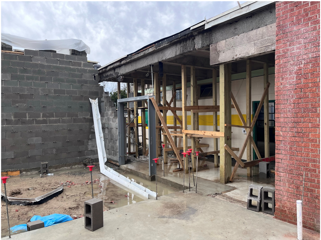
Figure 30 – TEHS Tie In at Existing Hallway
