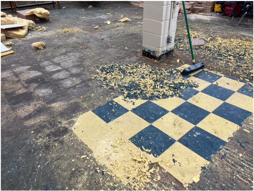
Figure 39 – TEHS Media Center Floor Demo
