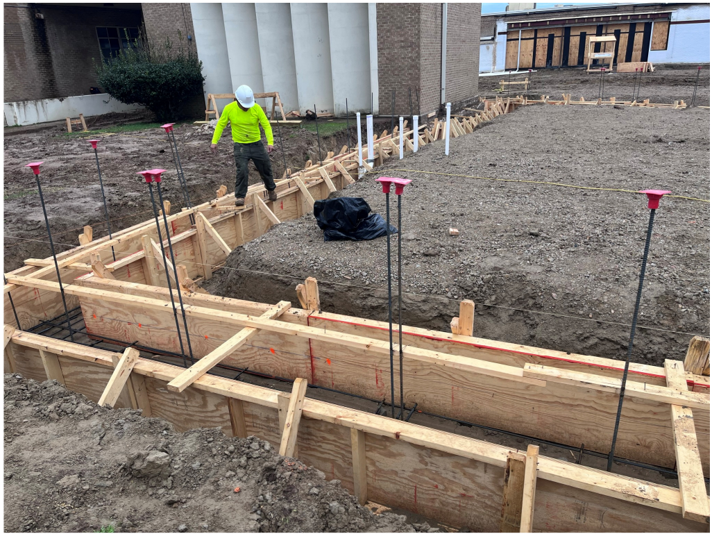
Figure 5 – GHS Formwork
