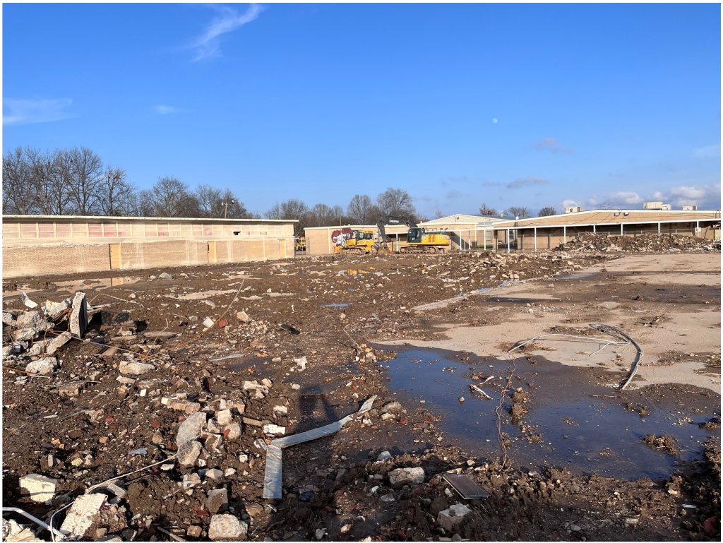
Figure 9 – Demolition @ Interior Yard with remaining buildings in background
