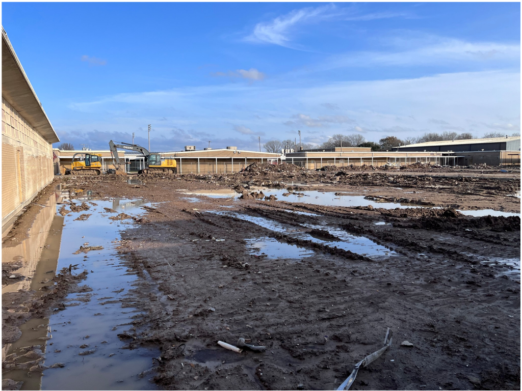
Figure 4 – Demolition @ Interior Yard with remaining buildings in background
