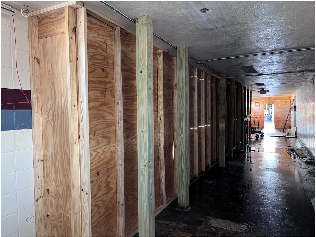
Figure 6 – Temporary construction @ West Hall
