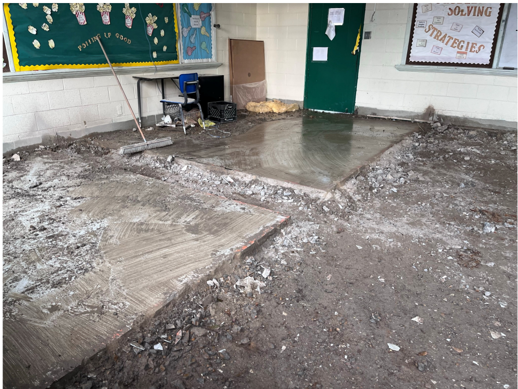
Figure 31 – Concrete demo at south building wing to remain @ Thomas Edwards
