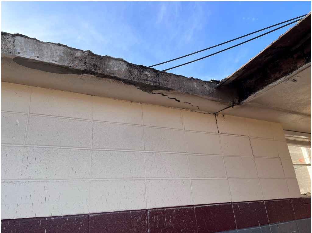
Figure 14 – Concrete Deck Cut back during demolition @ West Hall
