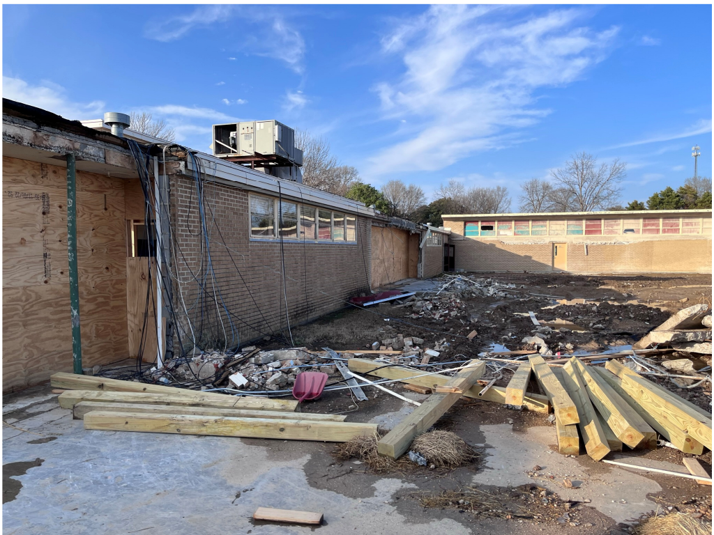
Figure 10 – Demolition @ Interior Yard with remaining buildings in background & foreground
