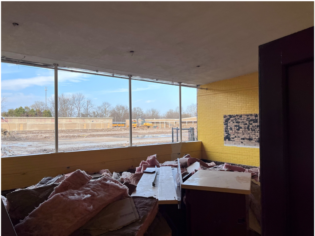
Figure 21 – South Building still to be Demolished
