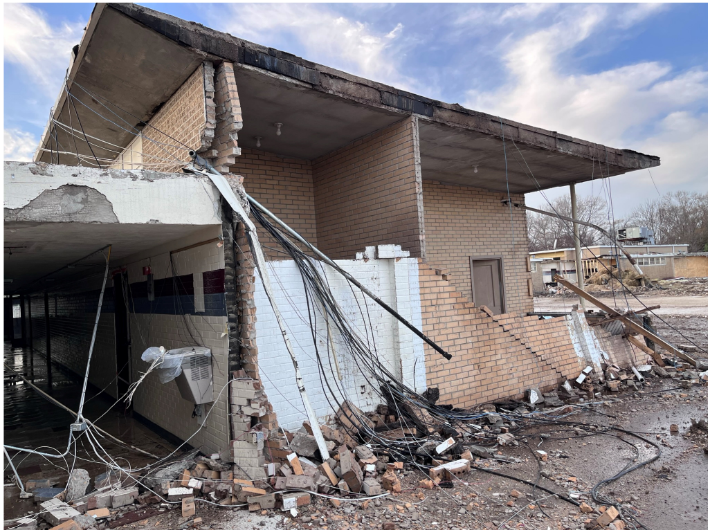
Figure 24 – South Building still to be demolished
