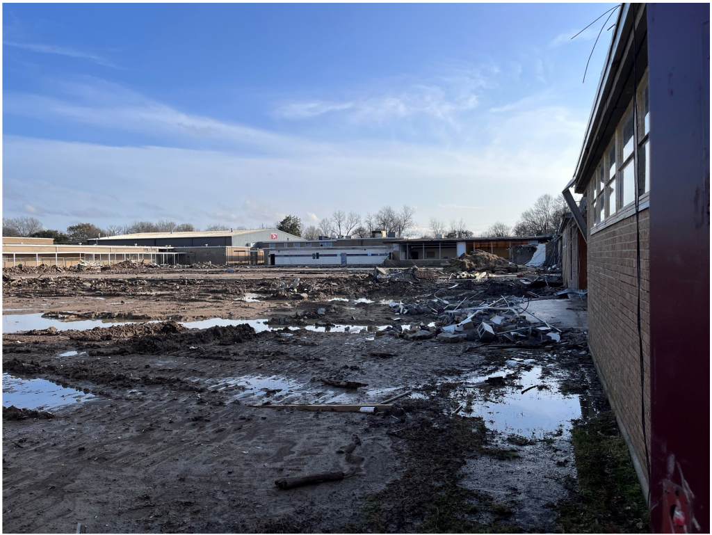
Figure 5 – Demolition @ Interior Yard with remaining buildings in foreground
