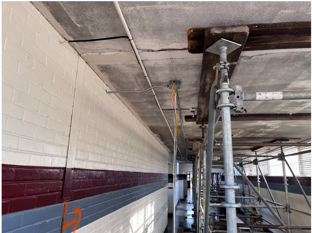
Figure 16 – Temporary Shoring at west building/hall to remain
