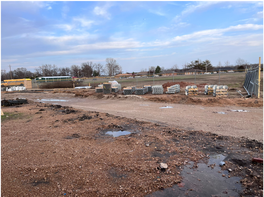
Figure 34 – Site work at Back of School
