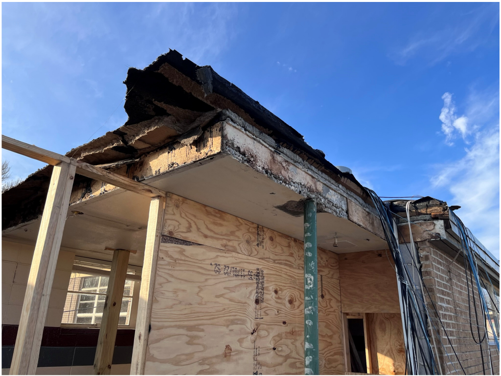
Figure 13 – Existing West Hall Construction
