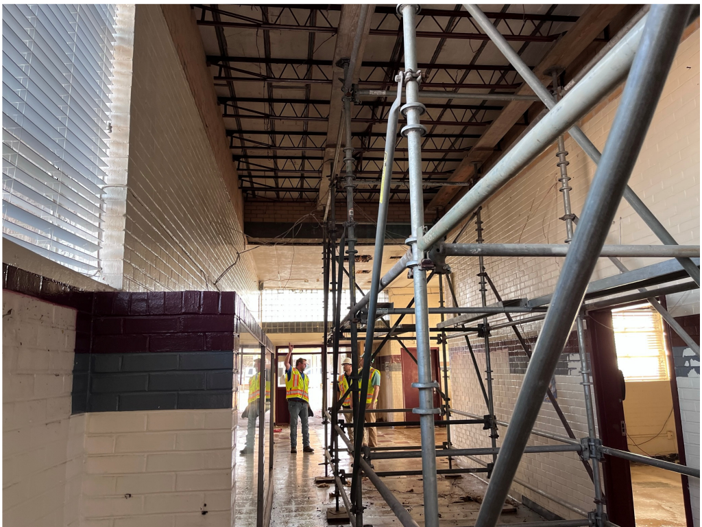
Figure 18 – Entry lobby (ceiling to remain [wall on left to be restructured])
