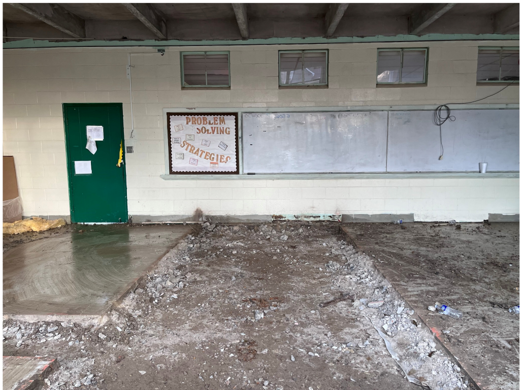
Figure 32 – Concrete demo at south building wing to remain @ Thomas Edwards
