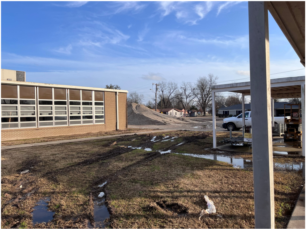
Figure 20 – Site work at Parking is Ongoing
