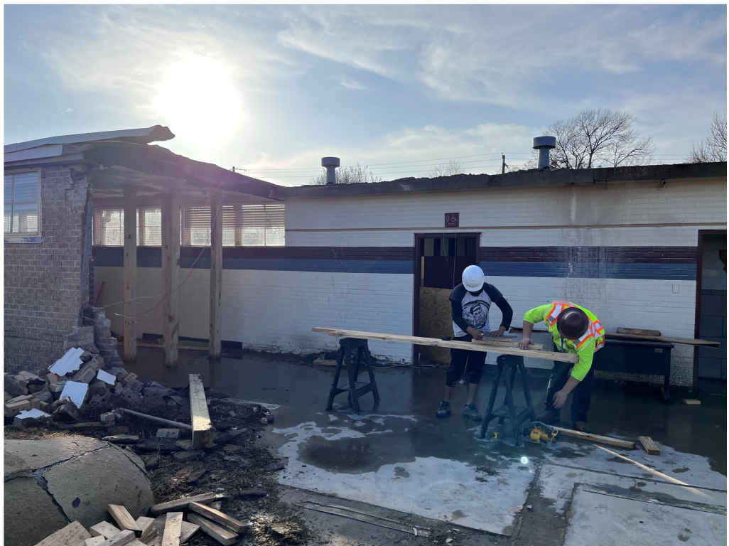
Figure 12 – Demolition @ West Hall
