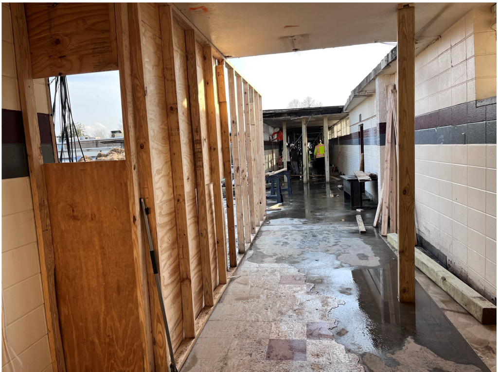
Figure 8 – Temporary construction @ West Hall
