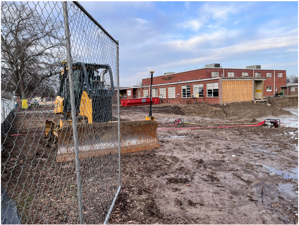
Figure 29 – Site Work is ongoing; pumping currently in progress
