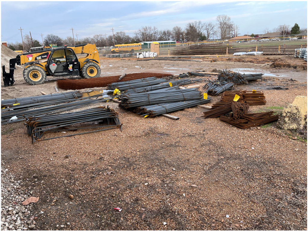
Figure 35 – Rebar Stored on Site
