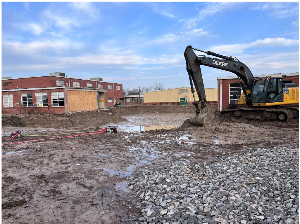
Figure 28 – Site Work is ongoing; pumping currently in progress
