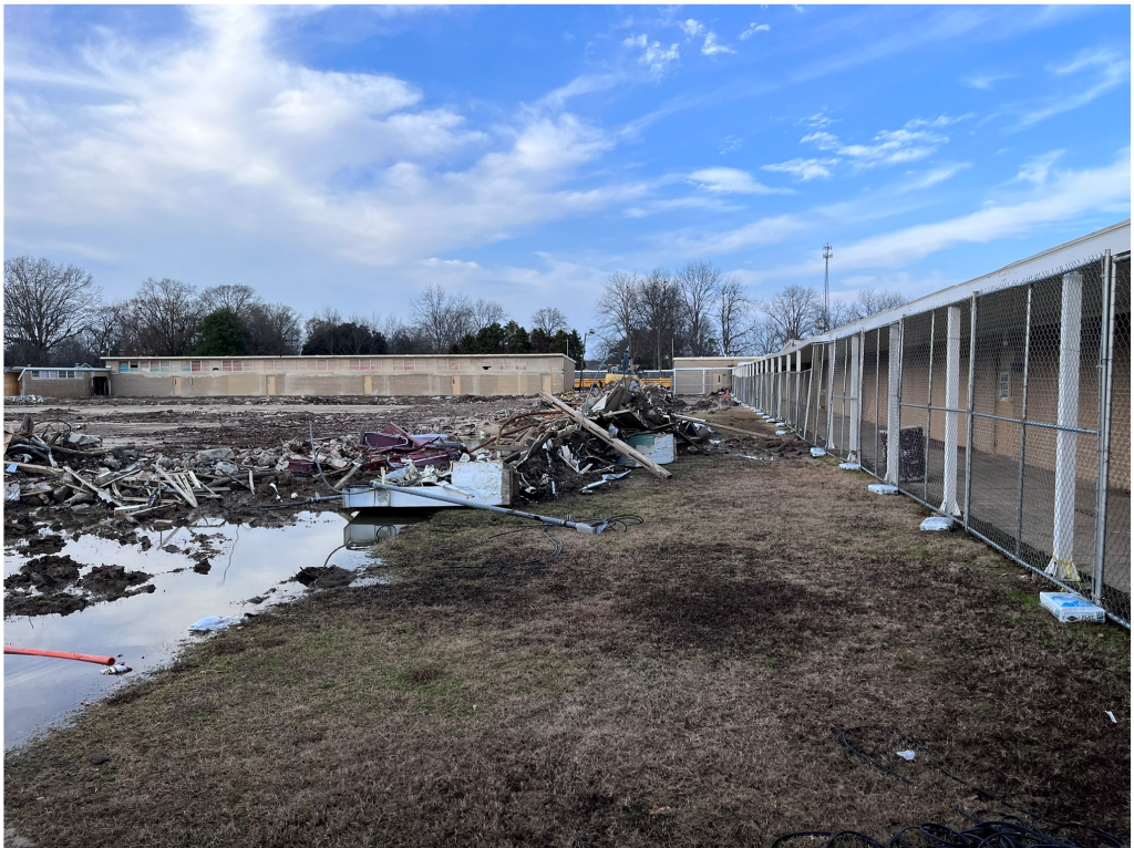
Figure 26 – Gentry Interior Courtyard Demolition/Site Work is Ongoing
