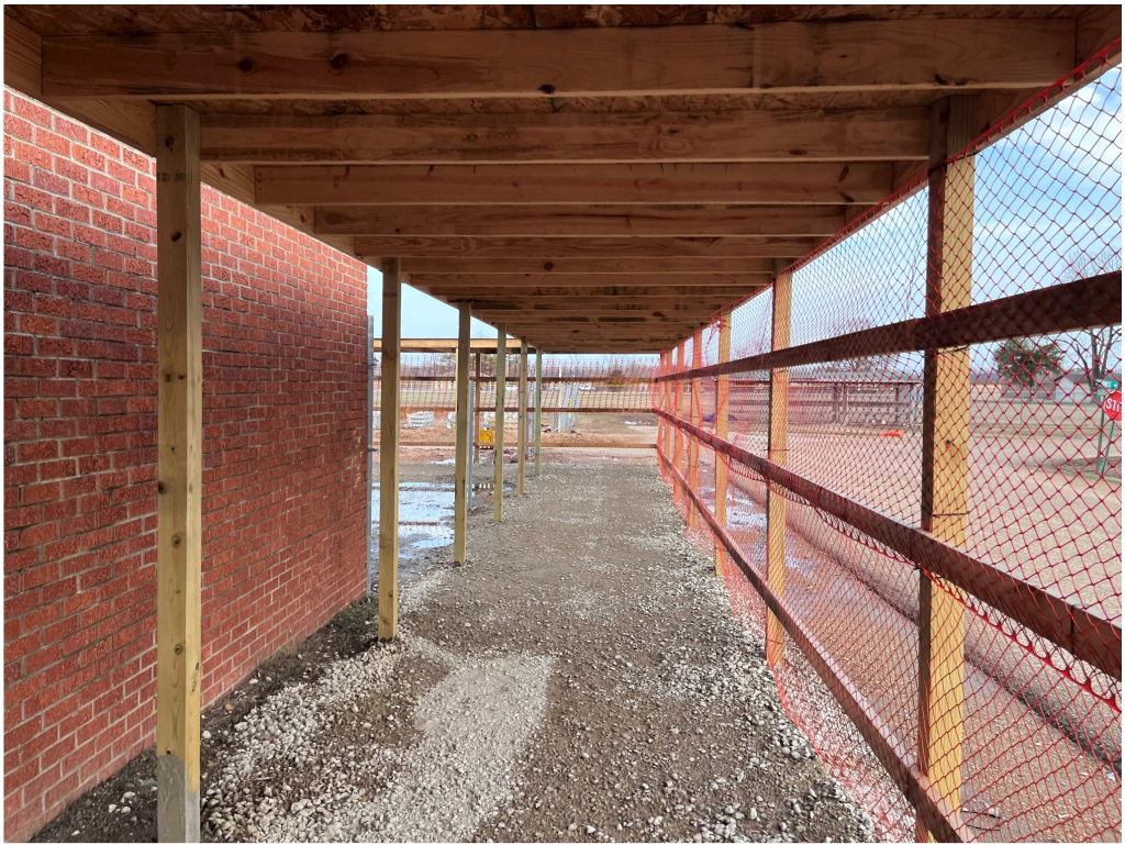
Figure 33 – Temporary Awning Appears in Good Shape; continue to maintain
