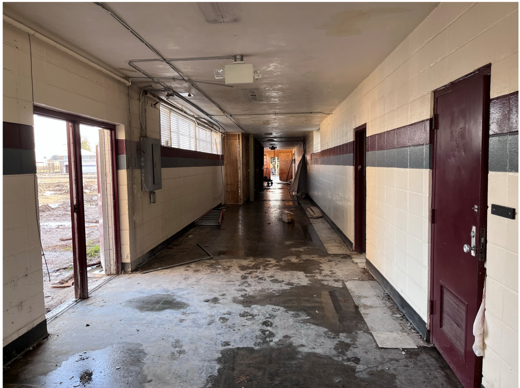
Figure 2 – Temporary construction @ West Hall looking south
