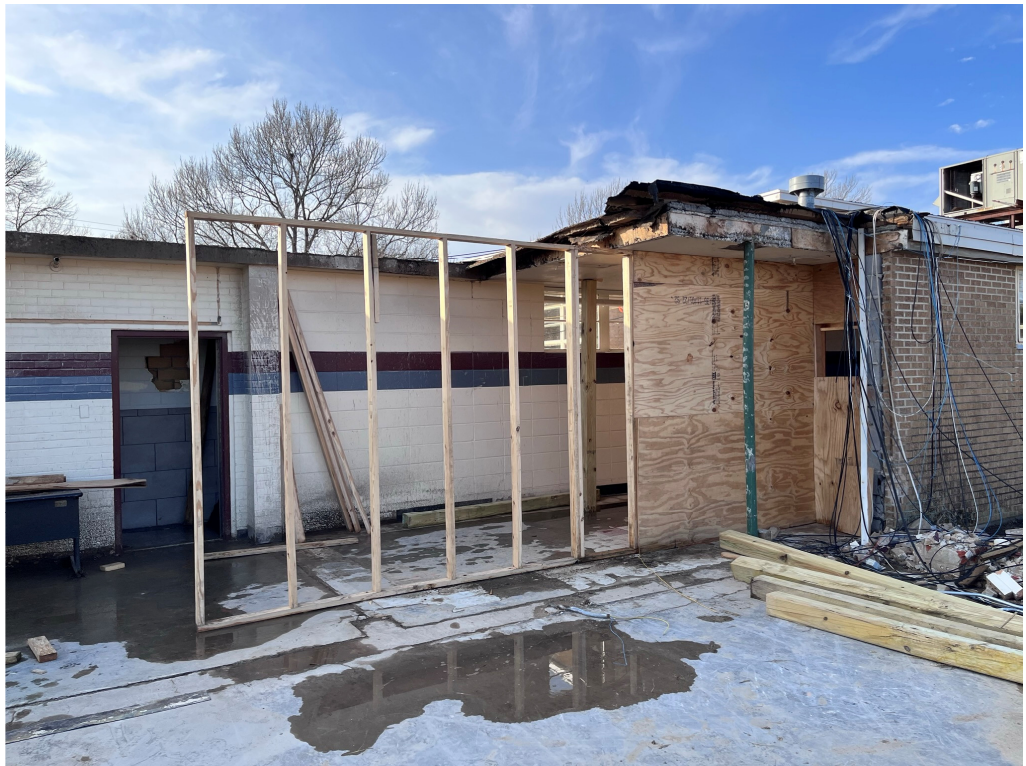
Figure 11 – Demolition @ West Hall
