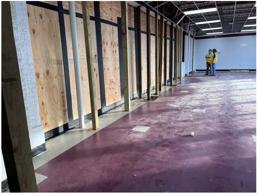
Figure 23 – Temporary Construction @ Cafeteria
