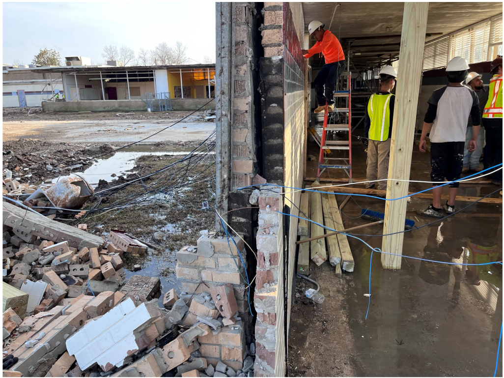
Figure 15 – Existing Wall Construction @ West Hall
