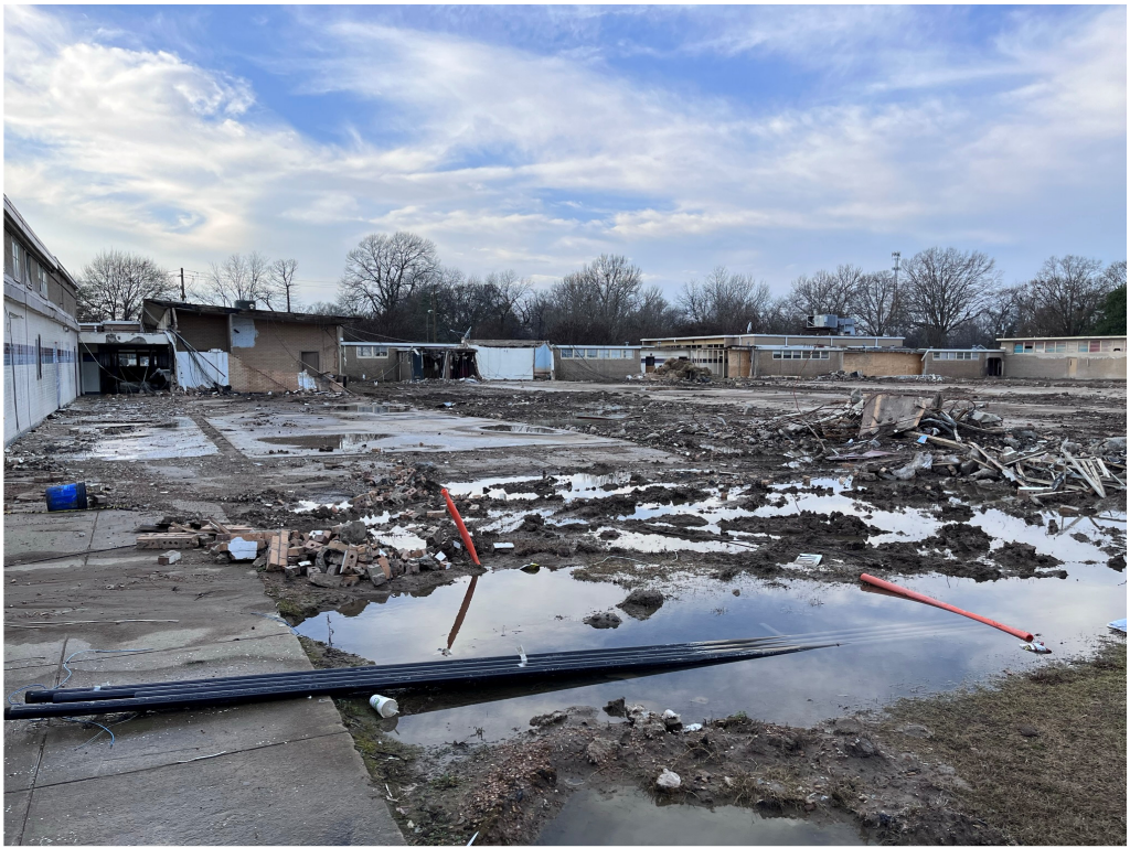
Figure 25 – Gentry Interior Courtyard Demolition/Site Work is Ongoing
