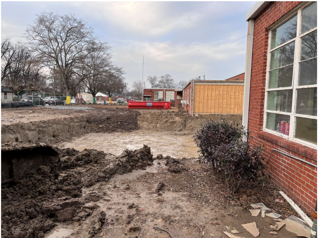
Figure 30 – Continued Excavation at Thomas Edwards New Construction
