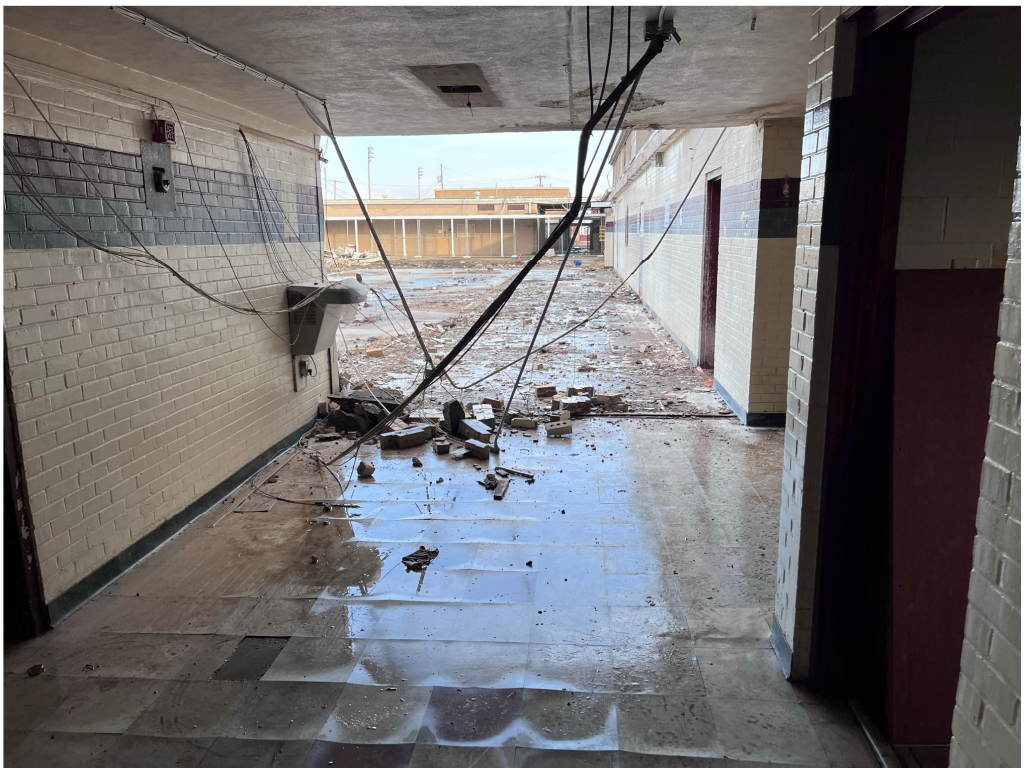
Figure 22 – South Building still to be Demolished
