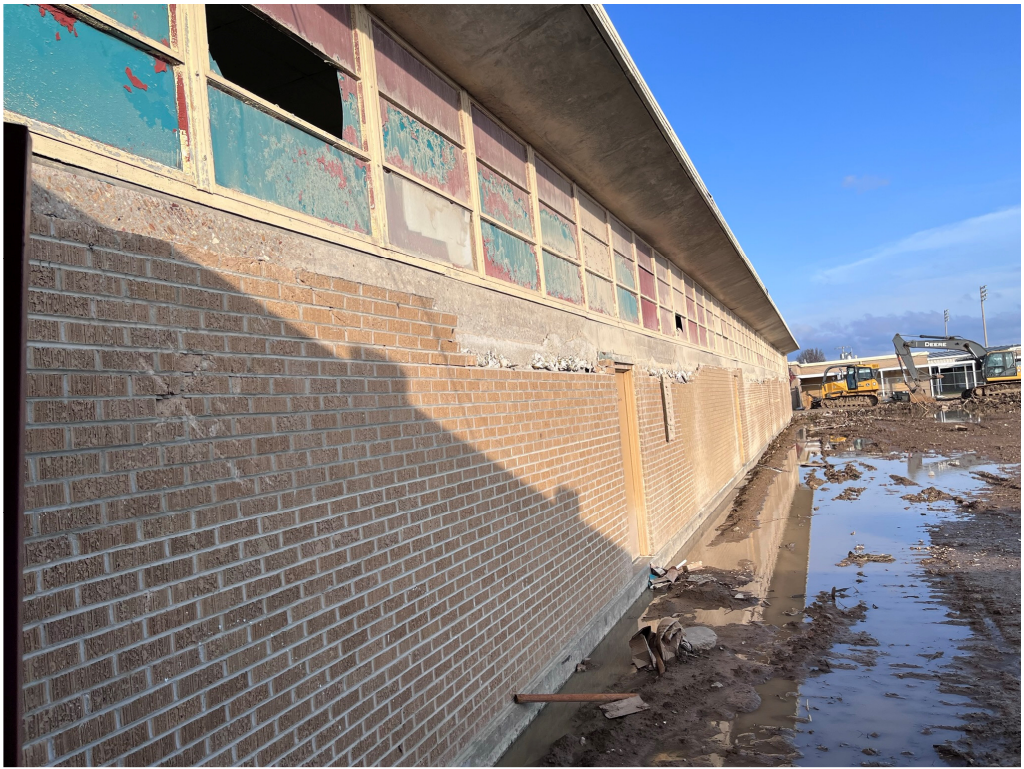
Figure 3 – Demolition @ Interior Yard with remaining buildings in foreground & background
