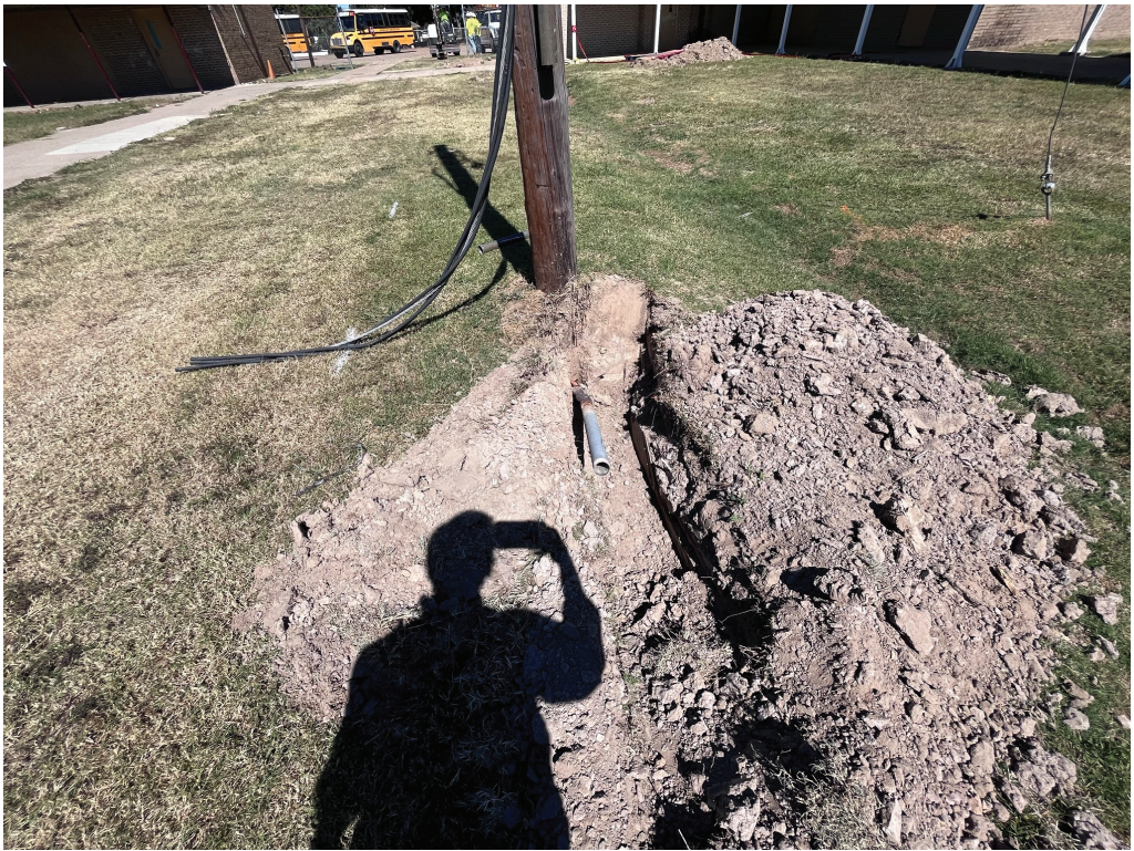
Figure 9 – Electrical Utilities removed
