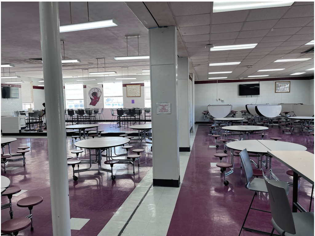
Figure 12 – Expansion joint that separates demo and what's to remain
