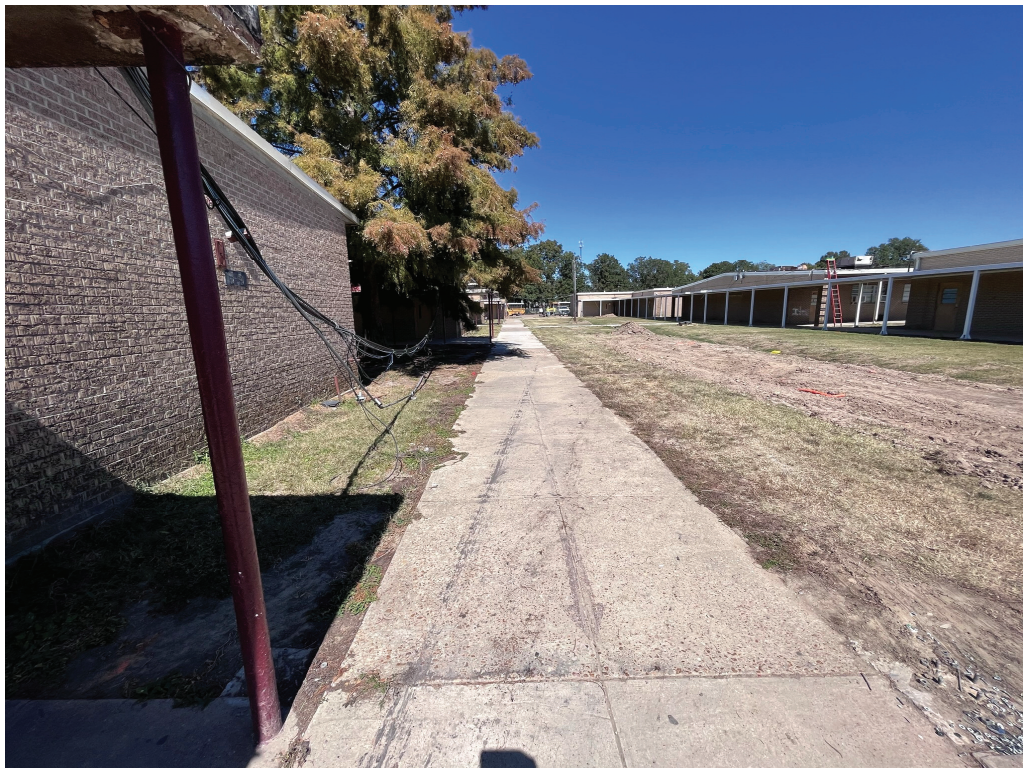
Figure 8 – Central open yard
