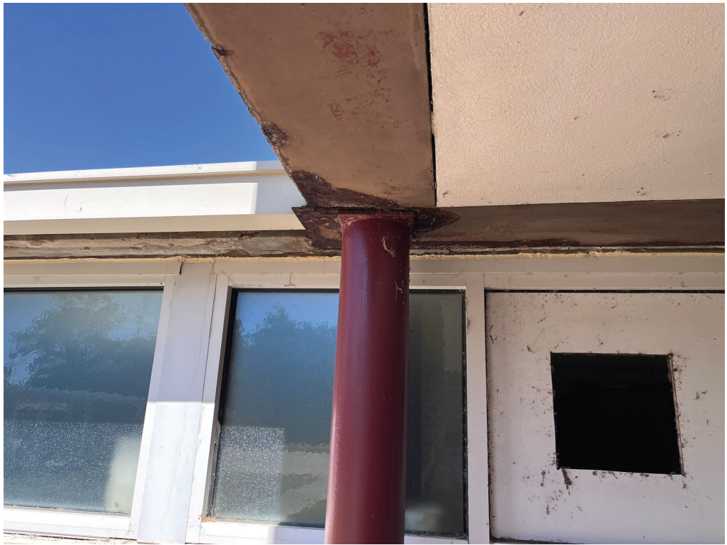
Figure 15 – Beam Column to be removed
