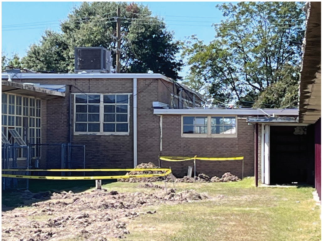
Figure 20 – SW Admin Building to be partially demolished
