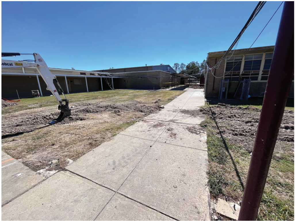
Figure 7 – Central Open Yard
