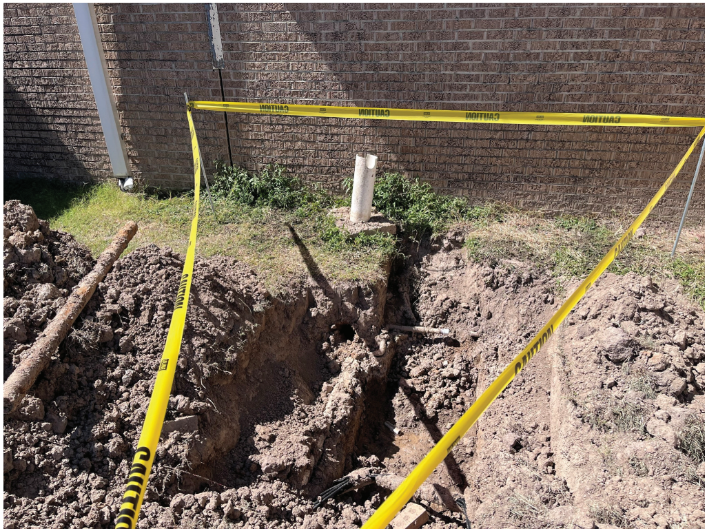
Figure 5 – Exploratory Excavation
