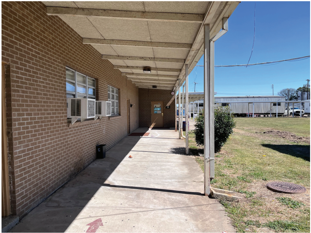
Figure 17 – South porch roof to be cleaned up and painted
