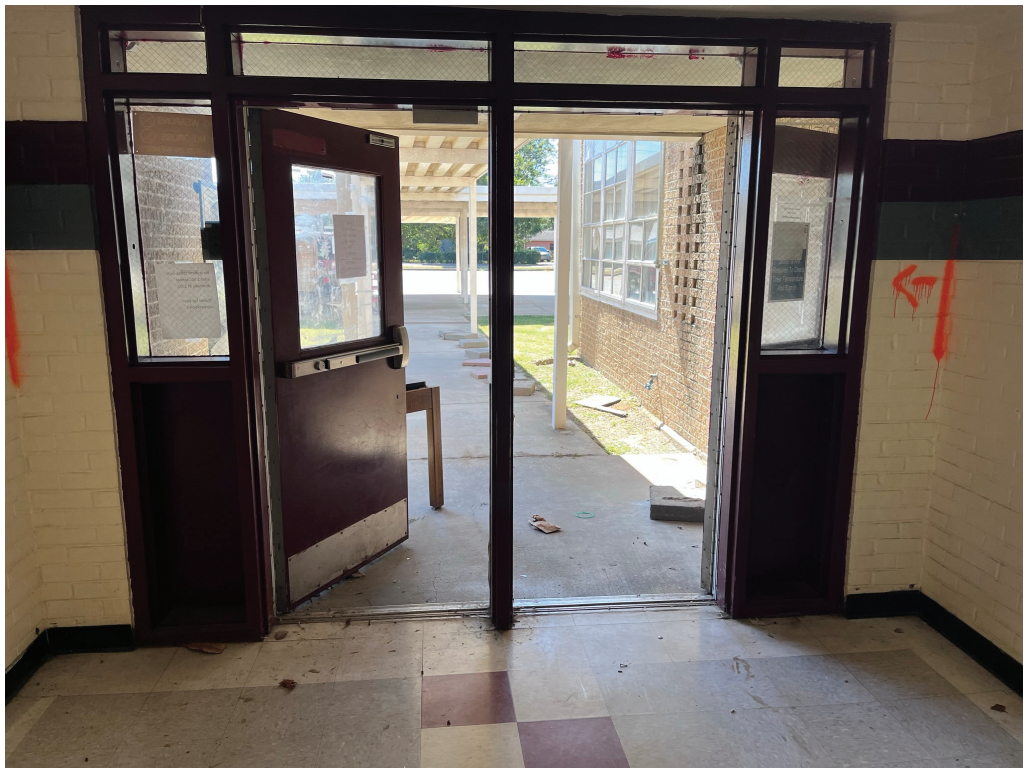
Figure 4 – Doors at SW Admin area to be demolished
