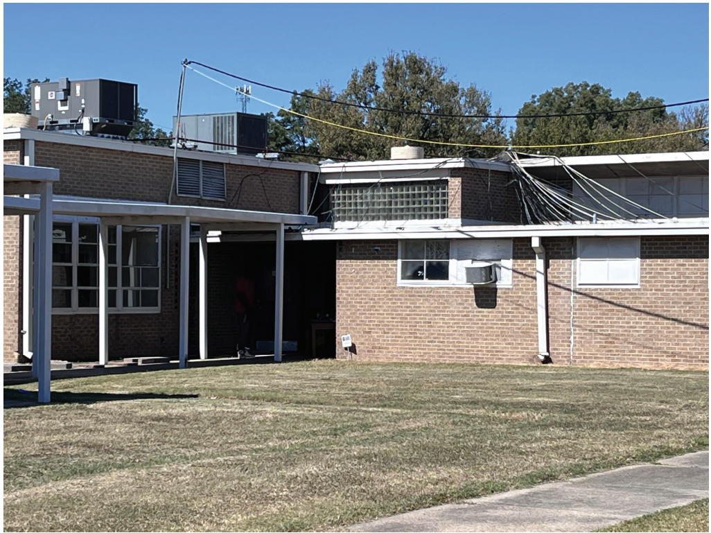
Figure 19 – SW Admin Building to be partially demolished
