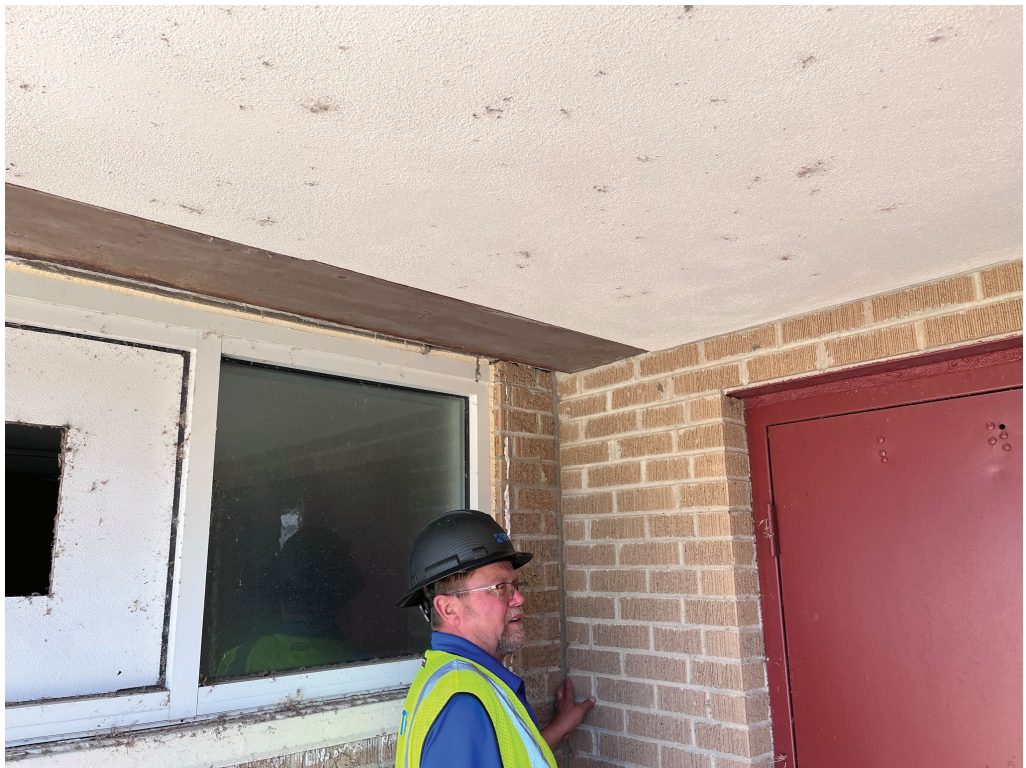
Figure 16 – Beam thru wall
