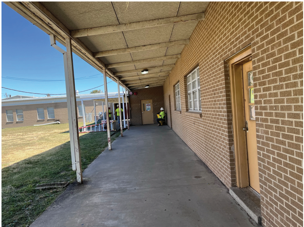
Figure 18 – North porch roof to be cleaned up and painted
