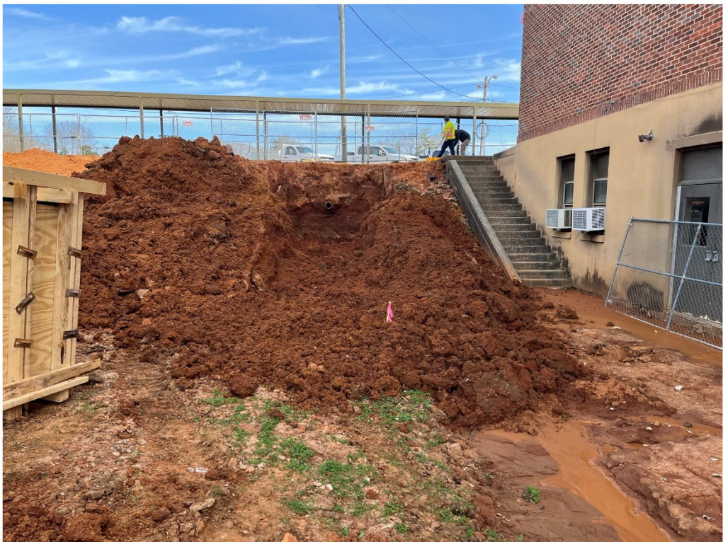
Figure 10 – Excavation @ JH Ramp
