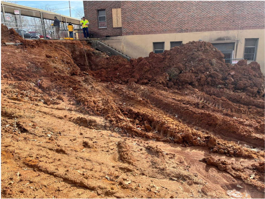
Figure 7 – Excavation @ JH Ramp
