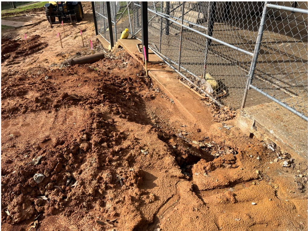
Figure 9 – Protective Site Barriers in Place
