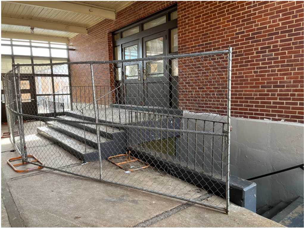
Figure 11 – Site Protective Barriers
