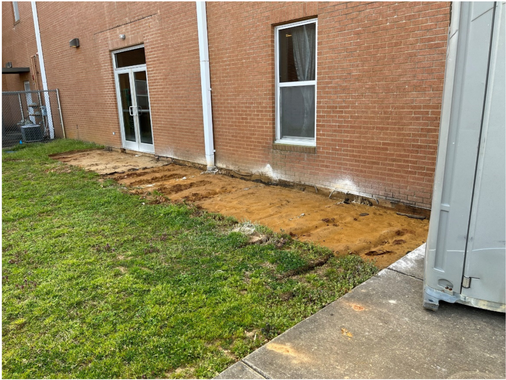
Figure 5 – HS Sidewalk Demo
