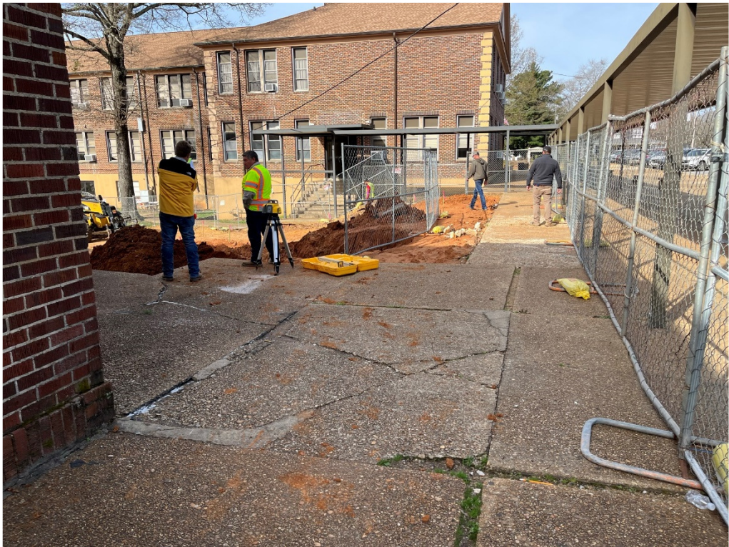
Figure 8 – JH Ramp Progress from Above
