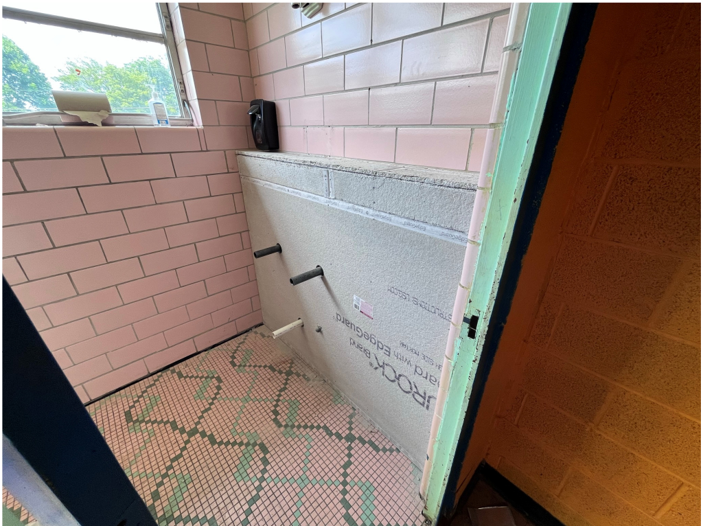
Figure 16 – Drew Hunter Gym Toilets
