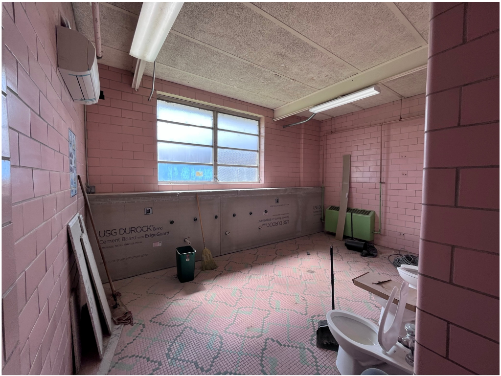
Figure 21 – AW James South Toilets
