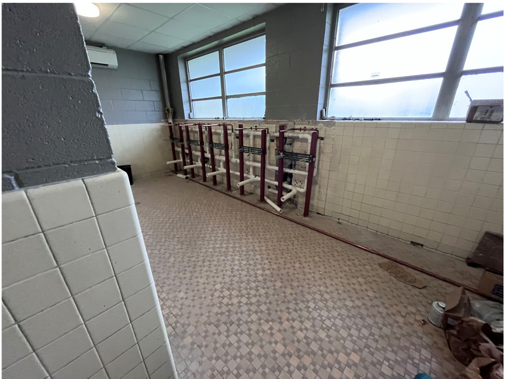
Figure 6 – Lockard North Wing Wall Carriers
