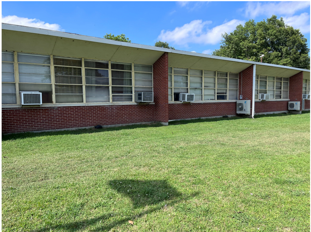
Figure 24 – RMS Exterior Unit Install
