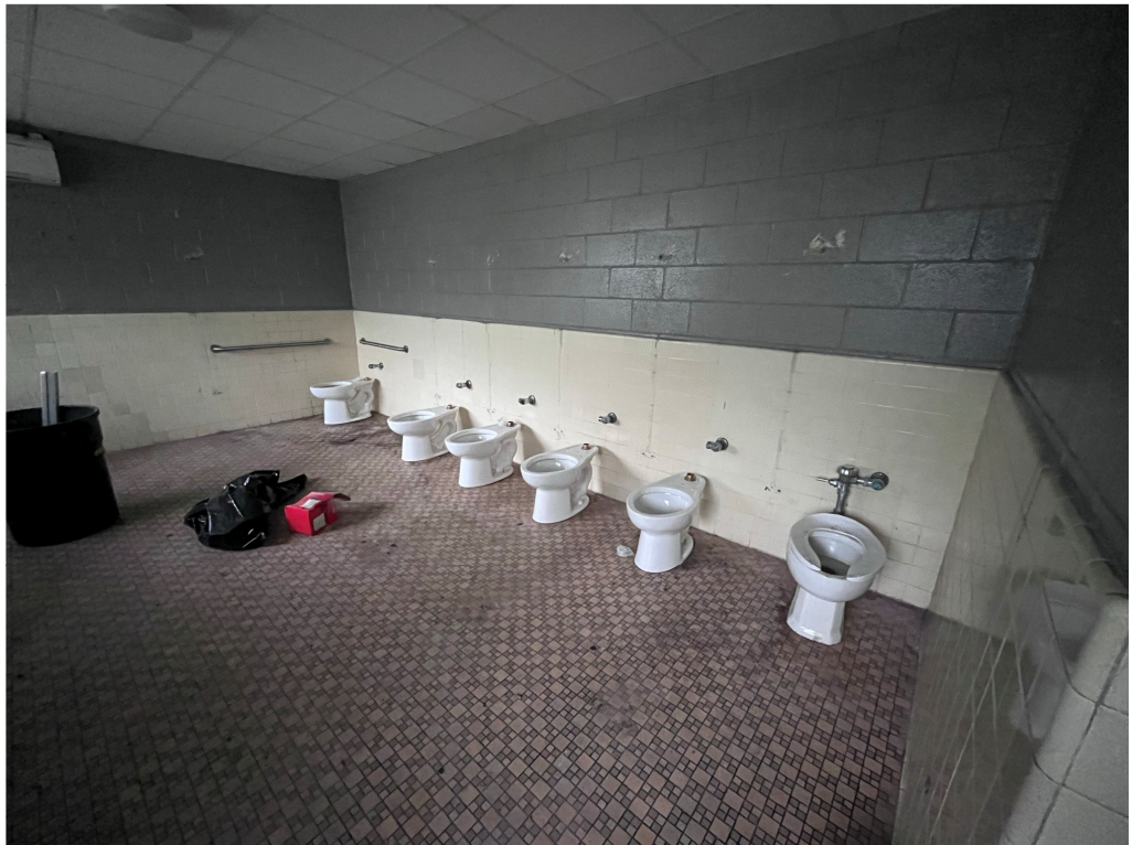
Figure 4 – Lockard North Wing Toilet Work
