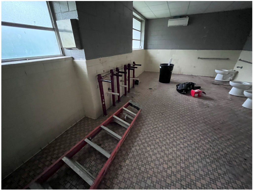
Figure 3 – Lockard North Wing Wall Carriers
