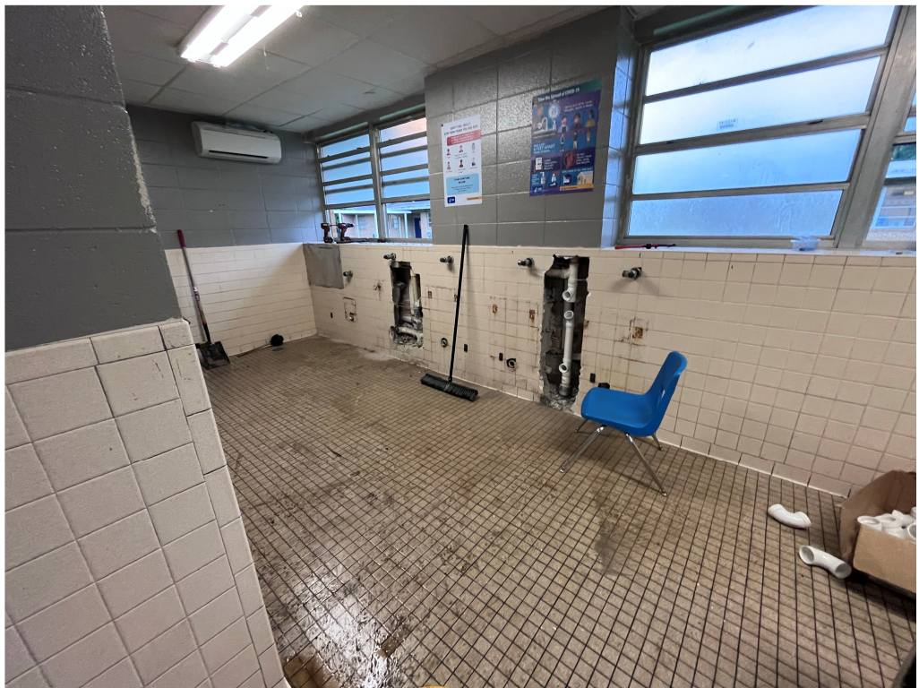
Figure 8 – Lockard 2 nd from North Wing Toilet Demo
