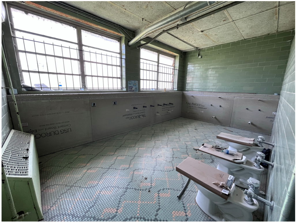
Figure 13 – Drew Hunter Central Toilets
