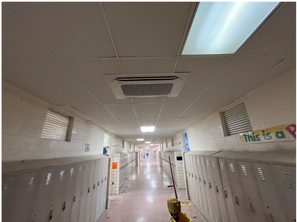
Figure 14 – Drew Hunter Typical Ceiling Unit Install
