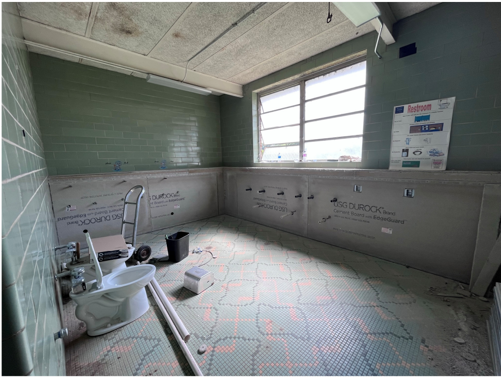
Figure 19 – AW James South Toilets
