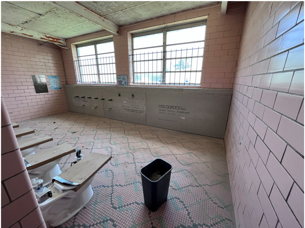
Figure 10 – Drew Hunter Central Toilets
