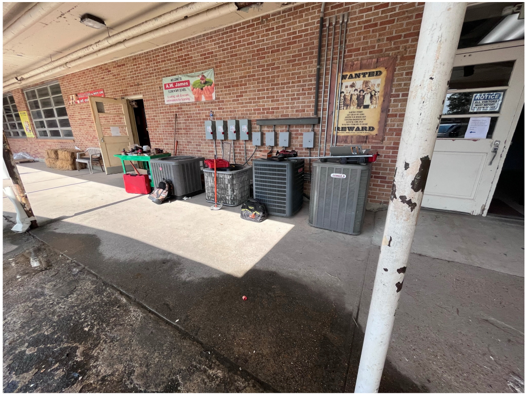
Figure 23 – AW James Electrical
