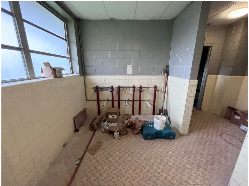
Figure 7 – Lockard North Wing Wall Carriers
