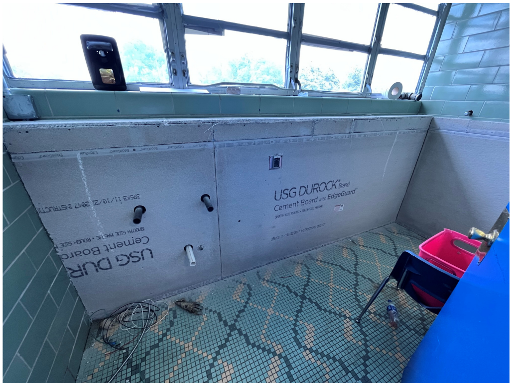
Figure 17 – Drew Hunter Gym Toilets
