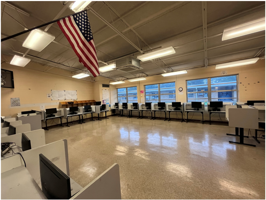
Figure 9 – Lockard Ceiling Unit Typical Install without Ceilings
