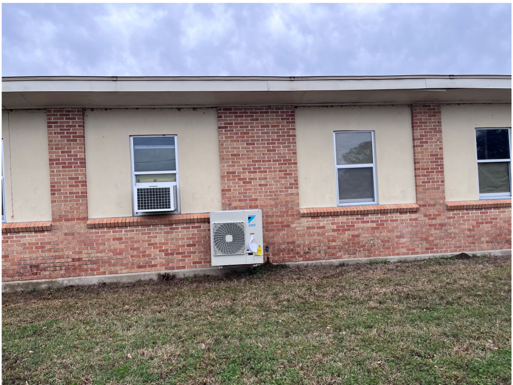
Figure 10 – Unit not centered or aligned on brick is not acceptable
