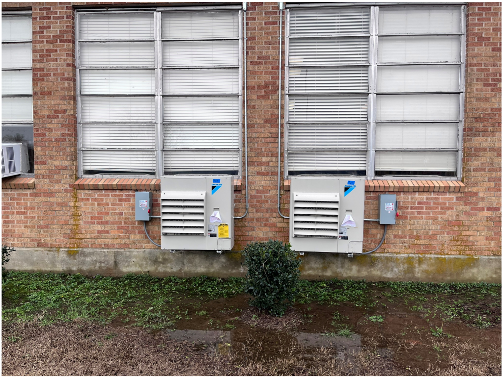
Figure 1 – Good Unit Install
