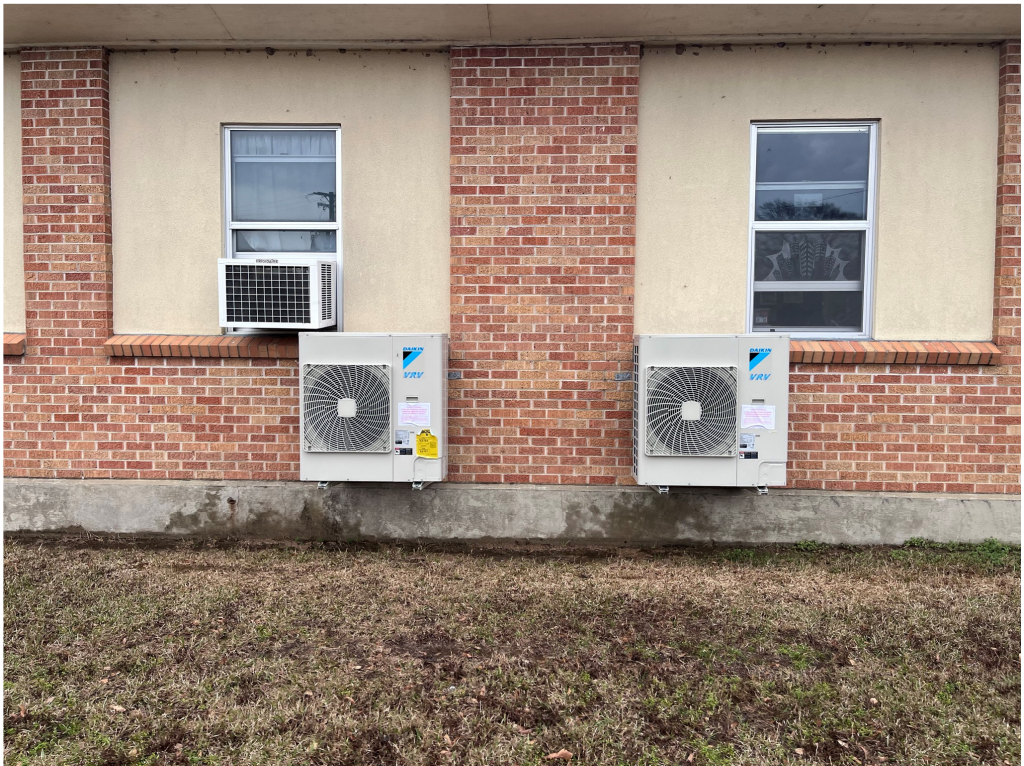
Figure 8 – Units lined up with brick edges are good installs
