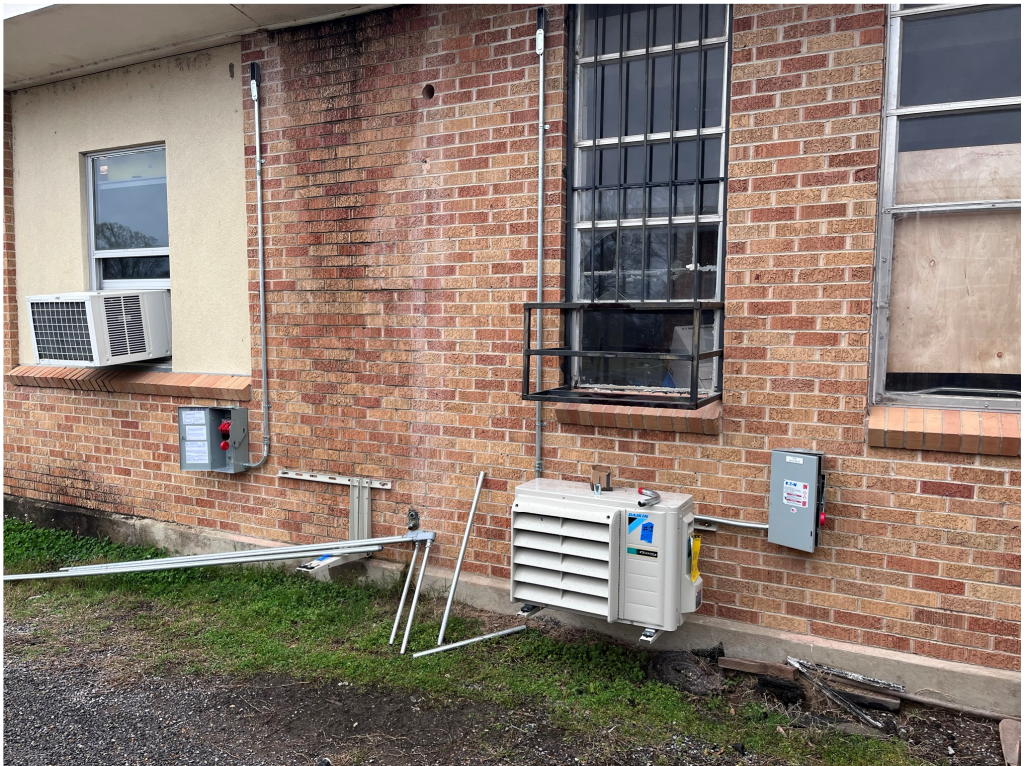
Figure 2 – Electrical Work is ongoing at Drew Hunter Middle
