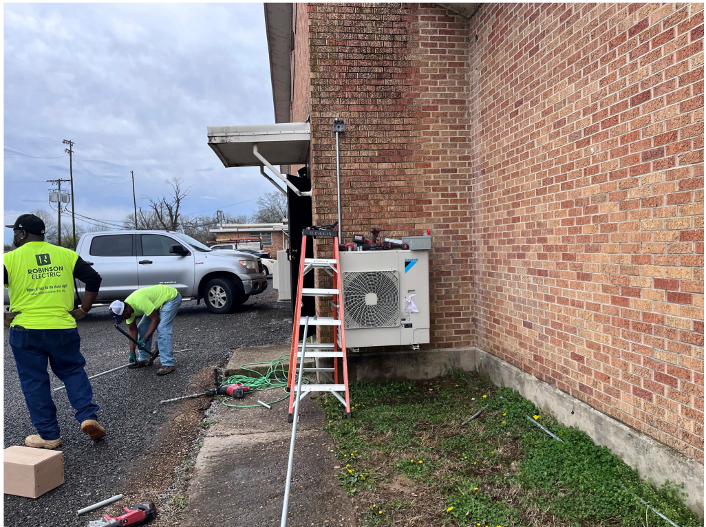
Figure 4 – Workers installing conduit
