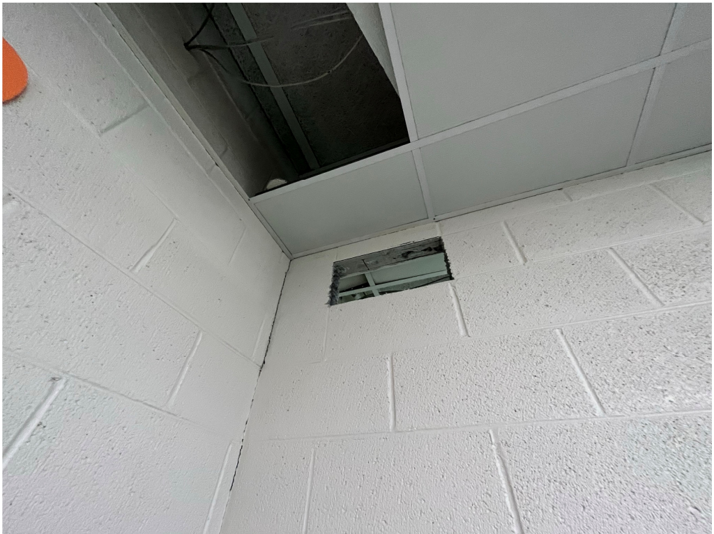
Figure 4 – Fresh air hole cut for ducting at Drew Hunter
