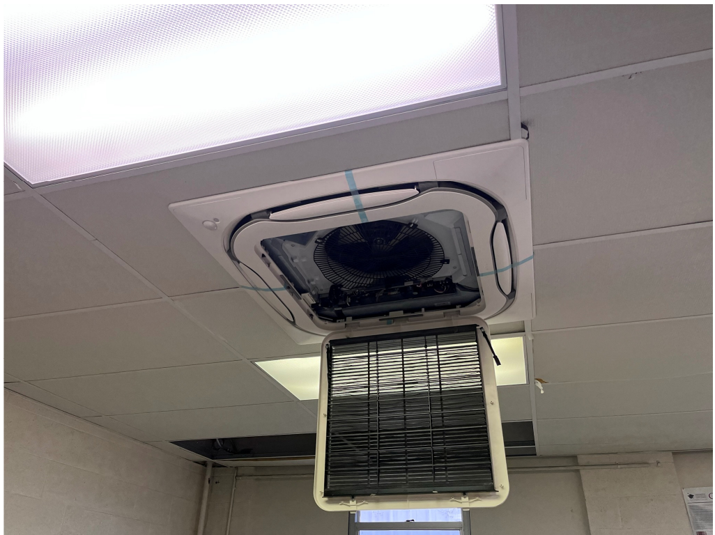
Figure 7 – Cassettes Installed at Drew Hunter
