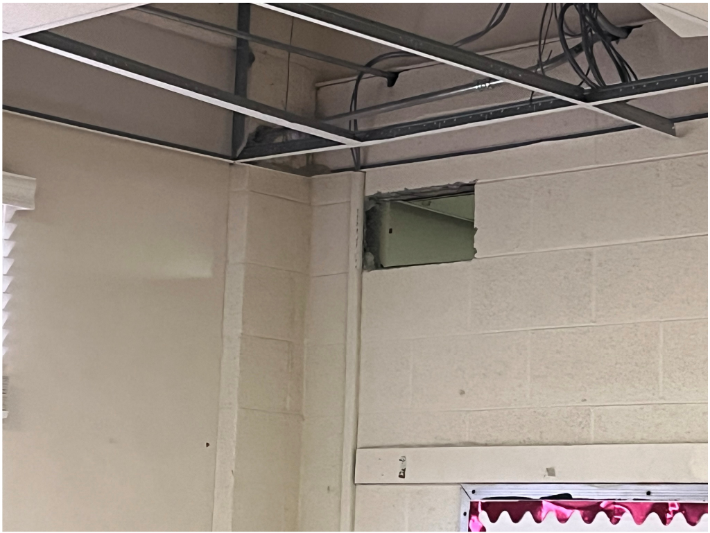
Figure 5 – Fresh air hole cut for ducting at Drew Hunter
