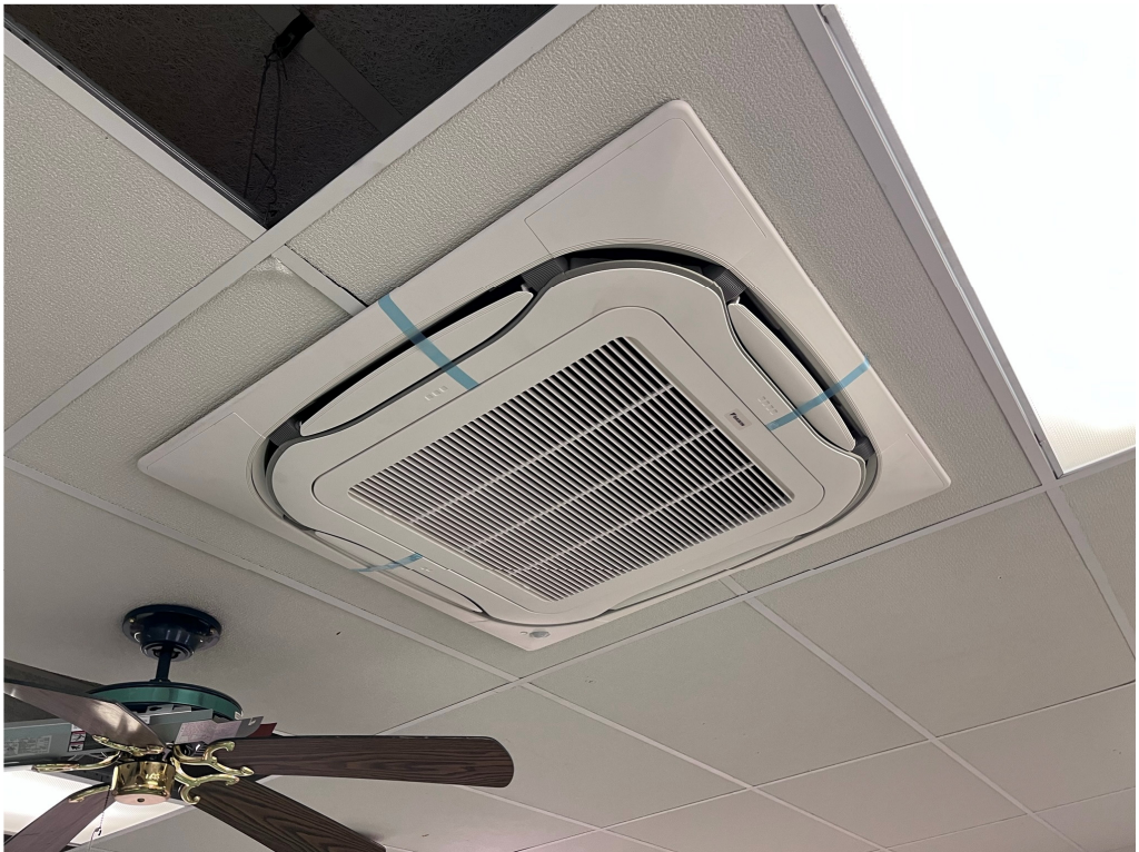
Figure 6 – Cassettes Installed at Drew Hunter
