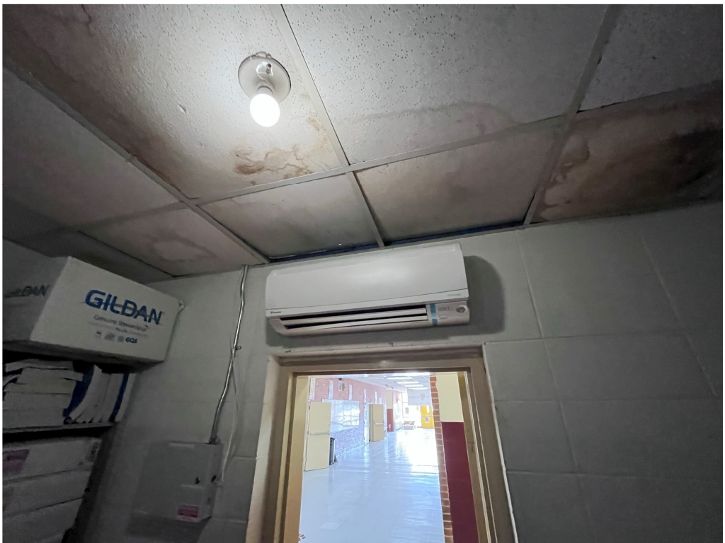
Figure 14 – Mounting height in low ceiling rooms (storage at Ruleville middle)
