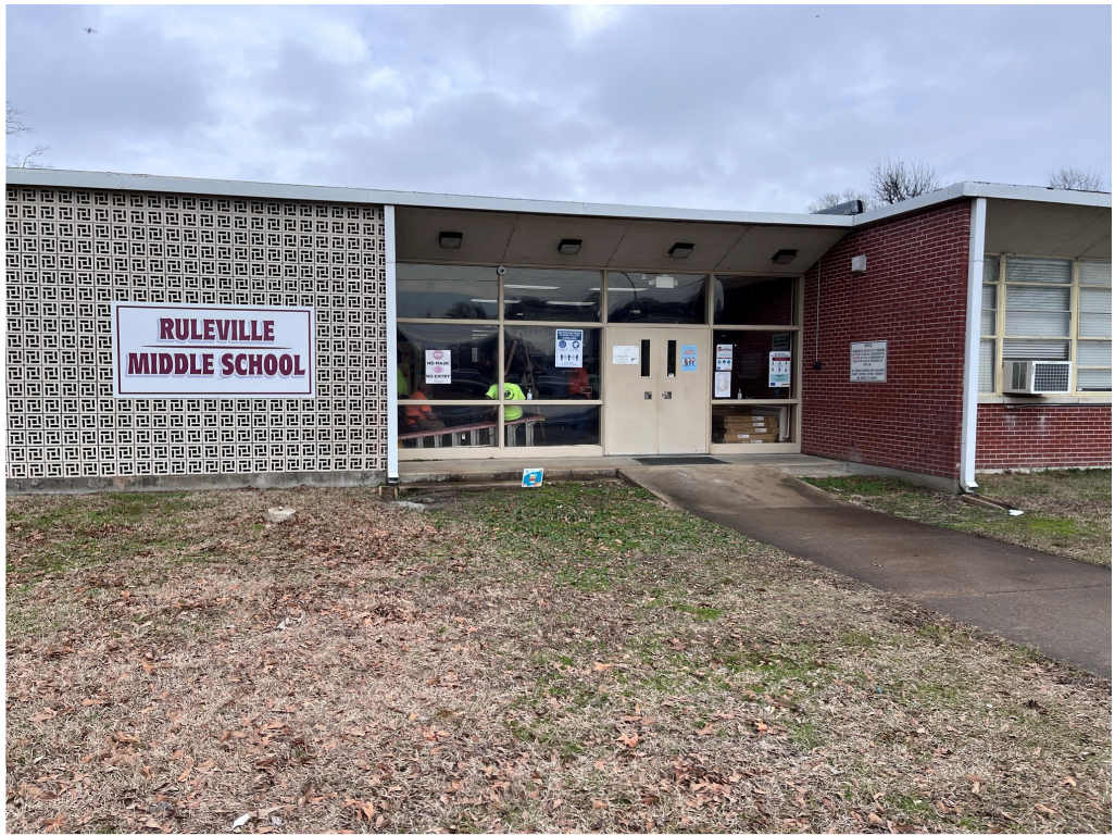
Figure 11 – Ruleville Middle work is ongoing
