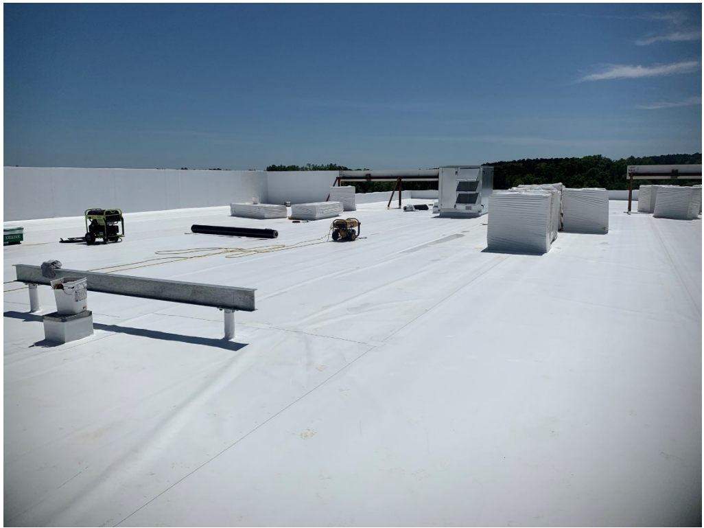
Figure 23 – Roofing Partially Installed
