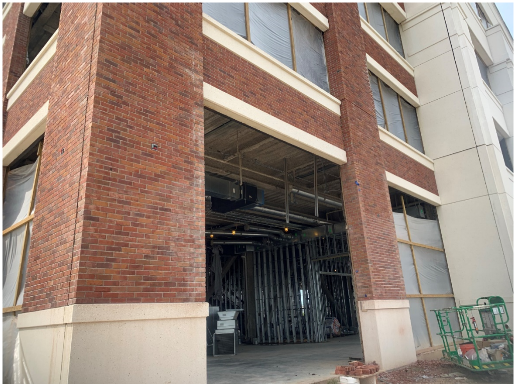
Figure 8 – Repairs to corner brick here (to be cleaned still)
