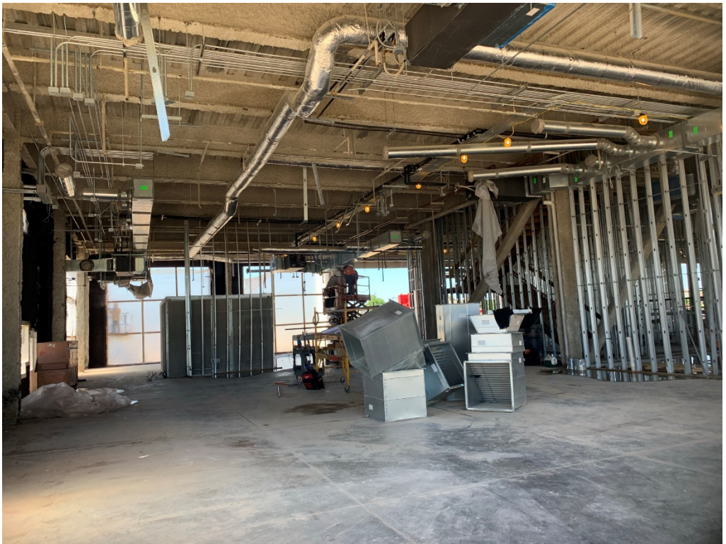
Figure 14 – Mechanical work is on going
