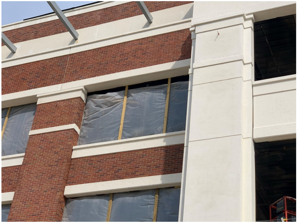
Figure 5 – Electrical Rough IN are not centered
