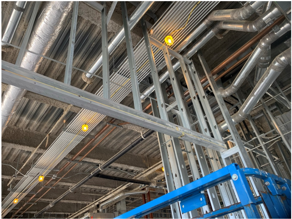
Figure 15 – Track is cut short exposing wood
