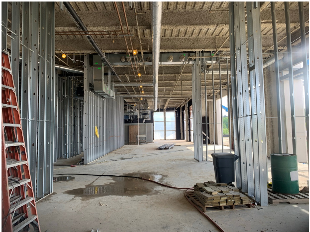
Figure 12 – First Floor at entry Looking South
