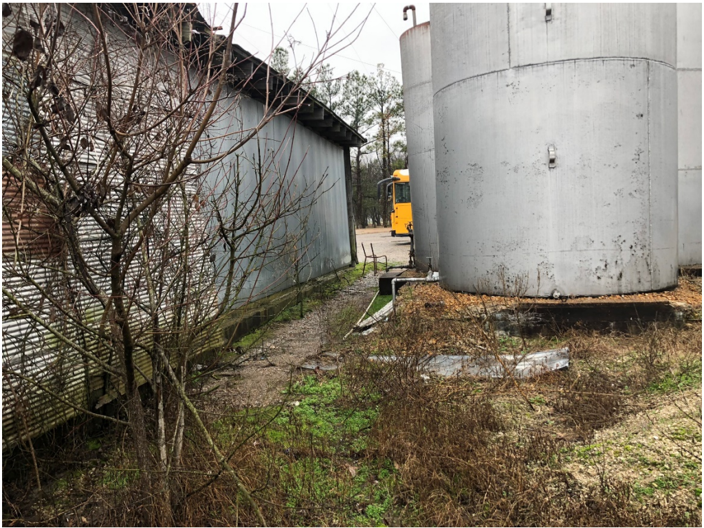
Figure 7 – North side & Fuel Tanks
