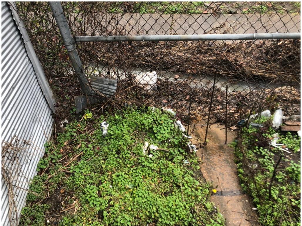
Figure 6 – Drainage Ditch @ East (no issues with overflow)
