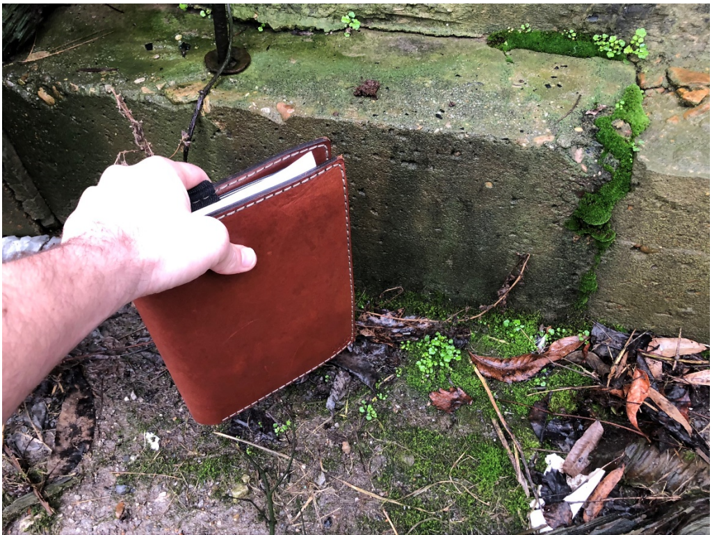
Figure 8 – 8" Existing Slab shown at North @ Wash Bay Slab
