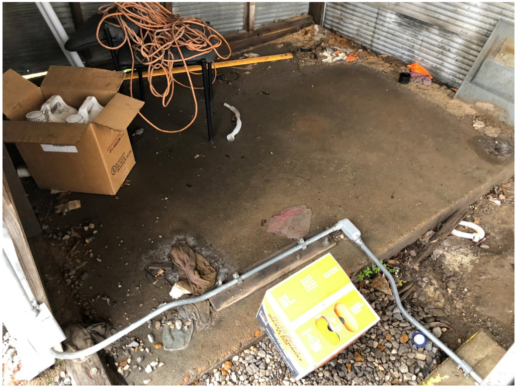
Figure 11 – Pump Storage Slab
