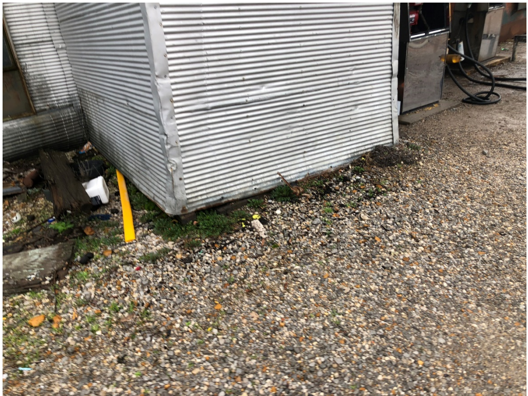
Figure 10 – Gas Pump Storage room (2 sides walled and open on pump side)
