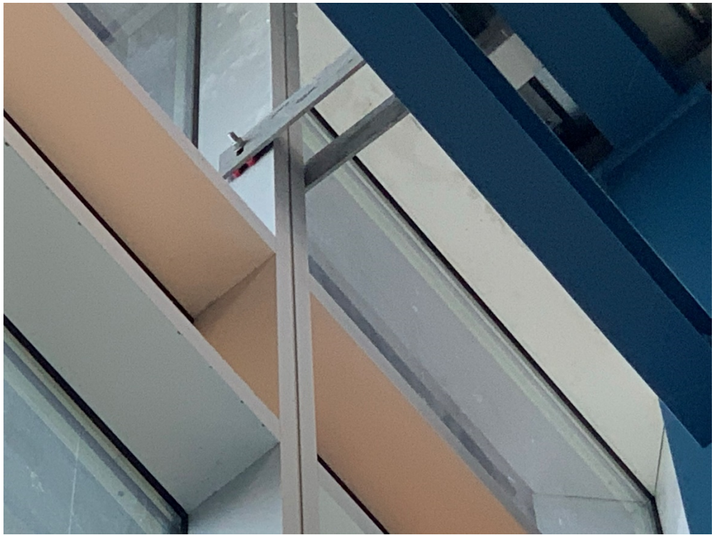
Figure 15 – All Shims need to be concealed Throughout
