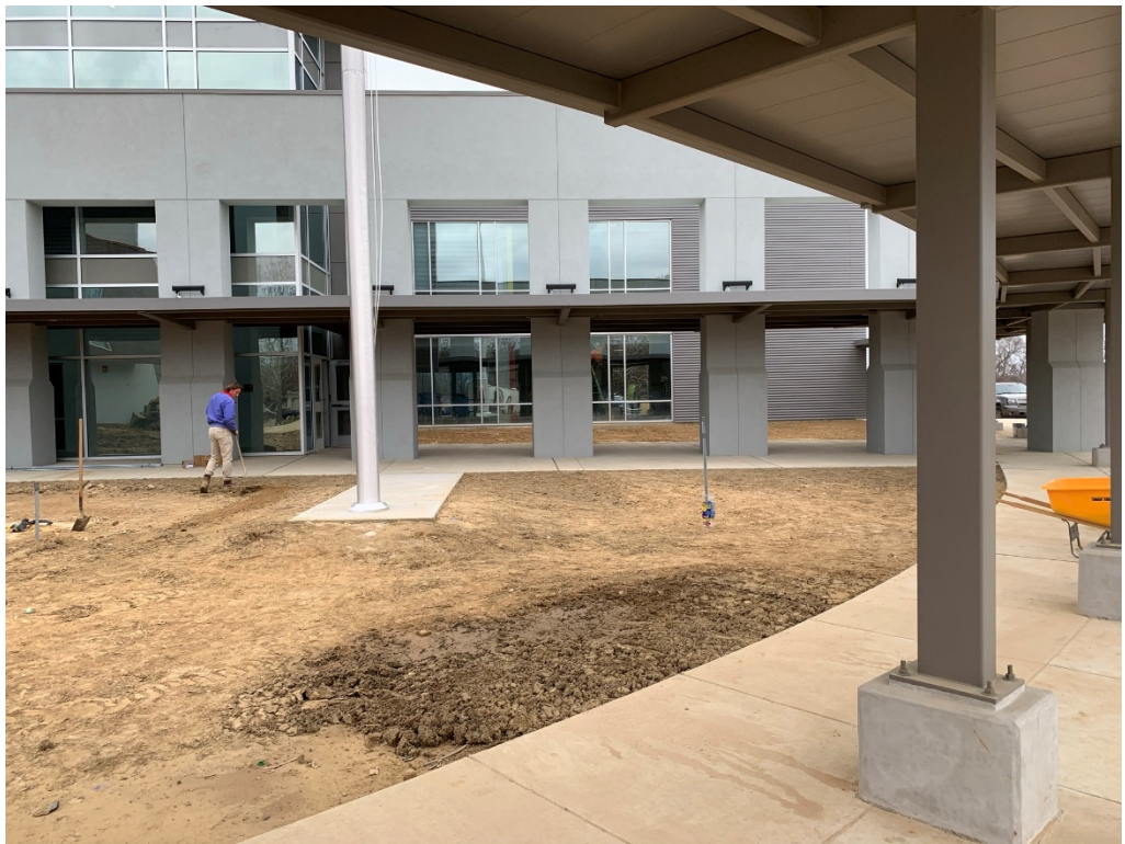
Figure 2 – Flag Pole Installed
