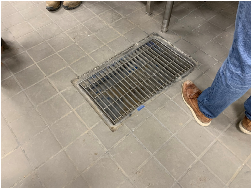
Figure 22 – Grates Need to be Raised in Kitchen flush with the Floor Tile
