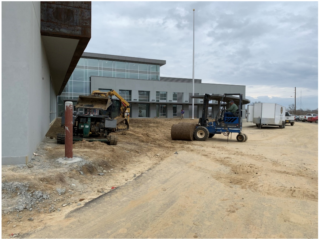
Figure 1 – Sod and grading at front courtyard
