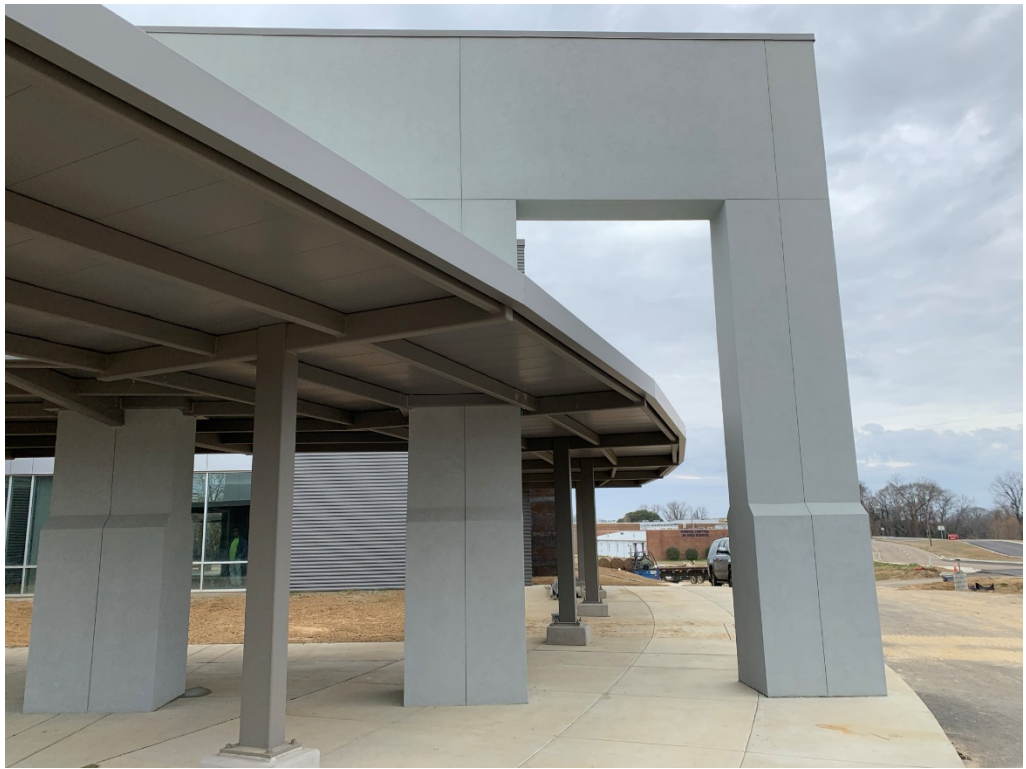
Figure 3 – Fixture Removed and Repair in Good Order
