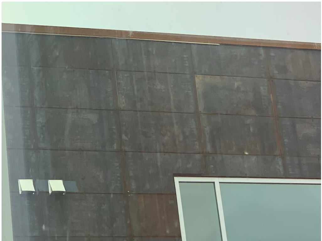
Figure 14 – Roof Membrane is exposed in some sections; This Membrane needs to be trimmed so that it is concealed from view
