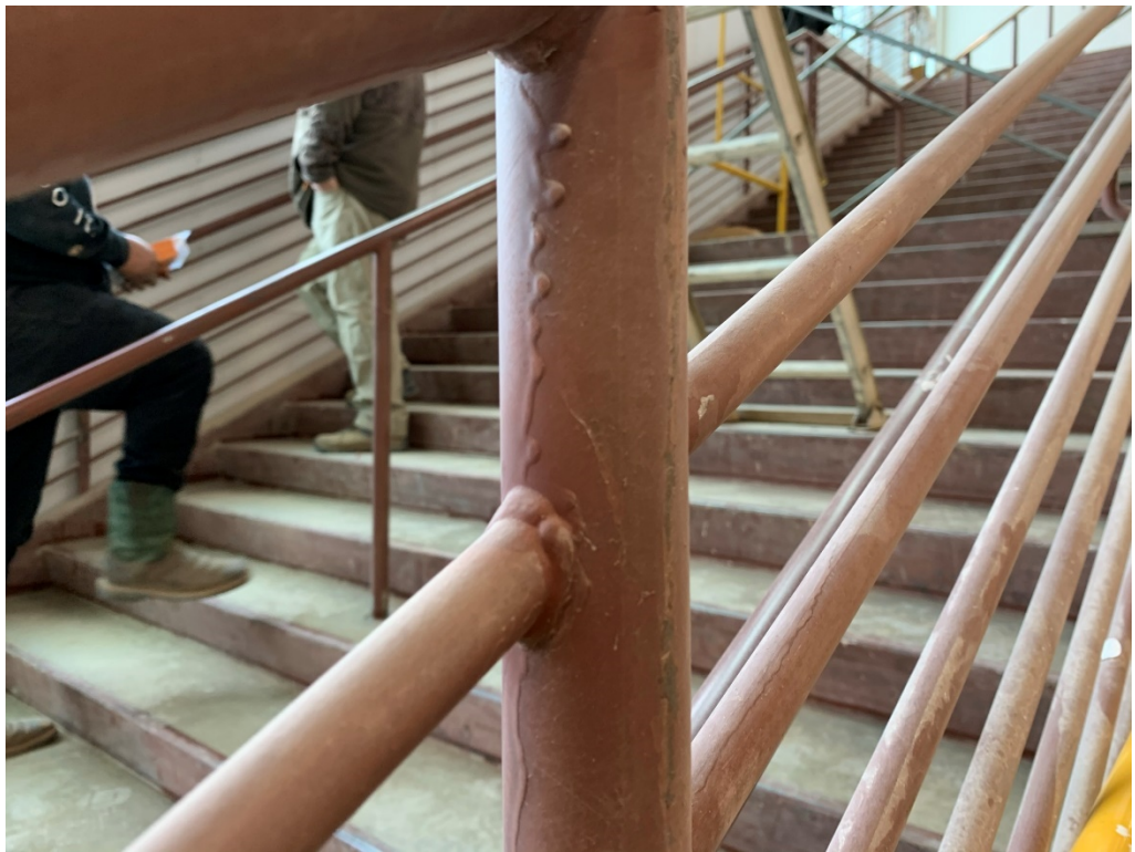
Figure 20 – Ensure that Paint is Sanded Smooth for Final Coat
