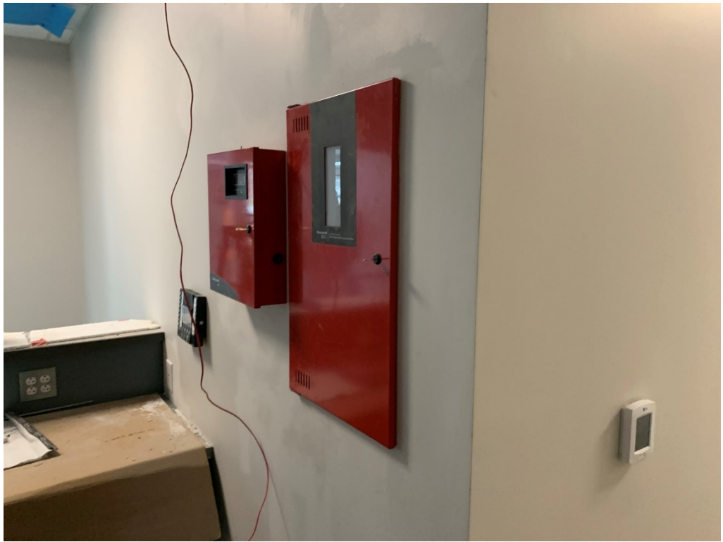
Figure 11 – Install Fire Equipment
