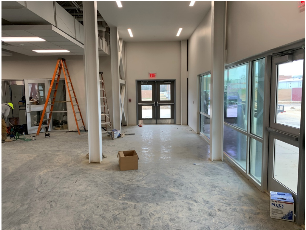
Figure 19 – Exit signs in a similar space need to be at the same height and centered on doors.
