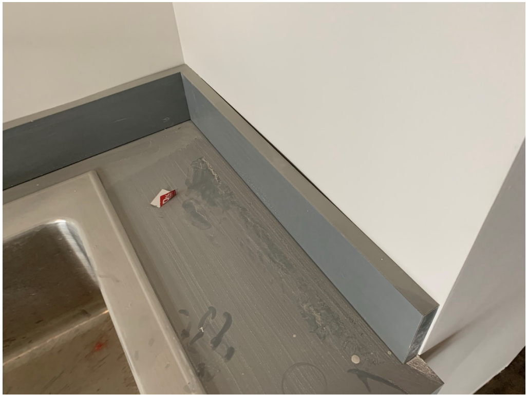
Figure 13 – Sealant is required at all backsplash/wall junctions
