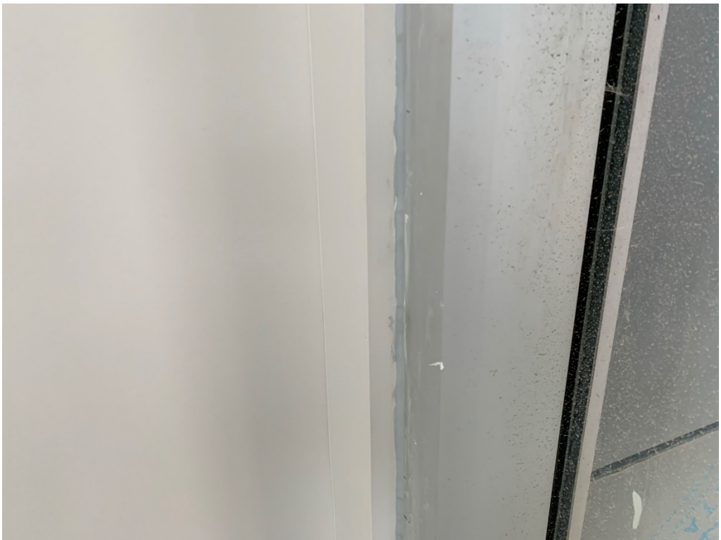
Figure 6 –All Sealant and paint lines need to be straight
