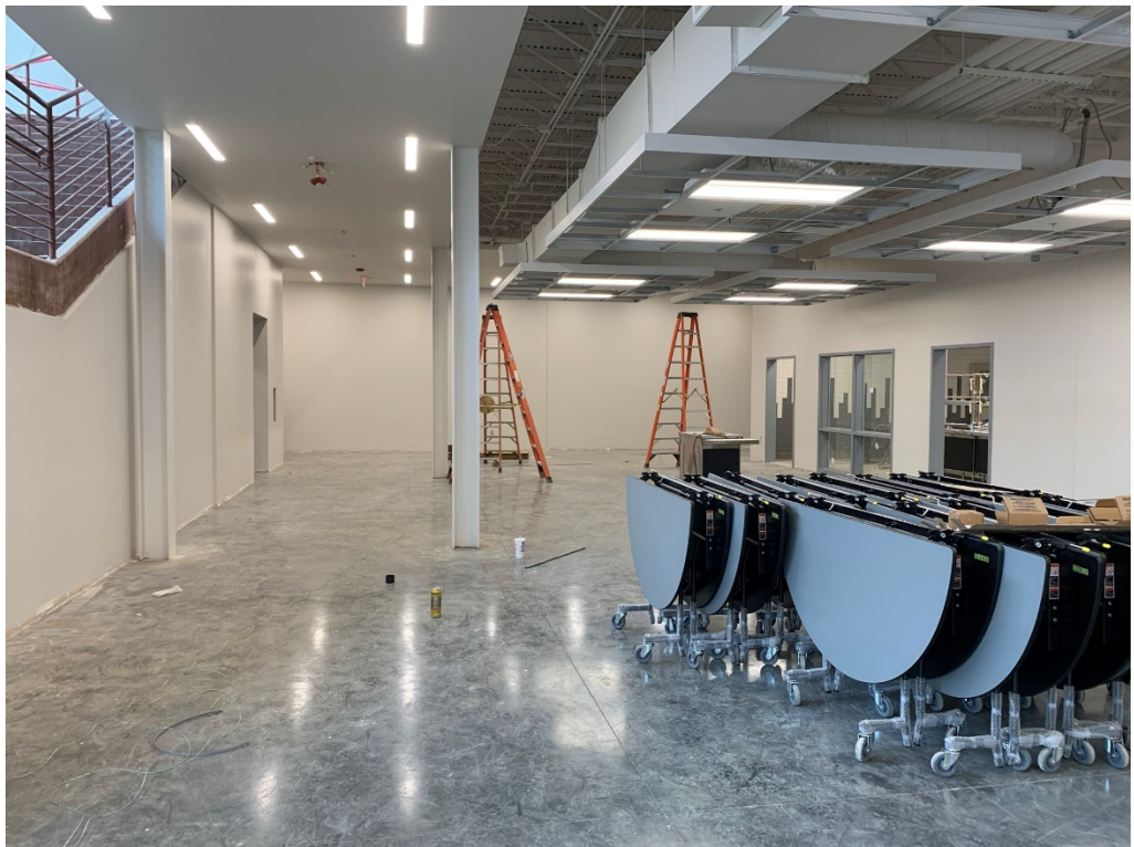
Figure 14 – Progress at Cafeteria
