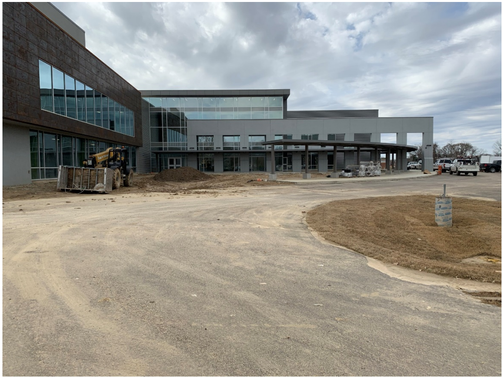
Figure 1 – Grass Installed at Site
