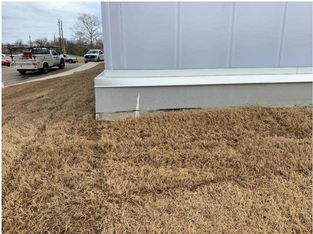
Figure 4 – Clean Up is Ongoing
