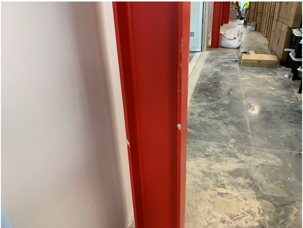
Figure 8 – Paint is Ongoing
