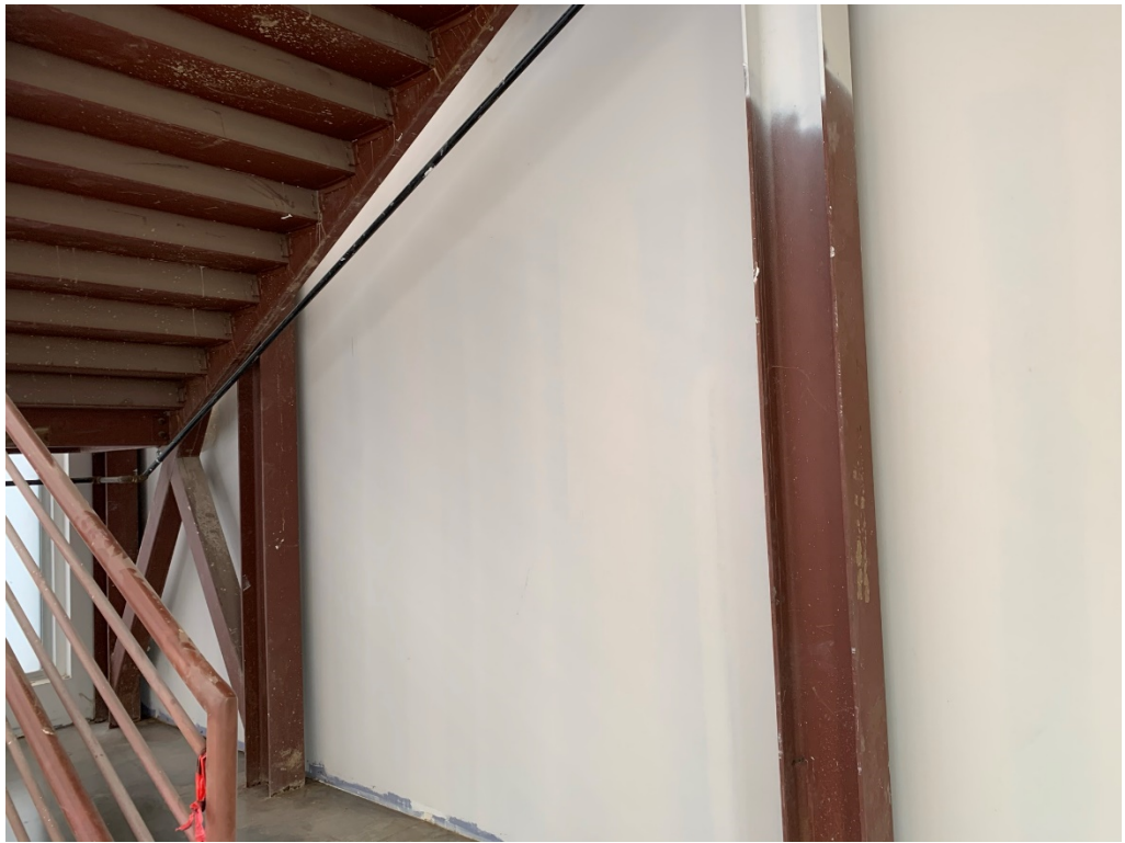
Figure 5 – Paint is Ongoing
