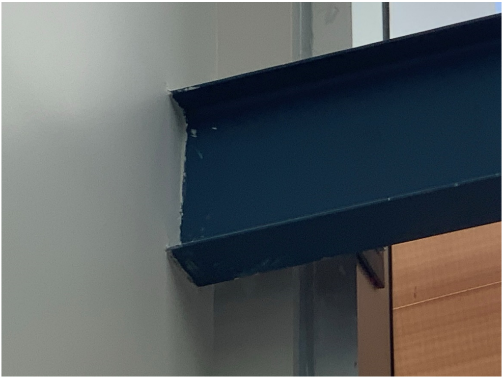
Figure 7 – Paint is Ongoing
