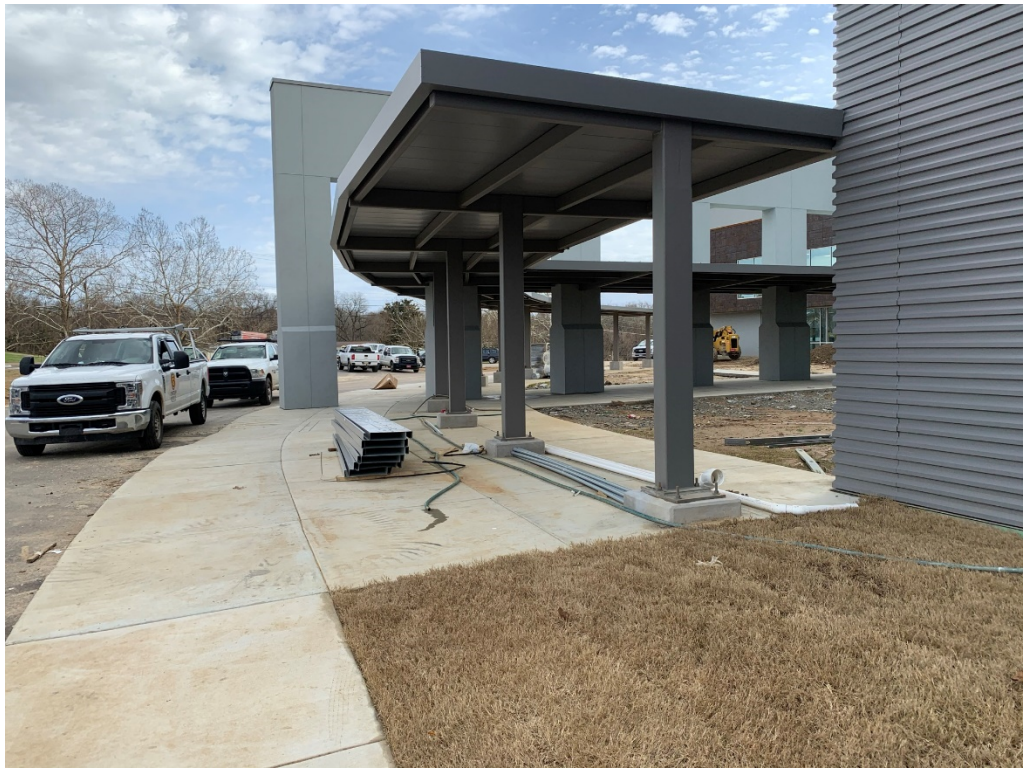
Figure 3 – Grass Installed at Site; Covered Awning Installation Appears Complete
