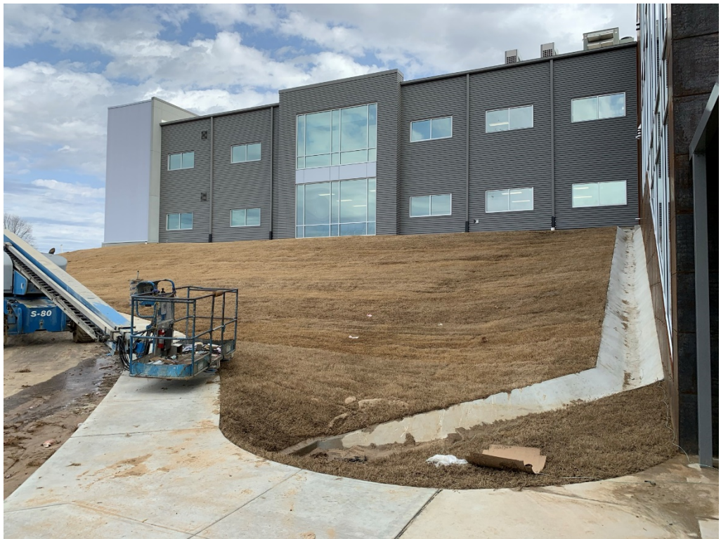
Figure 2 – Grass Installed at Site
