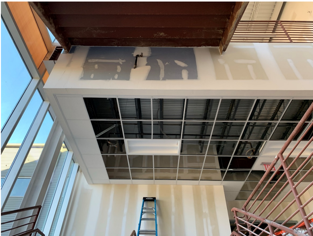
Figure 6 –Paint and Ceiling Install is Ongoing Throughout
