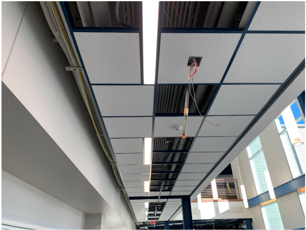
Figure 9 – Ceiling Grid Work Ongoing
