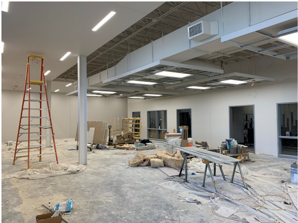
Figure 4 – Cafeteria Paint and Ceiling Install is Ongoing
