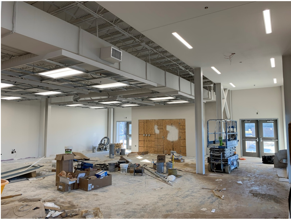
Figure 5 – Cafeteria Paint and Ceiling Install is Ongoing
