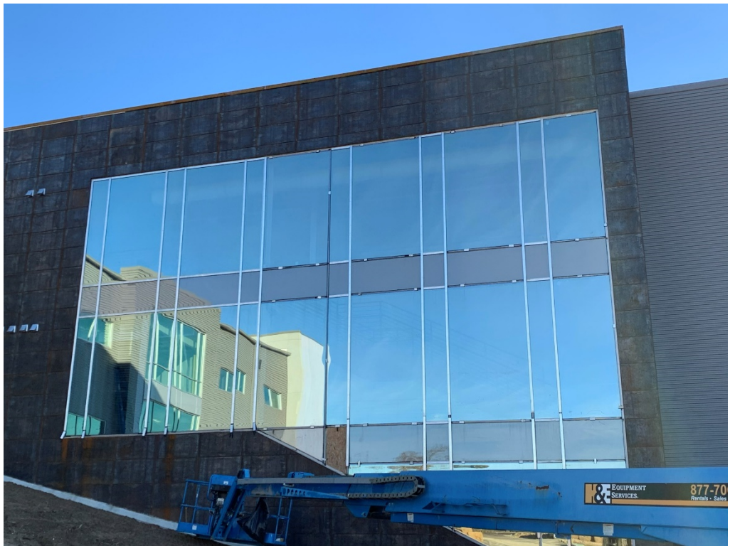
Figure 2 – Curtain Wall Installation is Ongoing
