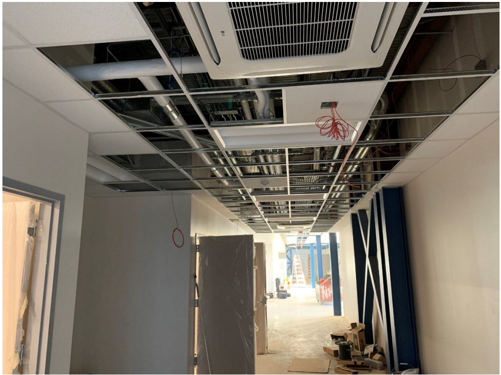
Figure 7 – Ceiling Grid Install is Ongoing Throughout
