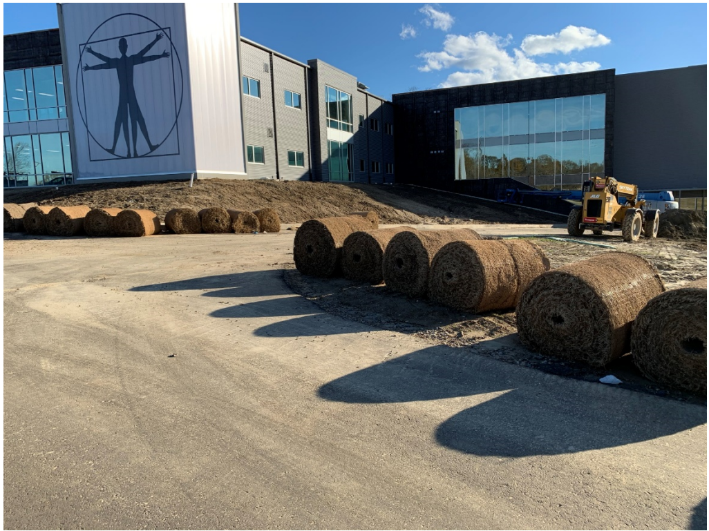
Figure 1 – Sod is on Site and Ready to Install
