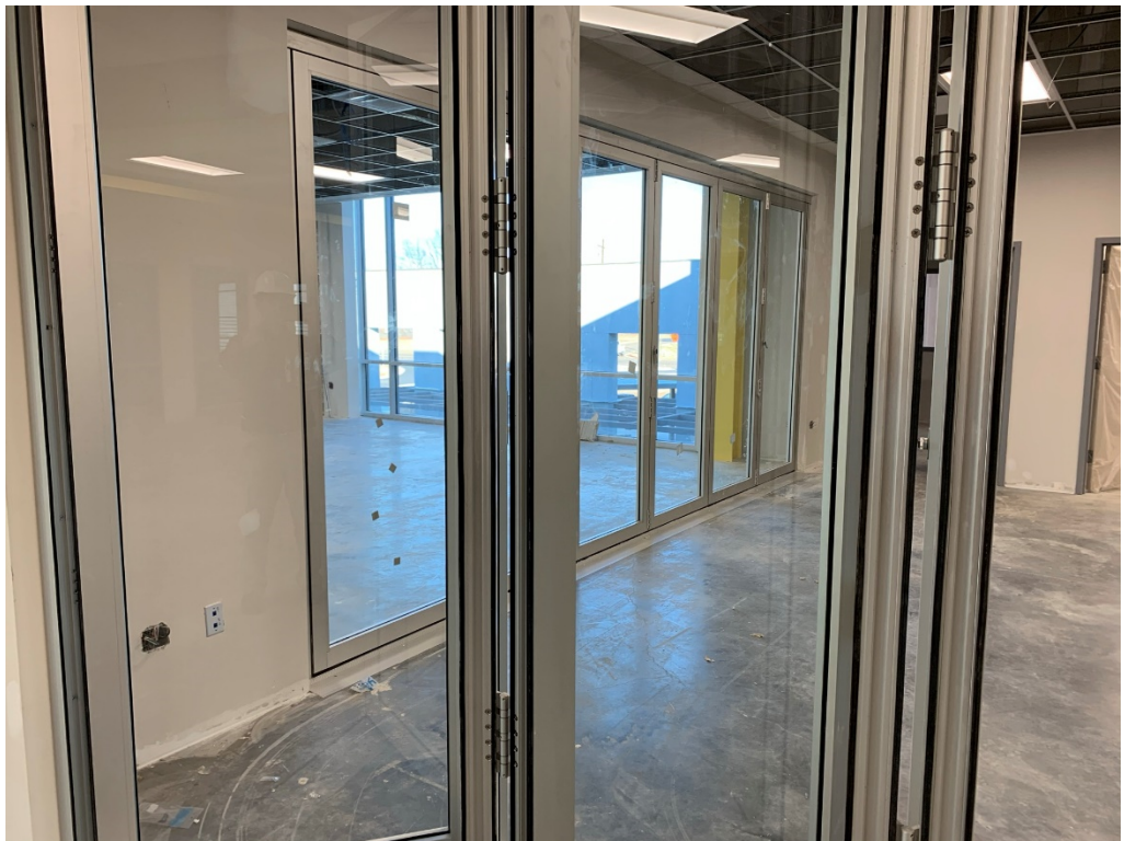
Figure 10 – Glass Installed at Moveable Partitions
