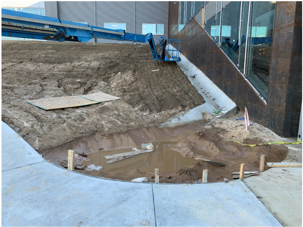
Figure 3 – Concrete Rework at Drop Off Entry
