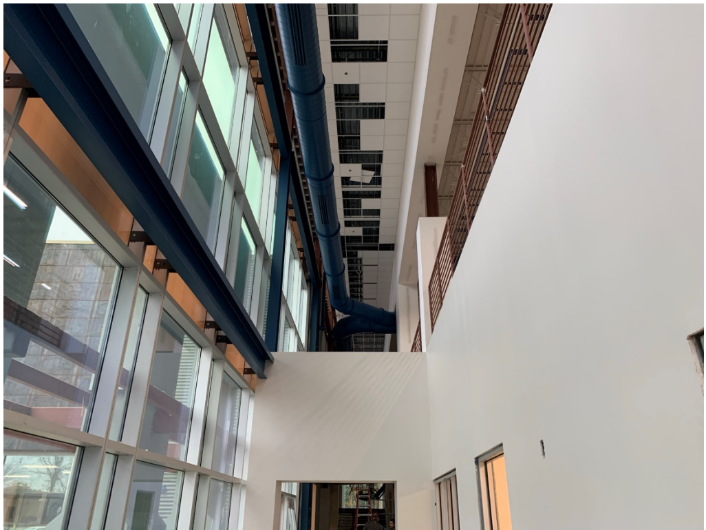
Figure 12 – Paint Work is Ongoing
