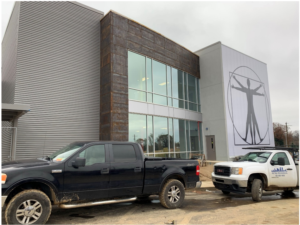
Figure 7 – North Central Façade
