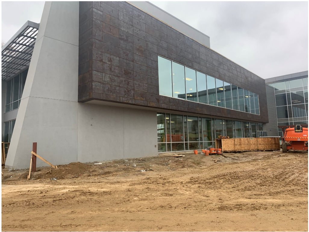
Figure 3 – North Façade at East Section of Building
