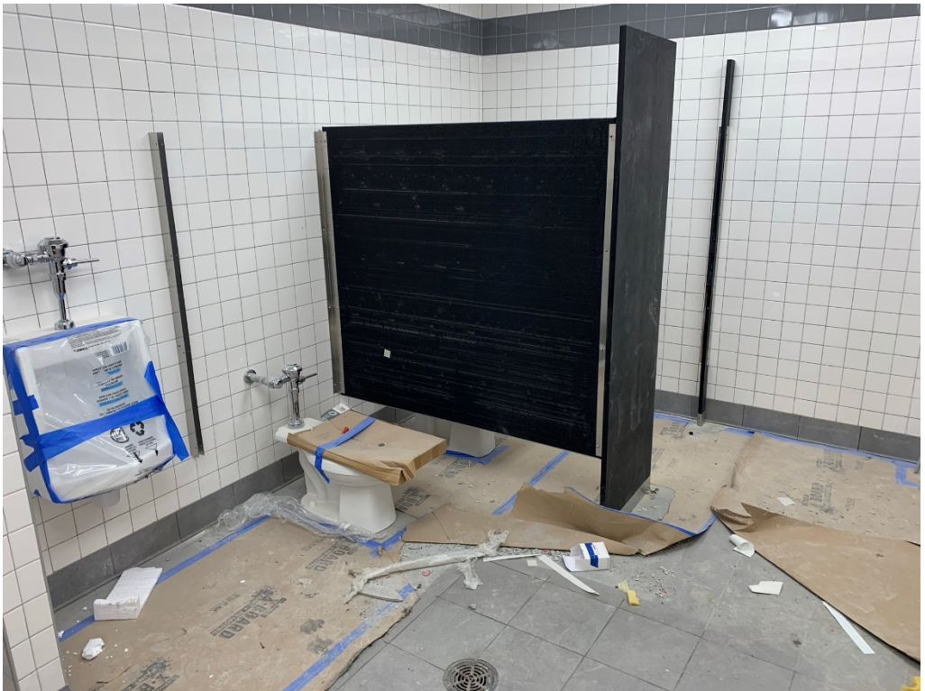
Figure 22 – Partition installation is ongoing
