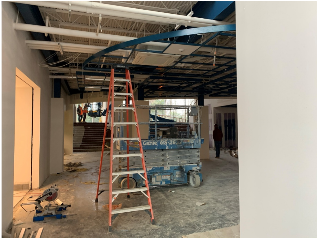
Figure 17 – Paint work at Lobby is ongoing
