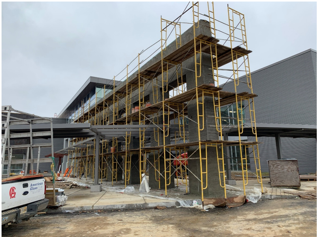
Figure 4 – Stucco work ongoing
