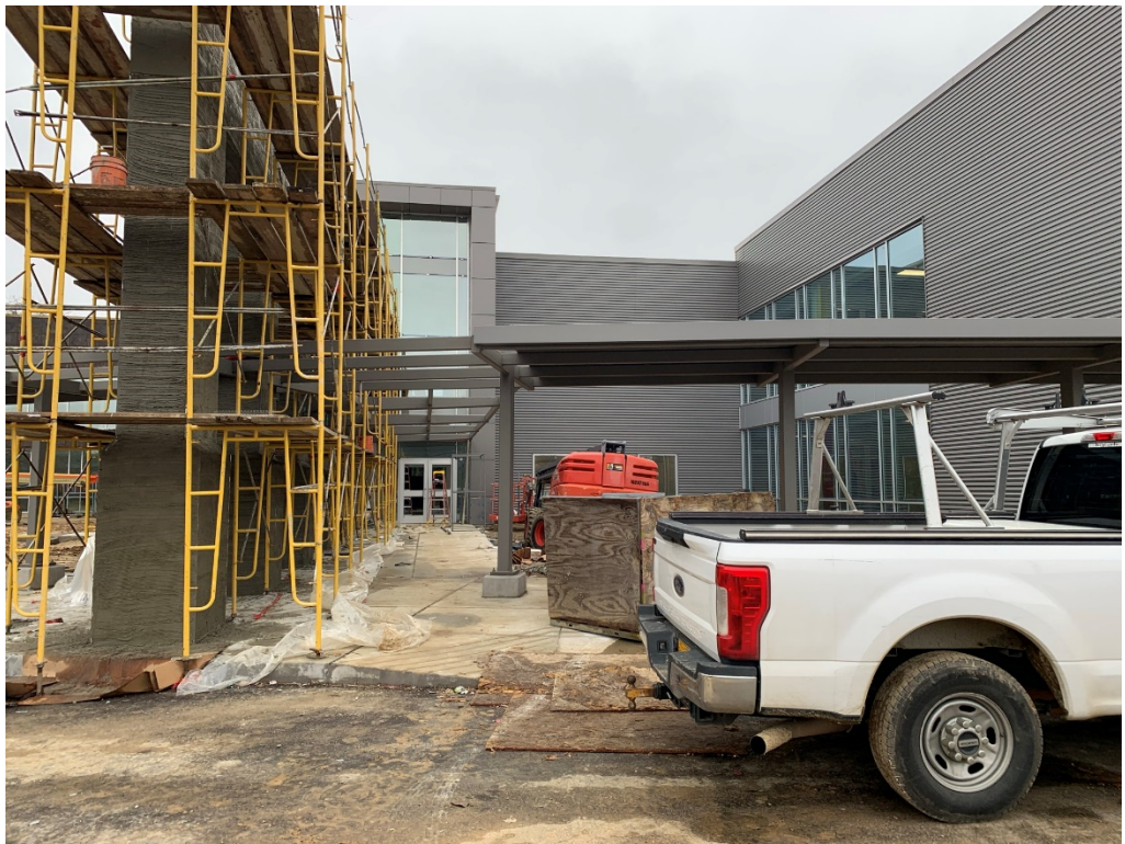
Figure 6 – North Central Façade
