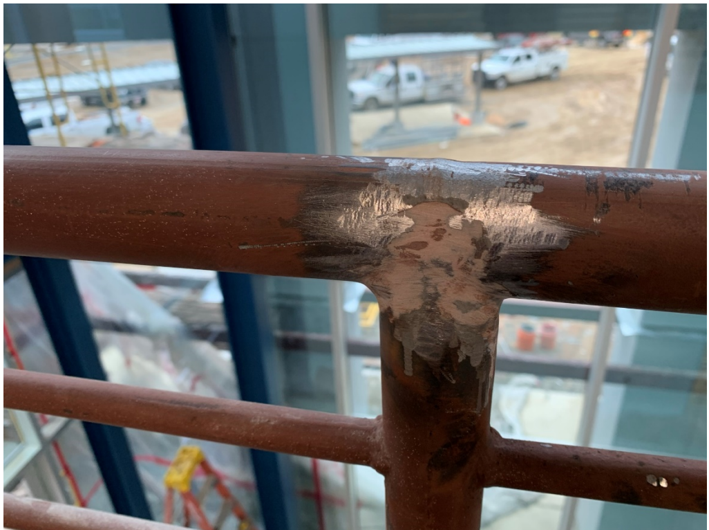
Figure 38 – Example of repair at handrail that should finish out well
