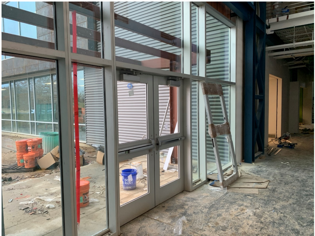
Figure 16 – Curtain wall and doors installed
