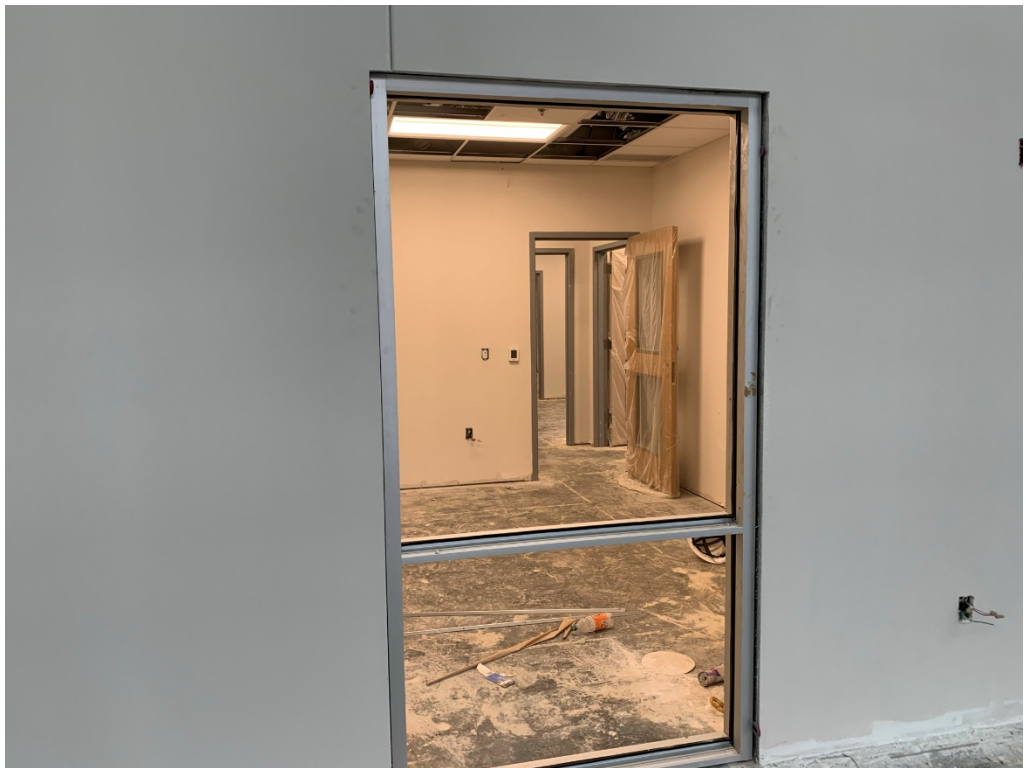
Figure 14 – Storefront at Main Entry
