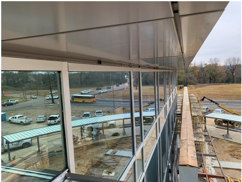
Figure 46 – Central Building Top of Storefront
