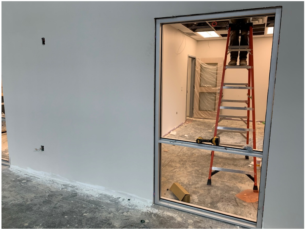
Figure 13 – Storefront at Main Entry
