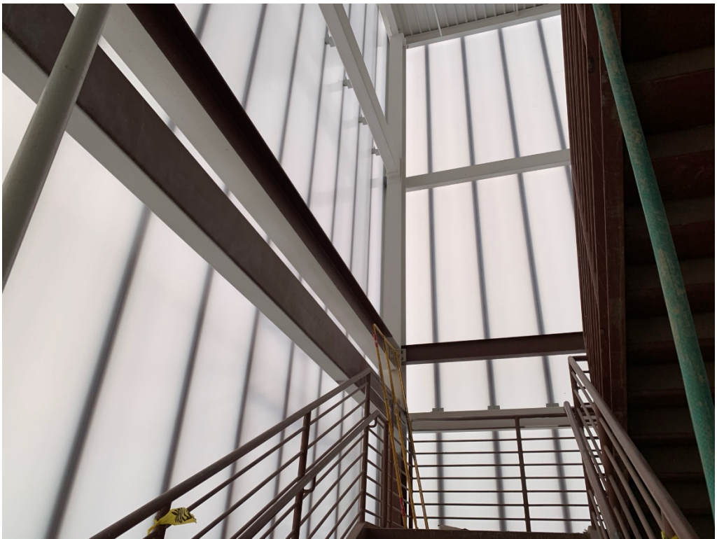
Figure 28 – SE Stair on going
