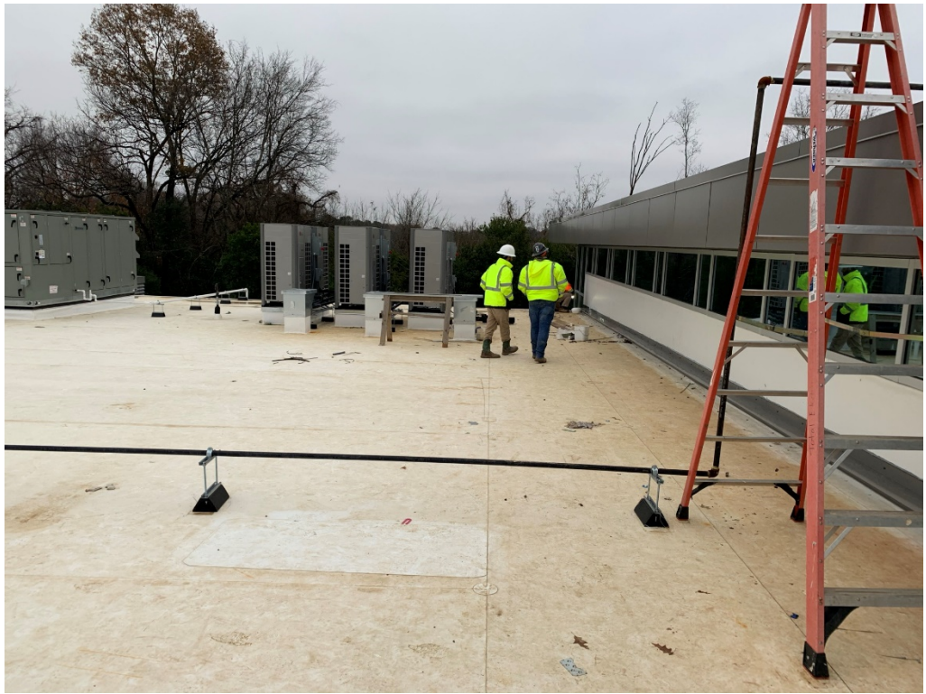
Figure 41 – Rooftop storefront Wall
