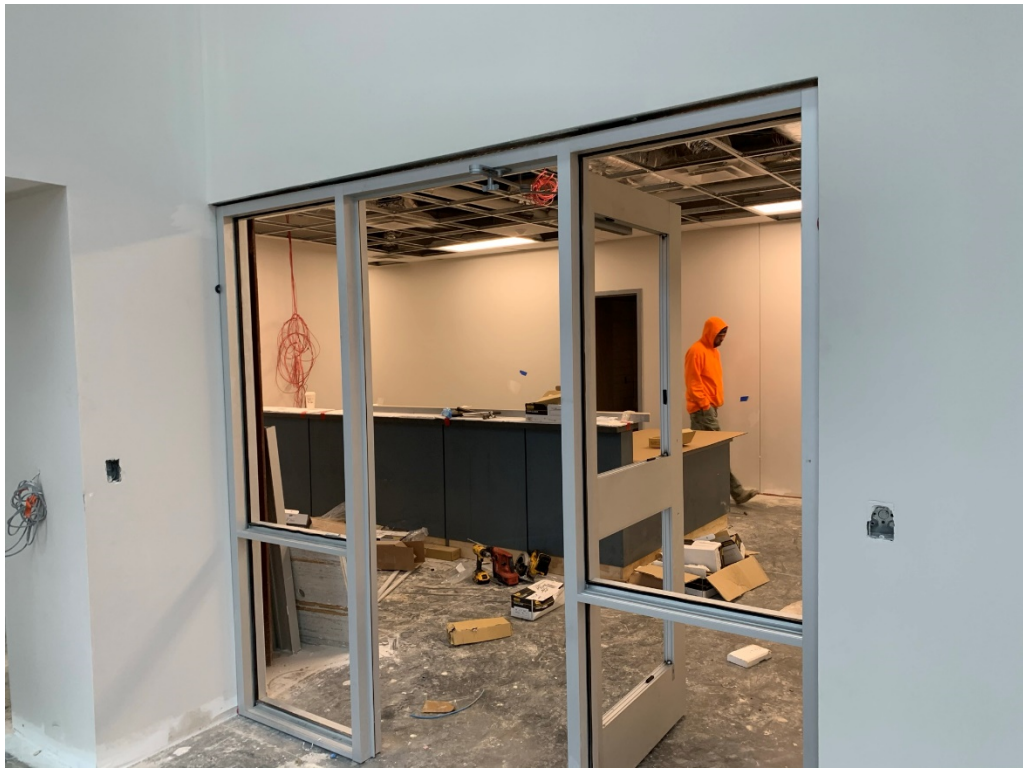
Figure 15 – Storefront at Main Entry
