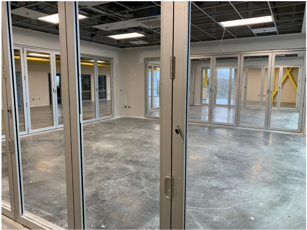
Figure 31 – Foldable Door Frames In Place Throughout
