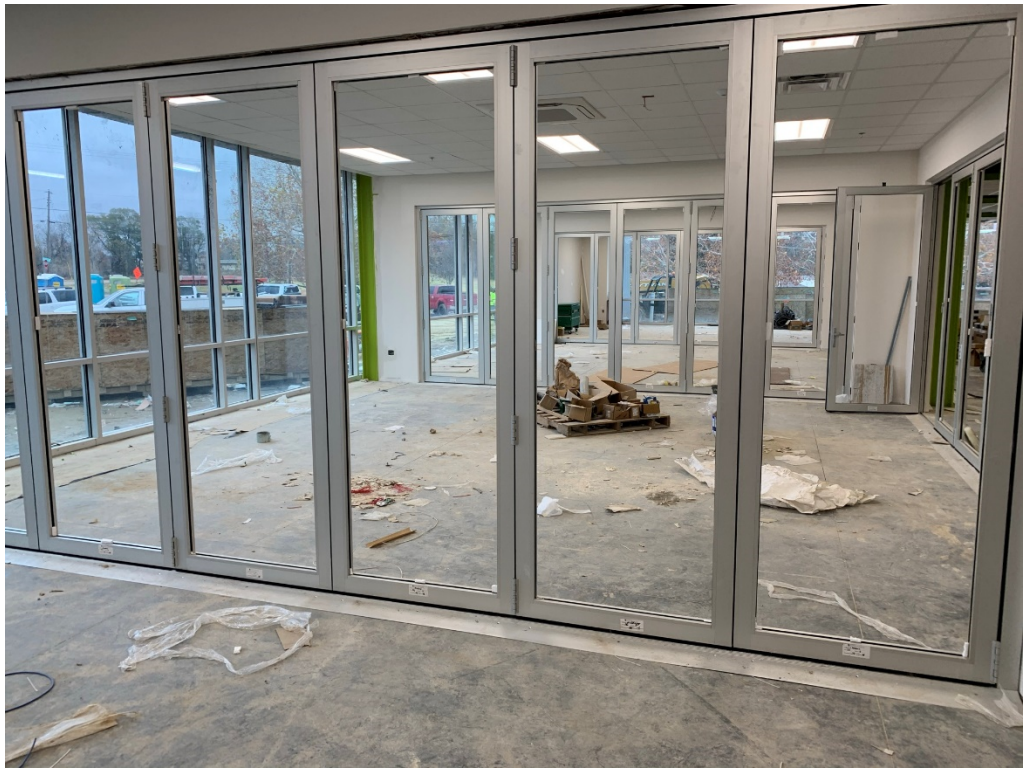
Figure 25 – Foldable partitions are installed throughout
