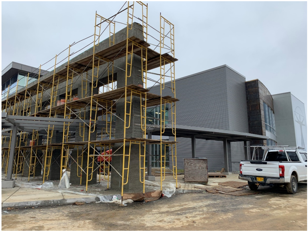
Figure 5 – Stucco work ongoing
