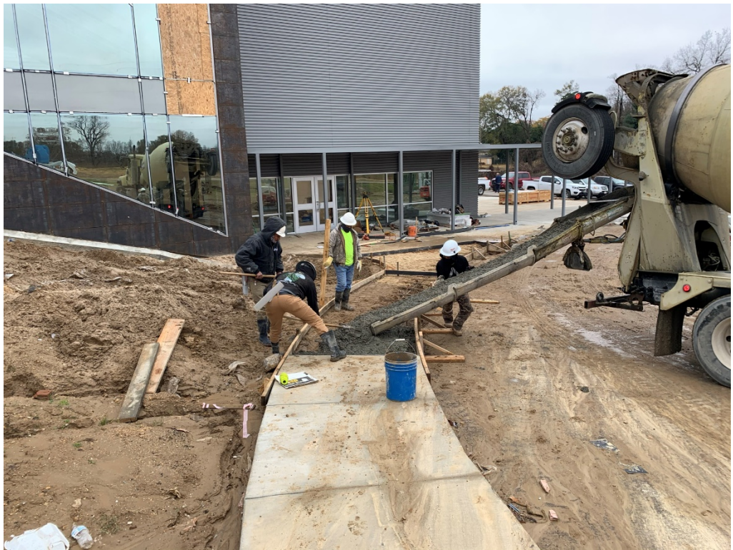
Figure 10 – Concrete work at Sidewalk correction
