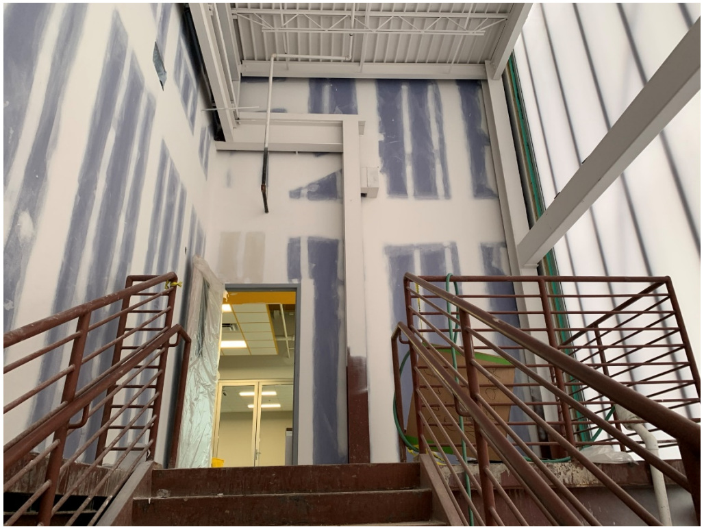
Figure 29 – SE Stair on going
