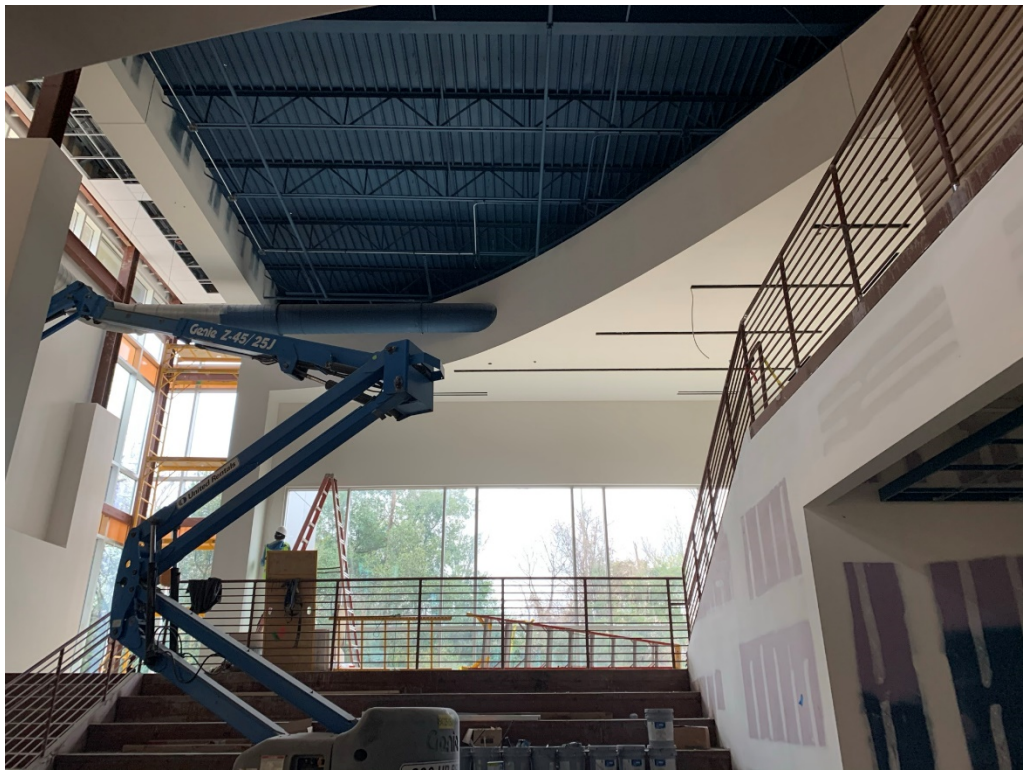
Figure 24 – Lobby Paint Work
