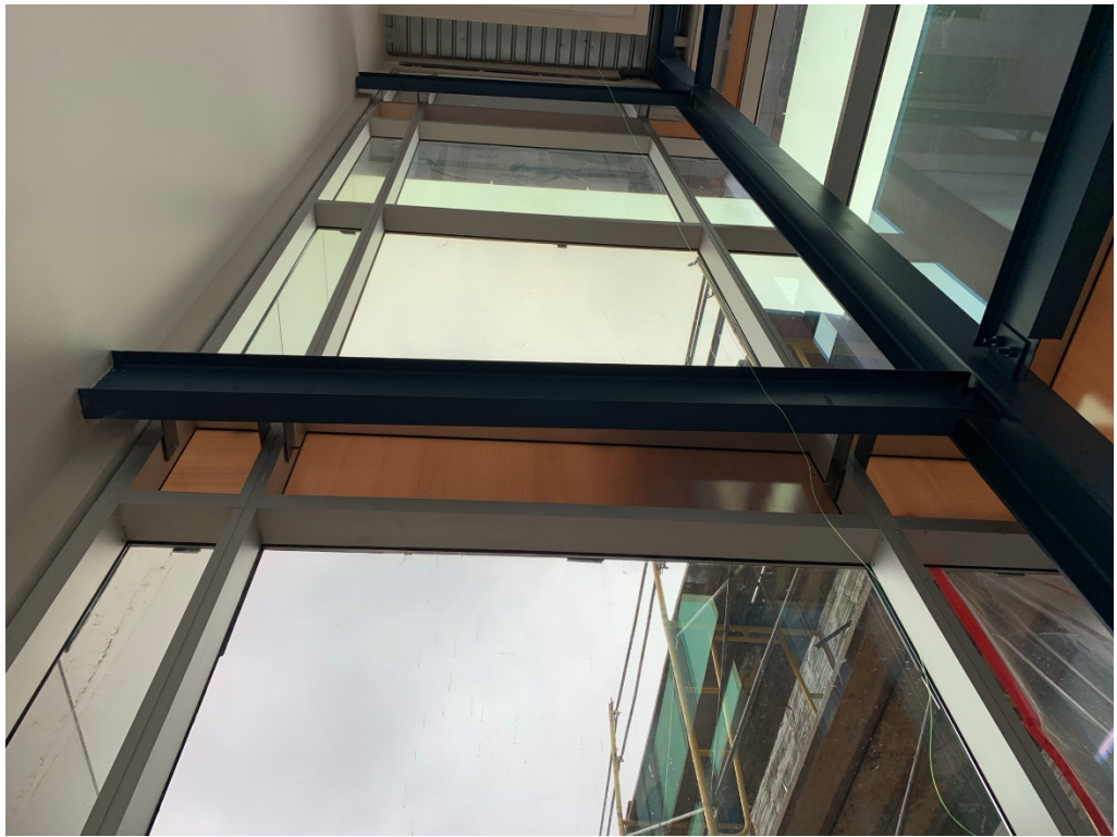
Figure 11 – Paint Work is Ongoing
