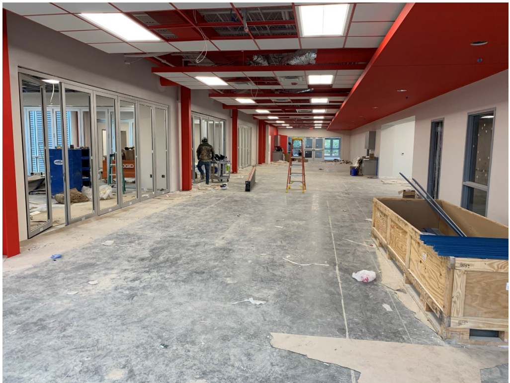
Figure 32 – Partition Wall Installation is Ongoing
