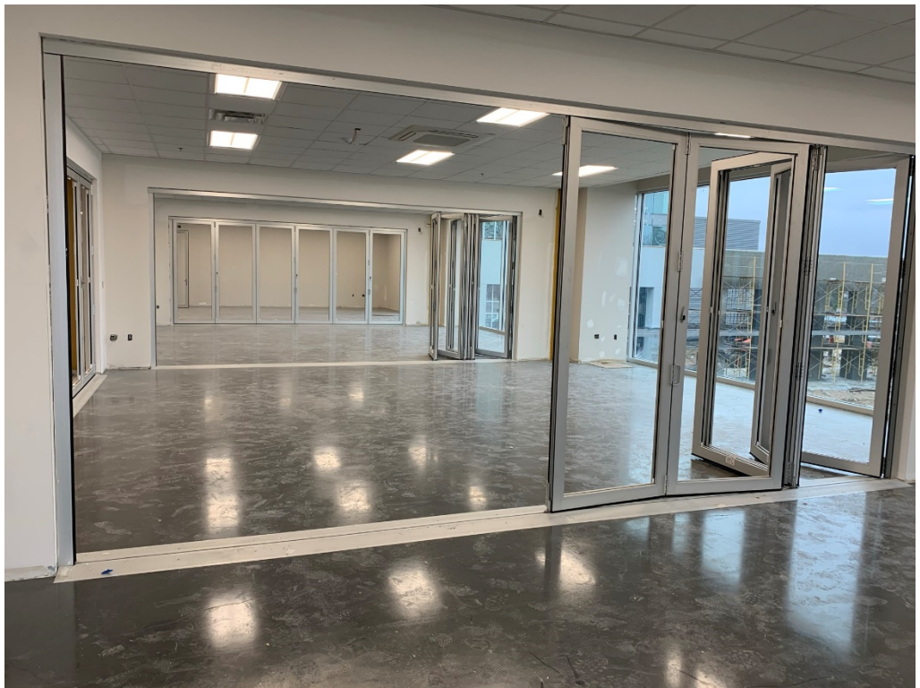
Figure 30 – East Wing nearly complete
