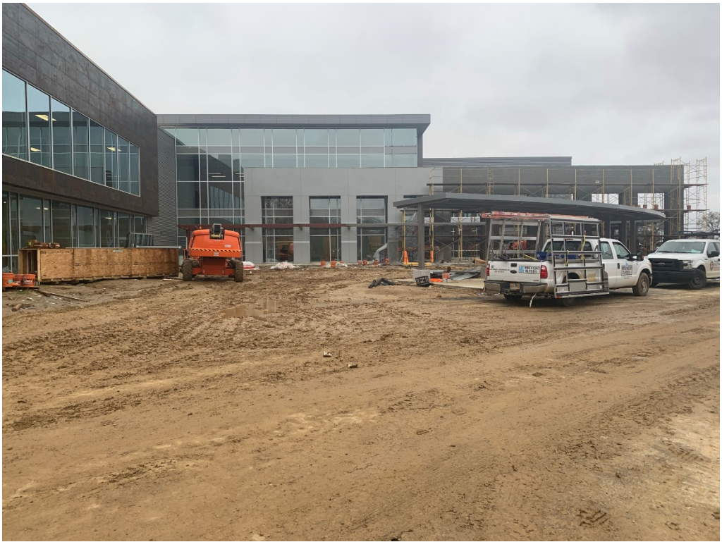
Figure 1 – East Façade at North Central Section of Building
