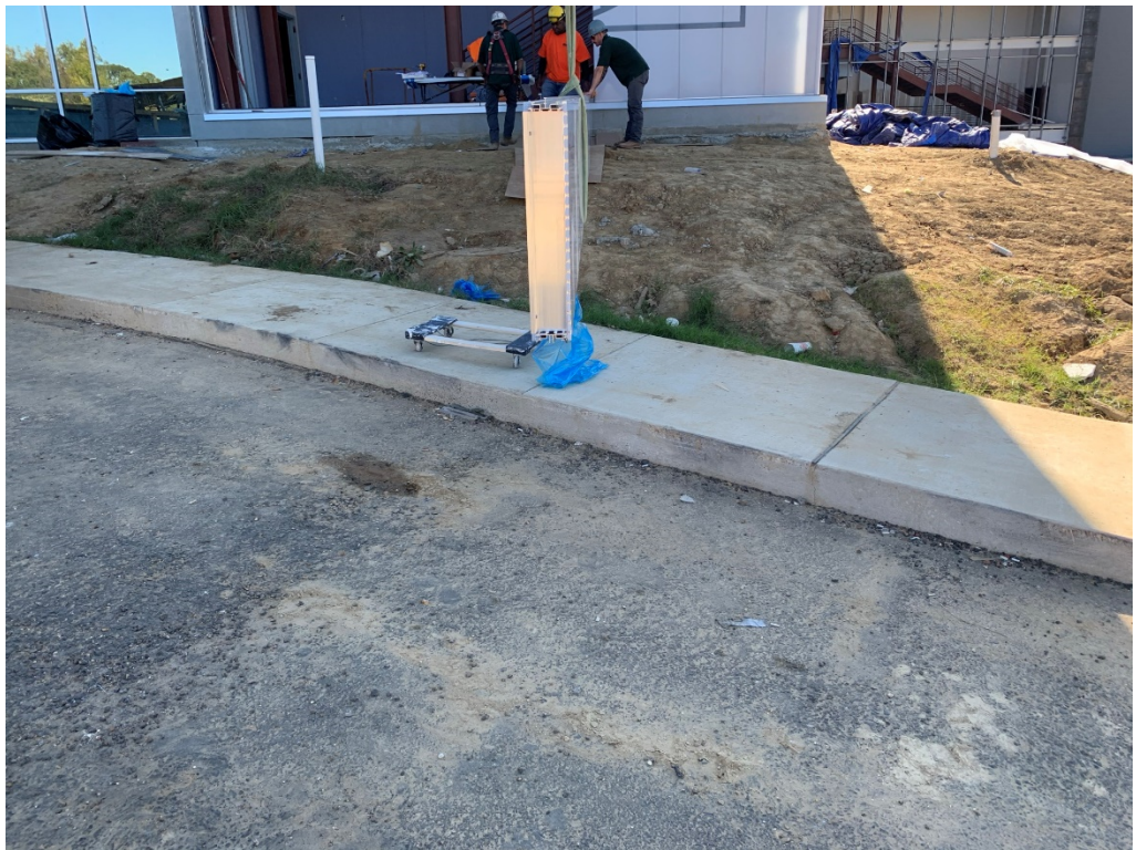
Figure 2 – Panel Installation is Ongoing
