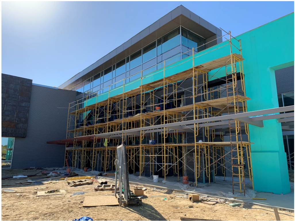
Figure 5 – Stucco work has begun at the main Entrance
