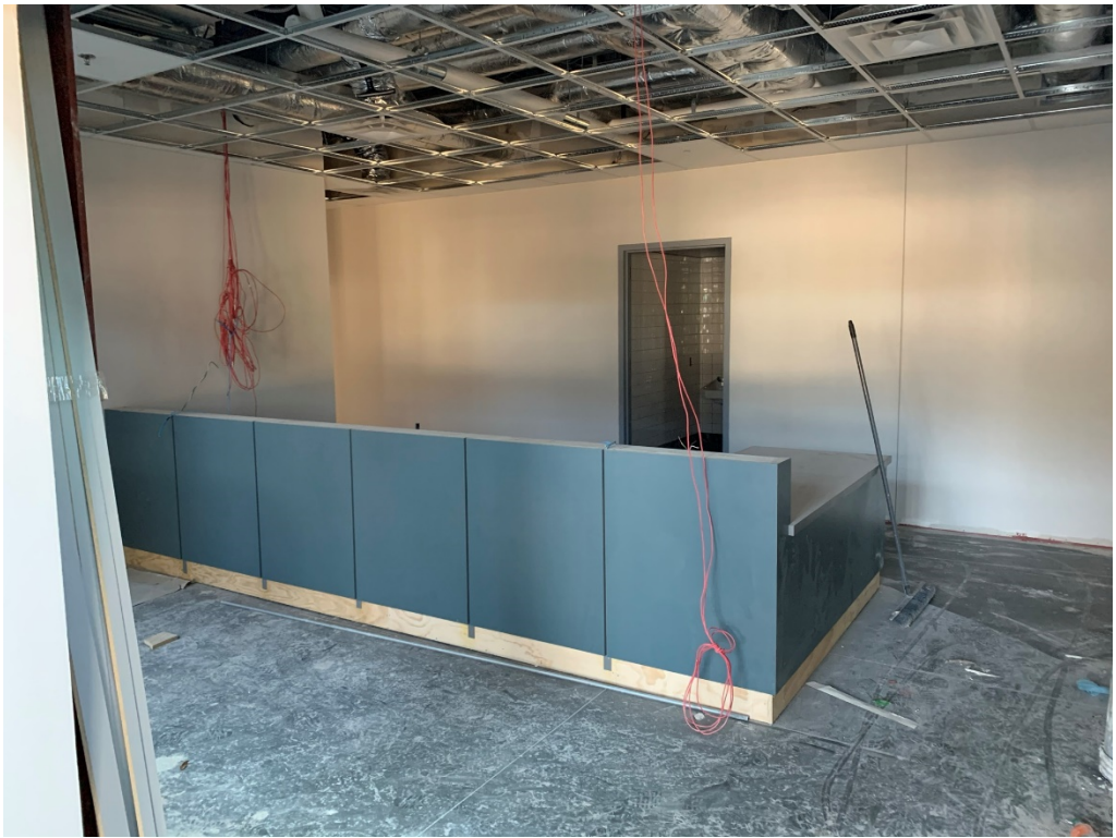
Figure 9 – Millwork at Main Entrance Check In
