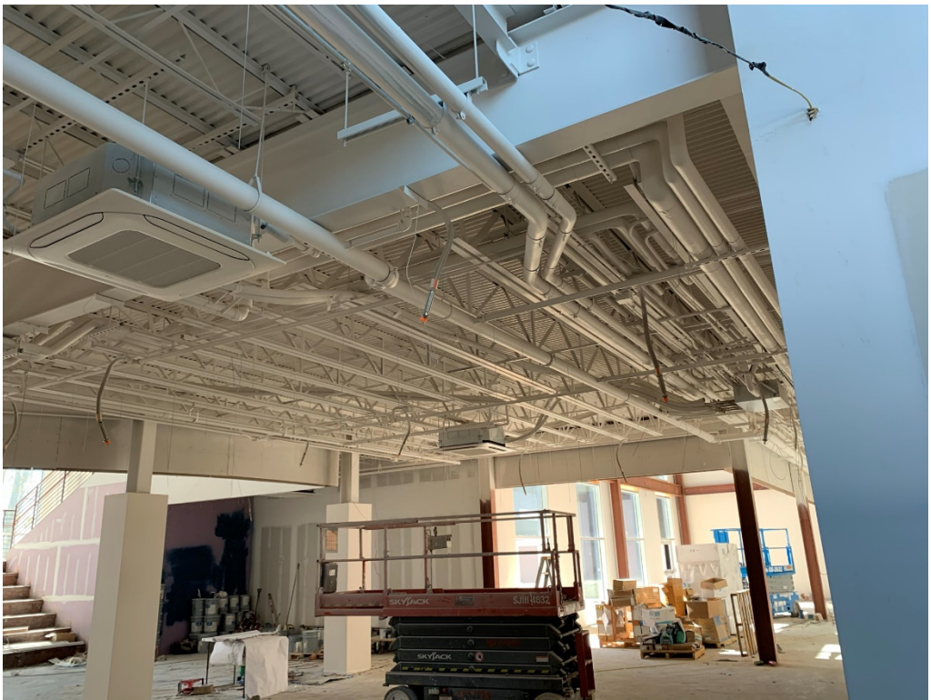
Figure 10 – Ceiling Paint Work
