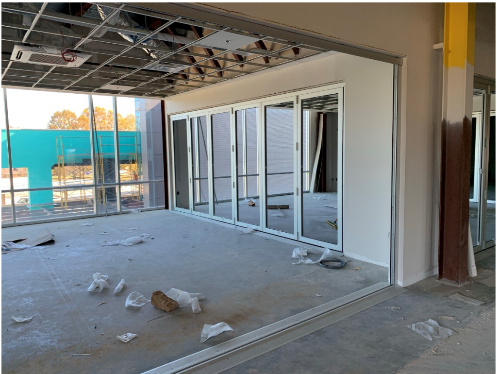
Figure 14 – Partition Wall Installation is Ongoing
