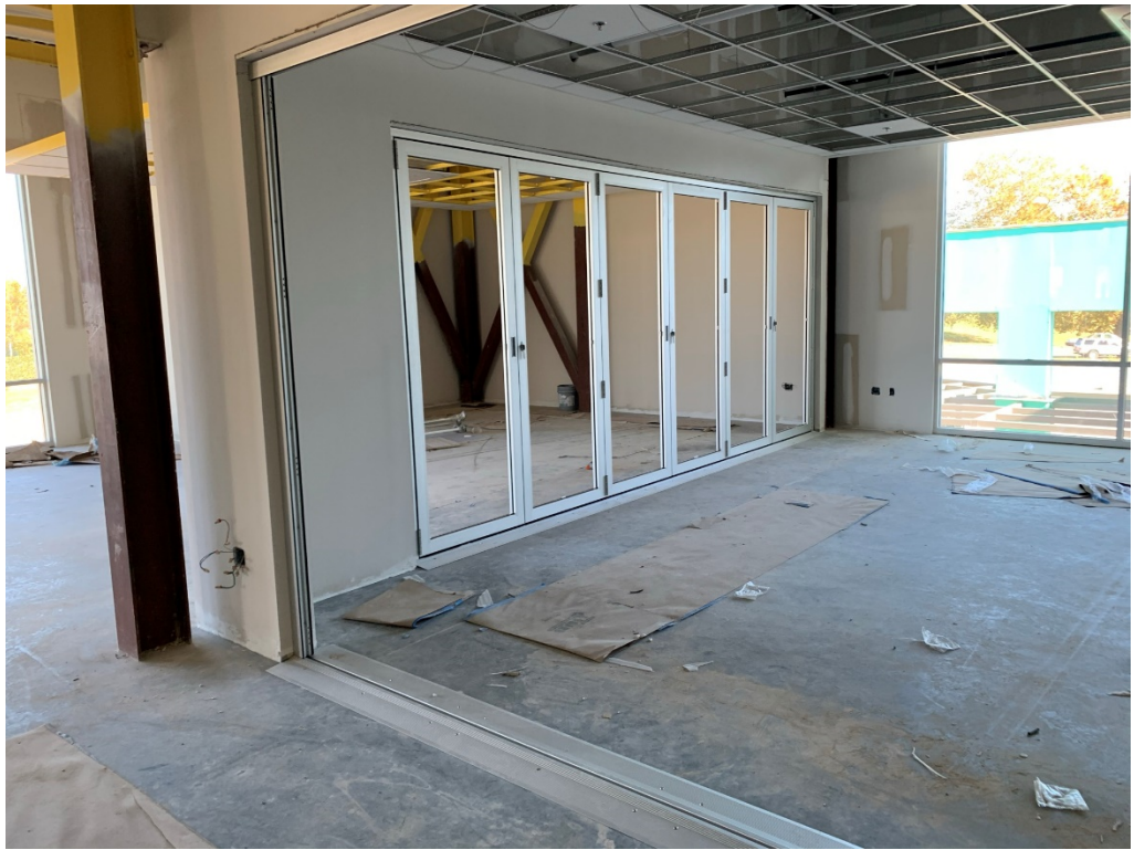
Figure 15 – Partition Wall Installation is Ongoing
