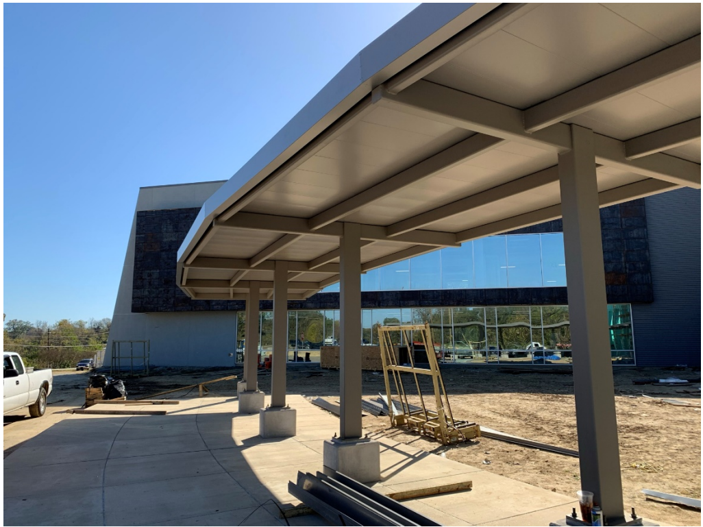
Figure 3 – Awning Covering Installation is Ongoing
