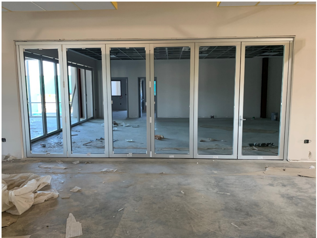
Figure 16 – Partition Wall Installation is Ongoing
