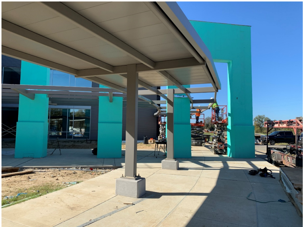
Figure 4 – Awning Covering Installation is Ongoing
