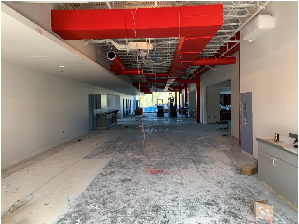
Figure 12 – Paint Work is Ongoing
