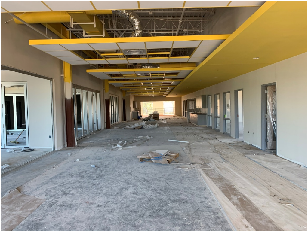
Figure 13 – Paint Work is Ongoing
