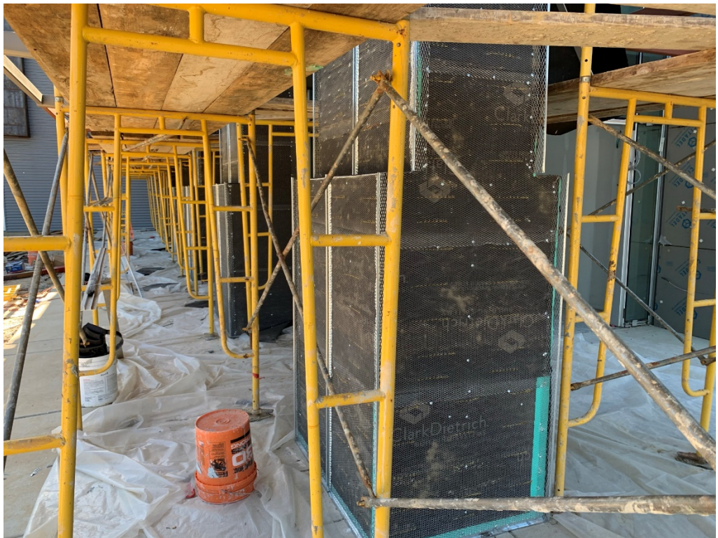
Figure 6 – Stucco work has begun at the main Entrance
