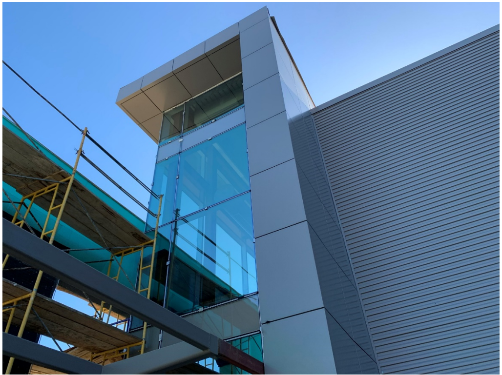
Figure 7 – Metal Paneling and Curtain Wall at the Entrance
