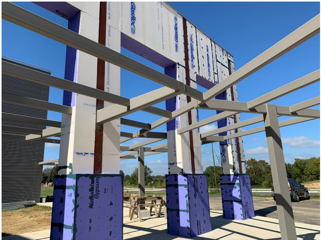
Figure 44 – Innovative Canopy Progress
