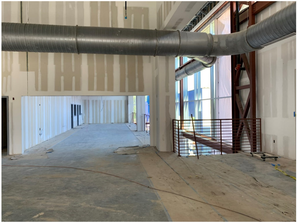
Figure 37 – 3 rd Floor Lobby Progress
