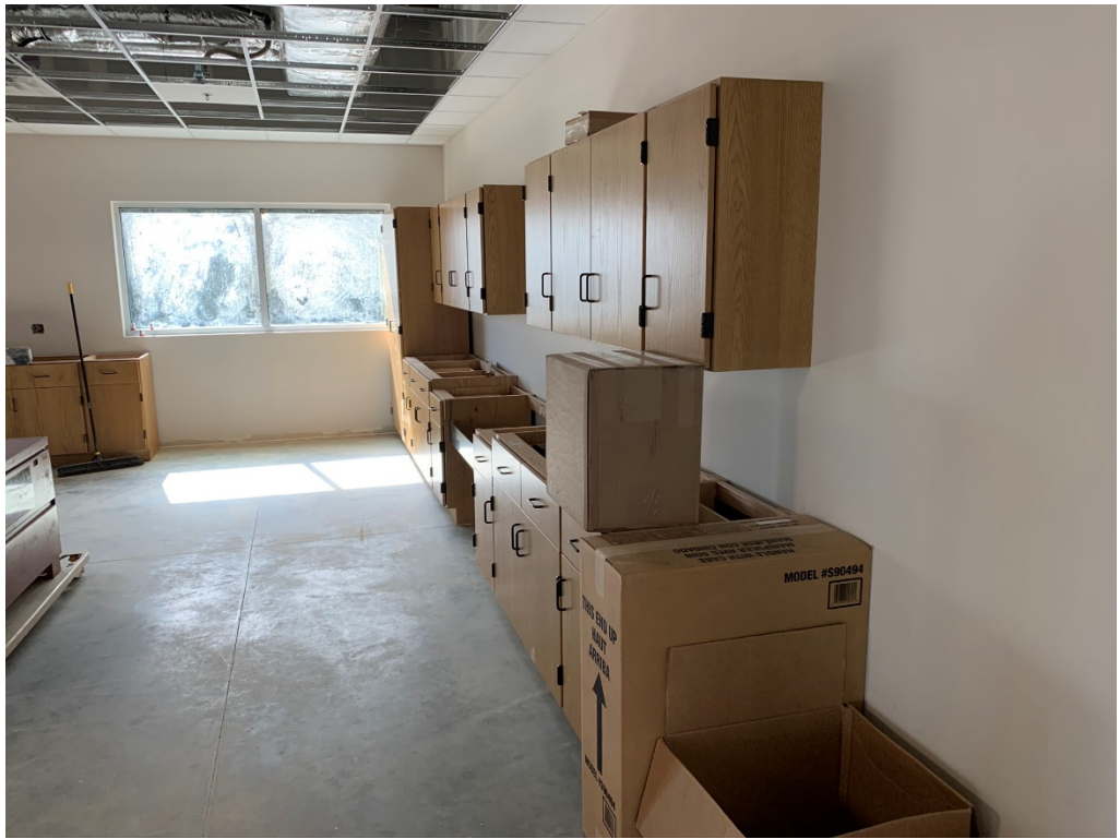
Figure 31 – Cabinets Installed at East Classrooms
