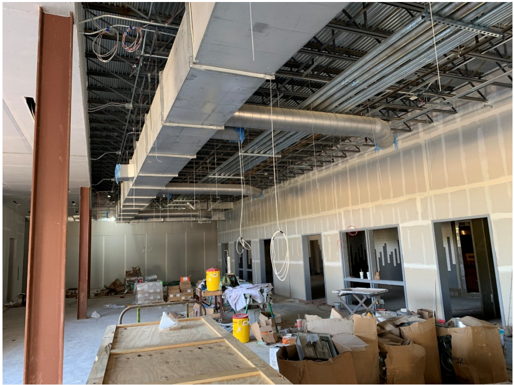
Figure 5 – Cafeteria Mech is Ongoing
