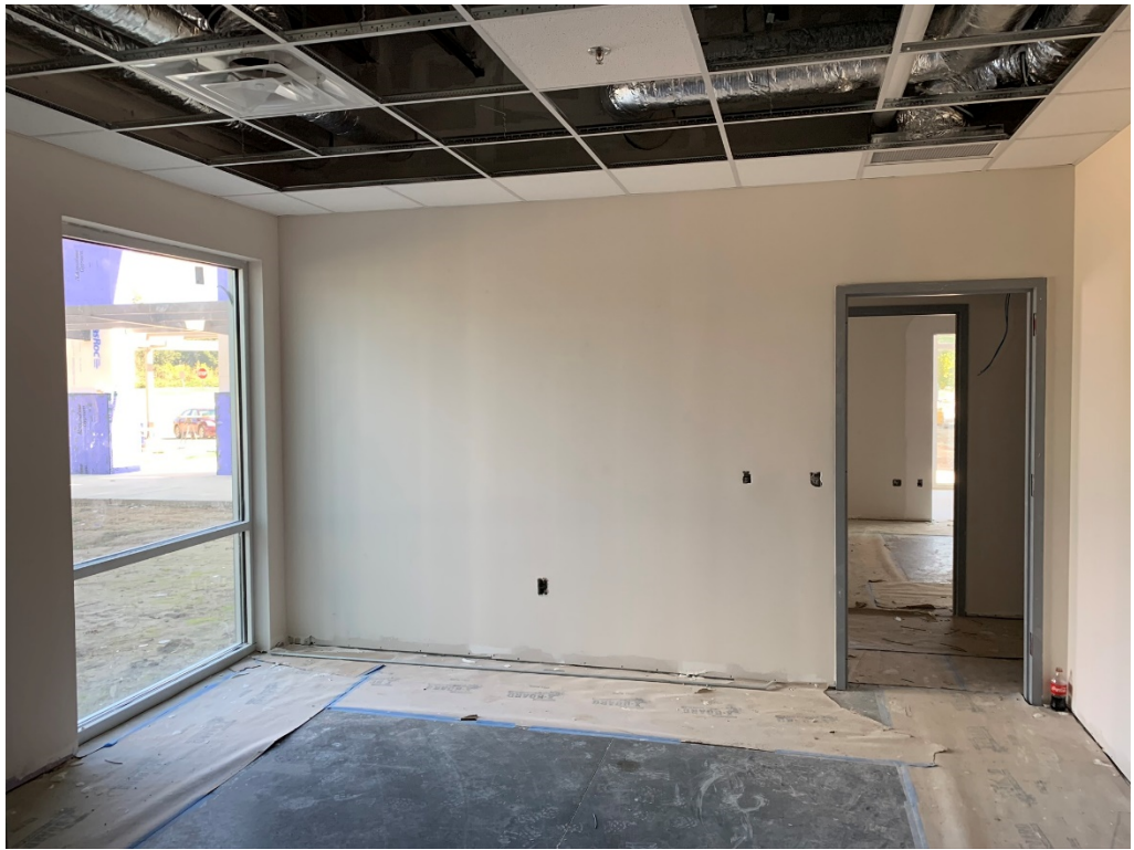
Figure 27 – Finishing Progress @ 2 nd Floor Office Area
