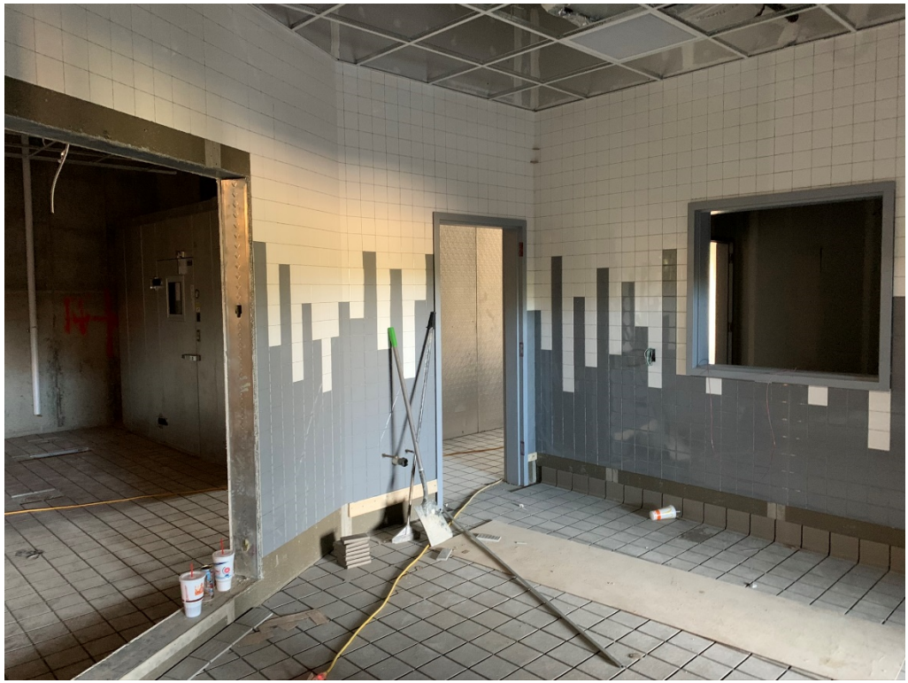
Figure 9 – Tile at Cafeteria Serving
