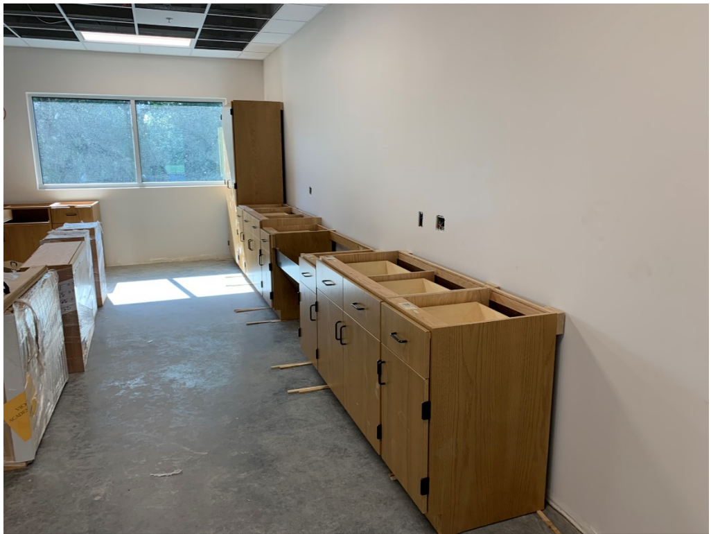
Figure 34 – Cabinets Installed at East Classrooms
