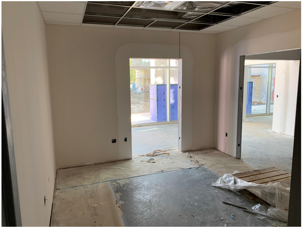
Figure 29 – Finishing Progress @ 2 nd Floor Office Area
