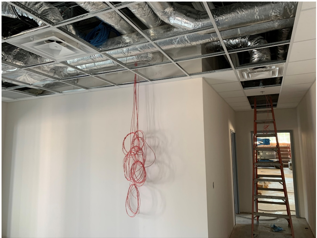
Figure 30 – Finishing Progress @ 2 nd Floor Office Area
