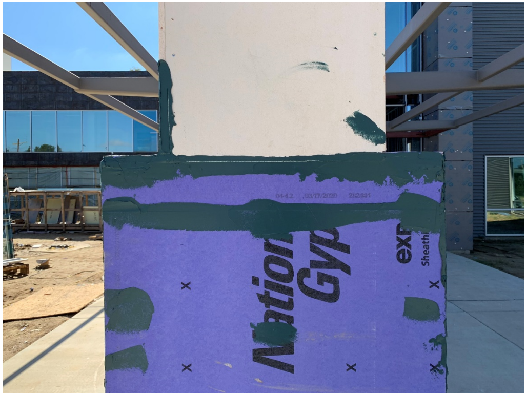
Figure 45 – Innovative Canopy Progress
