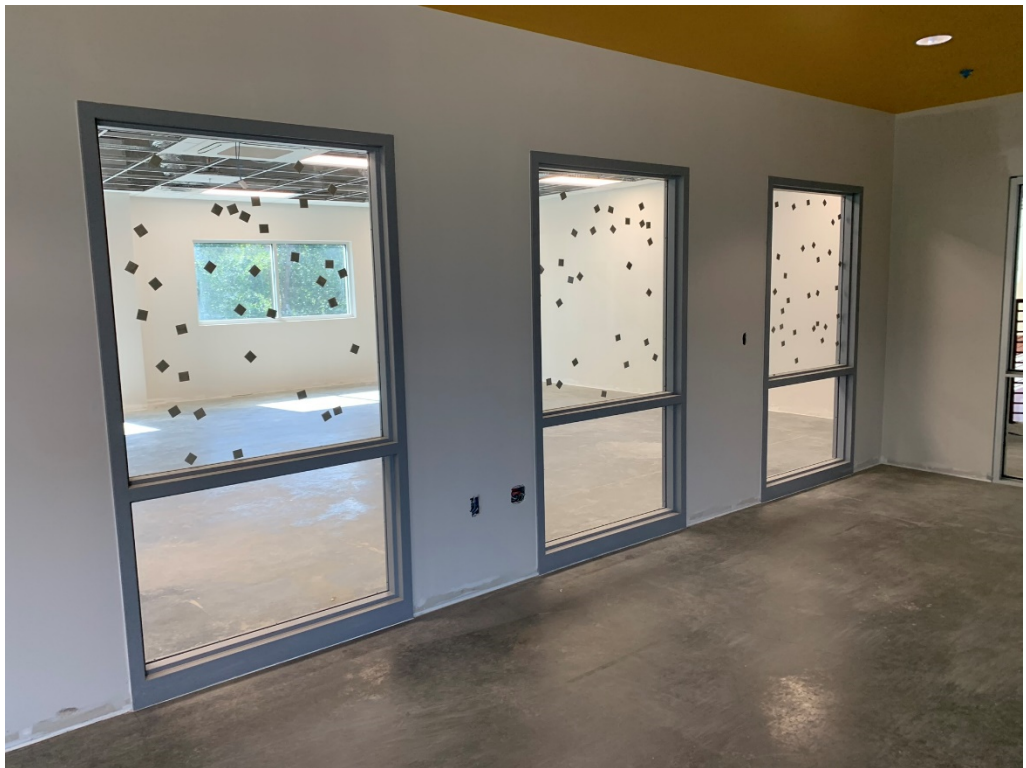
Figure 36 – 3 rd Floor Entry Glazing Install Progress
