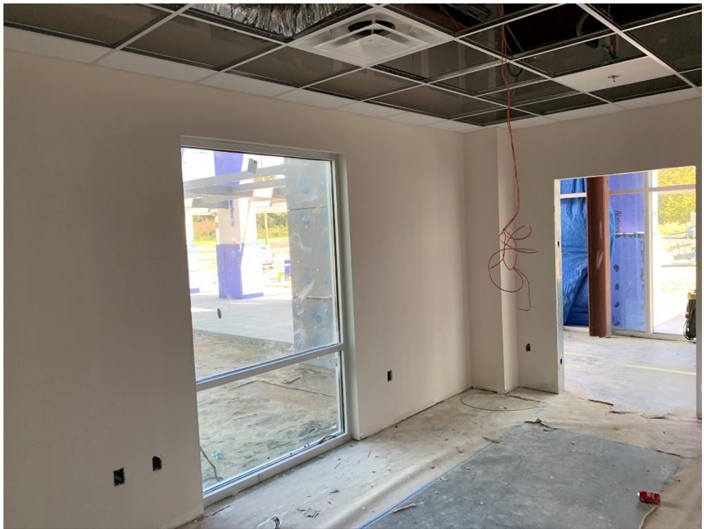
Figure 28 – Finishing Progress @ 2 nd Floor Office Area
