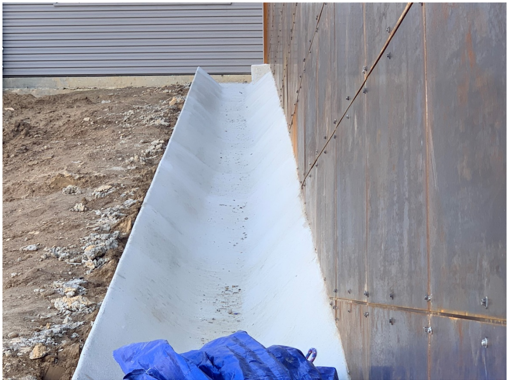
Figure 4 – Concrete Drainage Formed & Poured at Curtain Wall
