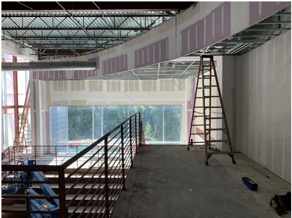
Figure 38 – 3 rd Floor Lobby Progress
