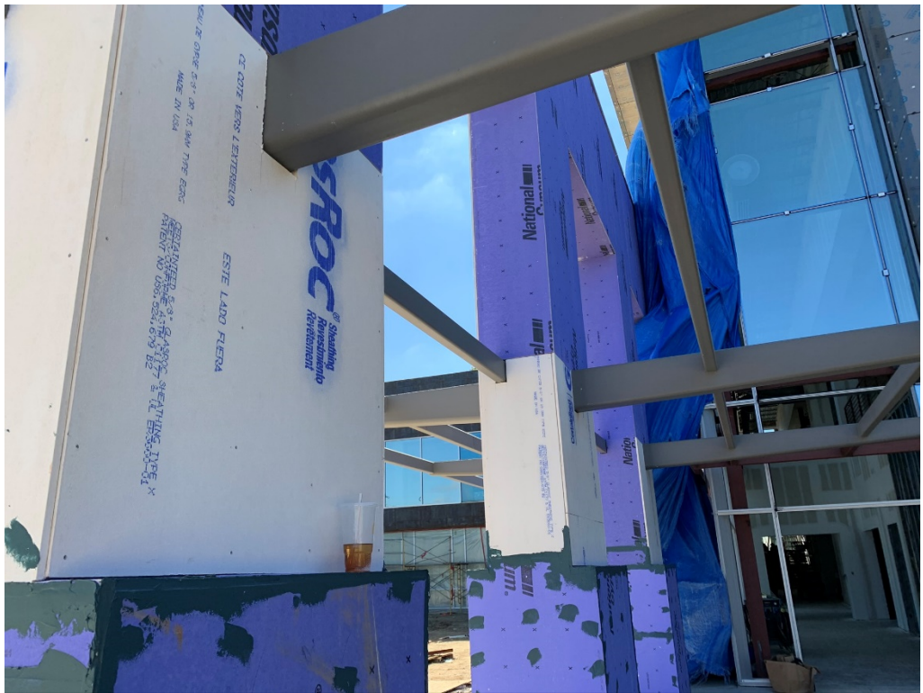
Figure 46 – Innovative Canopy Progress
