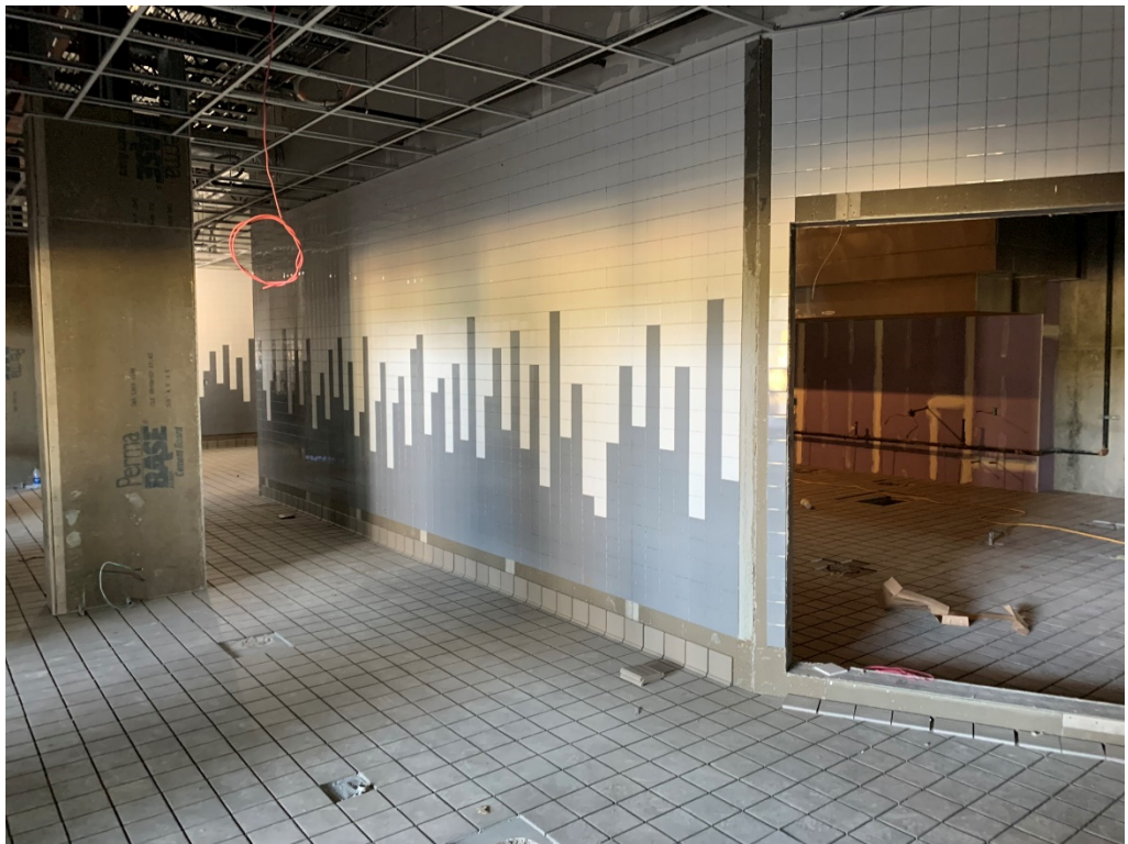
Figure 8 – Tile at Cafeteria Serving
