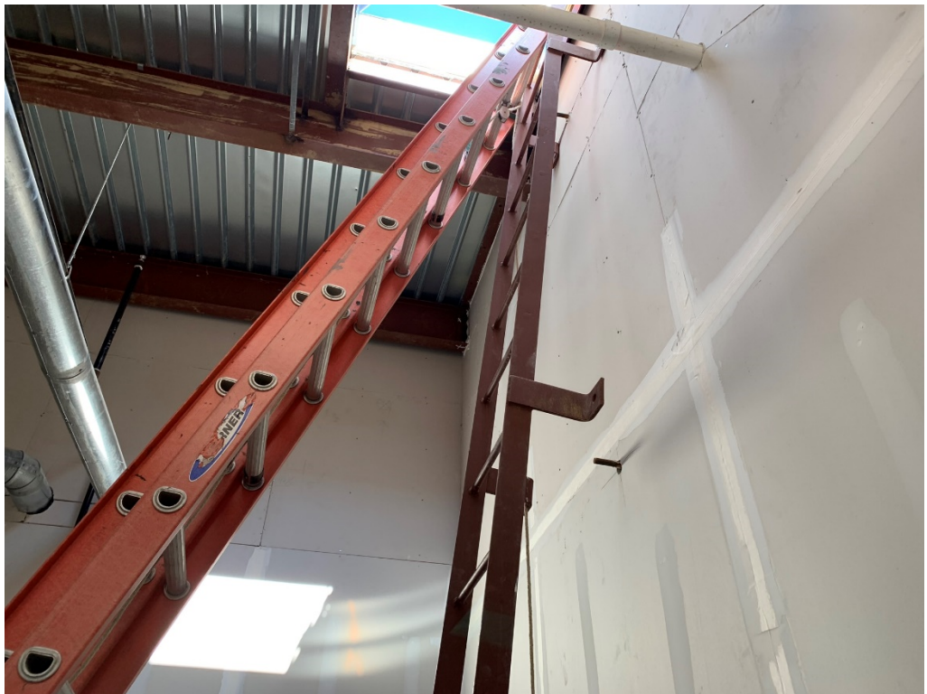
Figure 42 – Ladder Access Install
