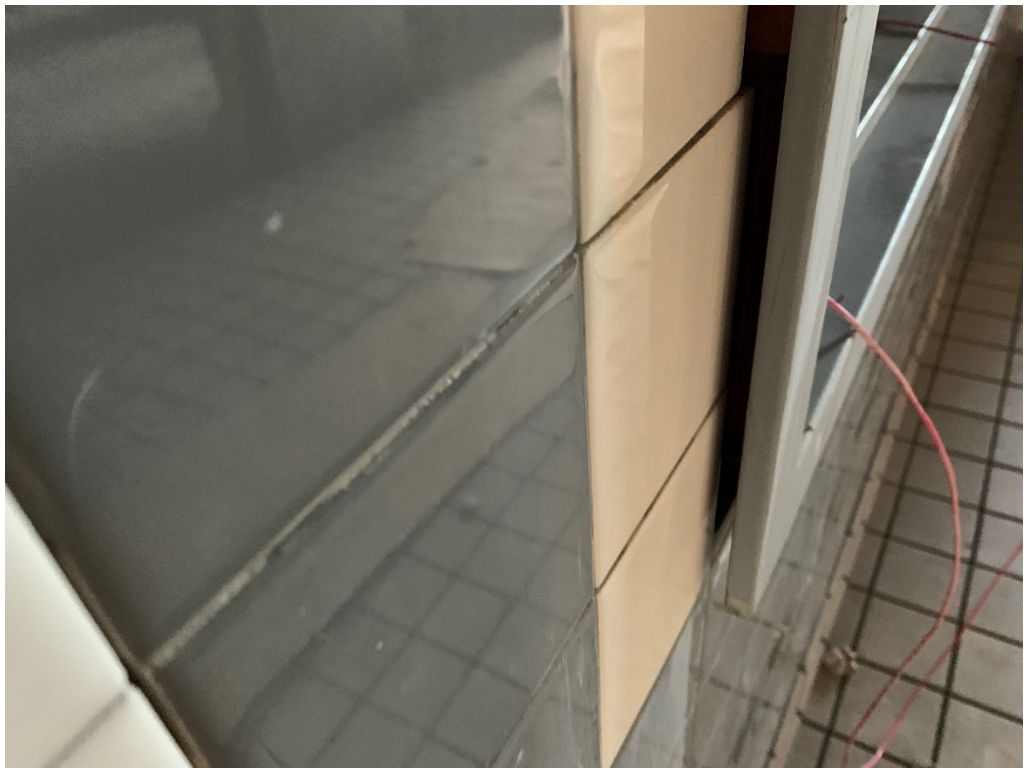
Figure 12 – Tile at Cafeteria Serving
