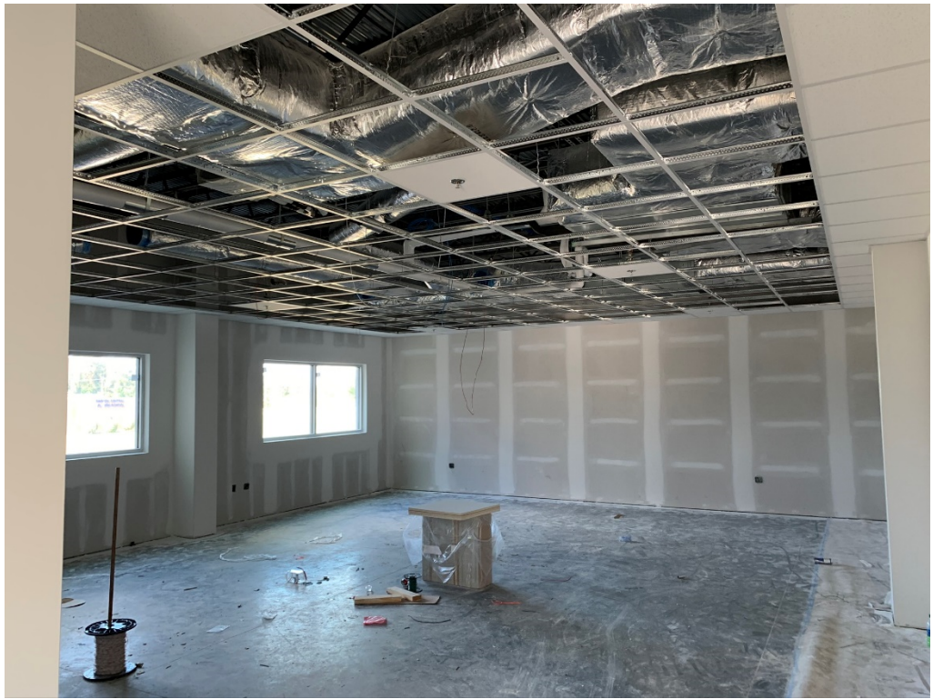
Figure 23 – Ceiling at 2nd Floor Classrooms at North End
