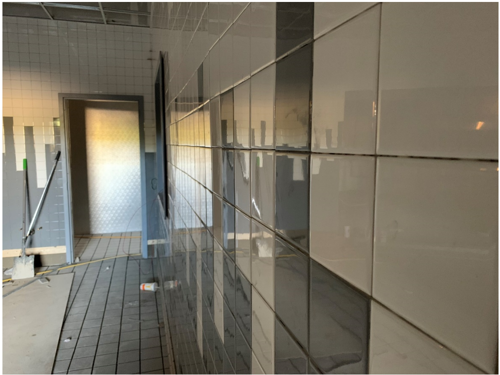
Figure 11 – Tile at Cafeteria Serving
