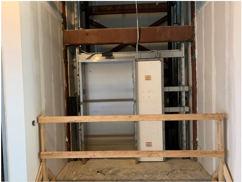
Figure 21 – 2 nd Floor Elevator Door Installed
