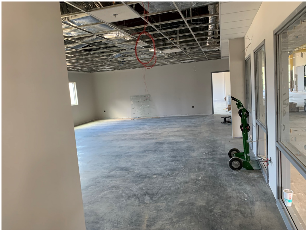
Figure 40 – 3 rd Floor Classroom Progress
