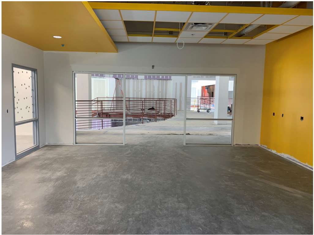
Figure 35 – 3 rd Floor Entry Glazing Install Progress
