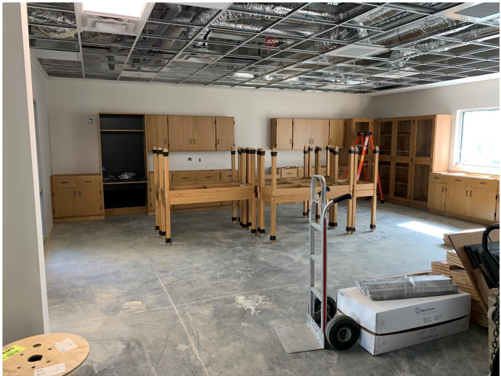
Figure 32 – Cabinets Installed at East Classrooms
