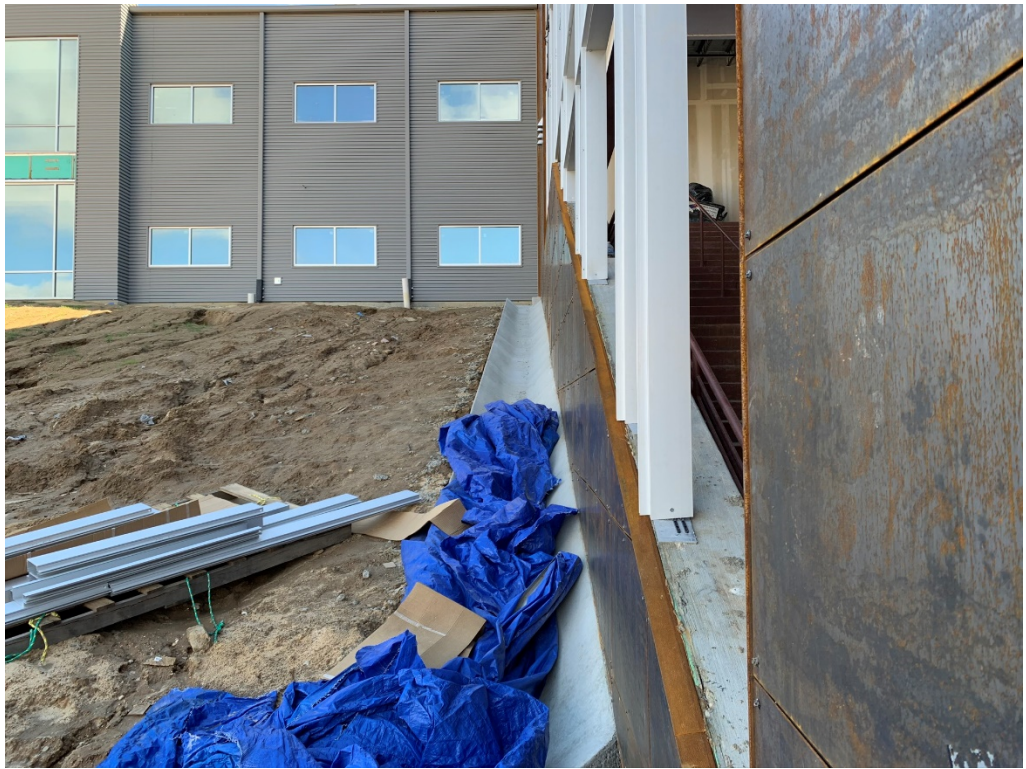
Figure 3 – Concrete Drainage Formed & Poured at Curtain Wall
