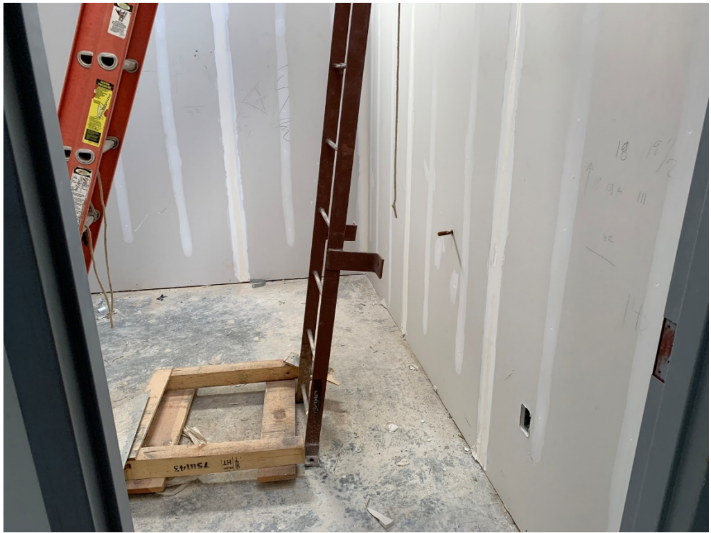
Figure 41 – Ladder Access Install
