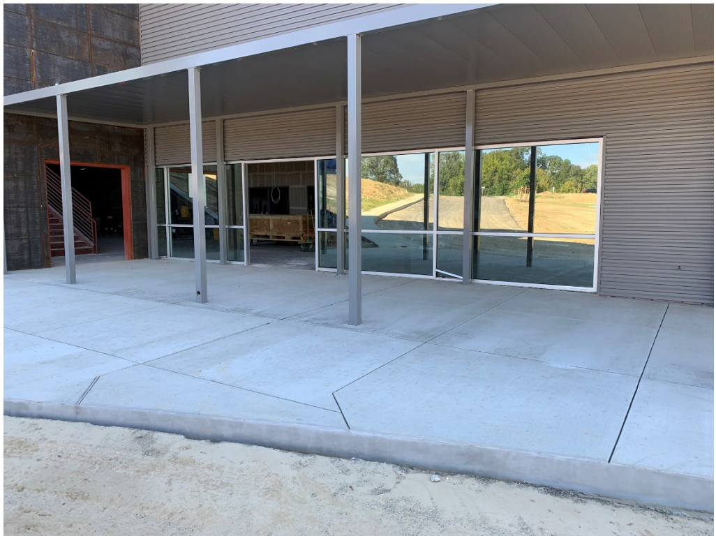
Figure 2 – Cafeteria Entry Glazing Install
