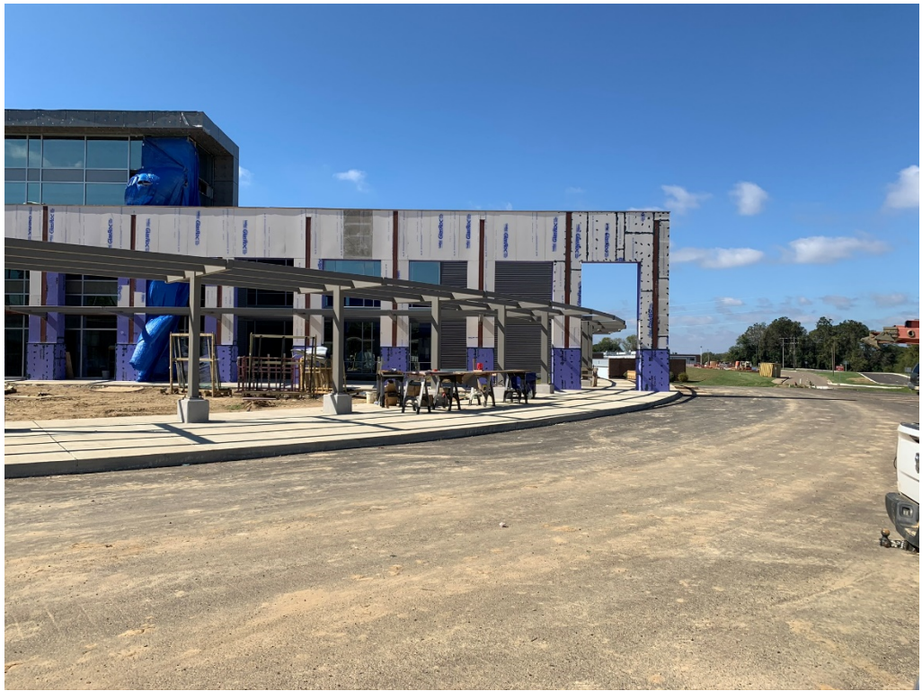
Figure 43 – Innovative Canopy Progress
