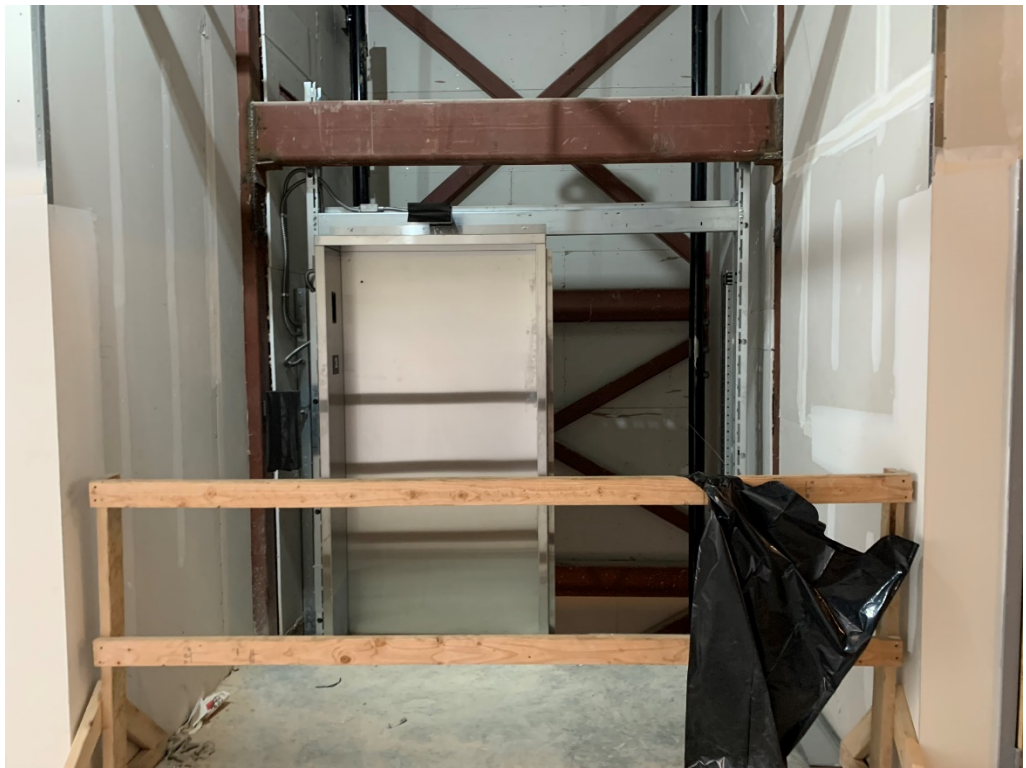
Figure 22 – 3 rd Floor Elevator Door Installed
