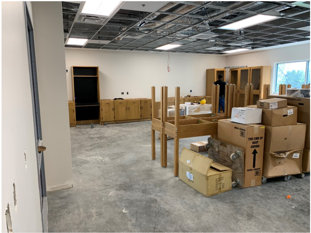
Figure 33 – Cabinets Installed at East Classrooms
