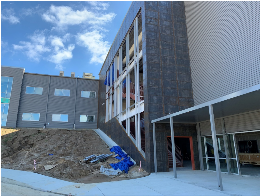
Figure 1 – West Section of Building North Elevation Curtain Wall Install Ongoing
