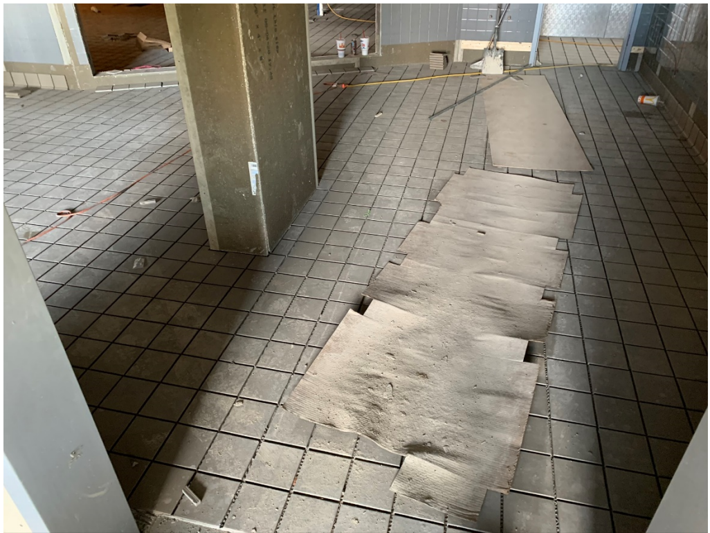
Figure 6 – Tile at Cafeteria Serving
