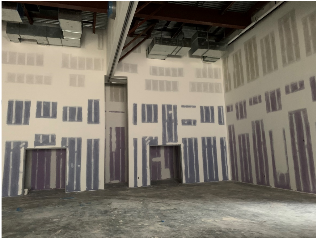
Figure 11 – Gym Ready for Paint
