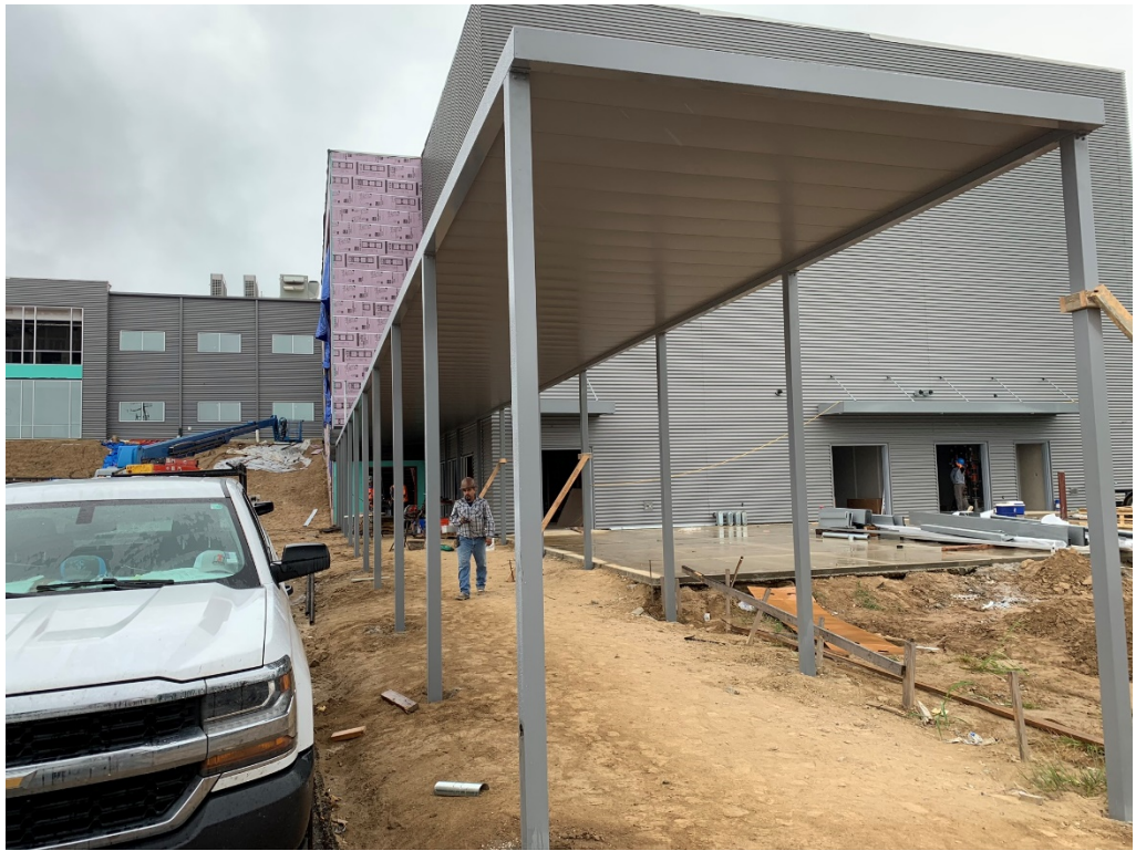
Figure 1 – Metal Drop Off Awning Installed
