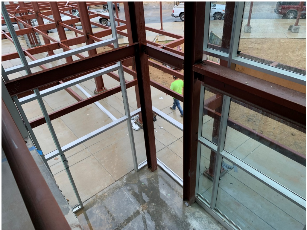
Figure 16 – Curtain Wall Progress Continues
