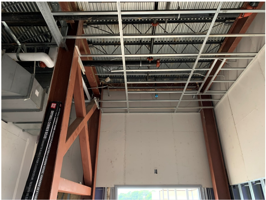
Figure 7 – Grid work at Cafeteria
