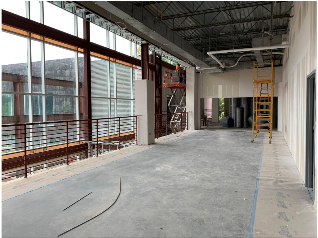
Figure 15 – Multi-Purpose at 3 rd Floor
