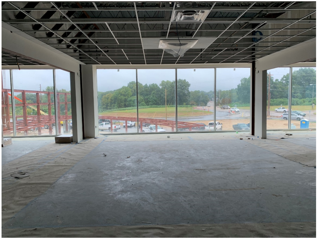
Figure 19 – Versatile Teaching Space 210 Grid Ready for Ceiling Tile
