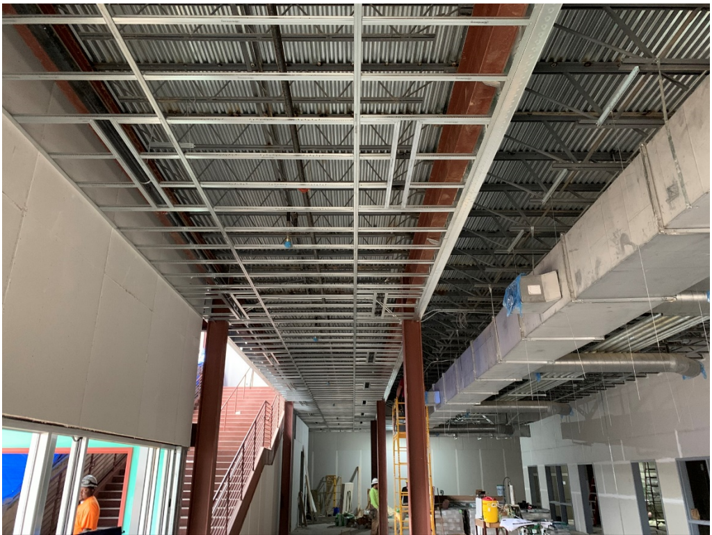
Figure 6 – Grid work at Cafeteria
