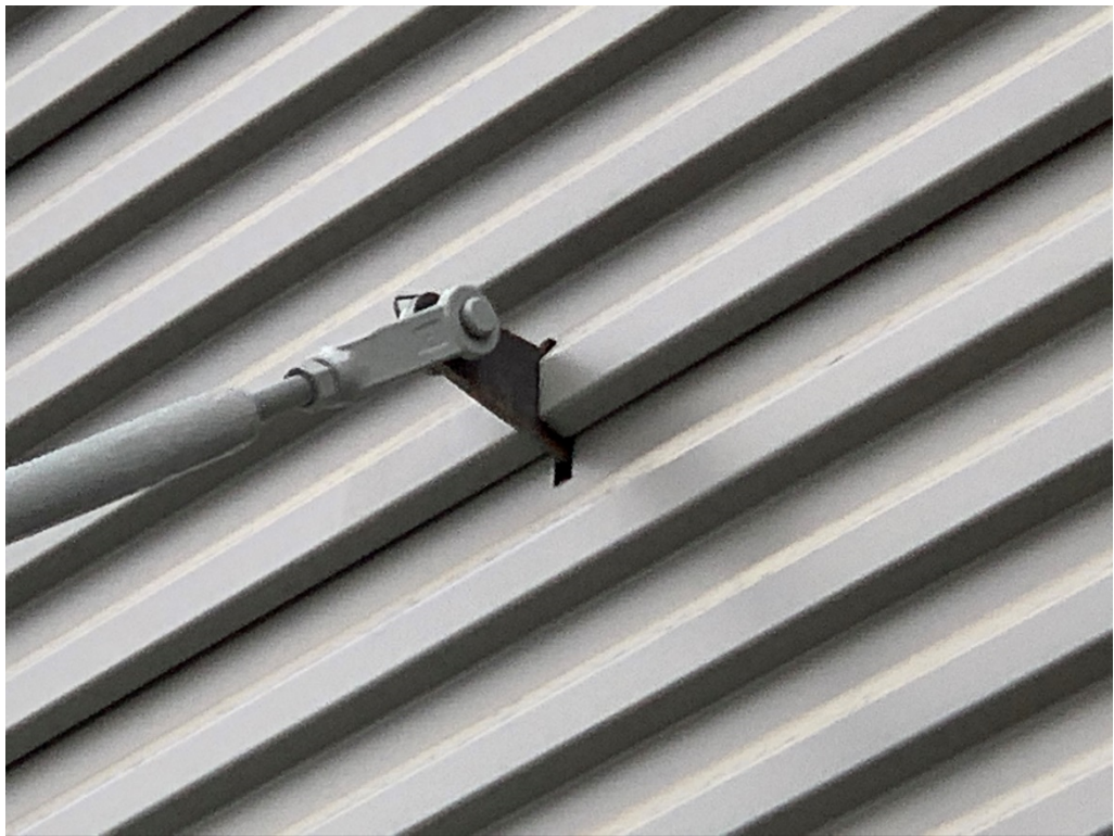
Figure 4 –Bracket Intersection with Siding
