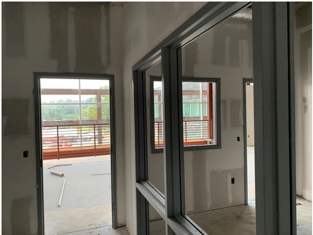
Figure 14 – 3 rd Floor Conference Area
