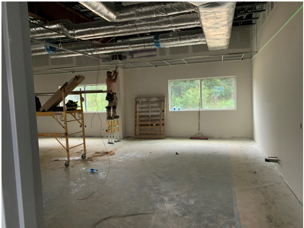
Figure 22 – Classroom Grid Install is Ongoing
