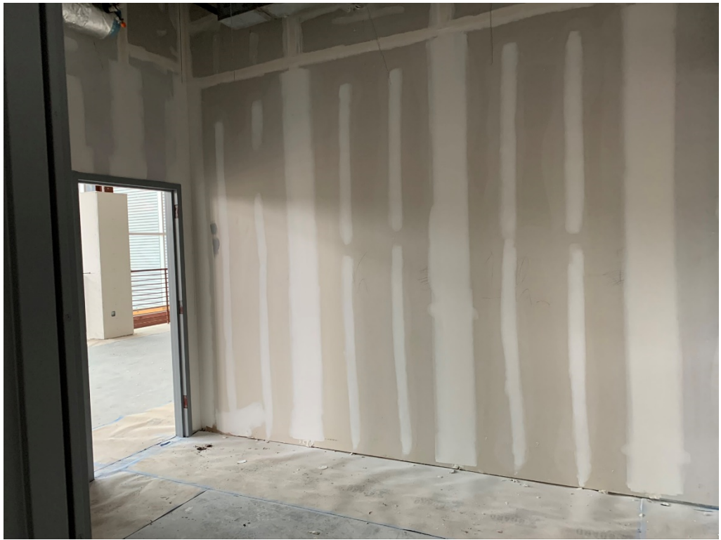
Figure 13 – 3 rd Floor Conference Area
