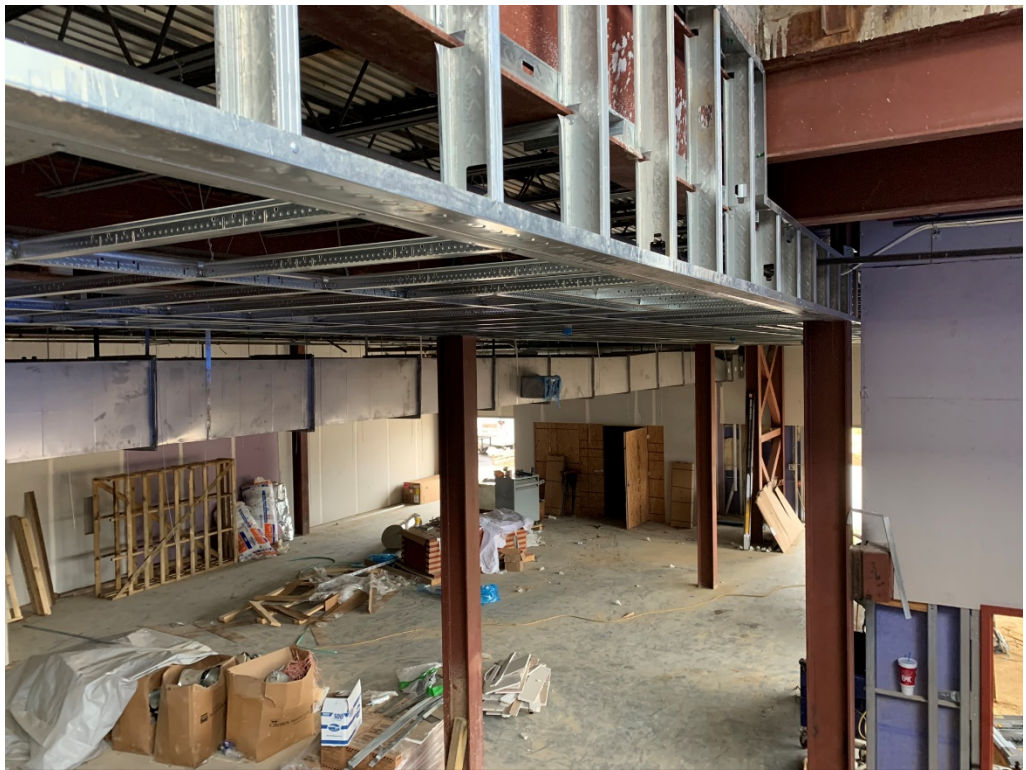
Figure 8 – Grid work at Cafeteria
