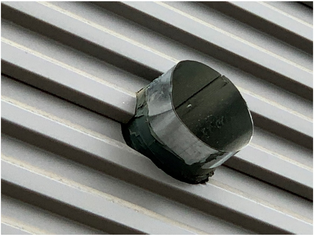
Figure 5 – Duct Intersection with Siding
