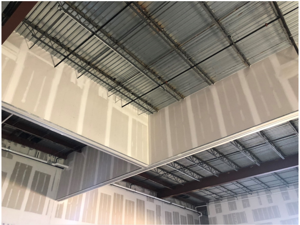
Figure 13 – Gym Drywall Finishing
