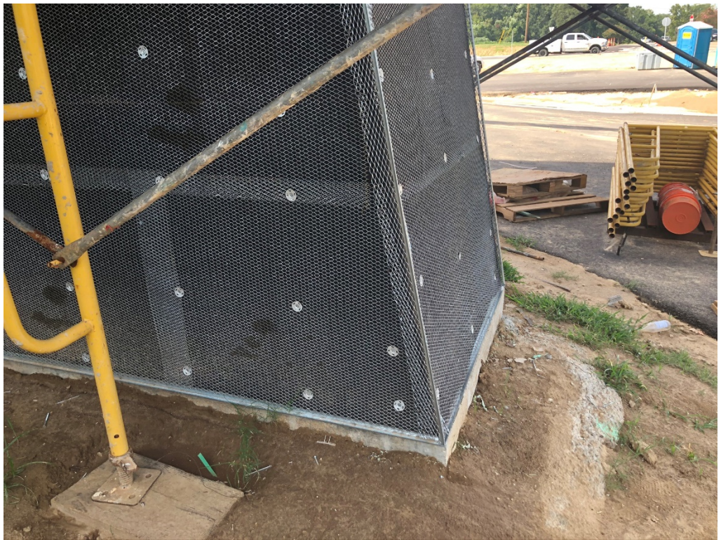
Figure 28 – Stucco Lathe Installed
