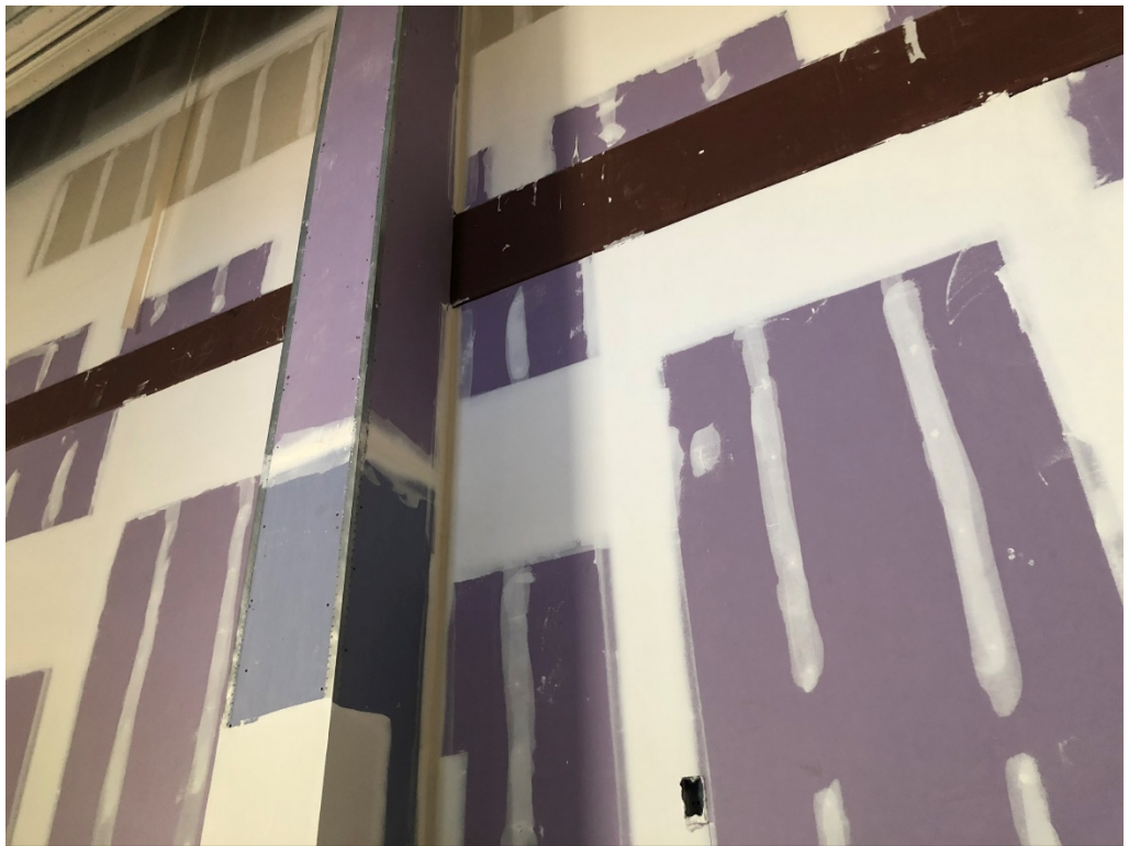
Figure 14 – Gym Drywall Finishing
