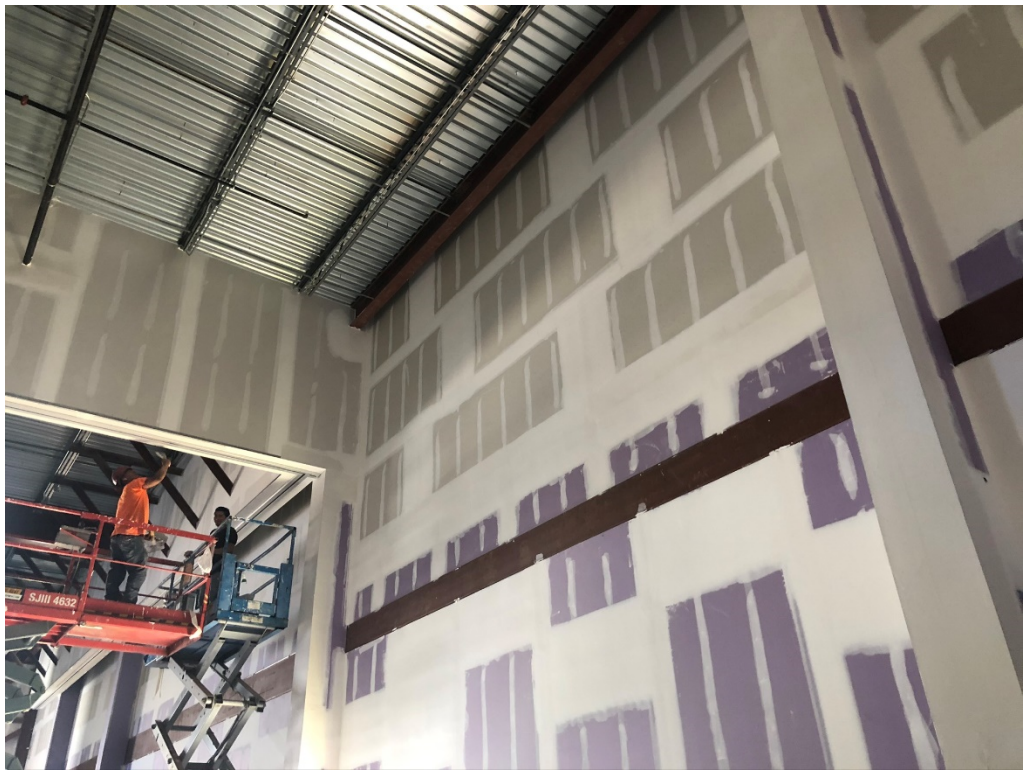
Figure 12 – Gym Drywall Finishing
