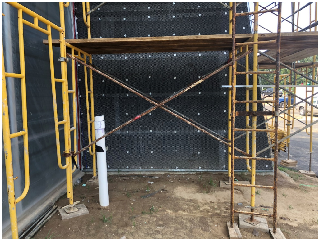
Figure 26 – Stucco Lathe Installed
