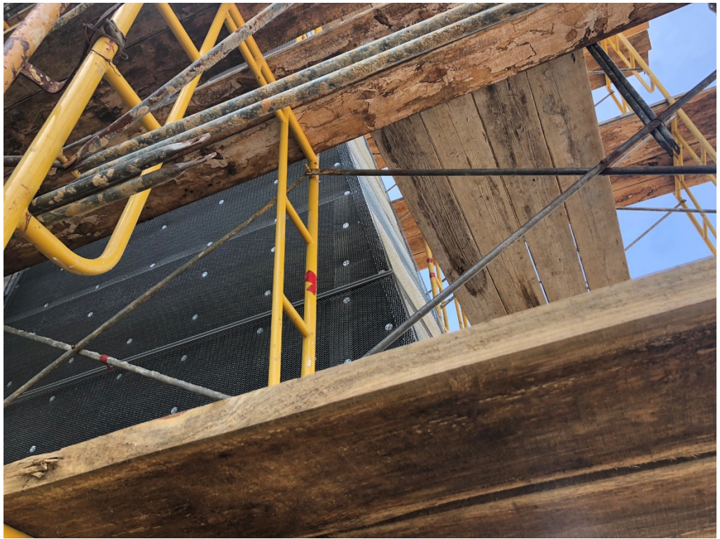
Figure 27 – Stucco Lathe Installed
