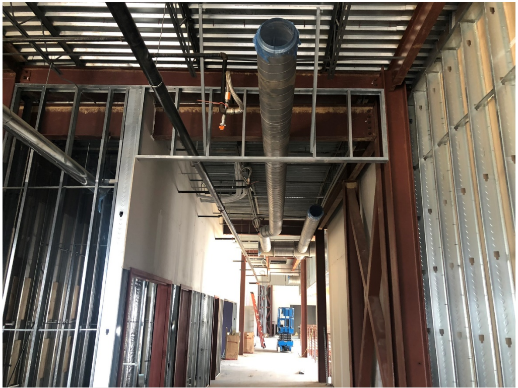
Figure 19 – HVAC is Ongoing
