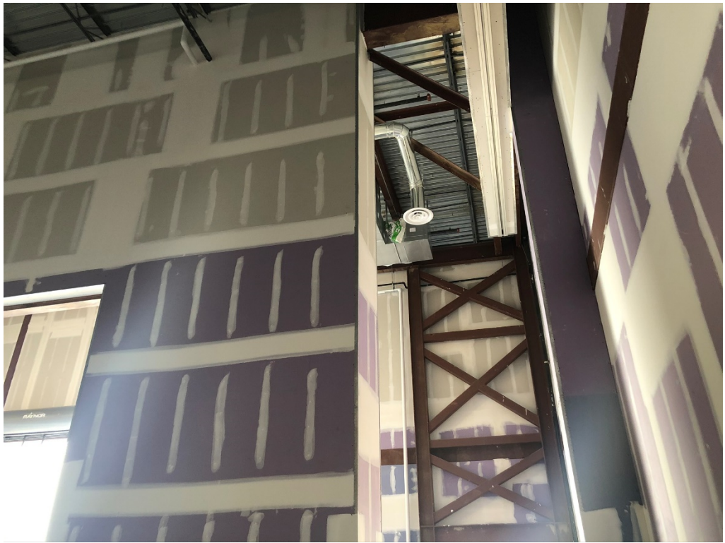
Figure 15 – Gym Drywall Finishing
