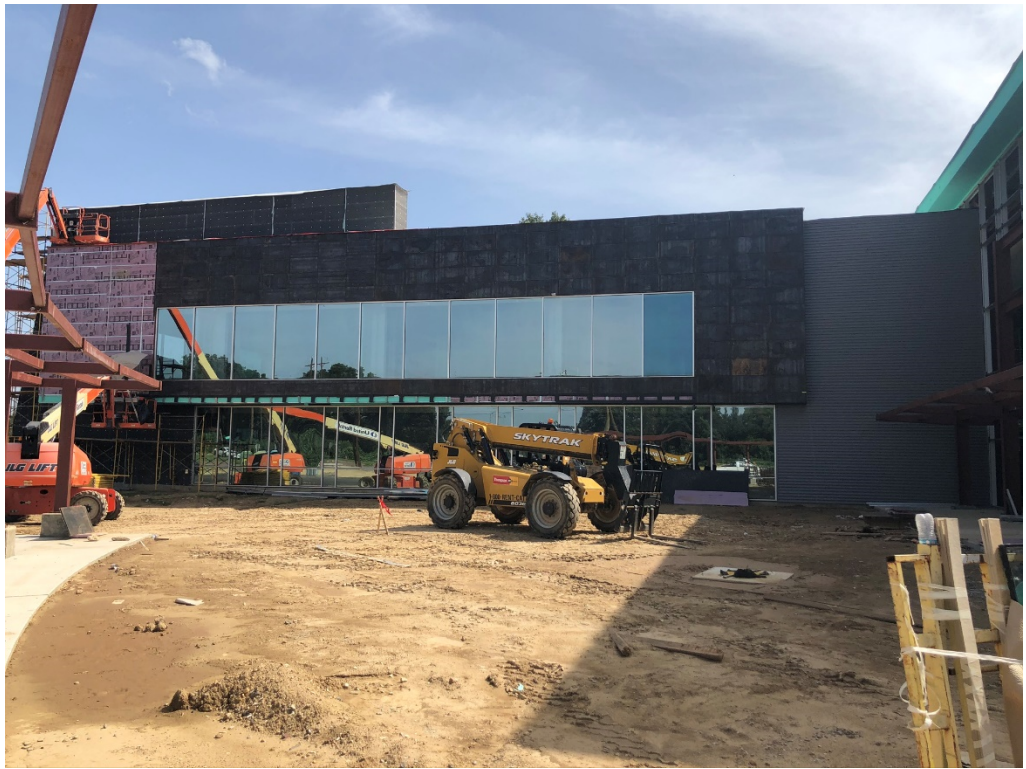
Figure 1 – Metal Siding Installed
