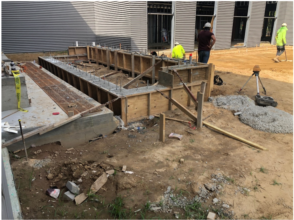
Figure 17 – Concrete Work at Rear Courtyard
