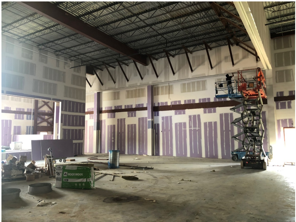
Figure 10 – Gym Drywall Finishing
