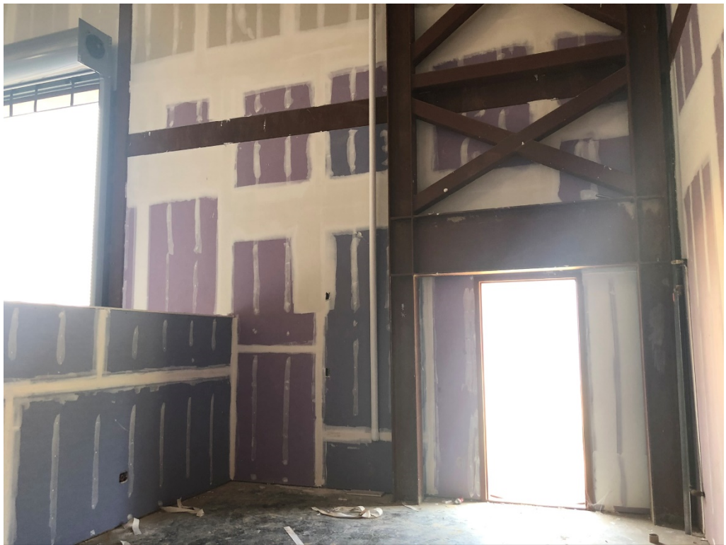
Figure 16 – Gym Drywall Finishing
