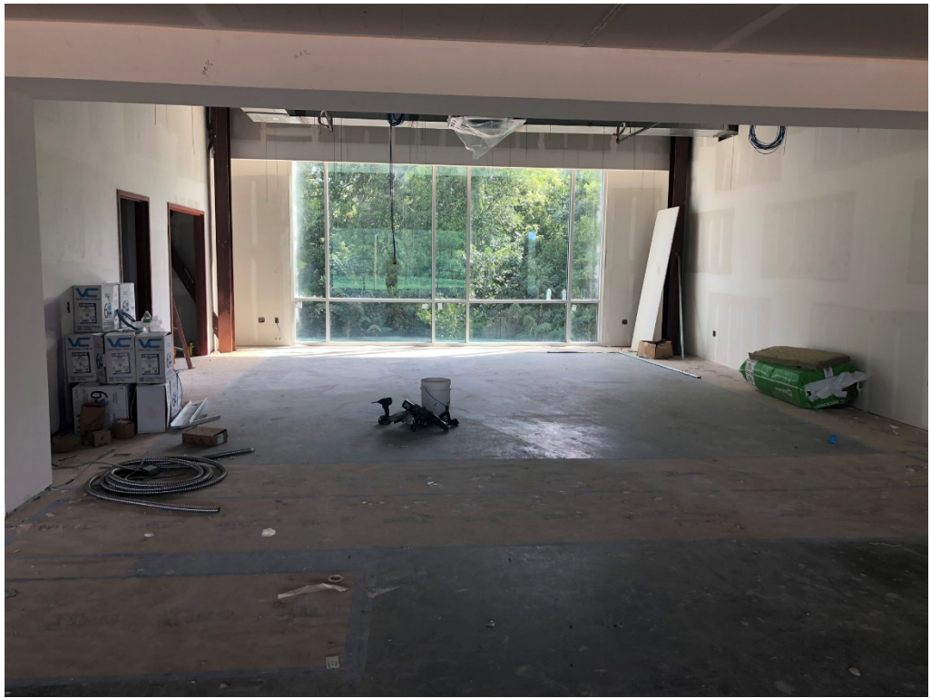
Figure 23 – Top Floor East Looking South
