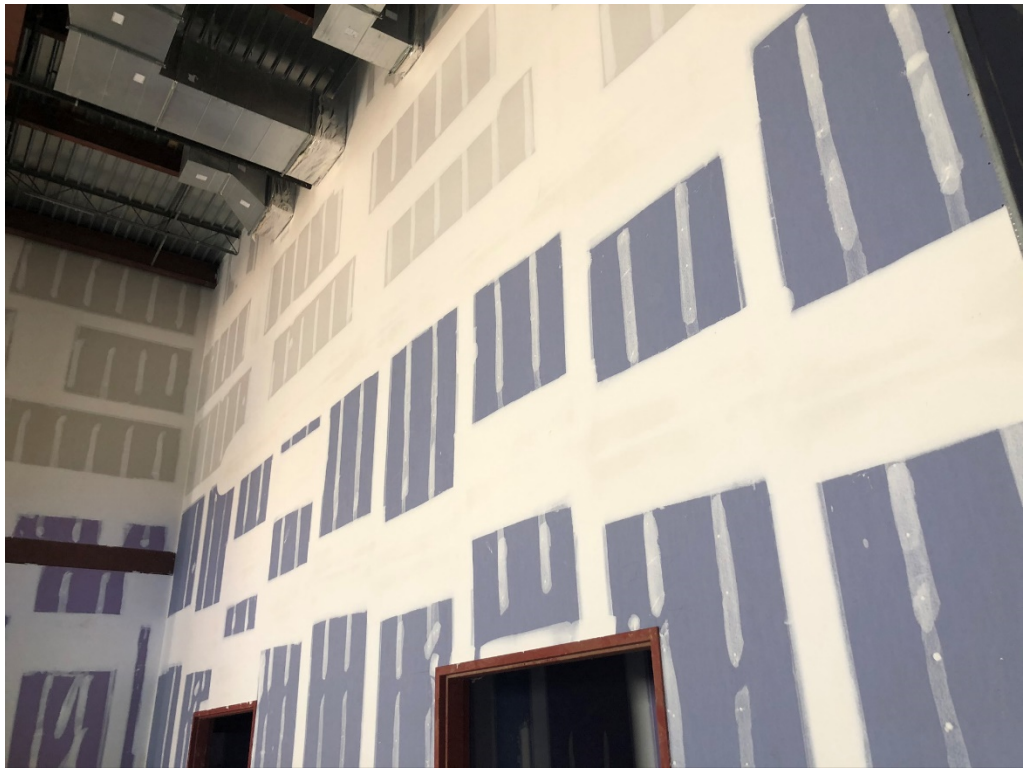
Figure 11 – Gym Drywall Finishing
