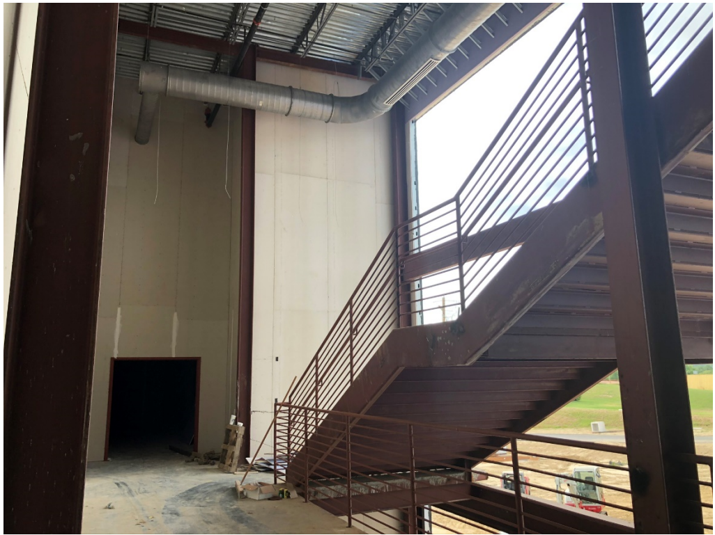
Figure 5 – 2 nd Floor at Corridor 154
