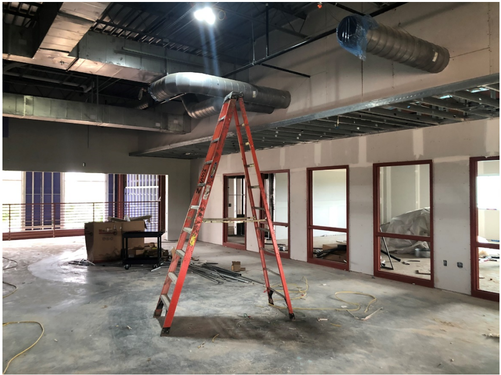
Figure 9 – HVAC Ducting Is On Going
