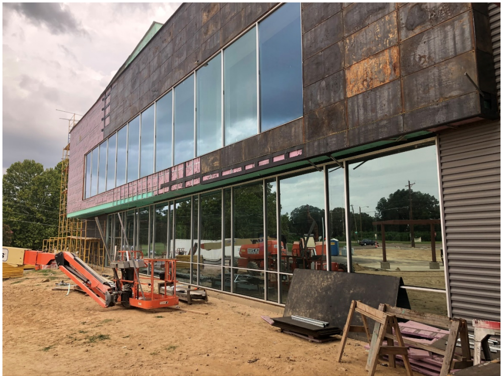
Figure 12 – North Elevation of East Structure
