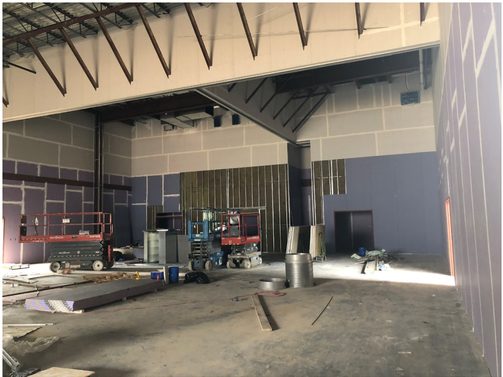
Figure 6 – Gym Drywall Mud Work
