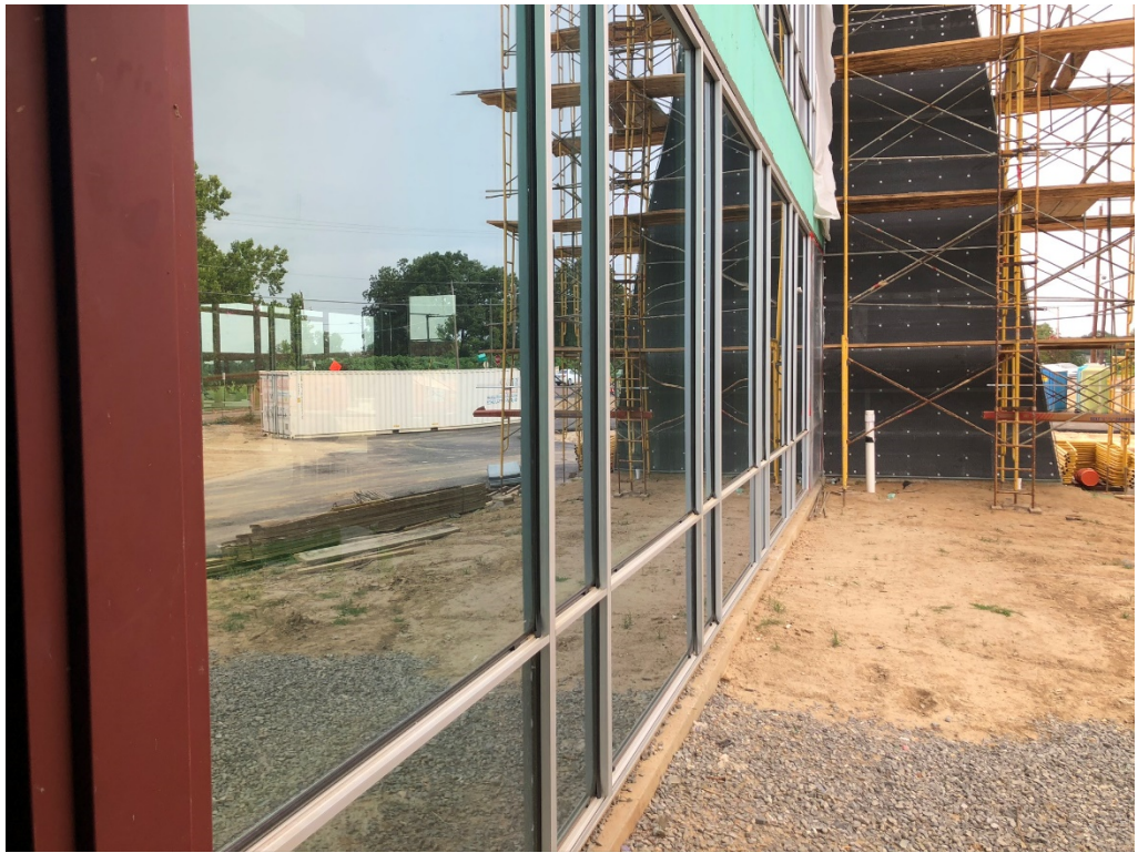
Figure 11 – East Elevation Glass Installed
