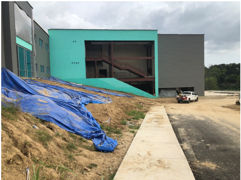
Figure 14 – North Elevation at West Structure
