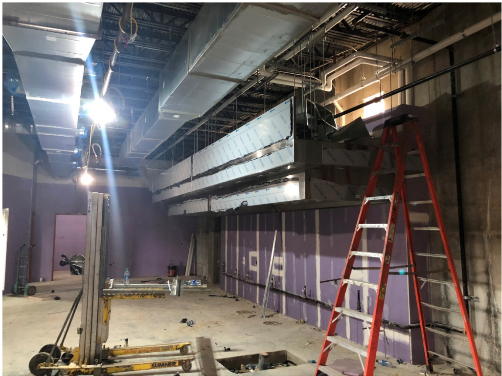
Figure 4 –Vent Hood Set In Place
