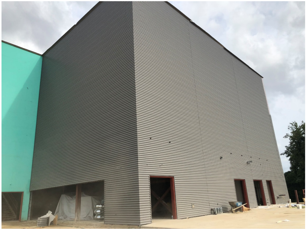
Figure 1 – Metal Siding Installed
