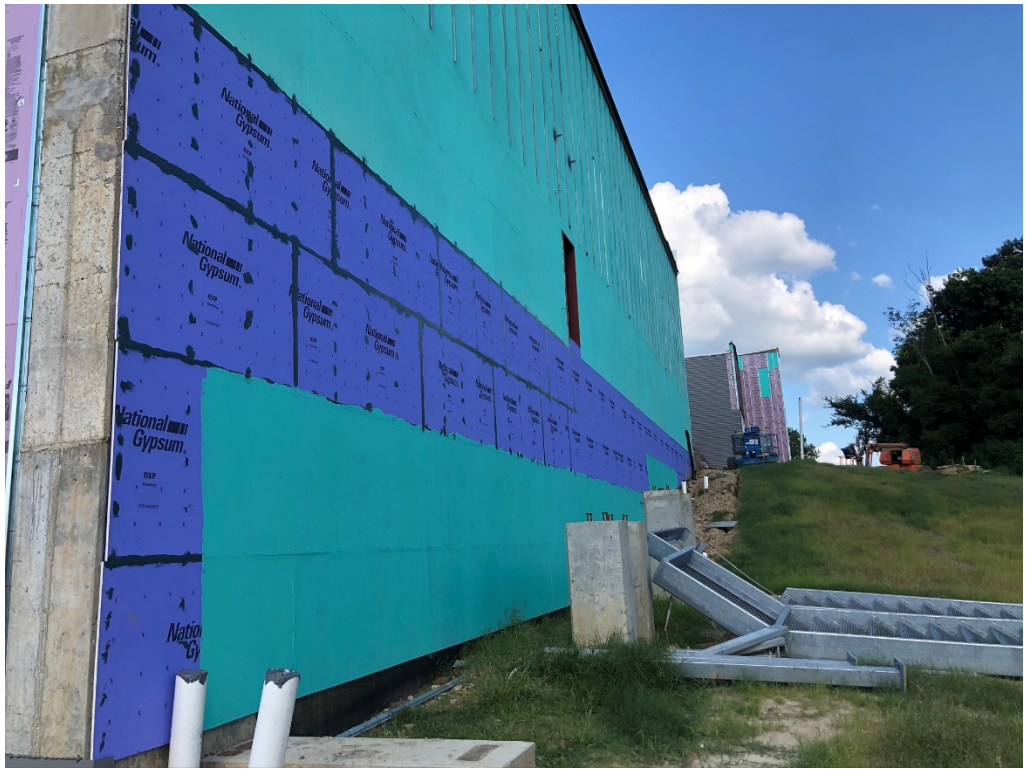
Figure 11 – South Façade of West Structure
