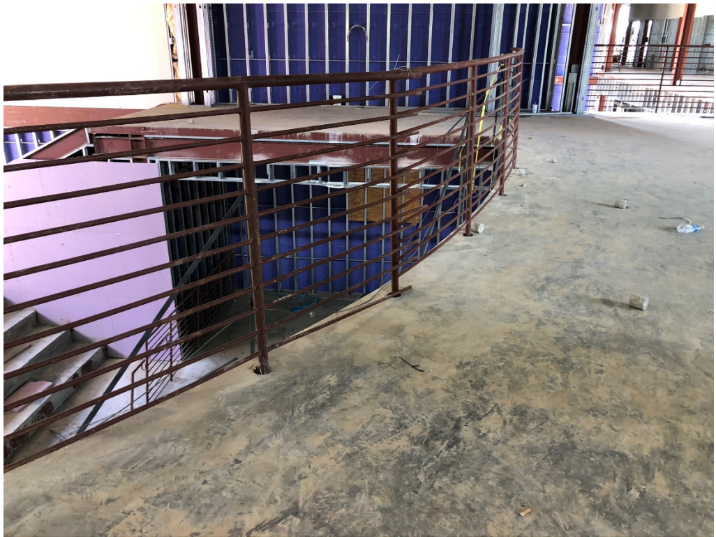
Figure 22 – Handrail Installation is Ongoing
