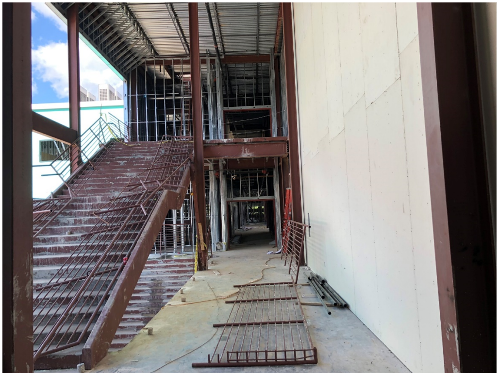
Figure 16 – Handrail Installation has Begun
