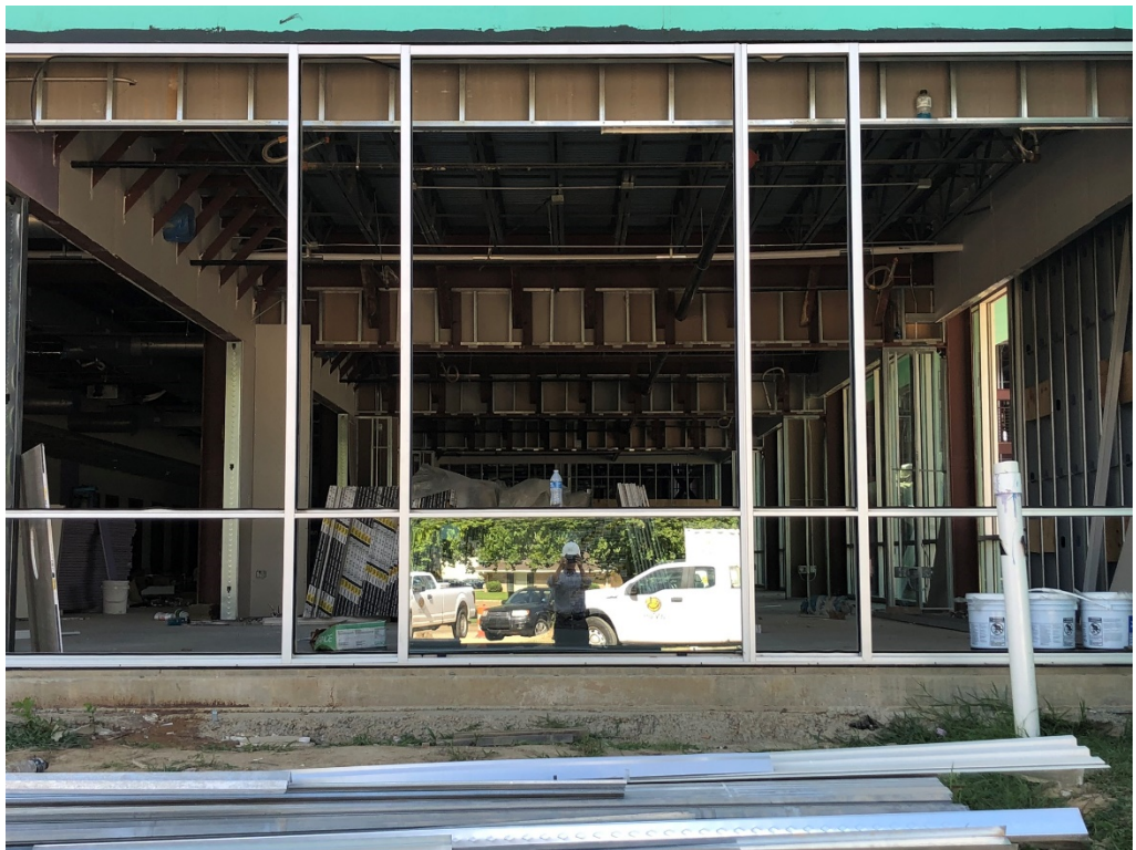
Figure 2 – Glass Installation has Begun
