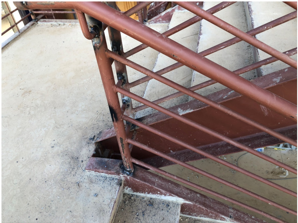
Figure 24 – Handrail Installation is Ongoing
