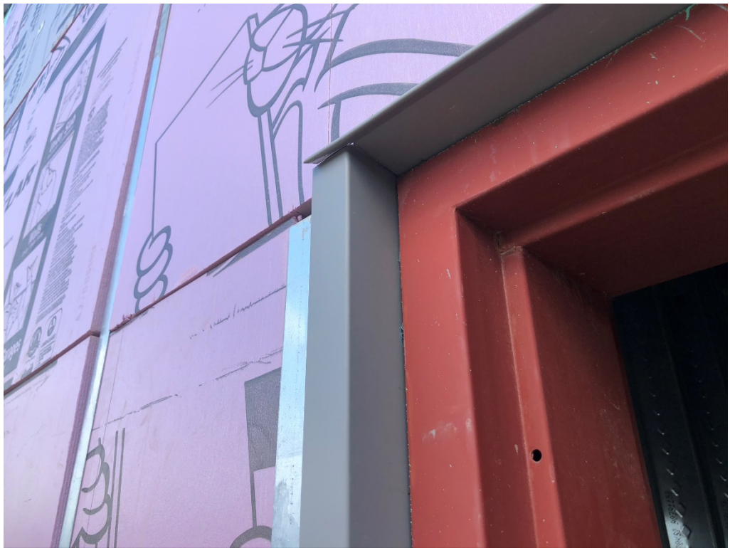
Figure 12 – Metal Trim Detail at Door
