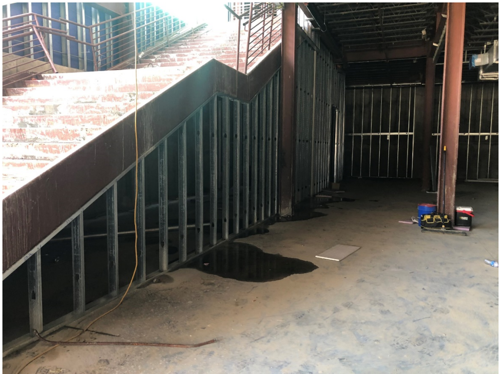
Figure 14 – Light Gauge Framing Under Main Stair
