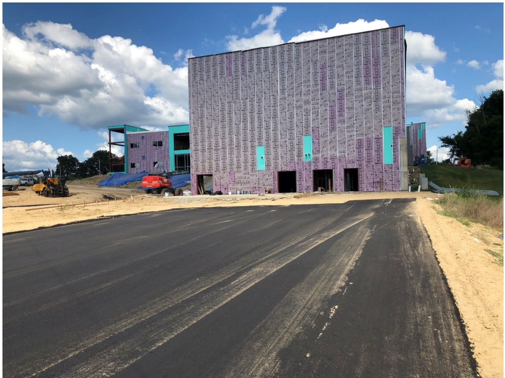
Figure 10 – Asphalt Installation is Ongoing
