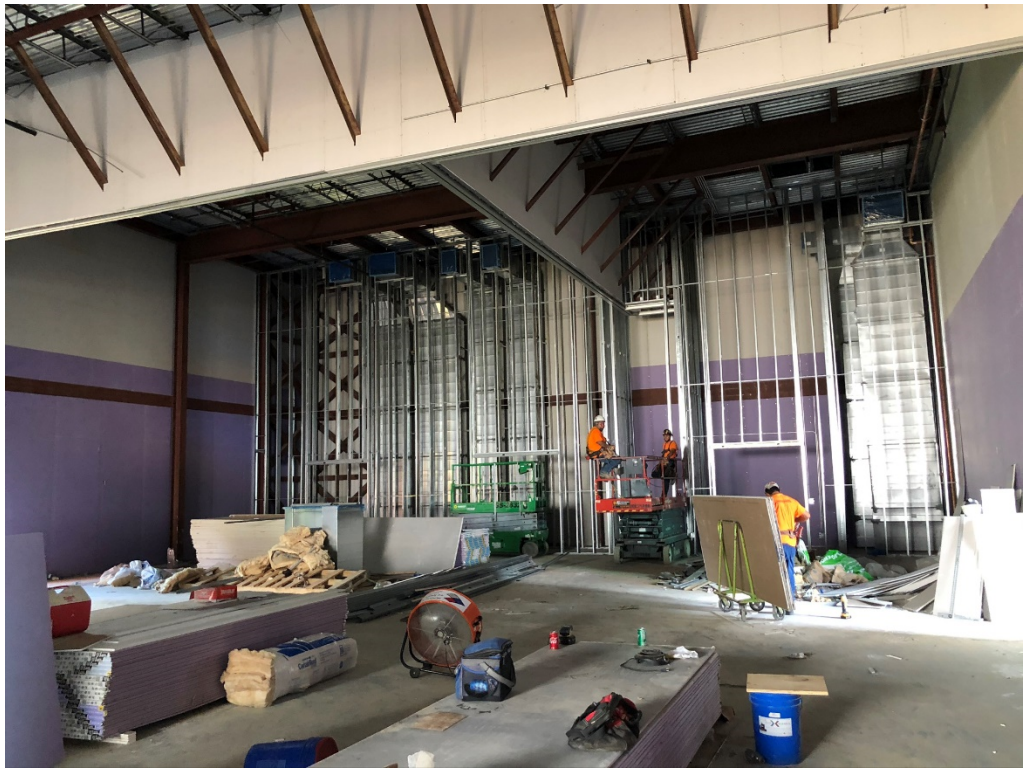
Figure 17 – Light Gauge Framing @ Gym
