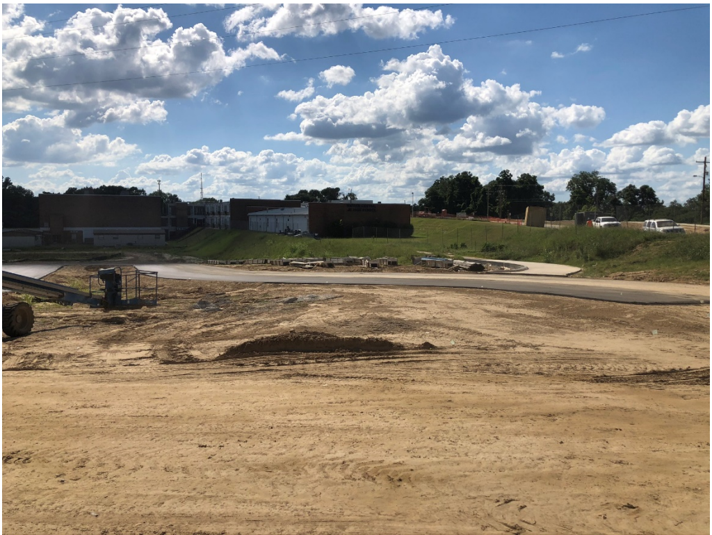
Figure 8 – Asphalt Installation is Ongoing
