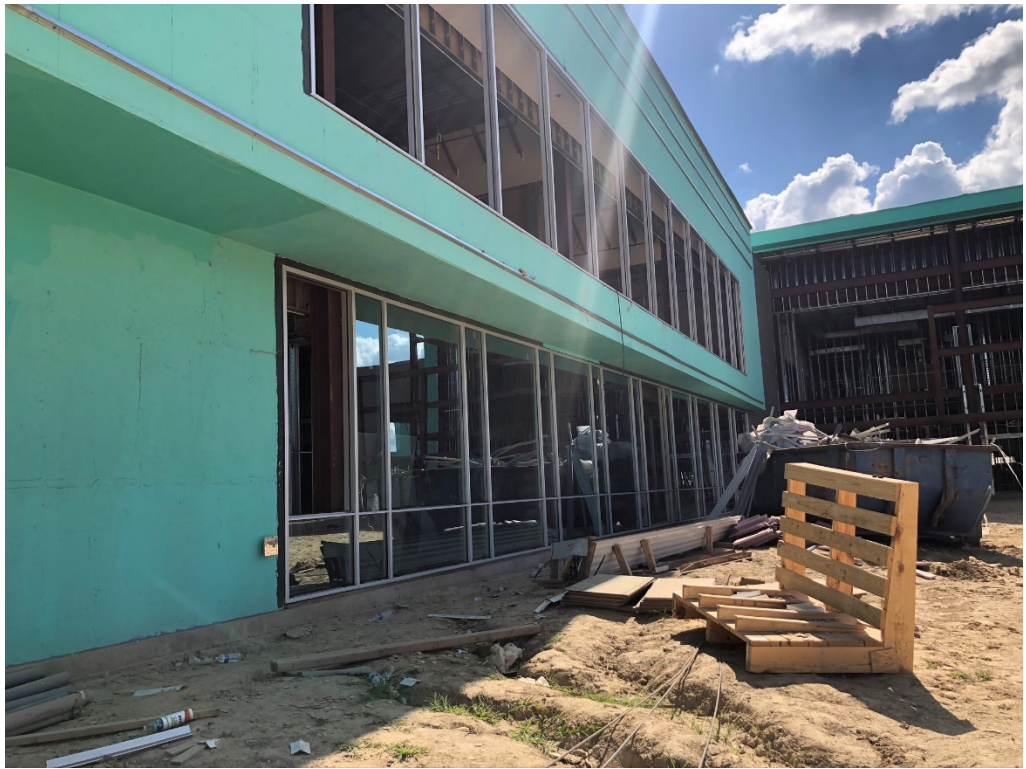
Figure 3 – Storefront Install is Ongoing
