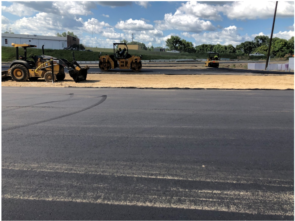
Figure 9 – Asphalt Installation is Ongoing
