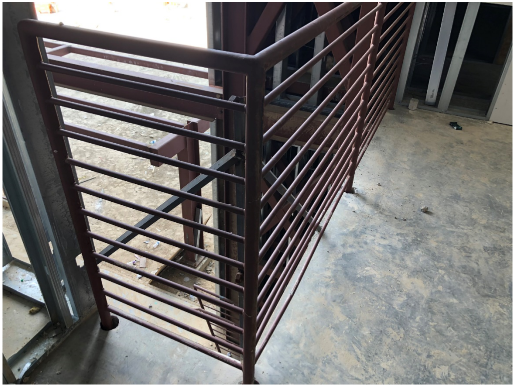
Figure 21 – Handrail Installation is Ongoing
