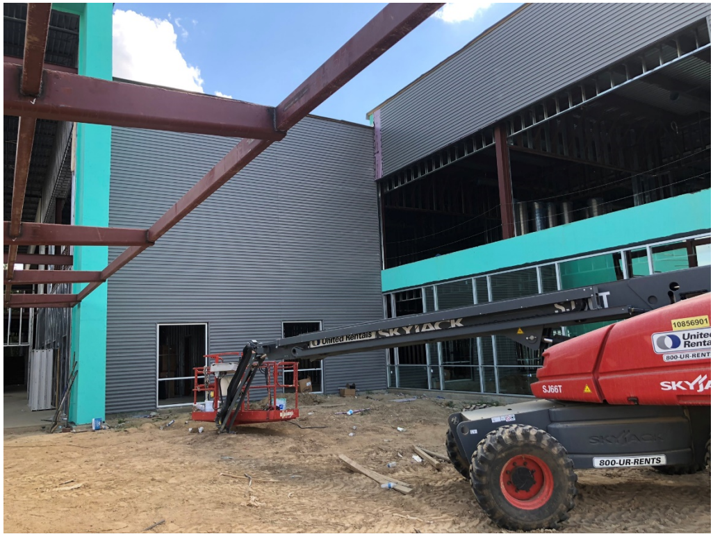
Figure 5 – Metal Siding Install is Ongoing
