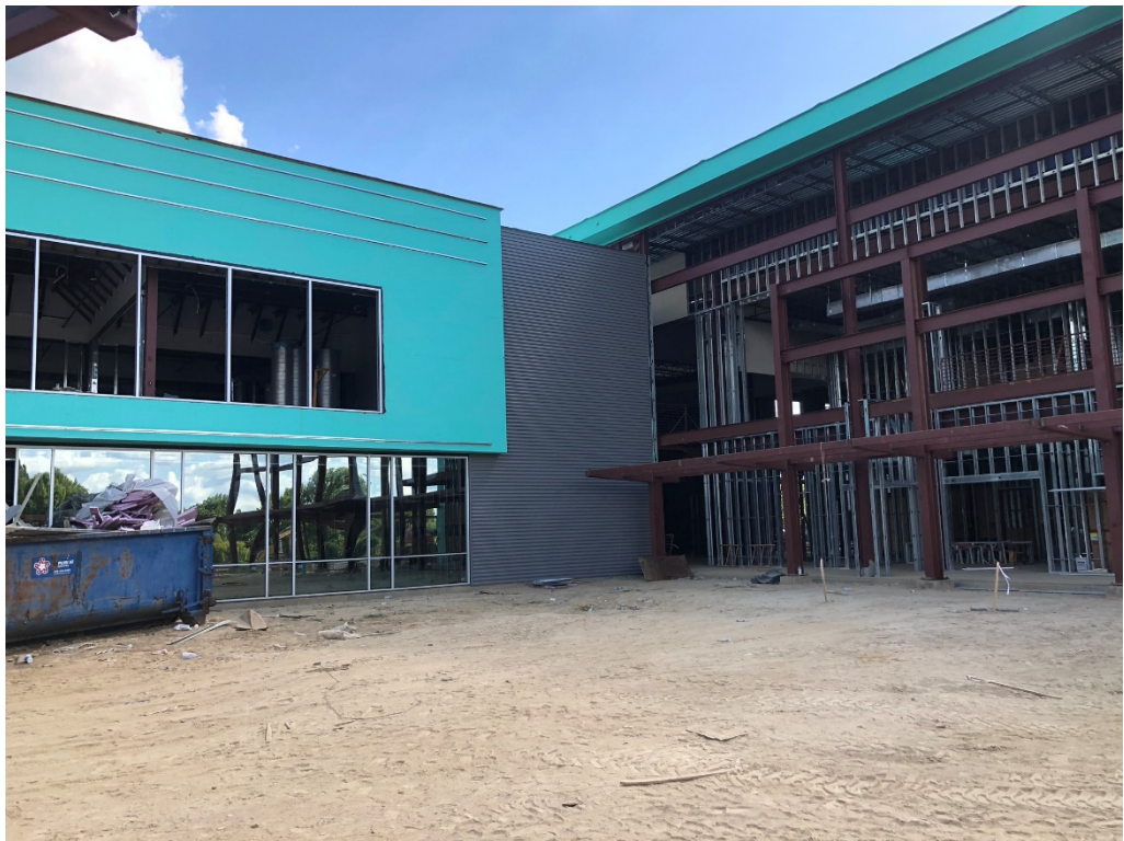
Figure 4 –Metal Siding Install is Ongoing
