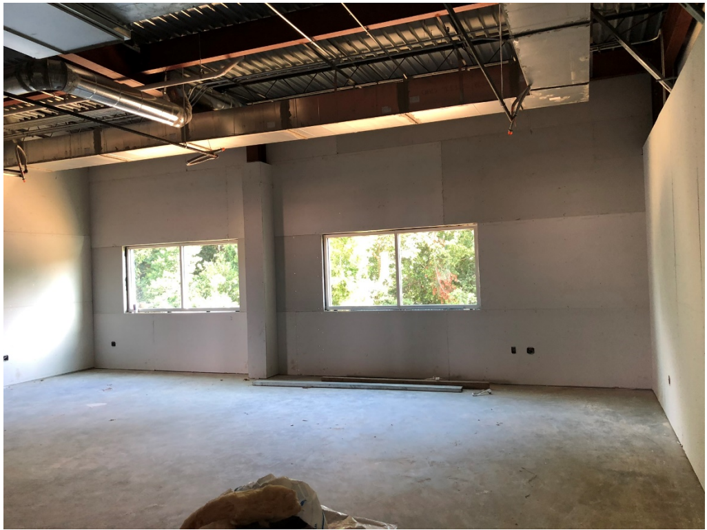
Figure 23 – Drywall Panel Installation at East Structure is Nearing Completion
