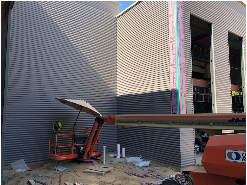
Figure 18 – Metal Panel Install at Rear Courtyard
