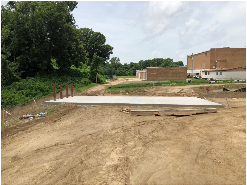
Figure 17 – Dumpster Pad Installed
