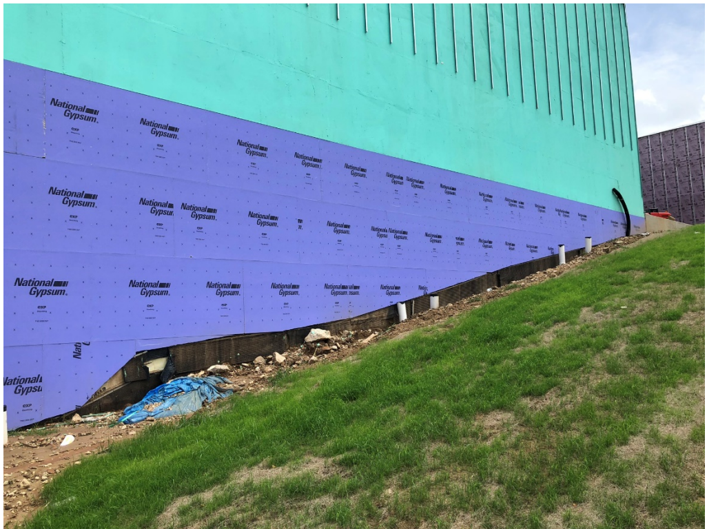
Figure 18 – Waterproofing is Ongoing
