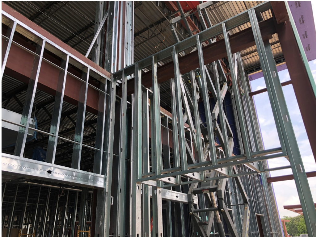
Figure 7 – Steel Light Gauge Framing is Ongoing
