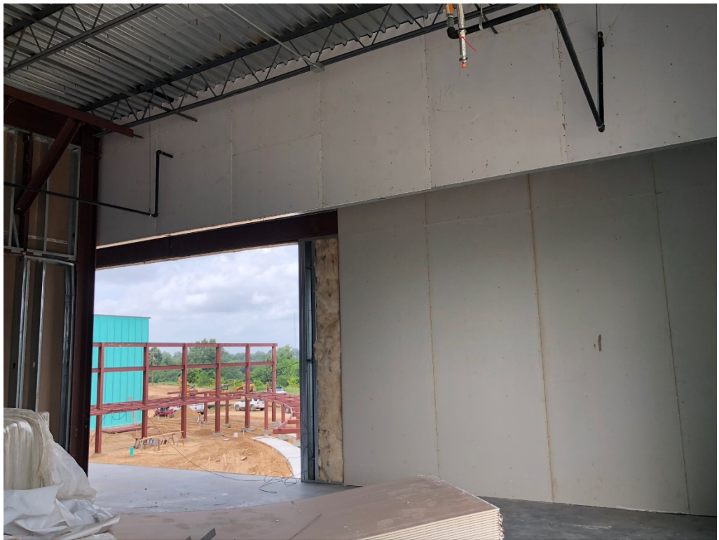
Figure 8 – Drywall Install is Ongoing
