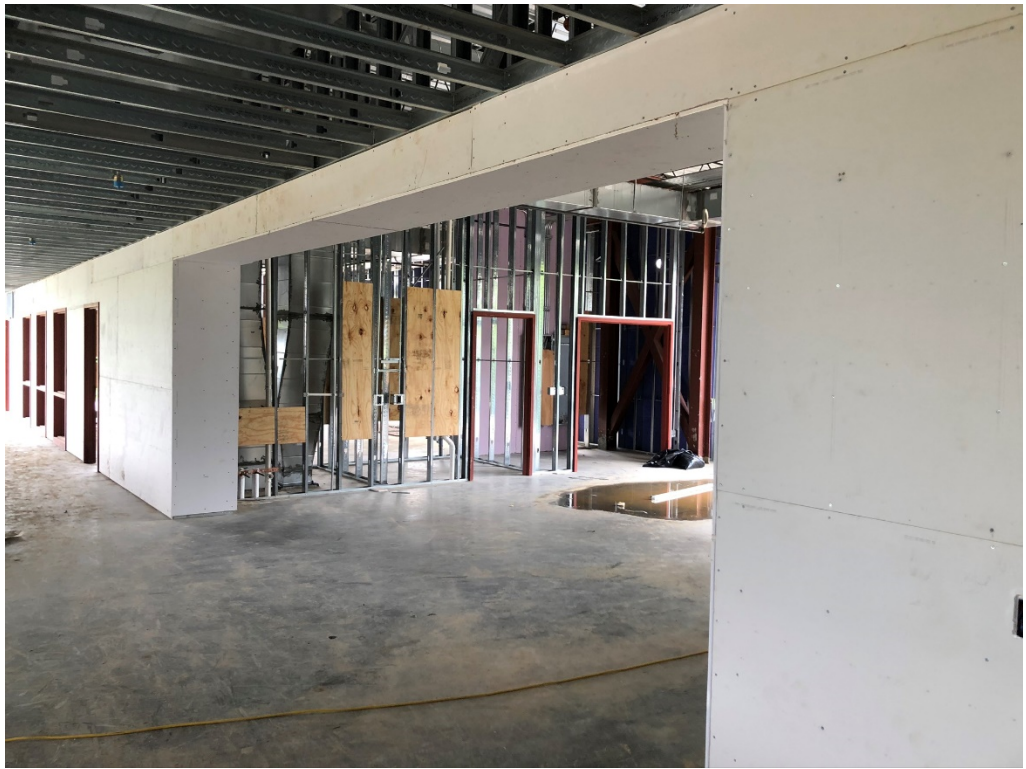
Figure 9 – Drywall Install is Ongoing
