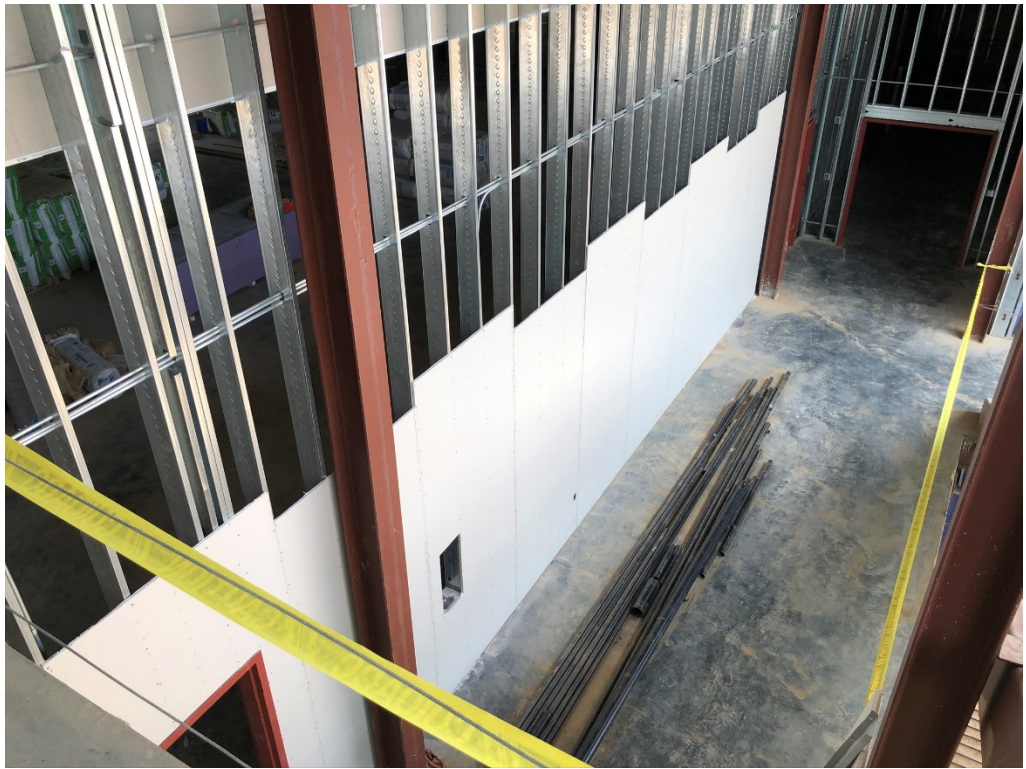
Figure 11 – Drywall Install at Gym
