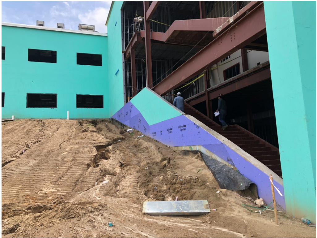
Figure 15 – Waterproofing is Ongoing
