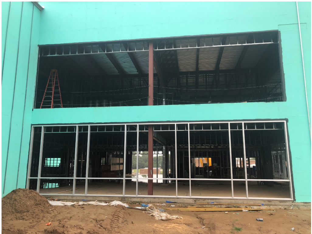
Figure 6 – Aluminum Storefront Installation is Ongoing
