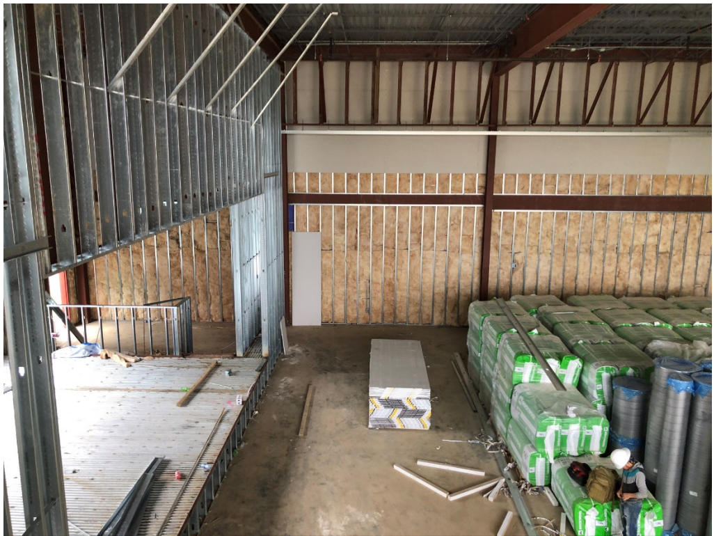
Figure 16 – Insulation & Framing @ Gym
