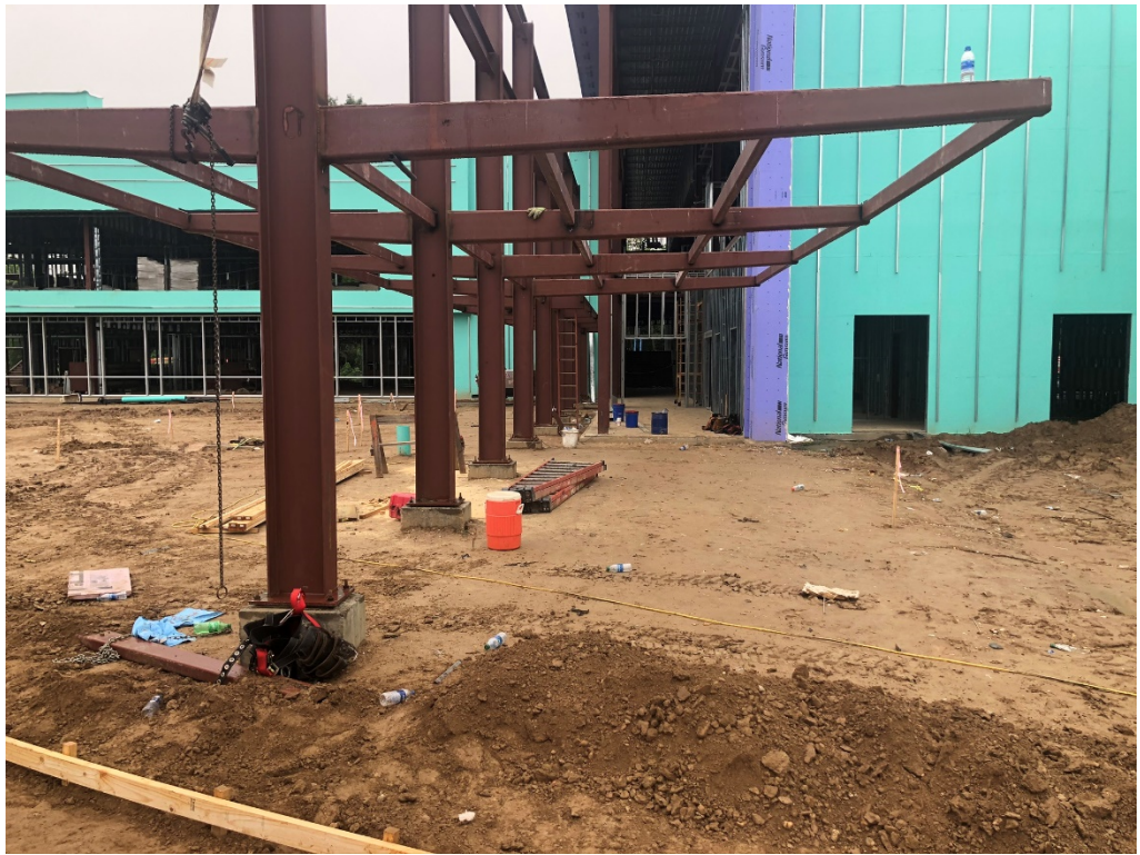
Figure 5 – Steel Framing @ Entry
