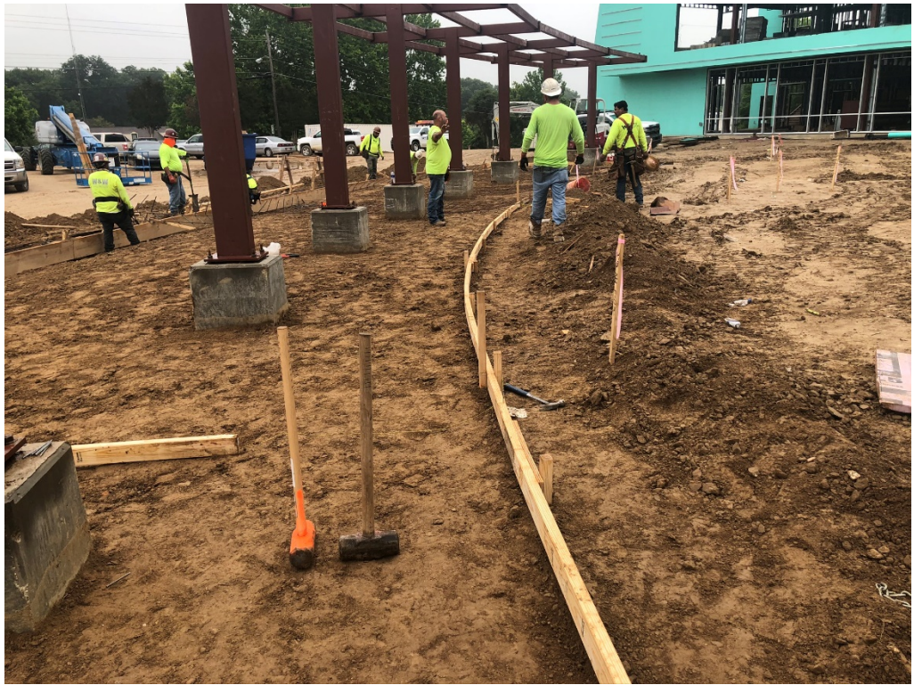
Figure 3 – Drop Off Concrete Form Curve
