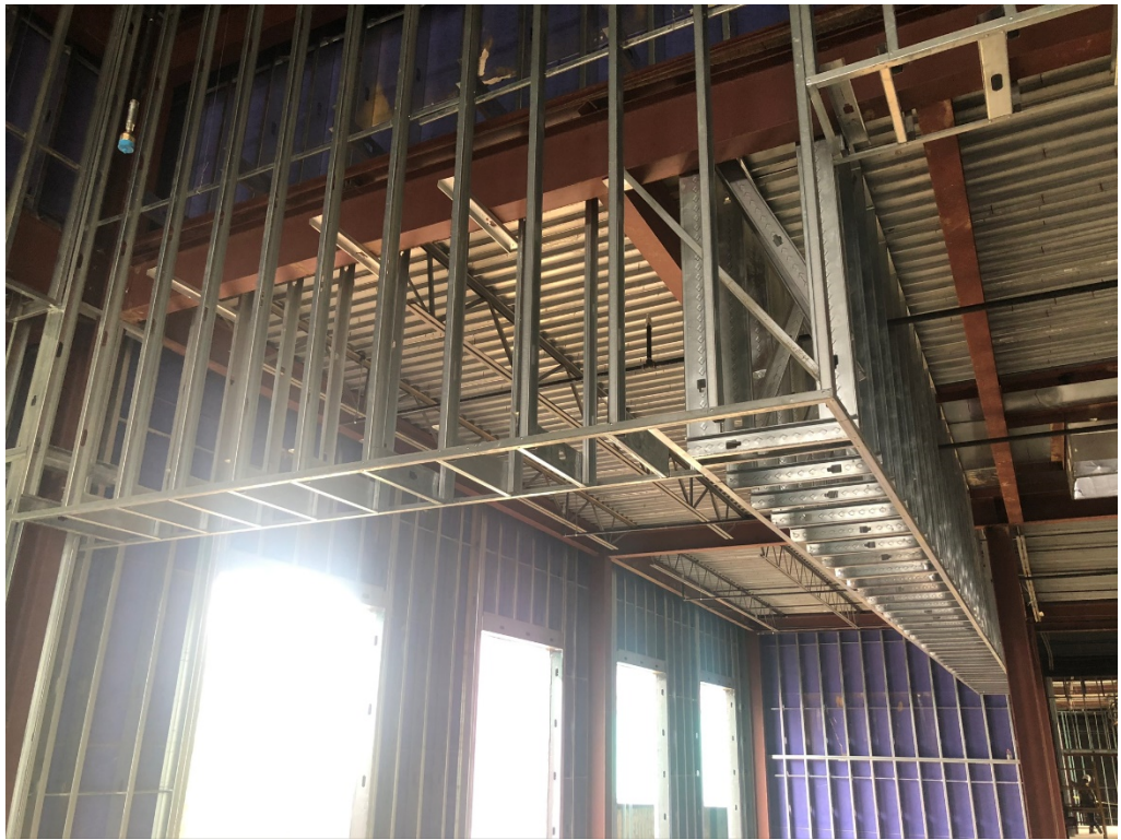
Figure 13 – Light Gauge Framing Furr Downs
