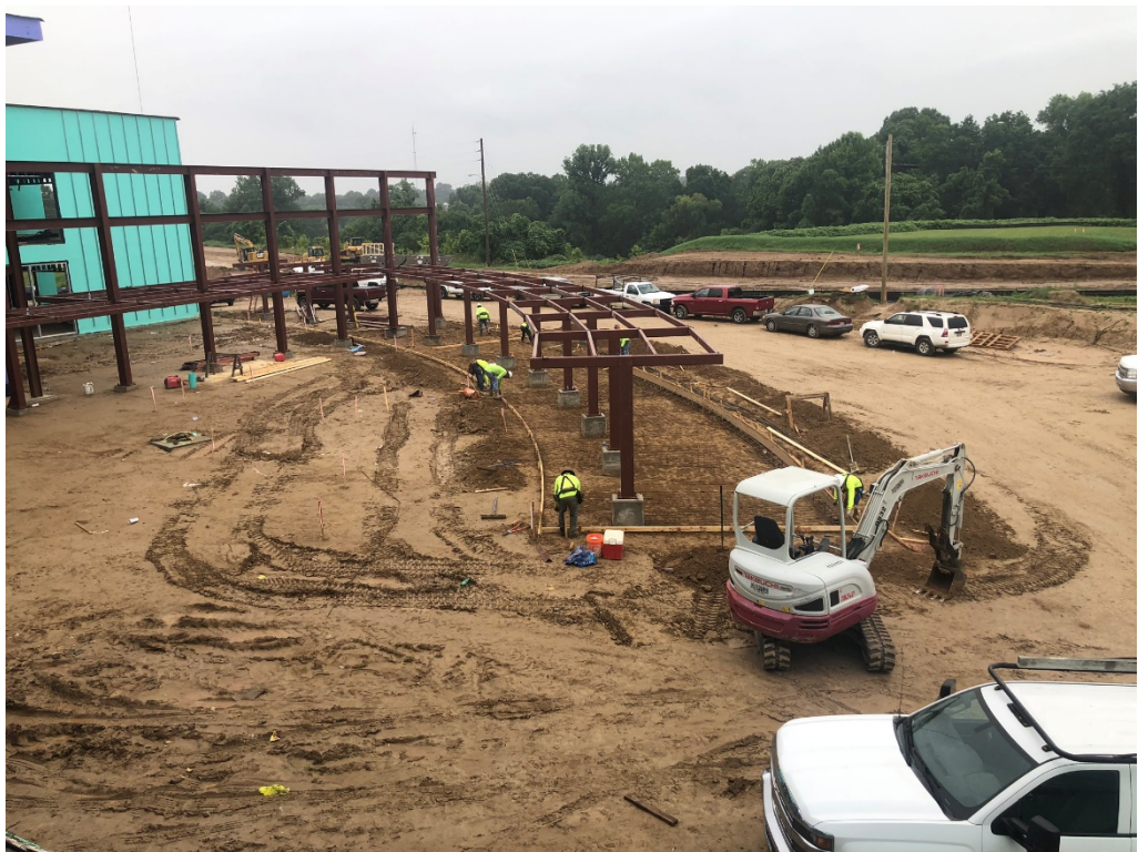
Figure 4 –Formwork from Above
