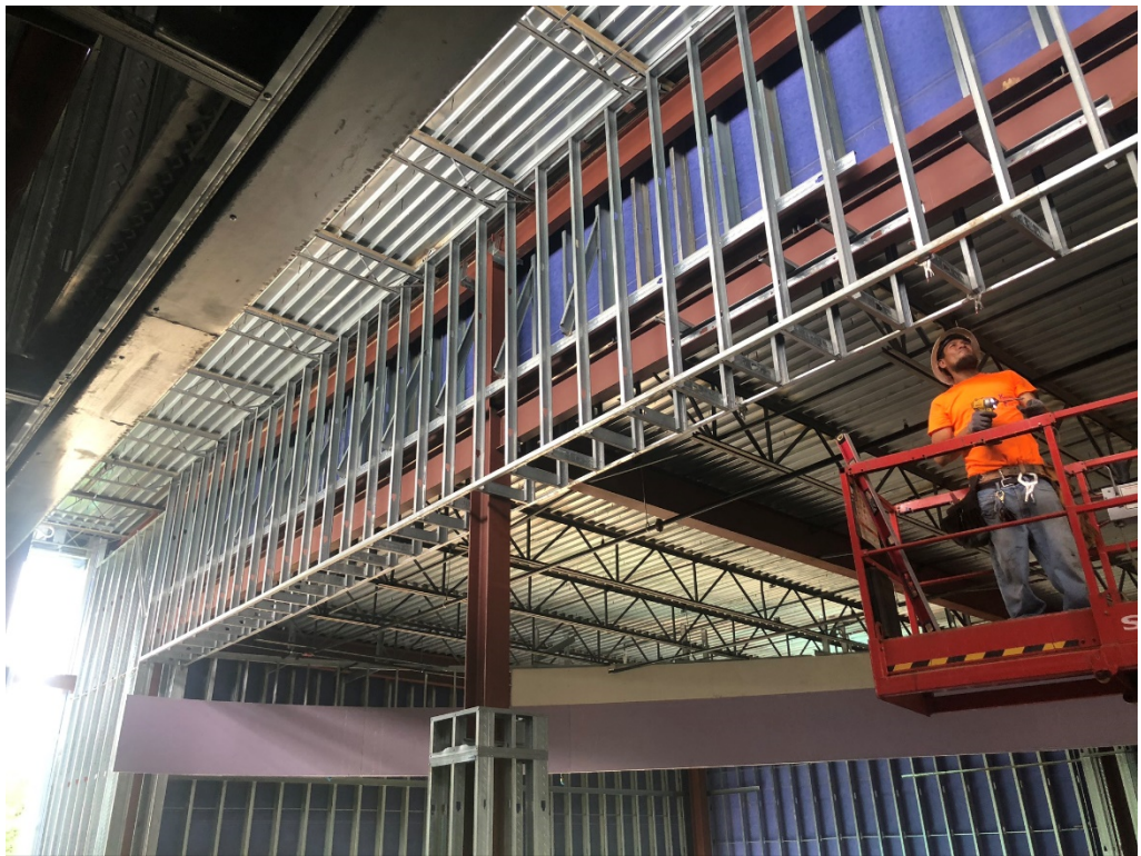
Figure 12 – Light Gauge Framing Furr Downs
