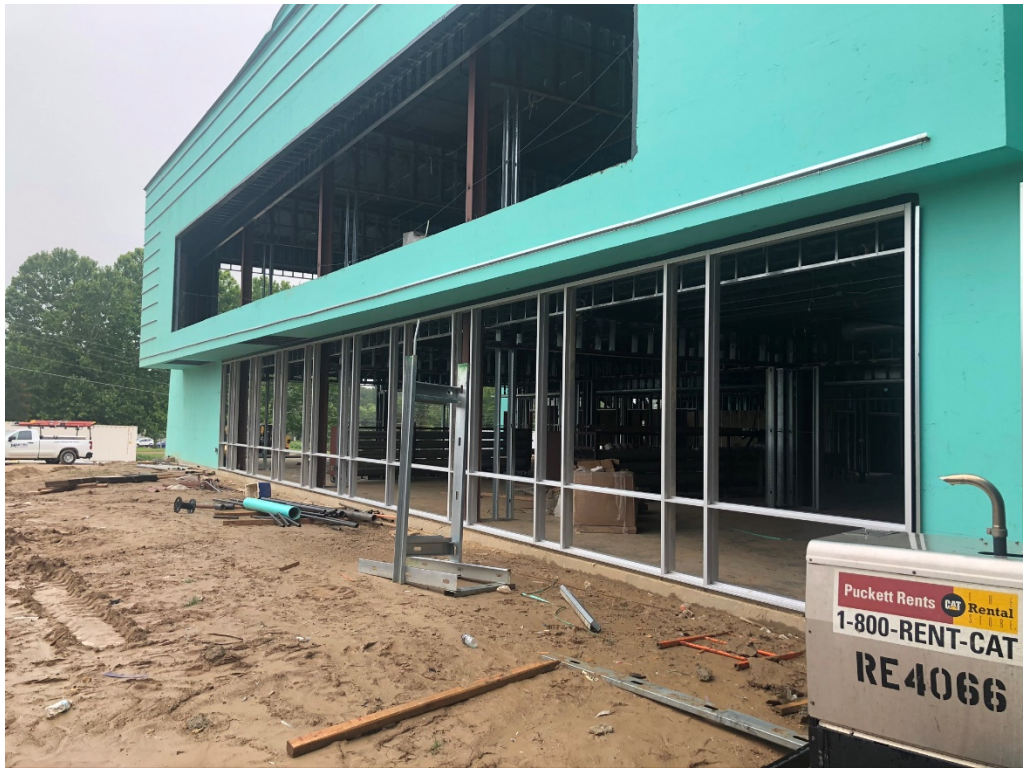
Figure 7 – Aluminum Storefront Installation is Ongoing
