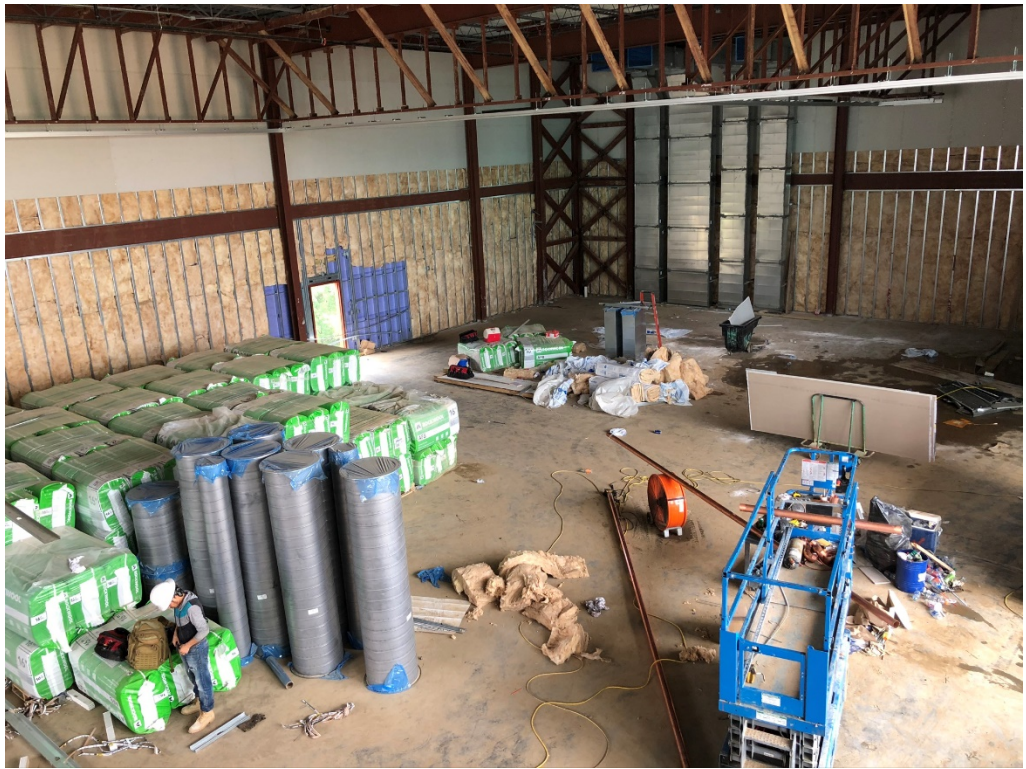
Figure 17 – Insulation & Framing @ Gym
