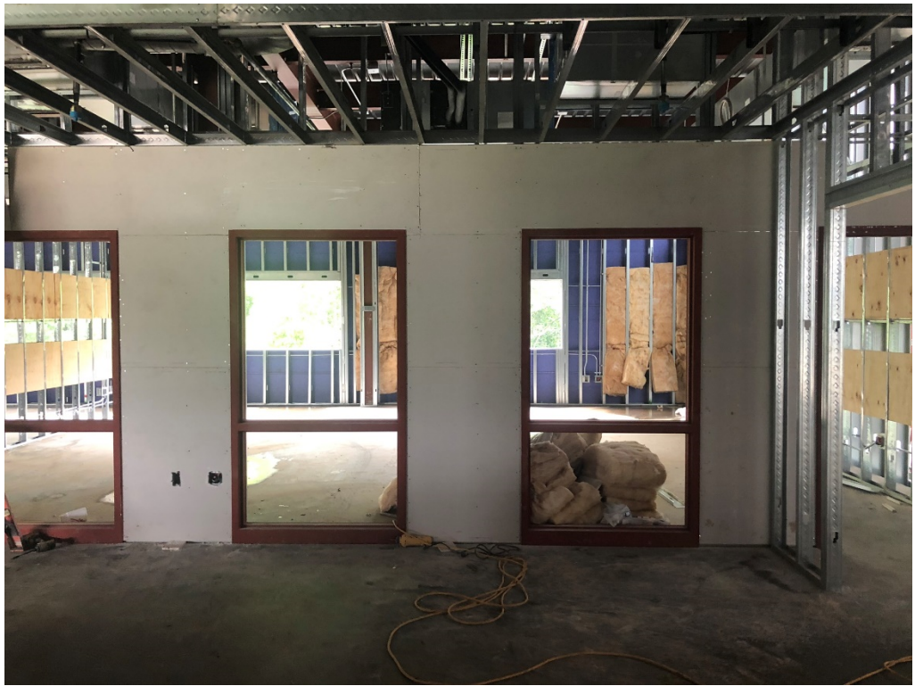
Figure 11 – Upper Level East Building Drywall and Insulation
