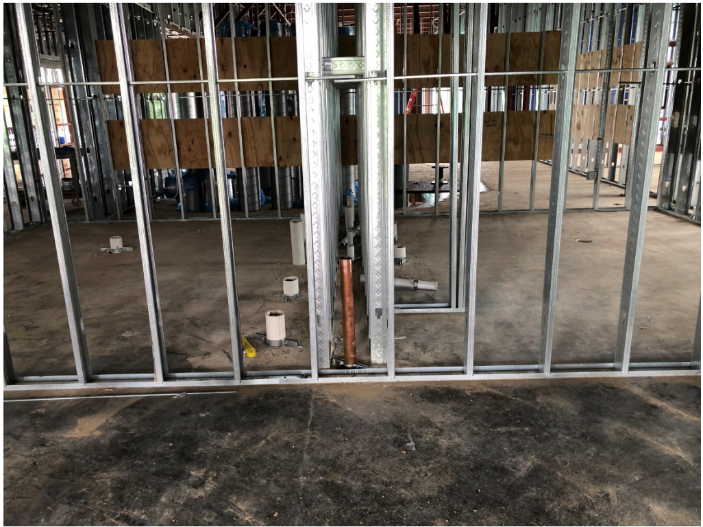
Figure 15 – Plumbing Rough in @ 228 & 229
