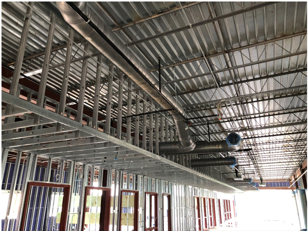
Figure 18 – Furr Down and Ducting Work @ Upper Level North Building
