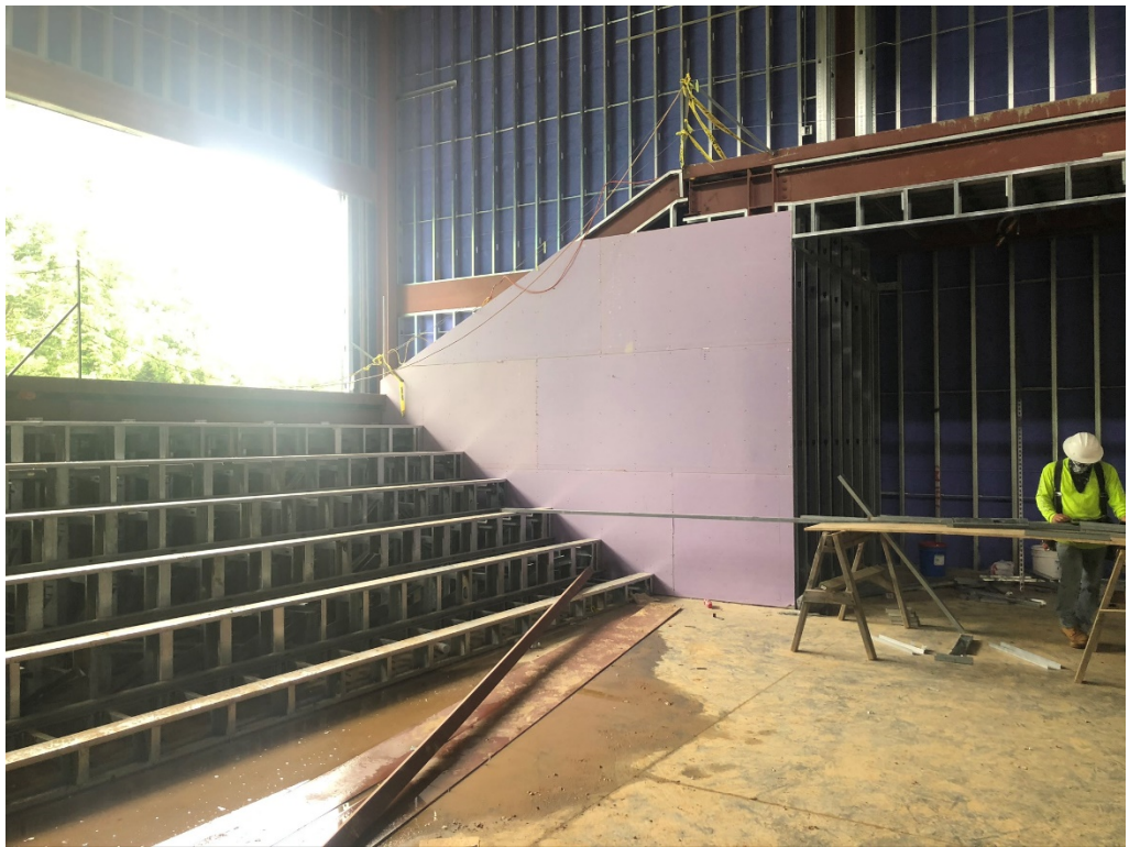
Figure 8 – Interior Drywall Work
