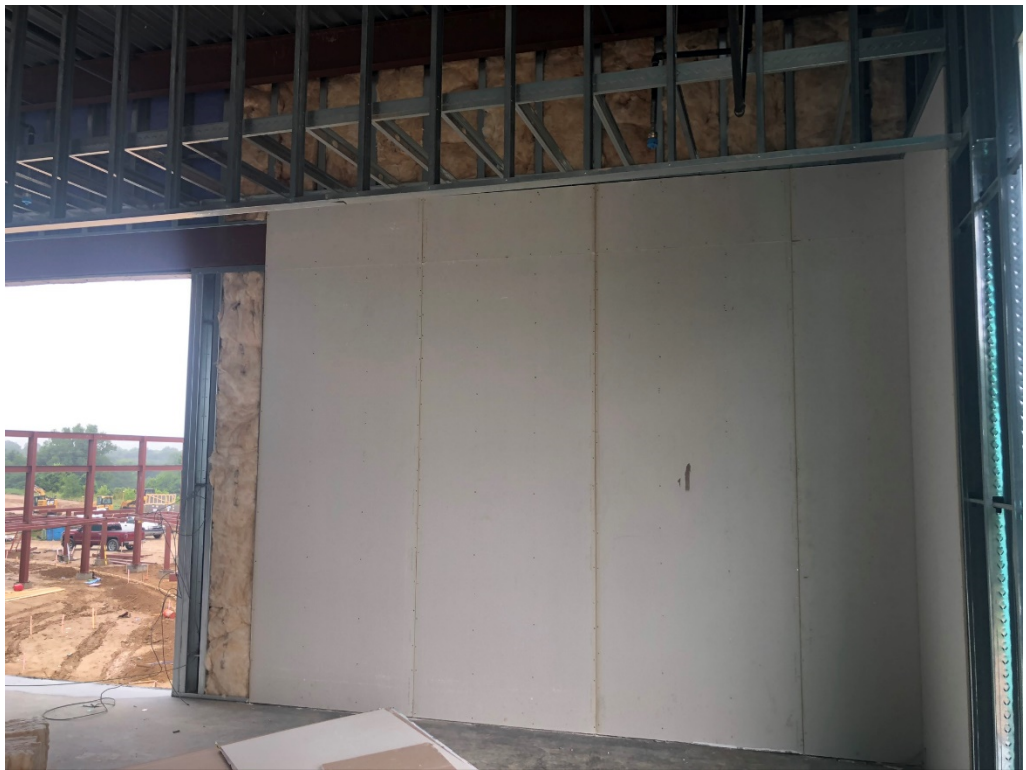
Figure 10 – Upper Level East Building Drywall and Insulation
