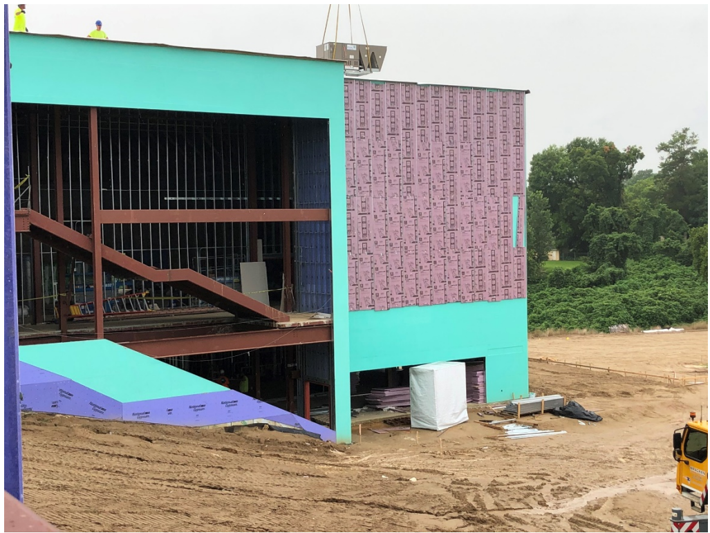
Figure 19 – Insulation Board Install @ Exterior Wall is Ongoing
