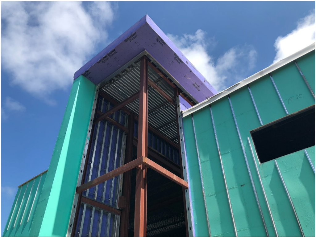
Figure 7 – South Curtain Wall
