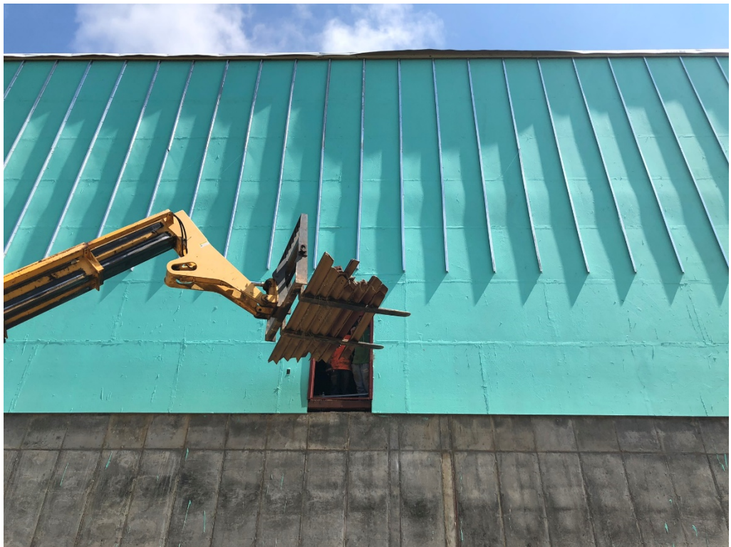
Figure 6 – Metal Panel Clip Installation Nearing Completion
