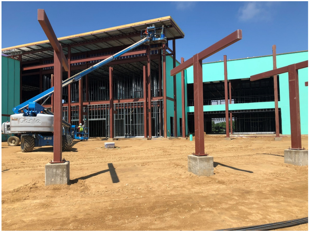
Figure 3 – Soffit Framing Hearing Completion
