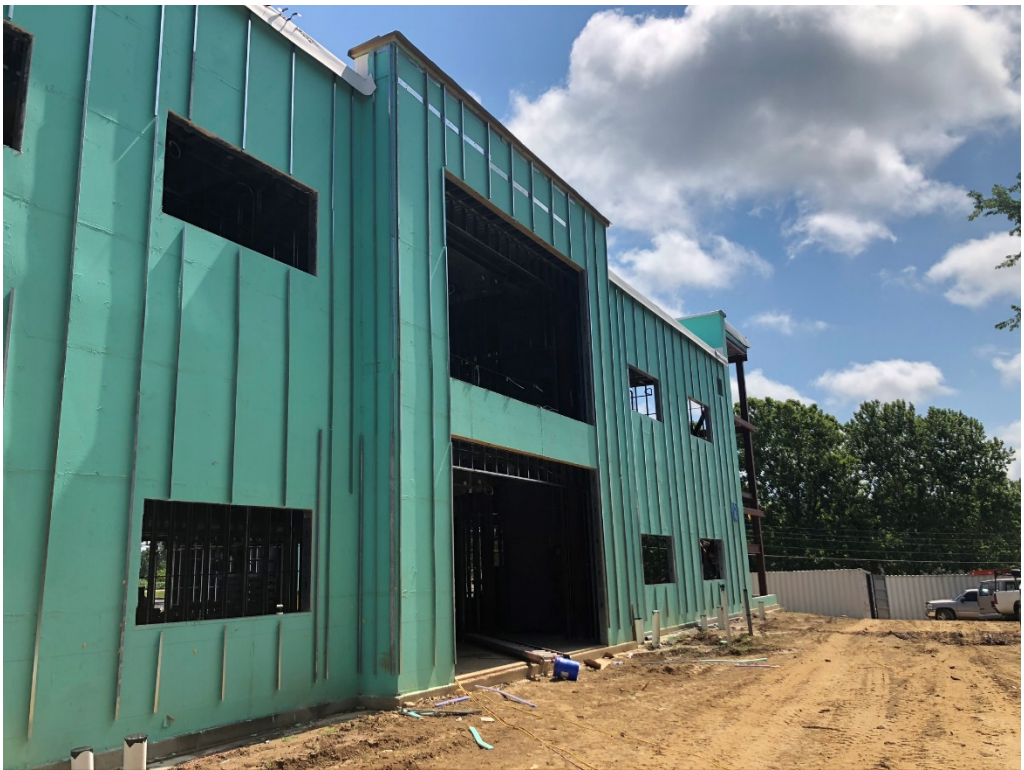
Figure 8 – East Section of Building
