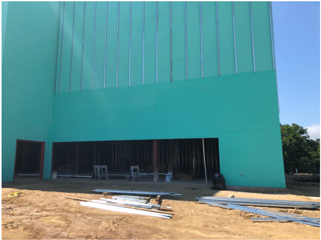
Figure 5 – West Building Seathing
