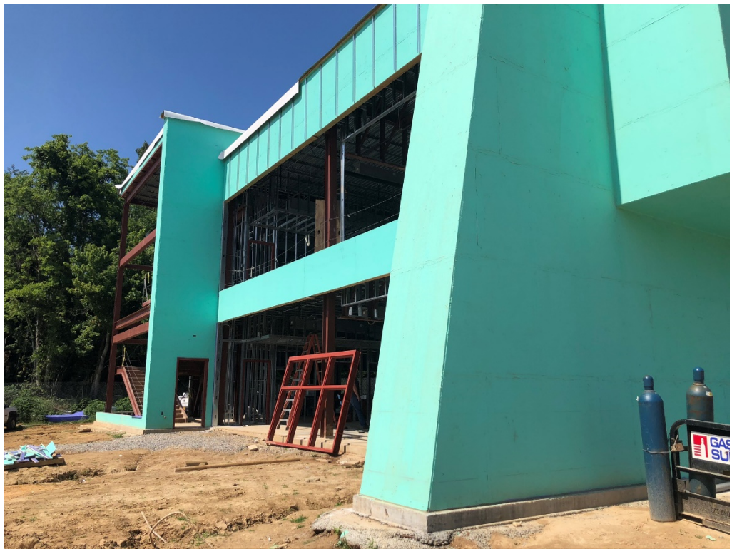
Figure 2 – Northeast Corner of Structure
