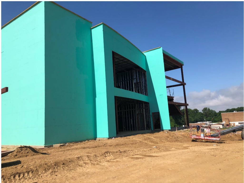
Figure 4 –Exterior Sheathing Nearing Completion; North Section of Building
