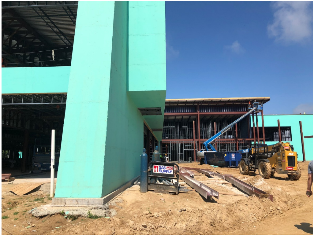
Figure 1 – Northeast Corner of Structure
