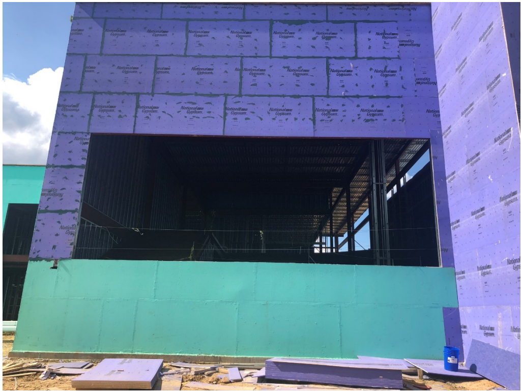
Figure 3 – South Lobby Stair
