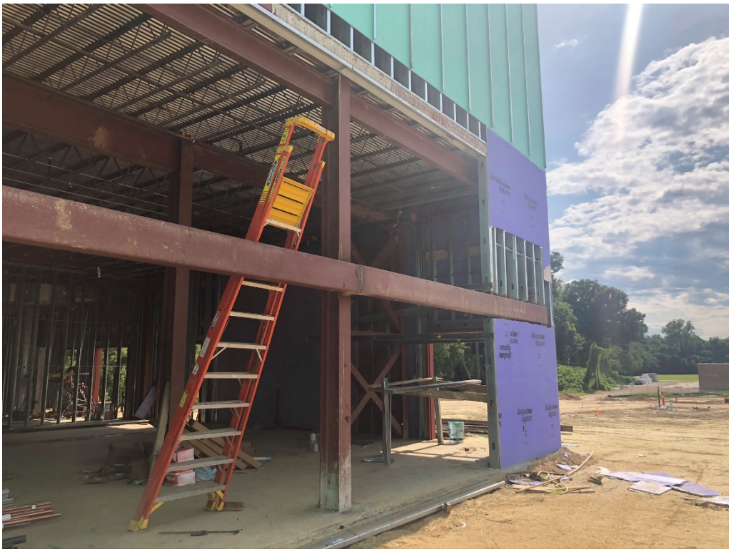
Figure 6 – Sheathing is Ongoing
