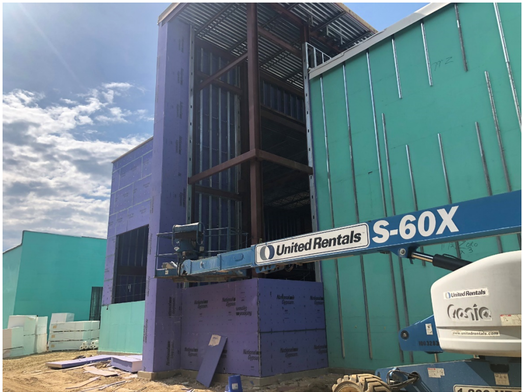
Figure 2 – South Lobby Opening
