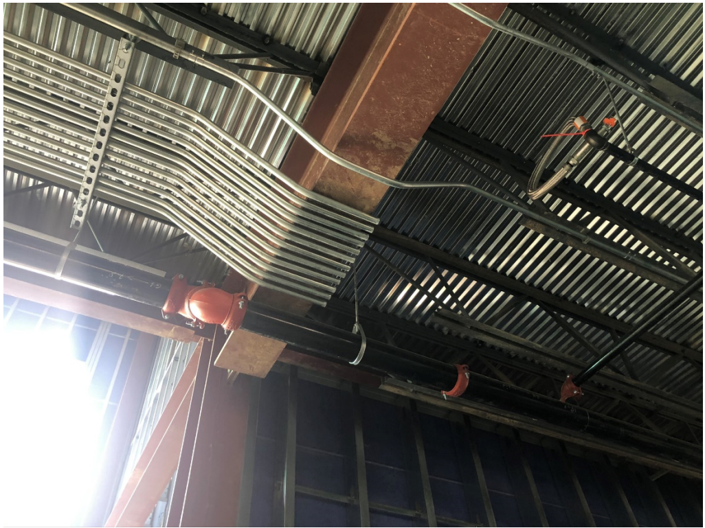
Figure 7 – Services Installation is Ongoing
