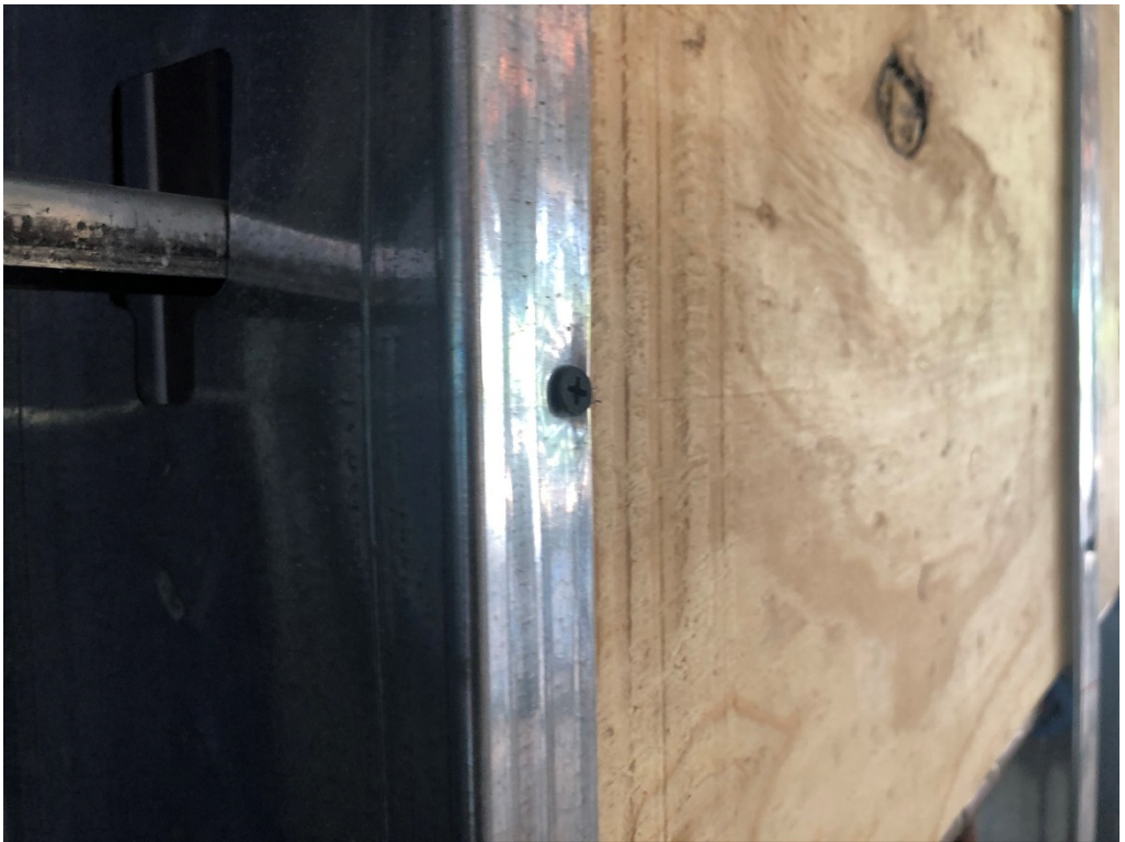
Figure 10 – Black Phosphate Screws used at Plywood Blocking
