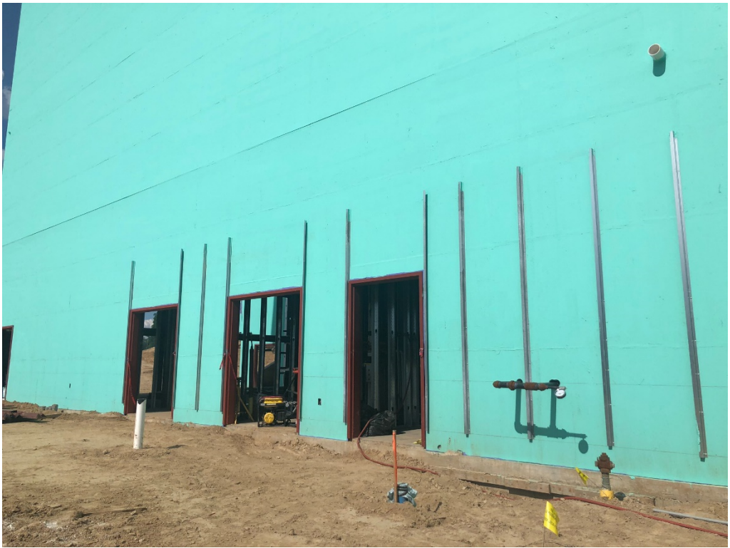
Figure 5 – Metal Channel Furring is Ongoing
