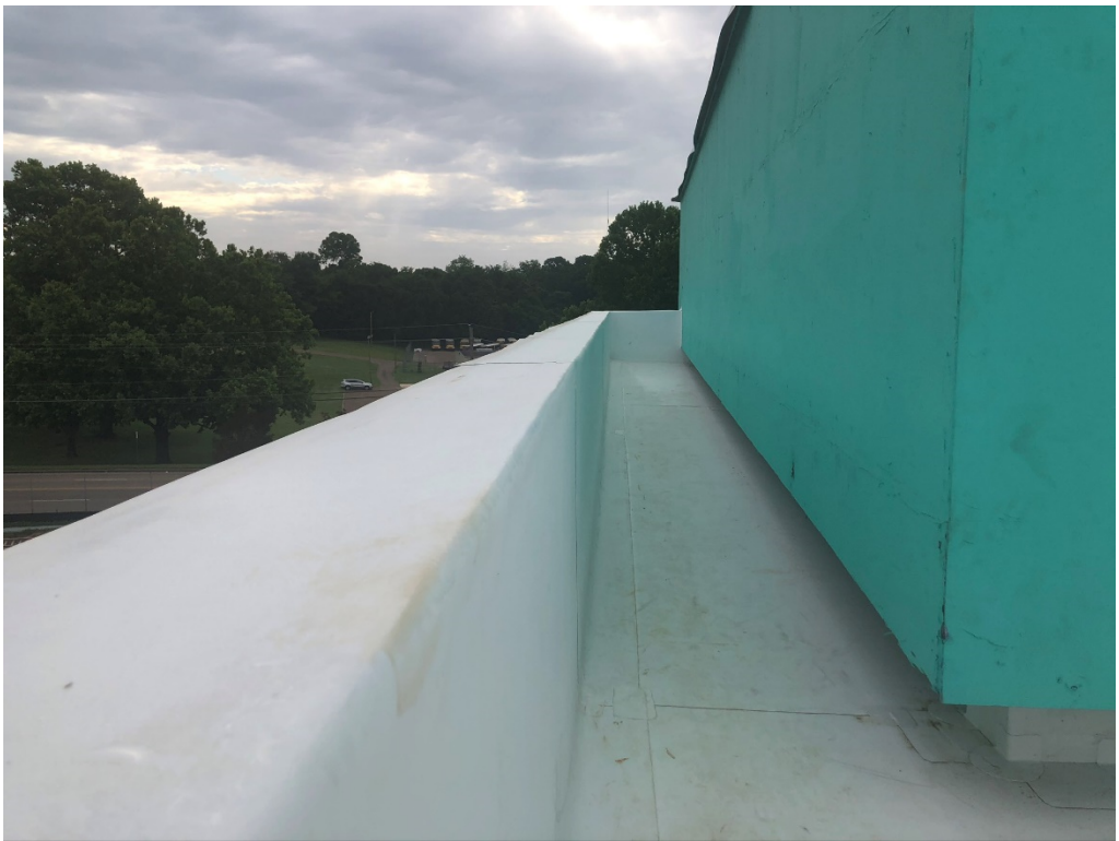
Figure 20 – North Parapet Wall at East Wing
