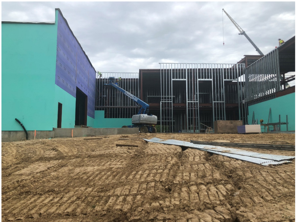
Figure 12 –South Façade at Center Building Section
