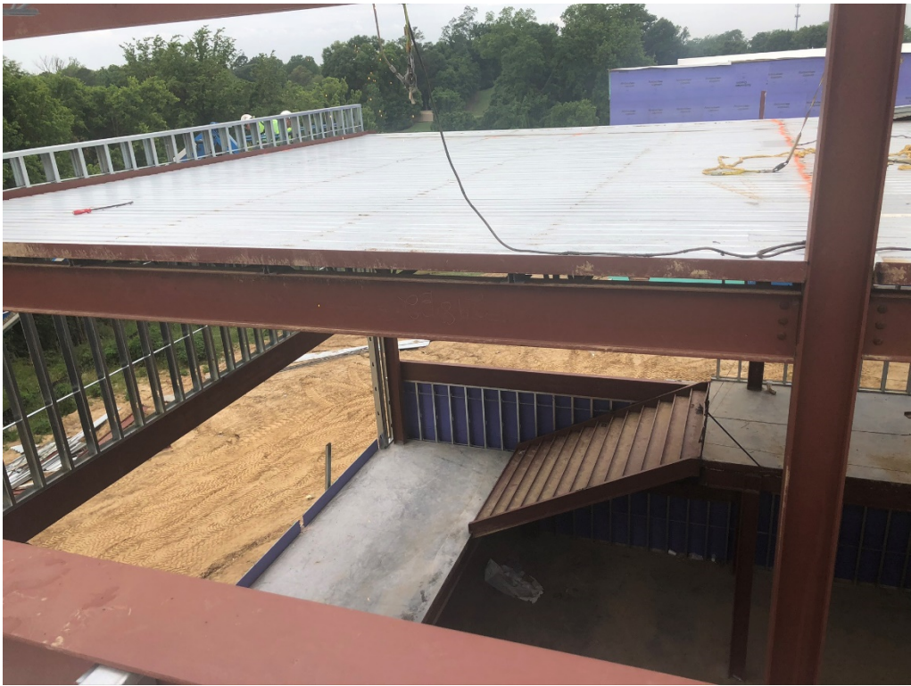
Figure 27 – Metal Decking is Ongoing at Center Section of Building
