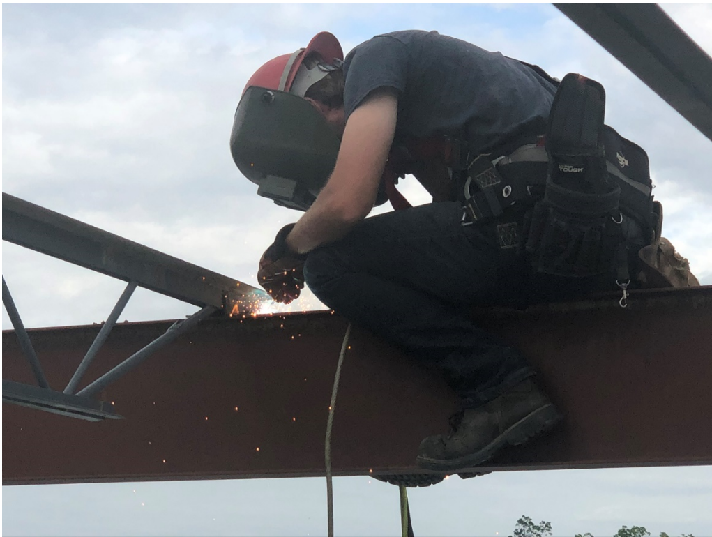
Figure 28 – Roof Joists Rafter Welding
