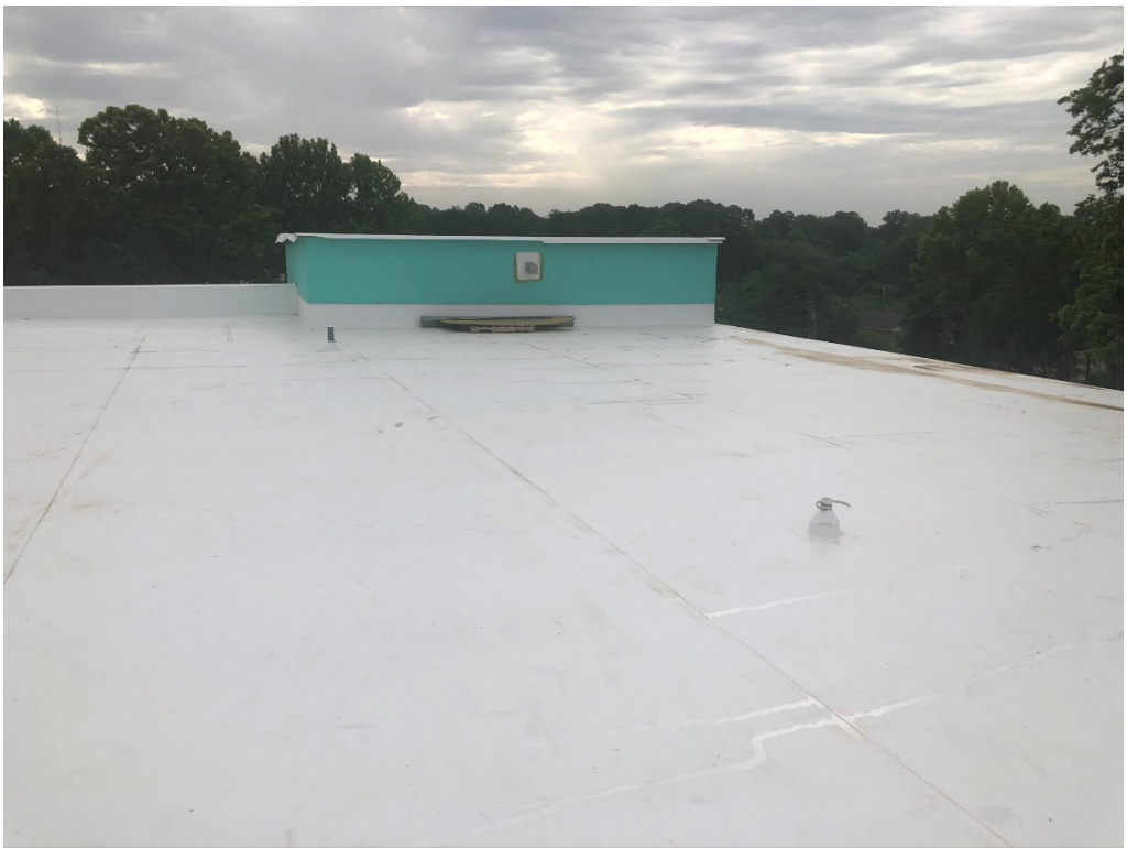
Figure 16 – East Wing Roof membrane Installed
