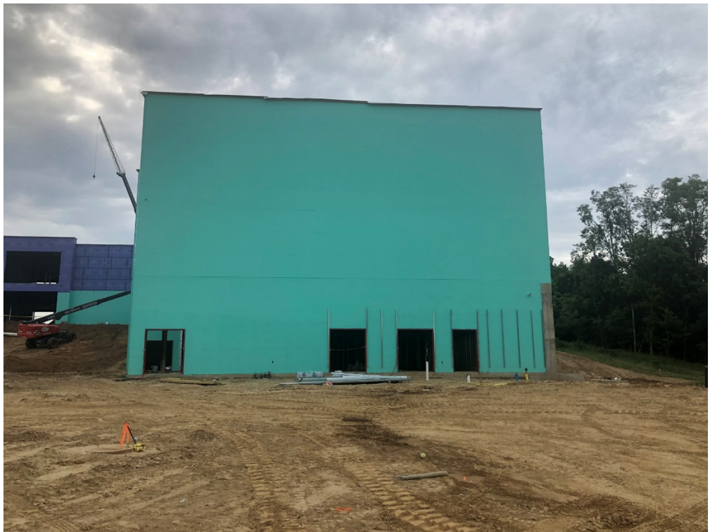
Figure 10 – West Façade at West Wing
