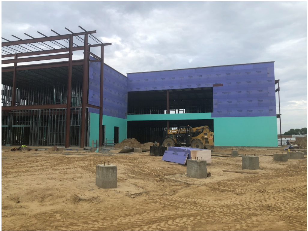
Figure 3 – North Structure Section, East Façade
