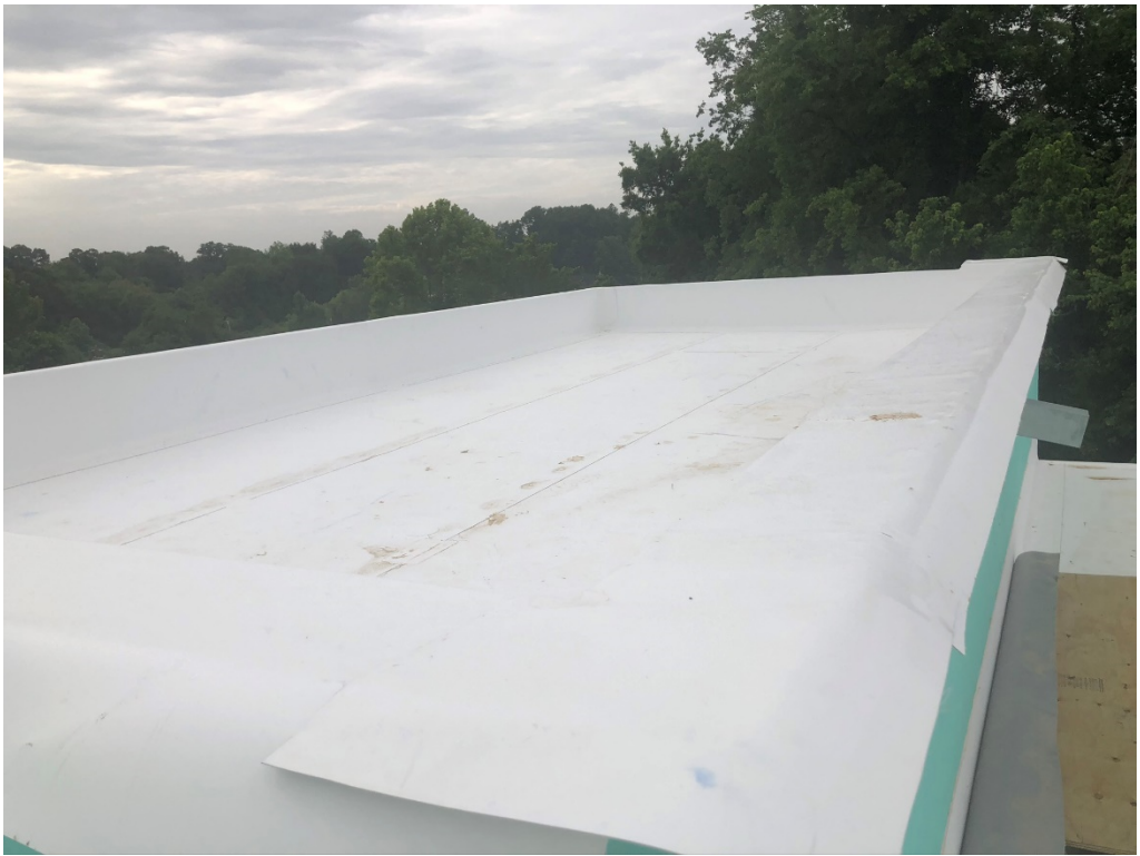
Figure 25 – Stair Well Roof Section
