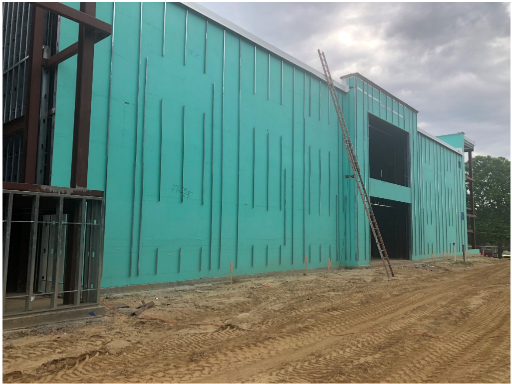
Figure 13 – South Façade at East Wing
