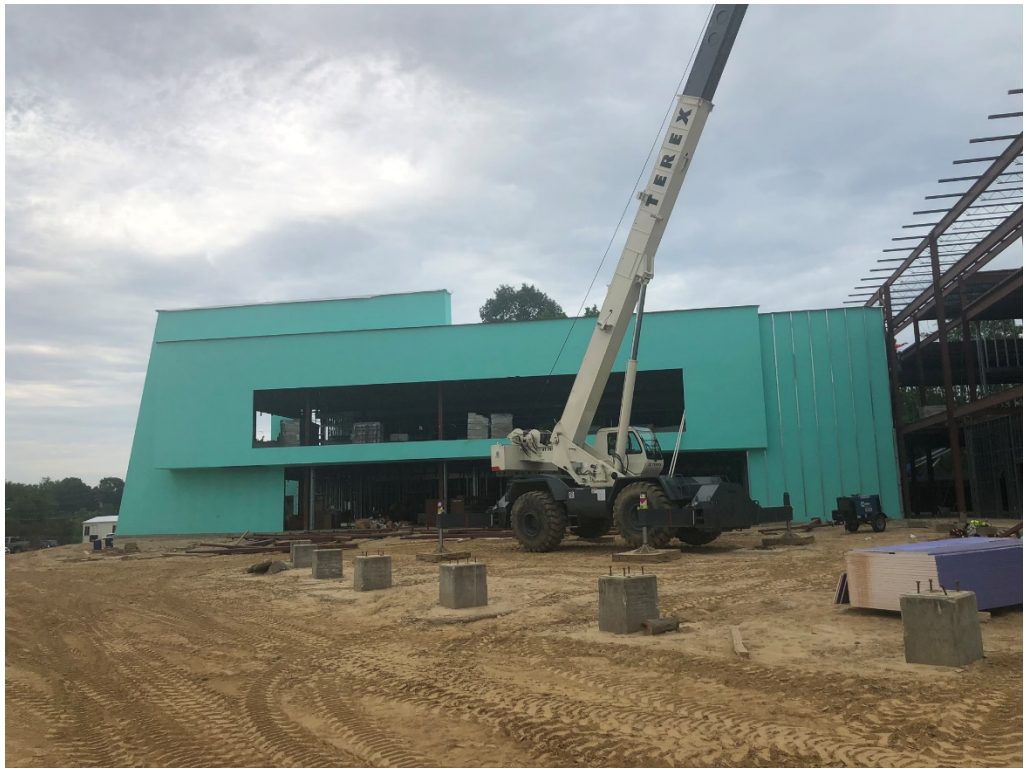
Figure 5 – North Façade, East Wing
