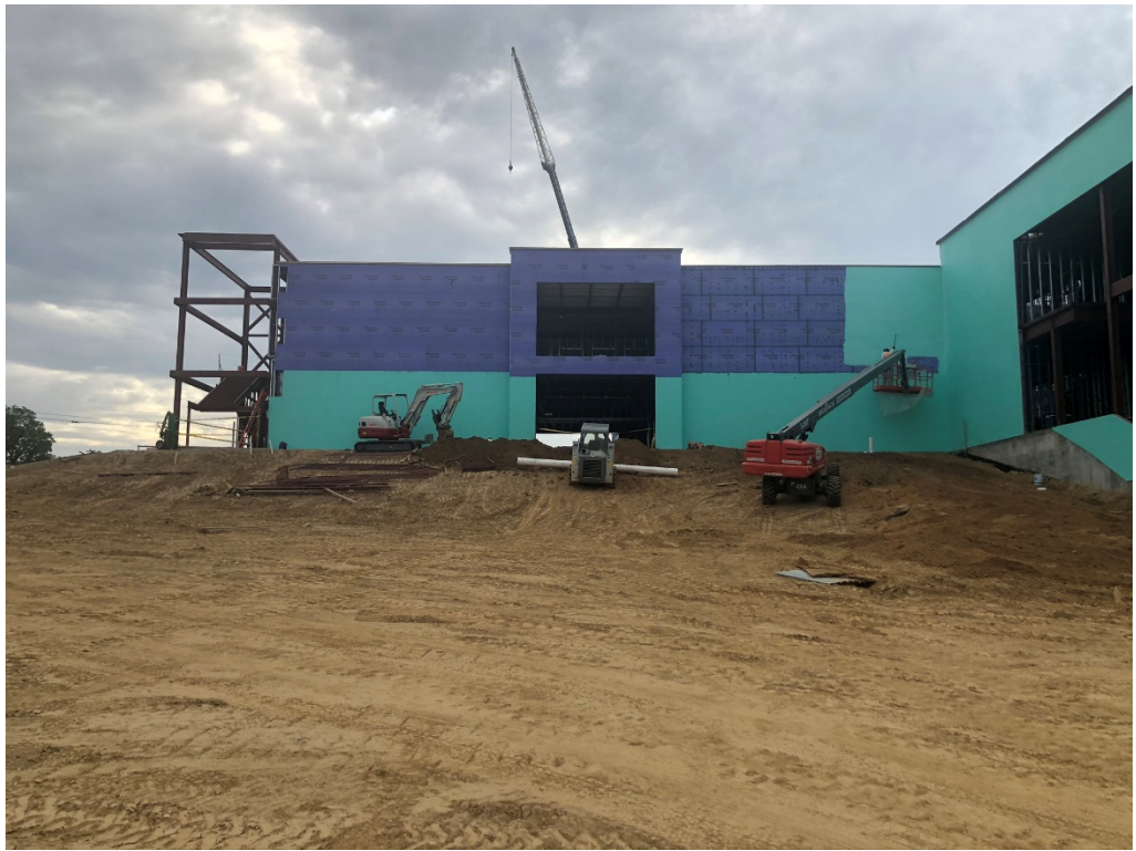
Figure 9 – West Façade at North Wing
