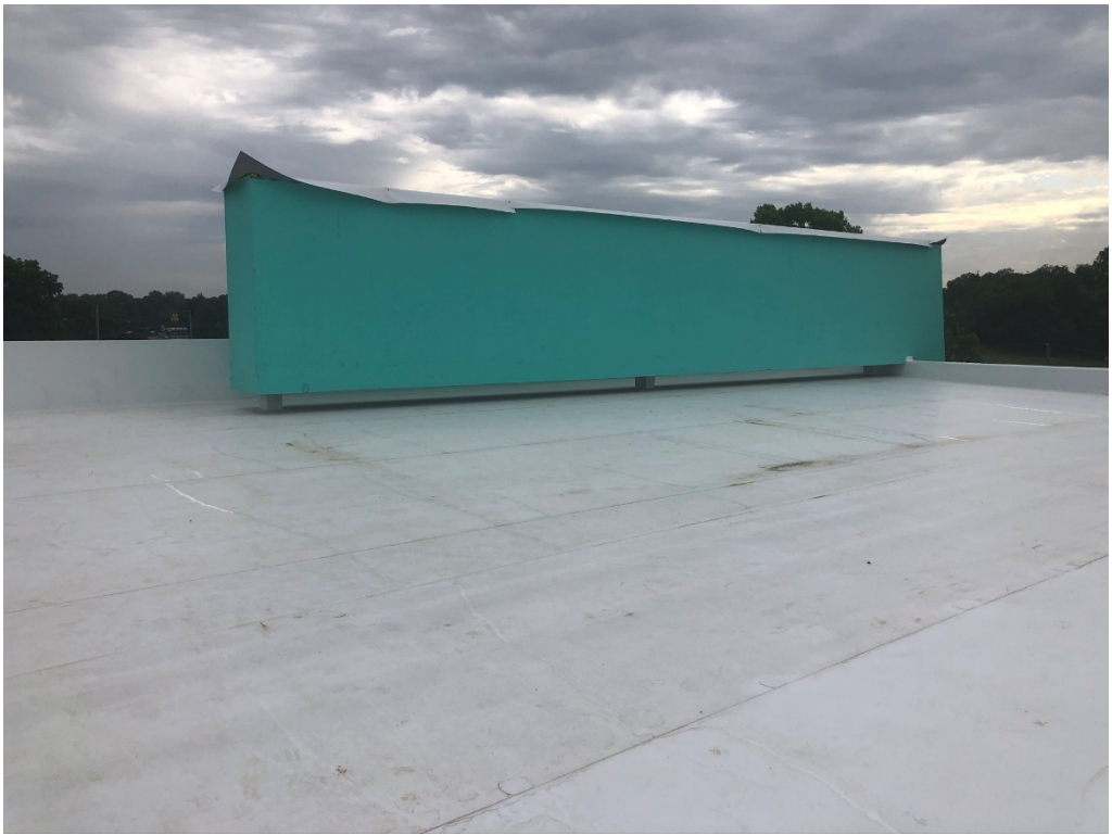
Figure 15 – East Wing Roof membrane Installed
