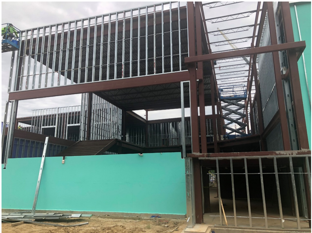
Figure 14 –Framing Ongoing at Exterior Façade
