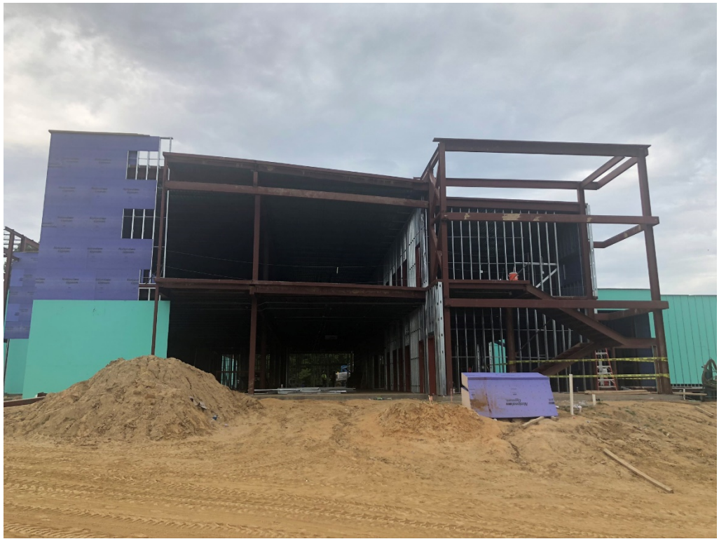
Figure 7 – North Façade at Center Section of Building
