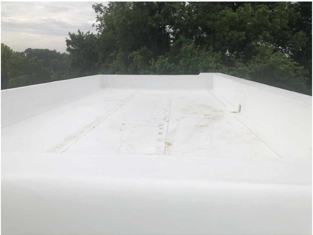
Figure 26 – Stair Well Roof Section
