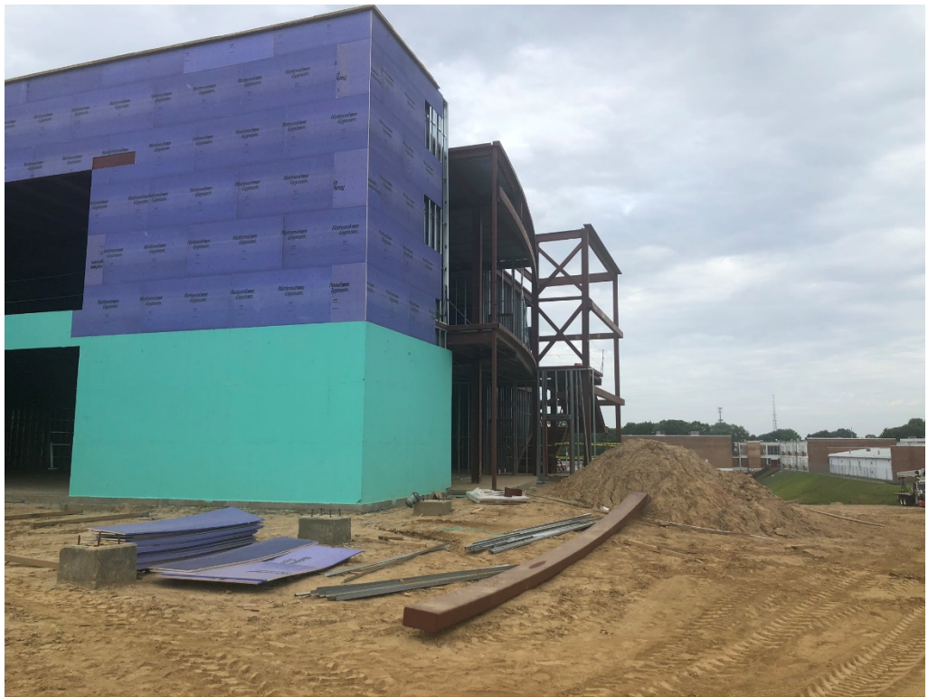
Figure 6 – North Section of Structure
