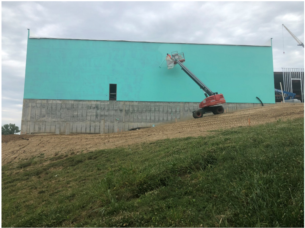
Figure 11 – South Façade at West Wing
