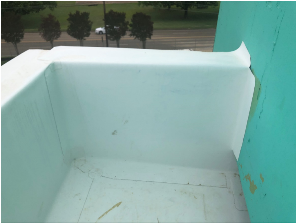
Figure 21 – Parapet Wall Detail to Sidewall Junction
