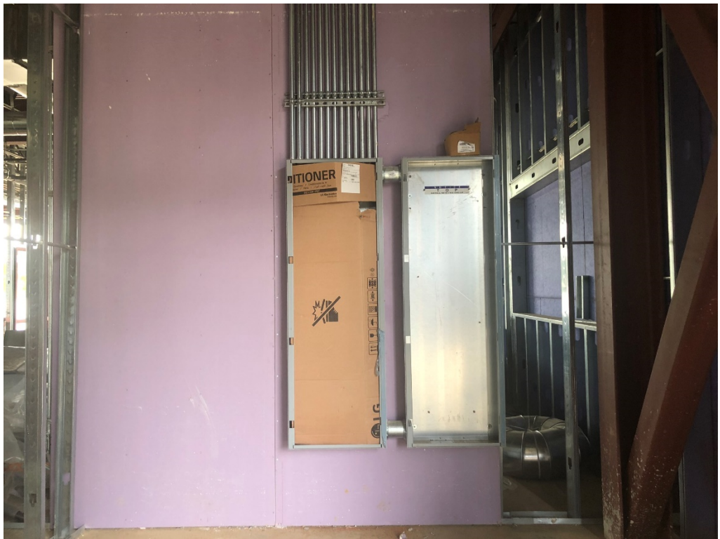
Figure 30 – Electrical Rough-IN is Ongoing
