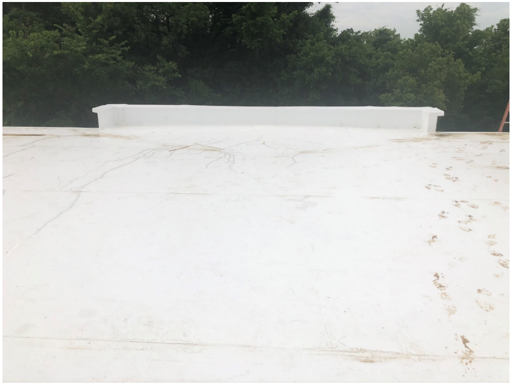
Figure 17 – East Wing Roof membrane Installed
