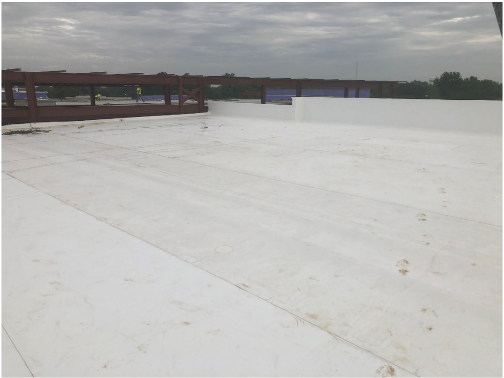
Figure 19 – East Wing Roof membrane Installed
