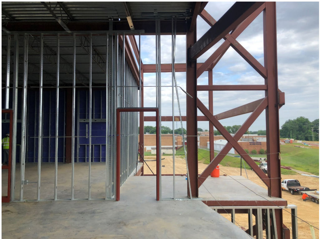
Figure 32 – North Metal Stairs Installed
