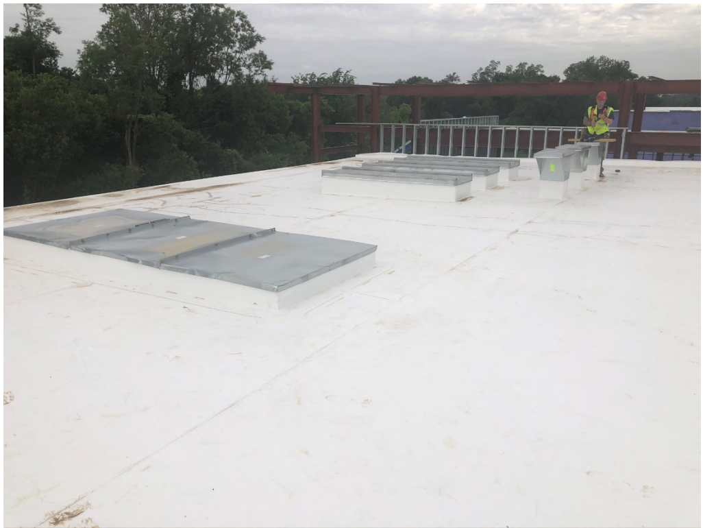
Figure 18 – East Wing Roof membrane and Curbs
