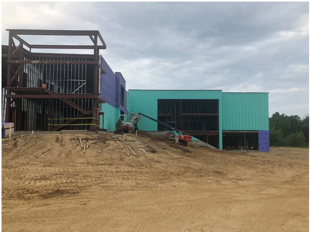
Figure 8 – North Façade at West Wing
