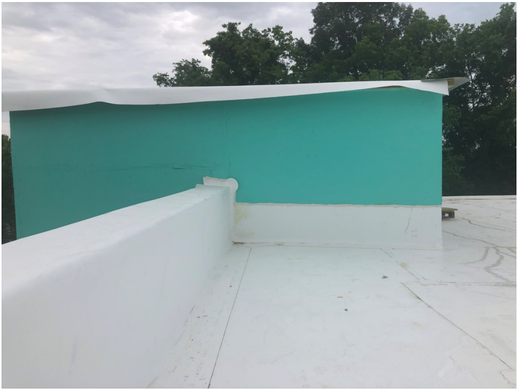
Figure 23 – Stair Well Roof Section
