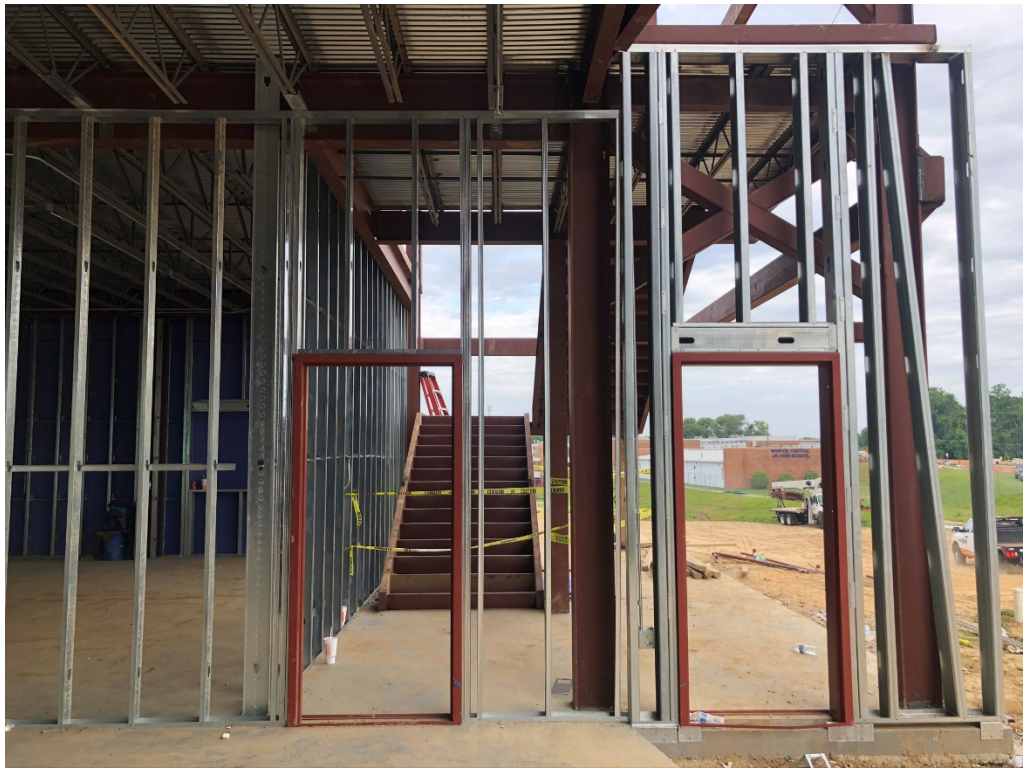
Figure 31 – North Metal Stairs Installed
