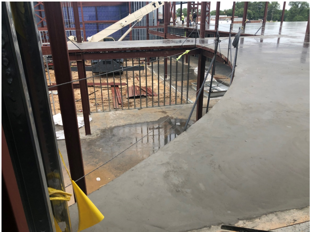
Figure 4 – Curved Concrete Edge in Public Gathering Space
