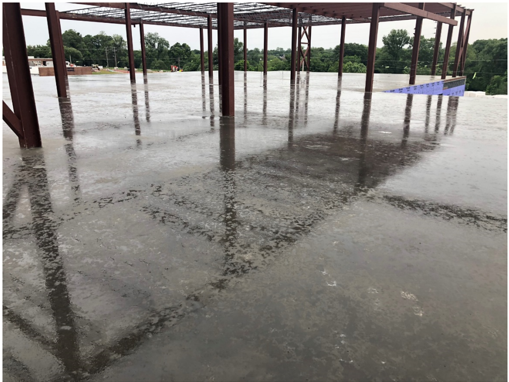
Figure 6 – Remesh Prep @ 2 nd Floor Slab
