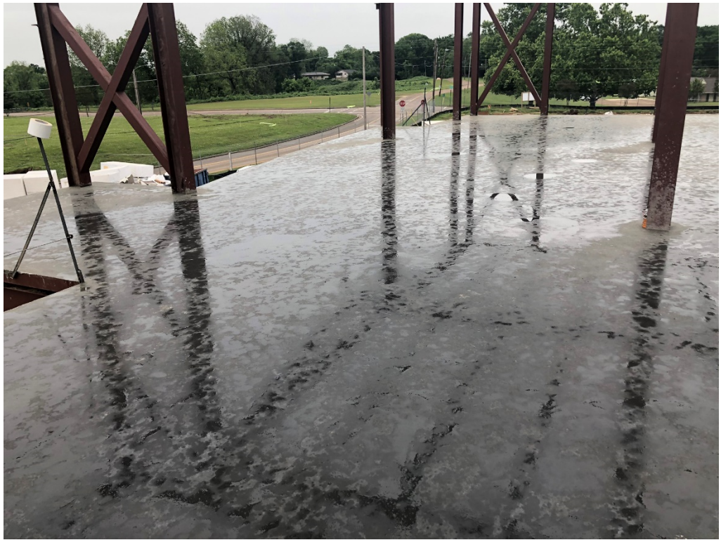
Figure 9 – Upper Slab Looking ENE
