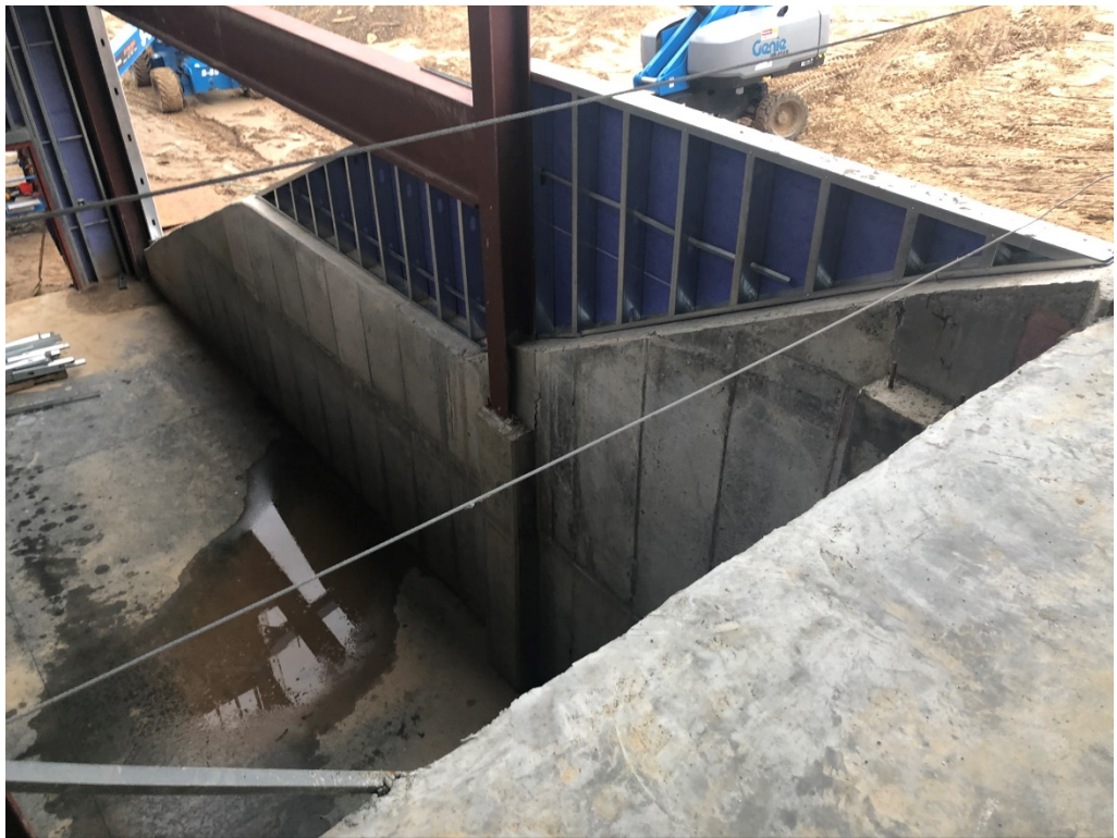
Figure 12 –Framed area Above Retaining Wall
