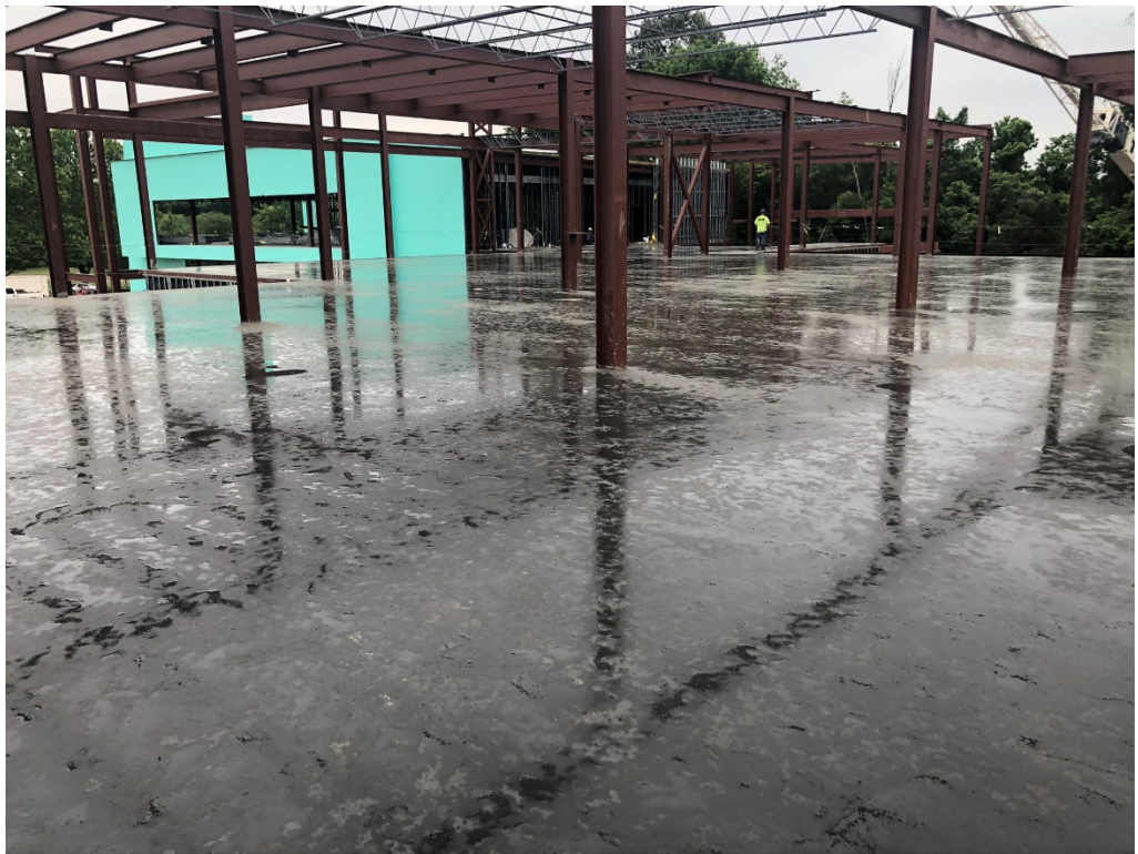
Figure 10 – Upper Slab Looking South
