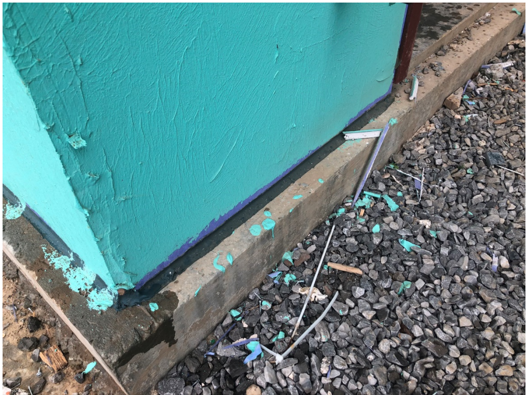
Figure 2 – Waterproofing Should be continuous to Corner
