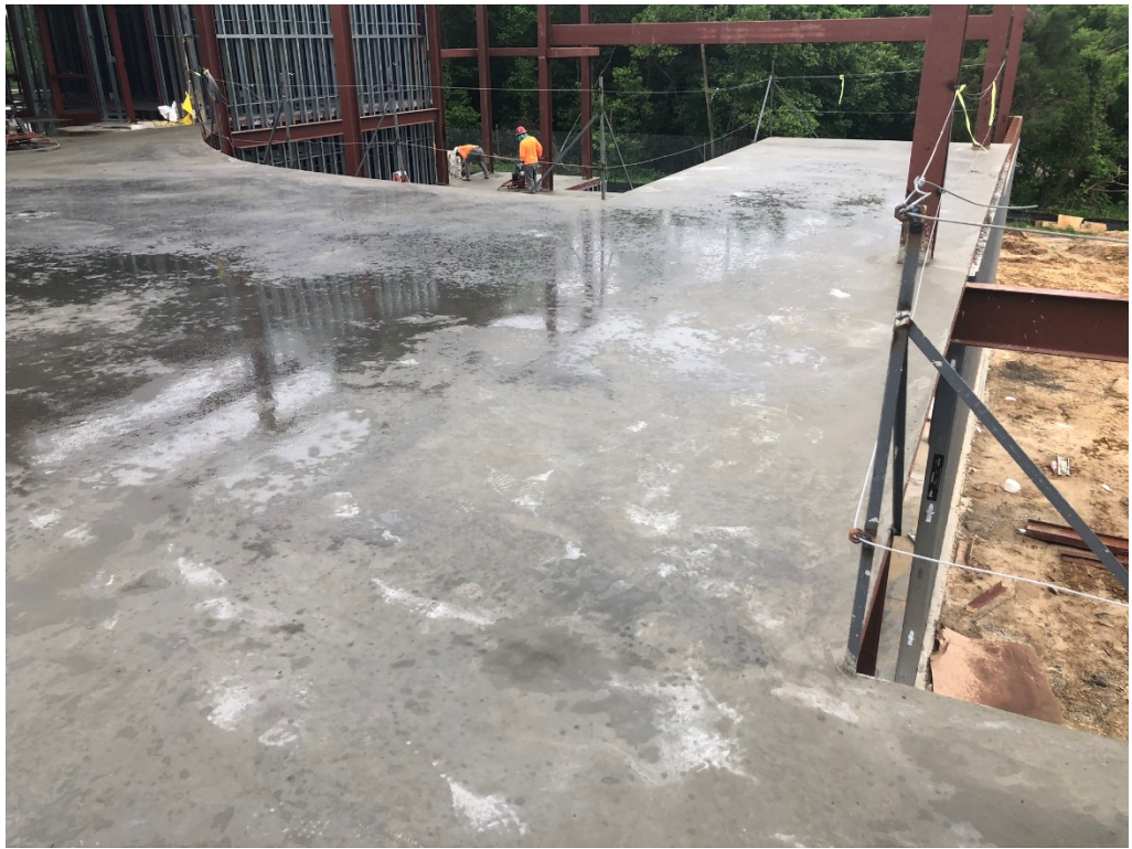
Figure 7 – Upper Slab Looking South
