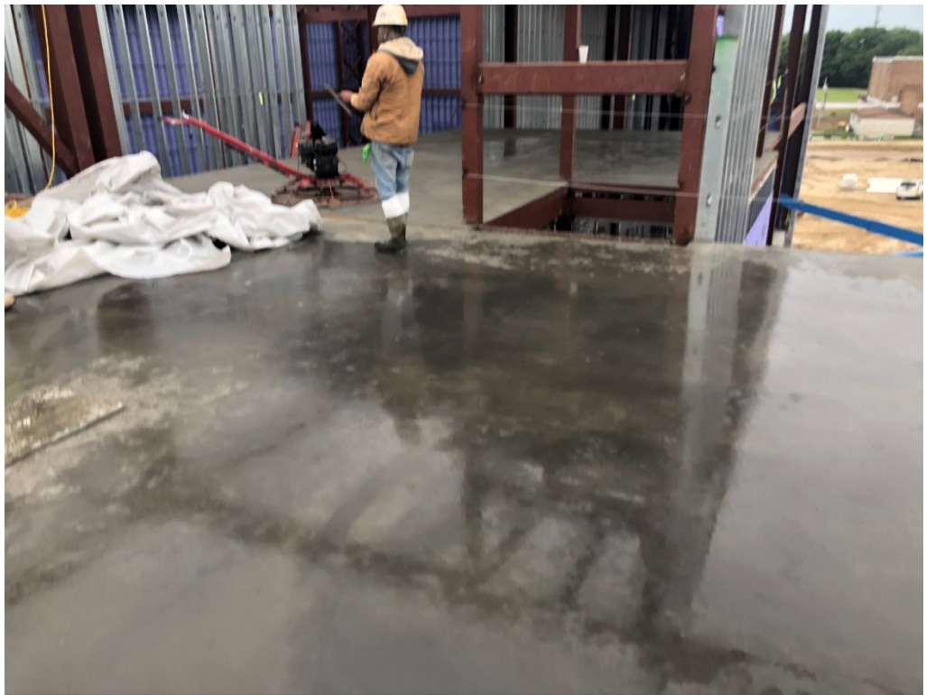
Figure 8 – Upper Slab Looking West
