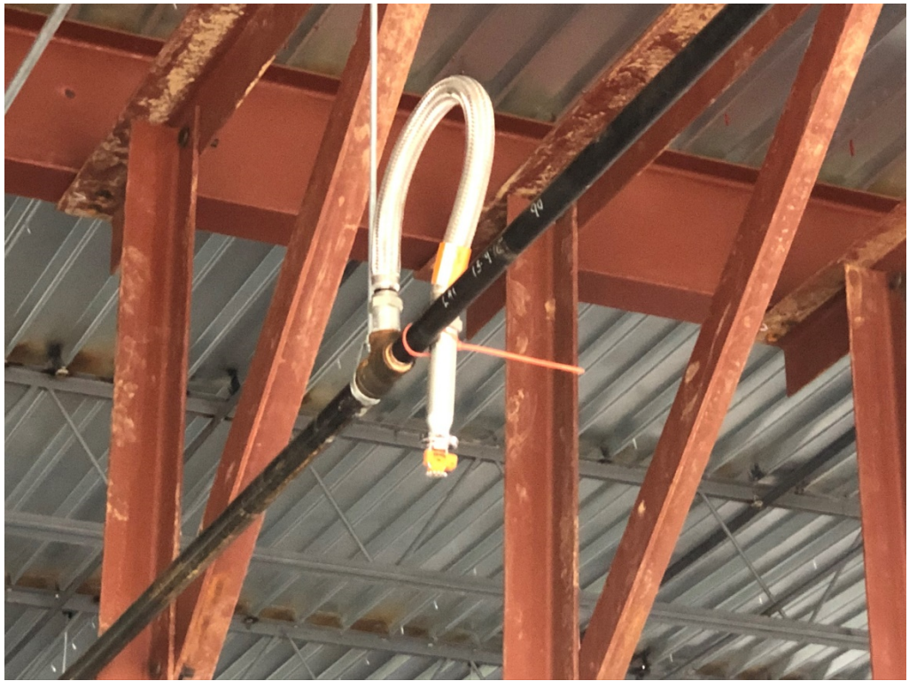
Figure 3 – Flex Drop for Sprinkler (typical and 90% complete in East structure)
