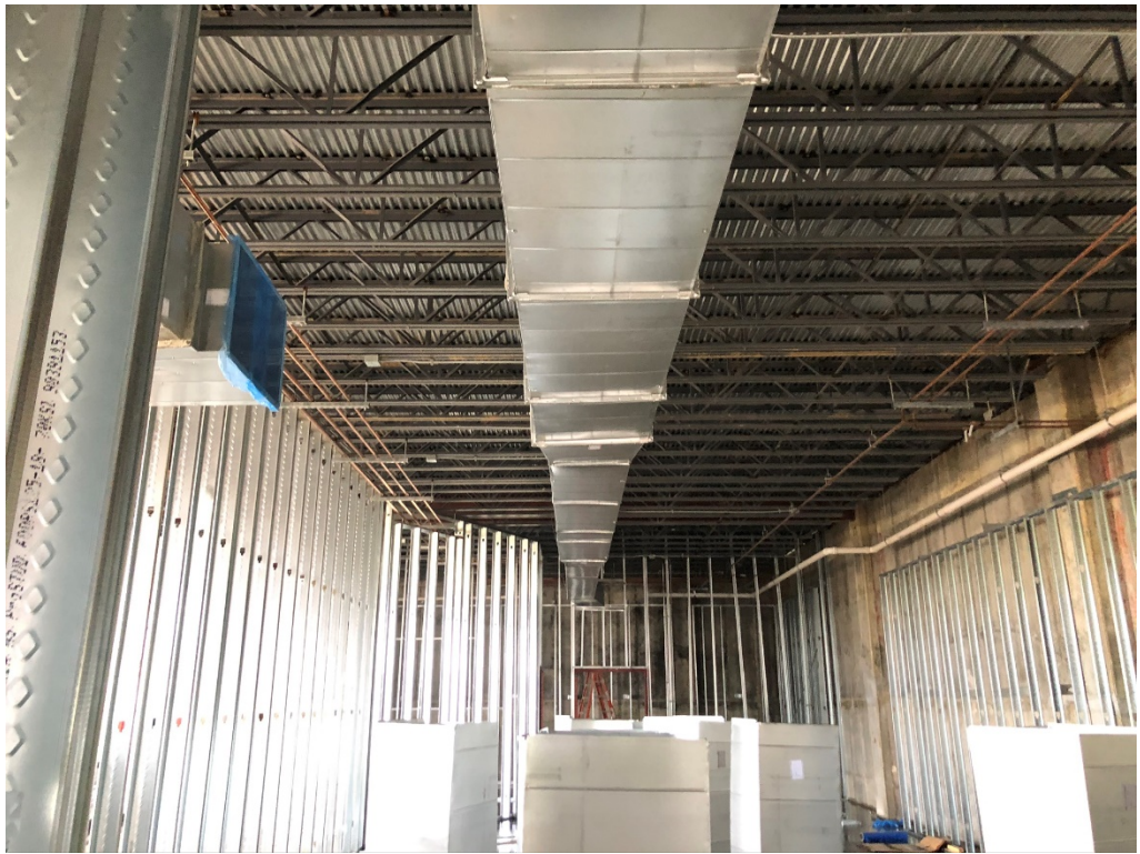
Figure 13 – Mech Rough in @ First Floor
