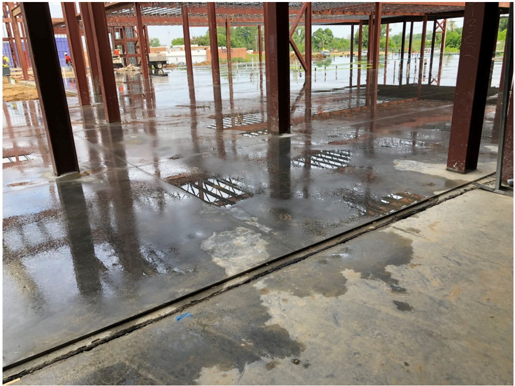
Figure 3 – Ponding Technique in use 4 days after pour
