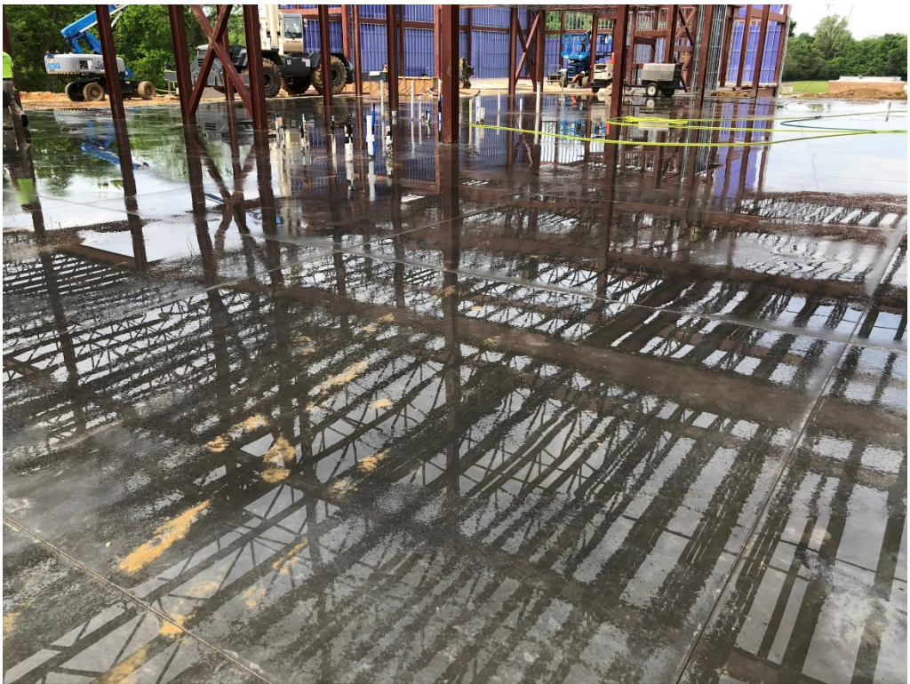
Figure 6 – Ponding Technique in use 4 days after pour
