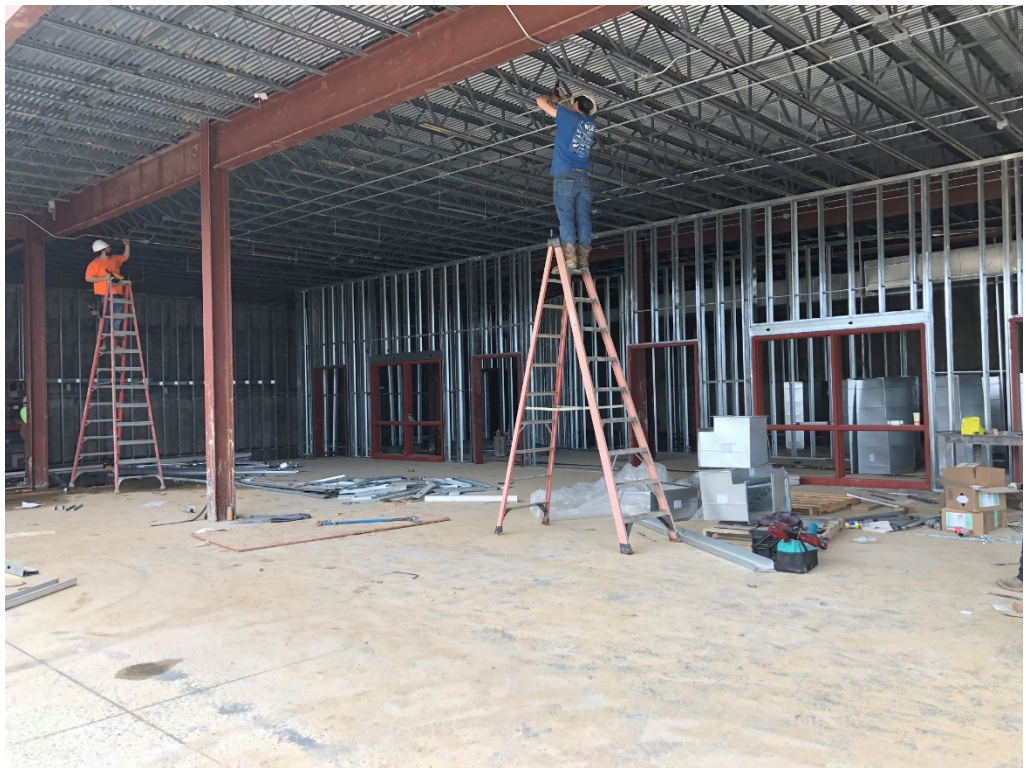
Figure 12 – Continued Rough-in Progress @ first floor cafeteria
