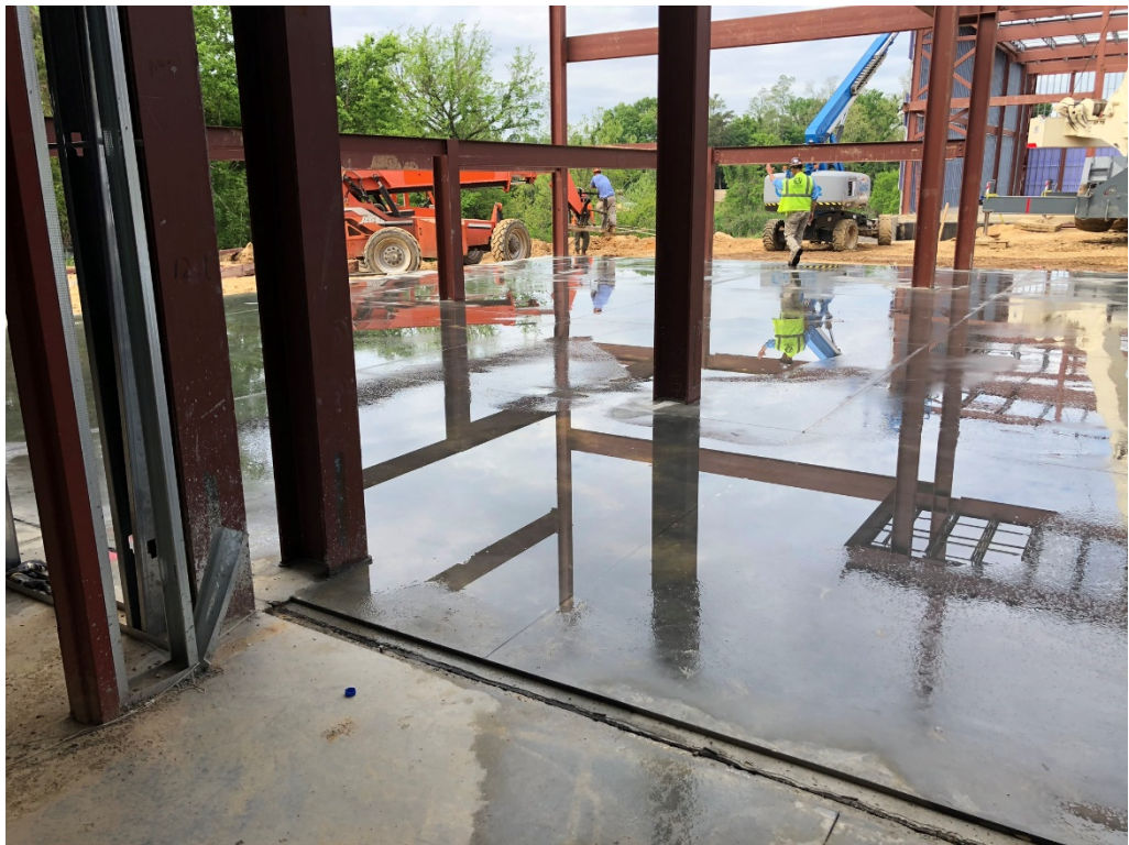
Figure 4 – Ponding Technique in use 4 days after pour
