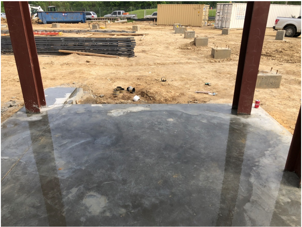
Figure 5 – North Section of New Slab
