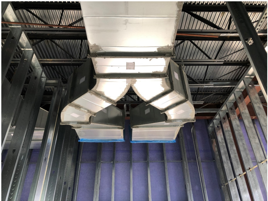
Figure 14 – Mech Rough in @ First Floor
