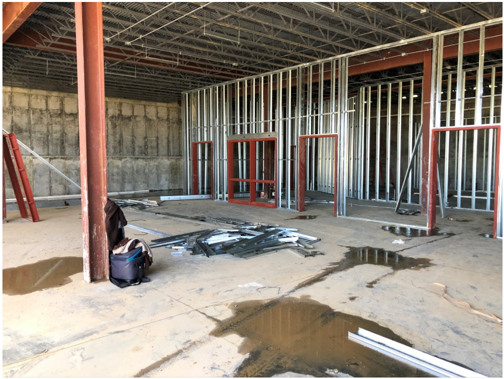
Figure 13 – Framing @ Cafeteria / Lower Level
