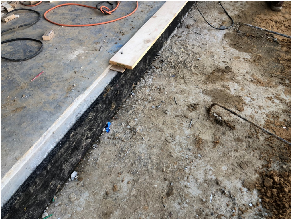
Figure 8 – Expansion Joint Installed
