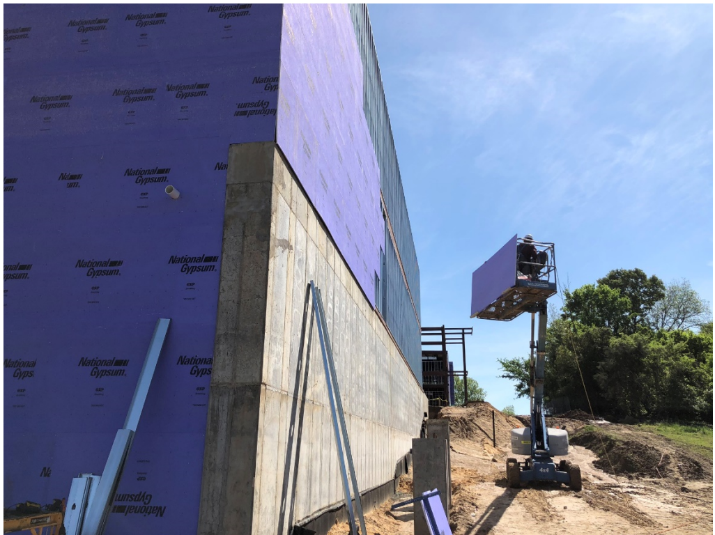
Figure 16 – Concrete and Gypsum Connection
