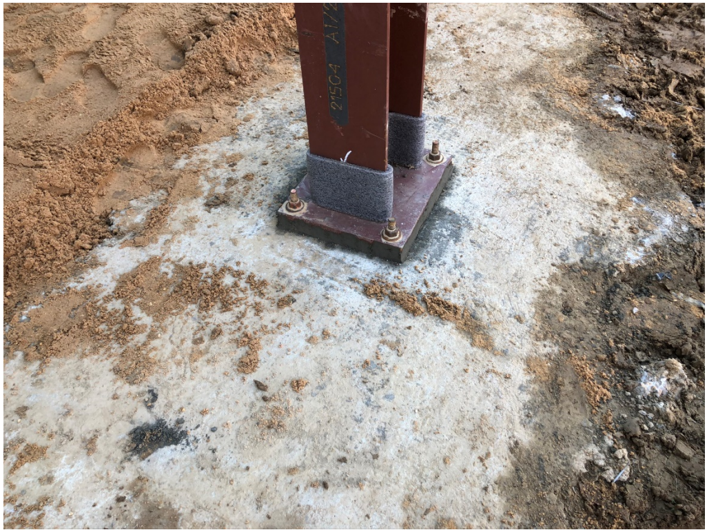
Figure 9 – Column Prepared for Concrete Pour
