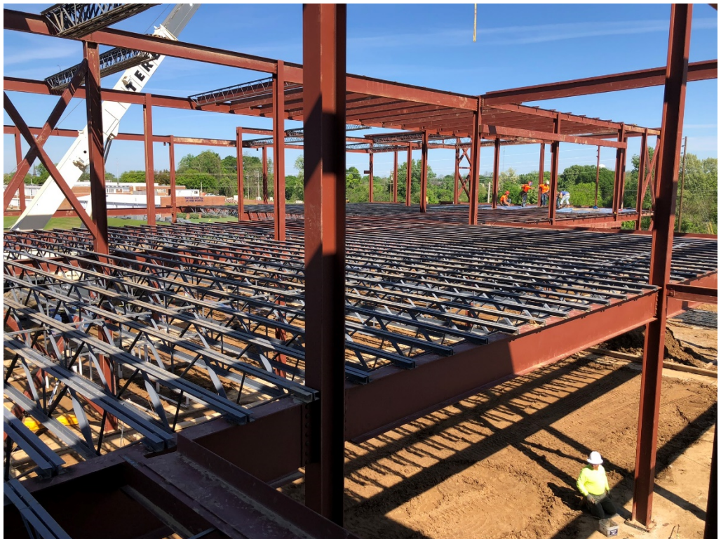
Figure 6 – Floor Joists Set
