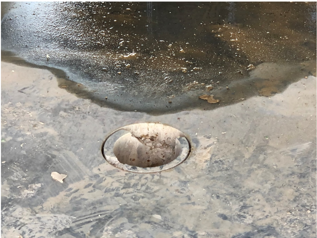
Figure 4 – Floor Drain at Upper Level 218
