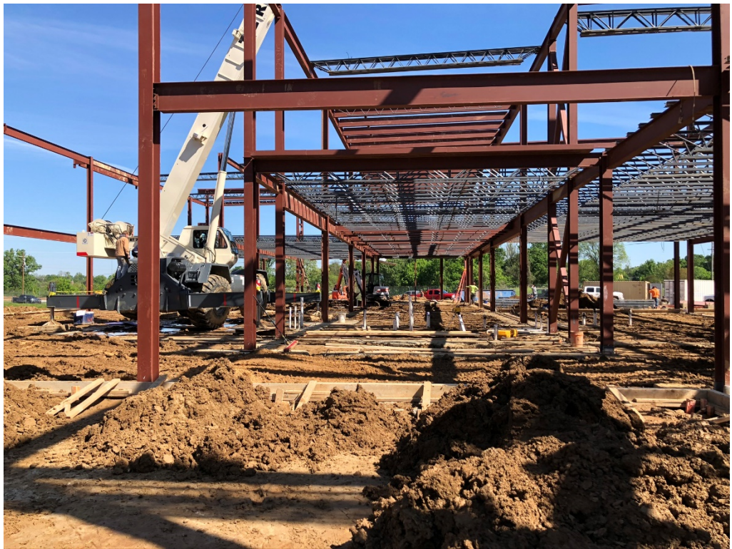
Figure 10 – Ground and Formwork Prep to Pour on Friday
