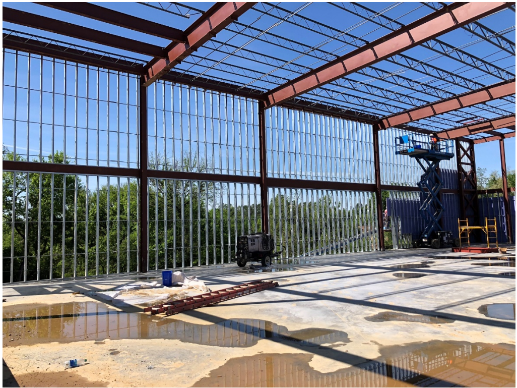
Figure 11 – Gym Area Framing
