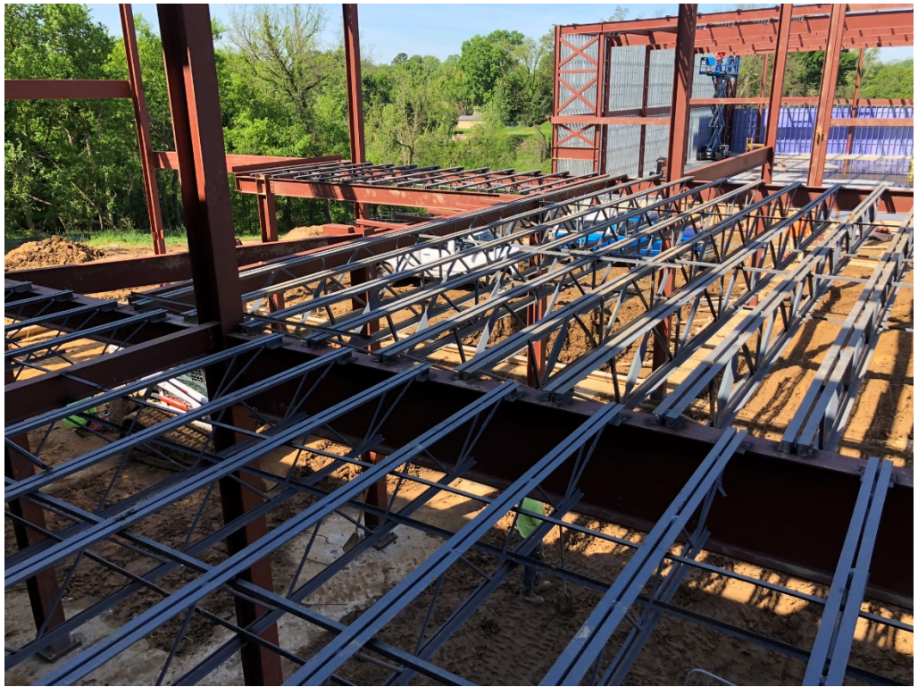
Figure 5 – Floor Joists Set
