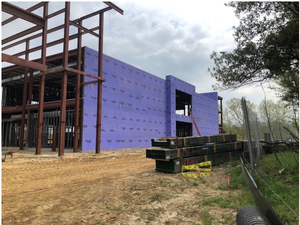
Figure 10 – South Center of Site Looking NE
