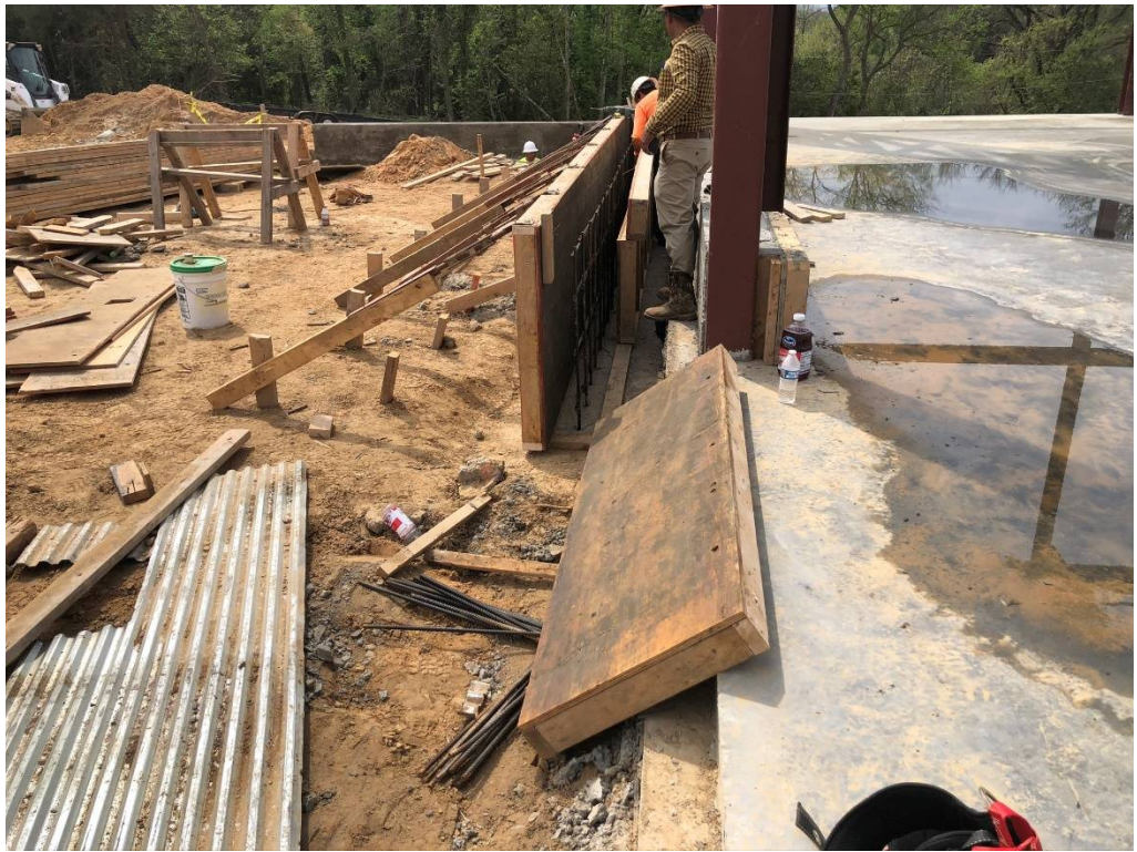
Figure 19 – Formwork at East Side Upper Floor West Section of Building
