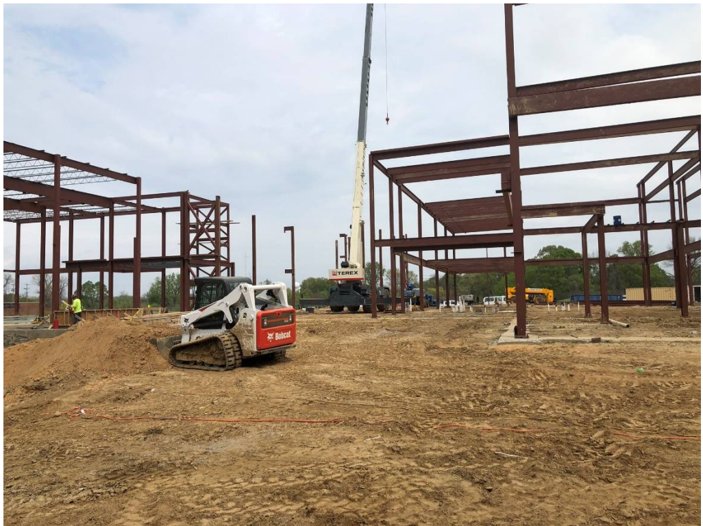
Figure 8 – South Center of Site Looking N
