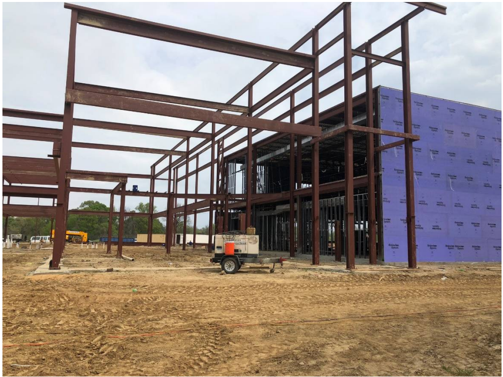
Figure 9 – South Center of Site Looking N
