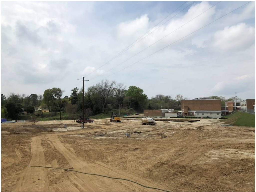
Figure 23 – North Central Entrance Looking WSW
