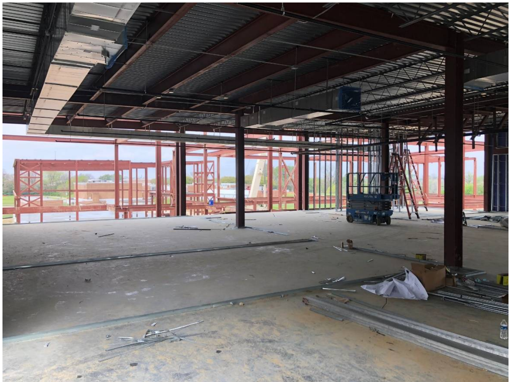
Figure 6 – East Section of Building Upper Floor Light Gauge Framing Laid Out
