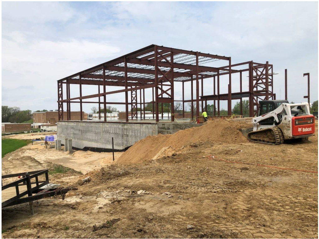
Figure 7 – South Center of Site Looking NW
