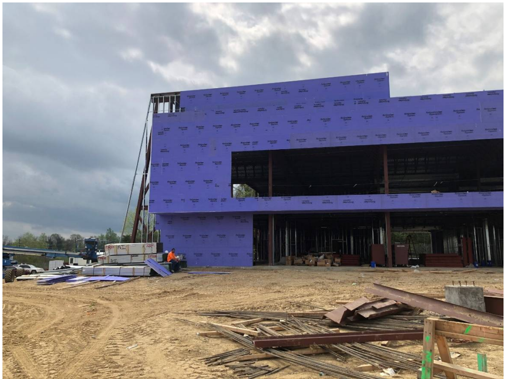
Figure 26 – North East Section of Site Looking S at North Elevation
