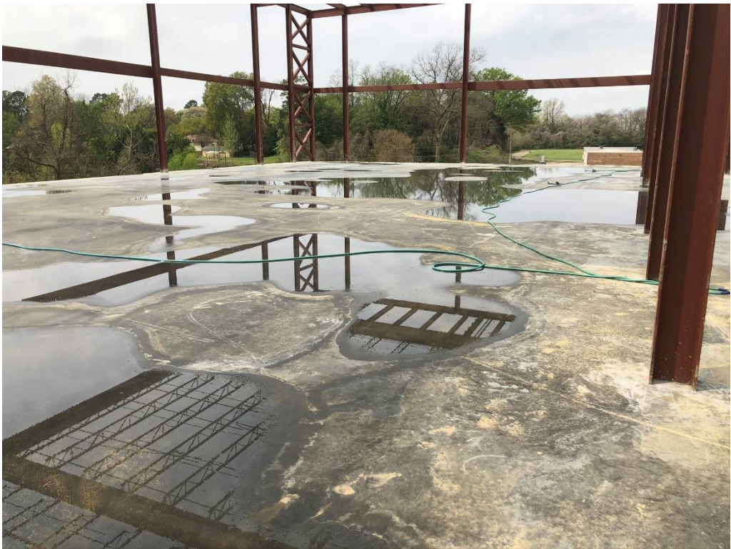
Figure 12 – West Upper Floor Slab
