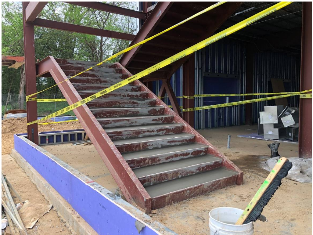
Figure 2 – Concrete Work at Pan Stairs
