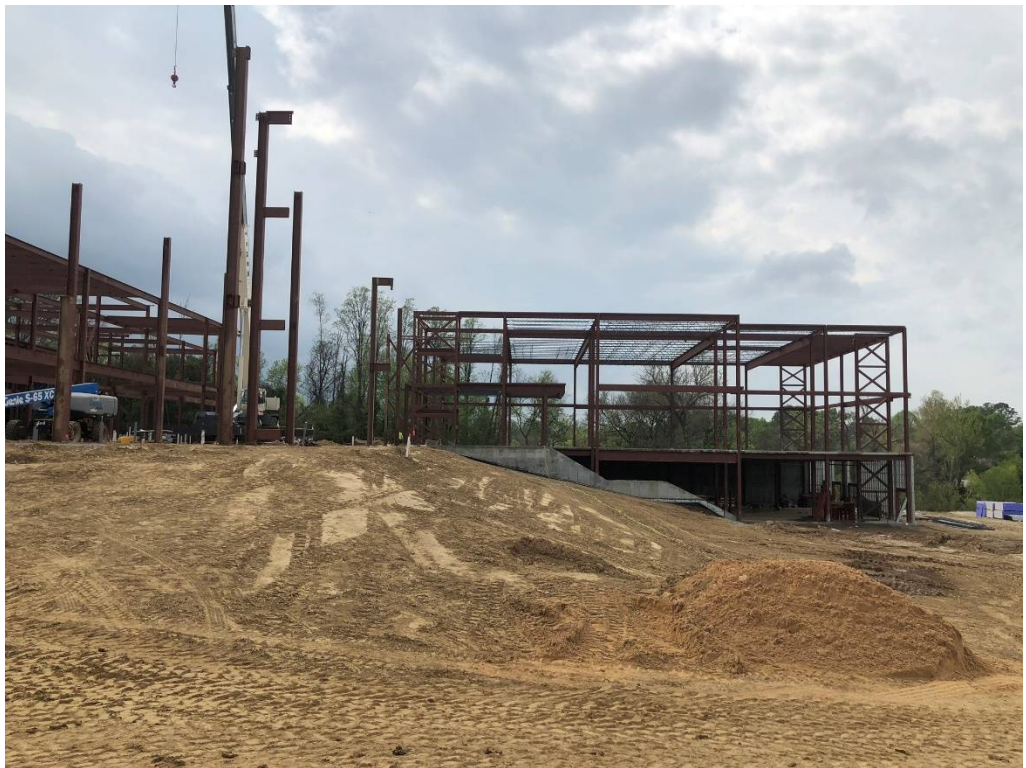
Figure 22 – North Central Entrance Looking S
