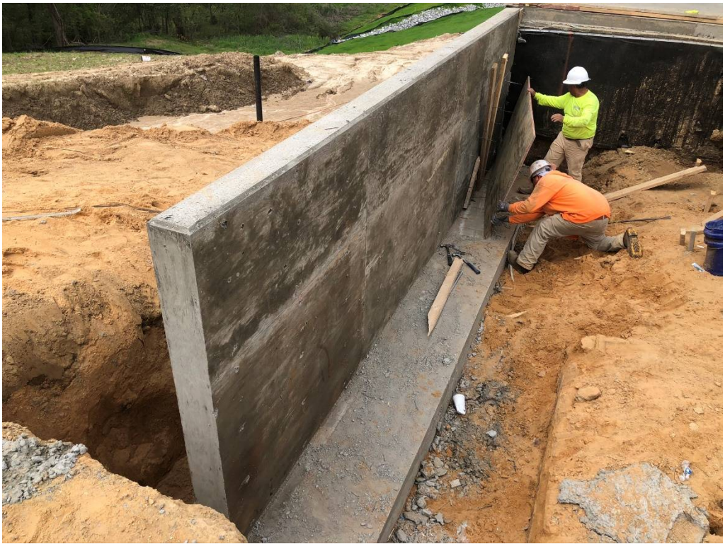
Figure 11 – Footing Complete at South Center of Building
