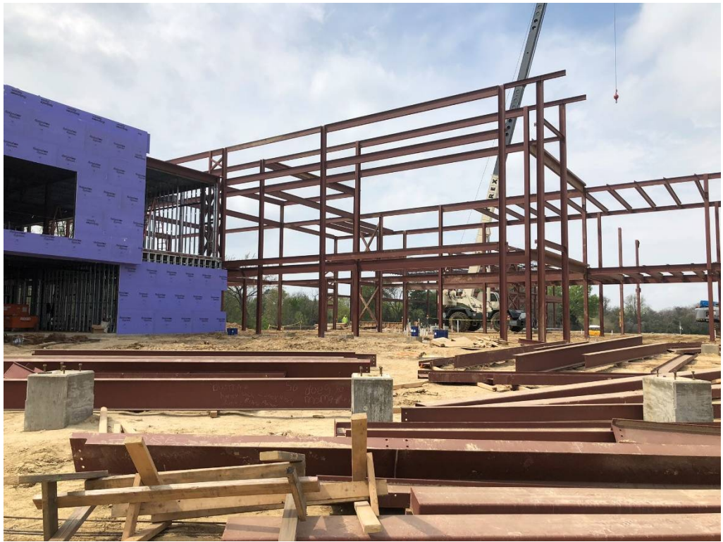
Figure 25 – North East Section of Site Looking SW
