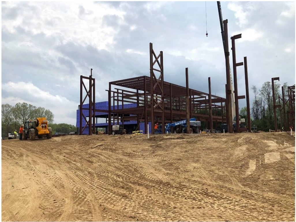
Figure 21 – North Central Entrance Looking ESE
