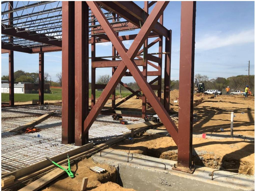
Figure 18 – Double Column Installed (Concrete Pour in West Structure can Commence)
