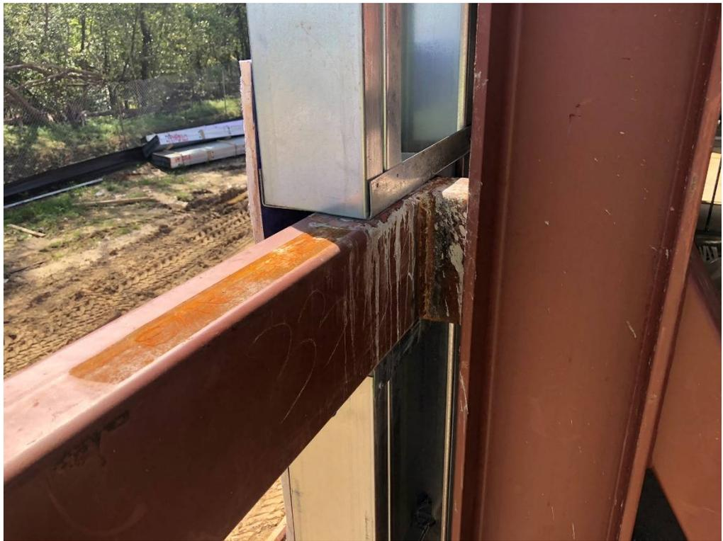
Figure 10 – Steel Header Light Gauge Framing Detail
