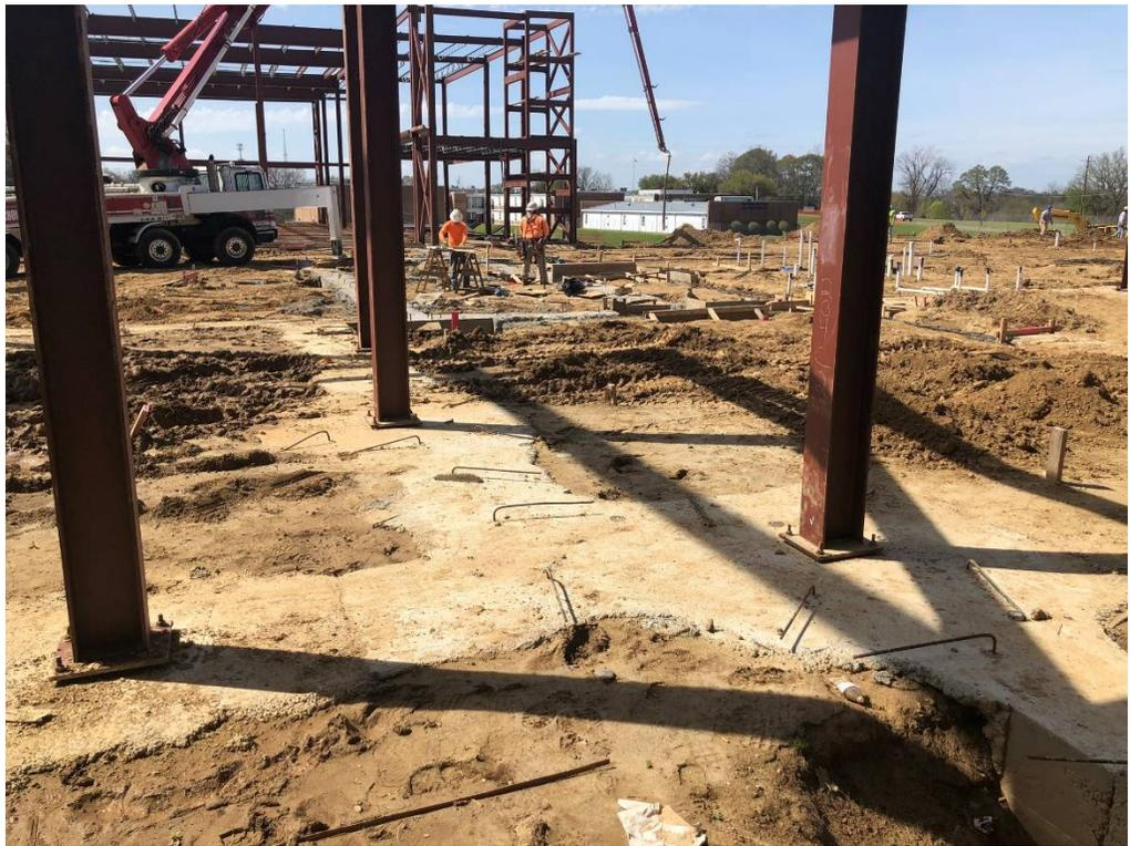
Figure 16 – Central Structure Footings (Concrete Pour On-Going)
