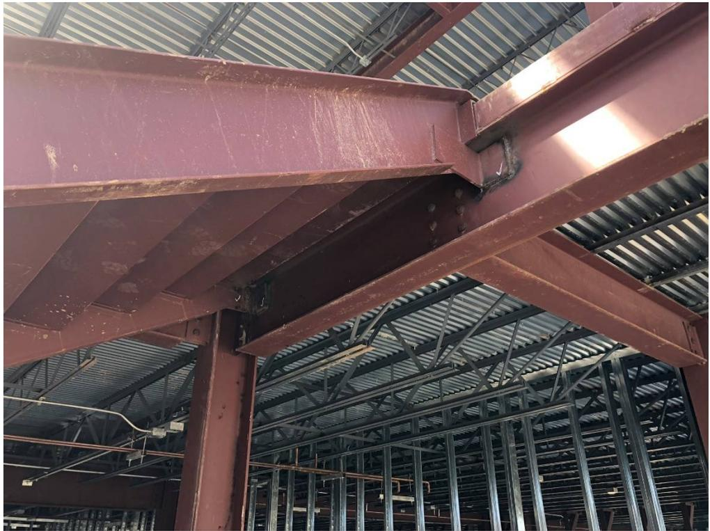
Figure 11 – SE Stair Connection to Second Floor
