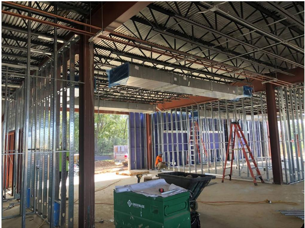
Figure 14 – Versatile Teaching Space Nook (Ducting Installation Begun)
