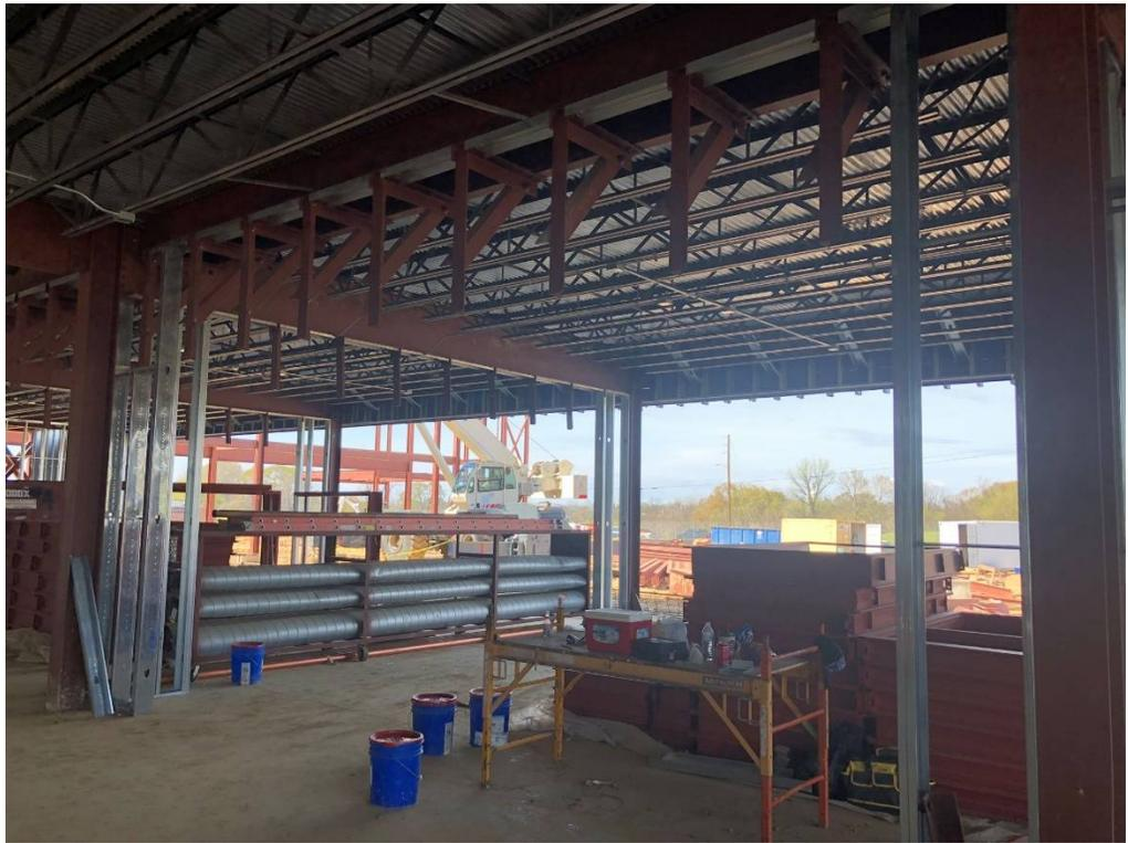
Figure 13 – Framing for Open Class Spaces
