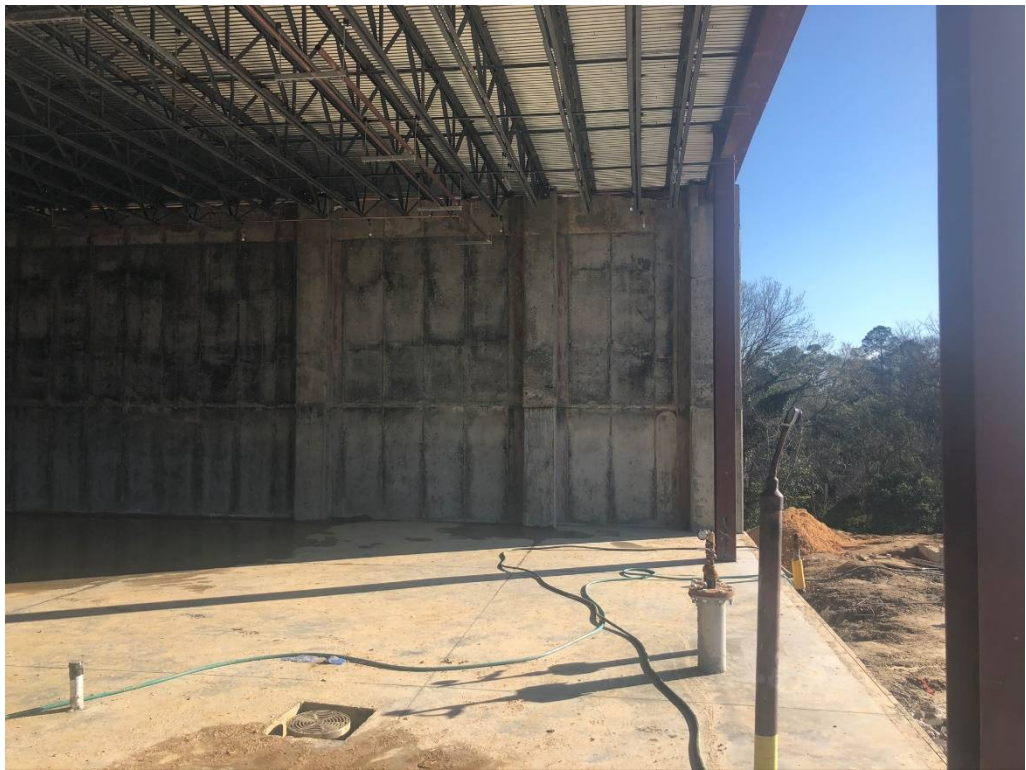
Figure 16 – West End of Lower Building Looking @ South West Corner
