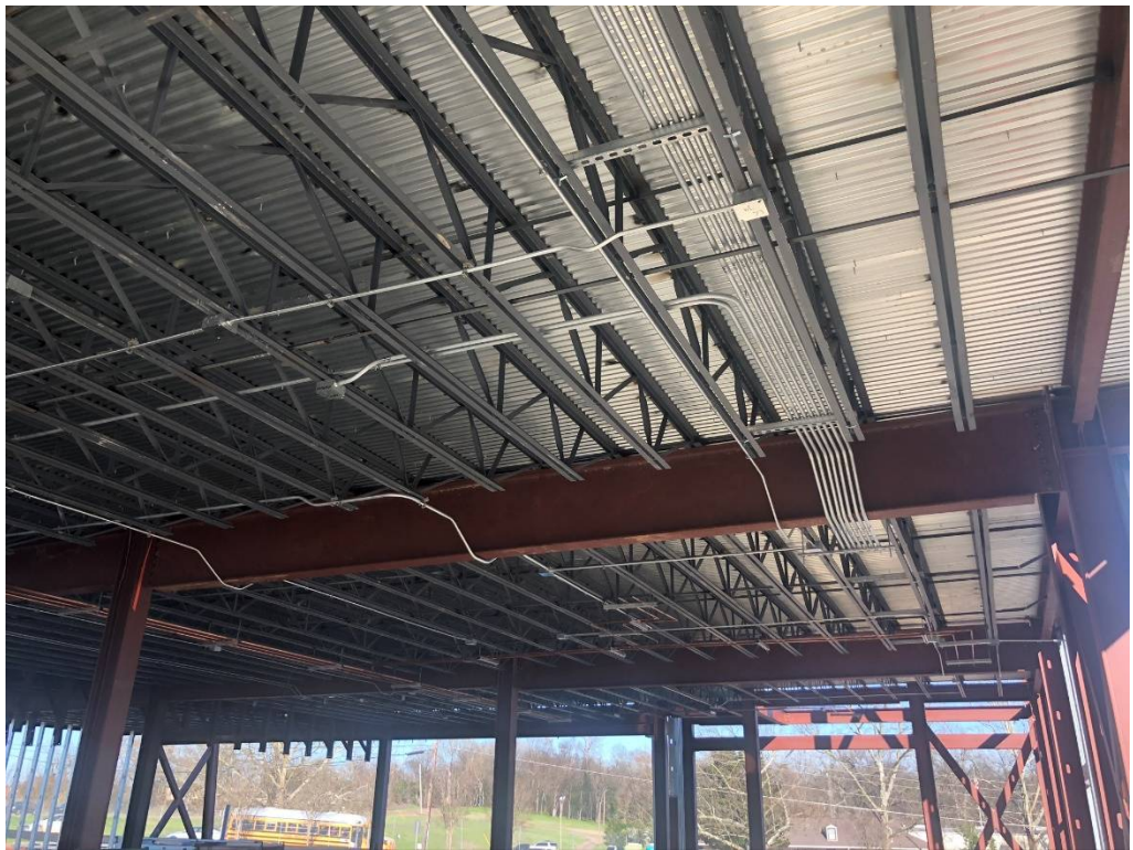
Figure 6 – Electrical & Plumbing Rough-in Ongoing in East Structure
