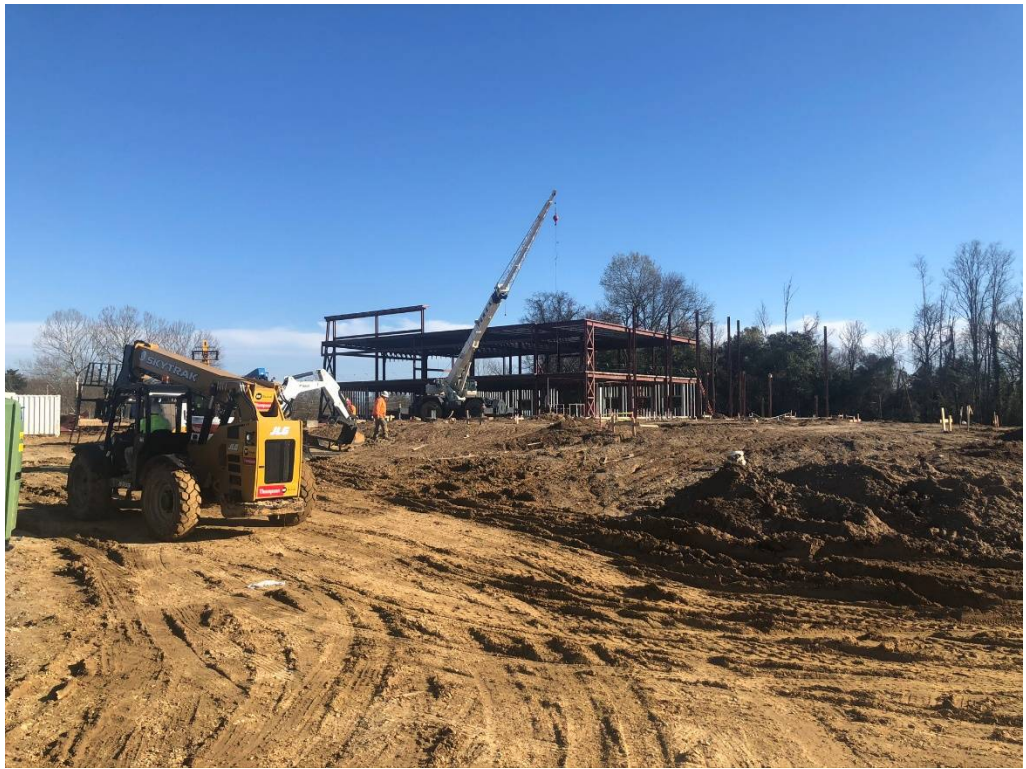
Figure 11 – North Entry Looking ESE
