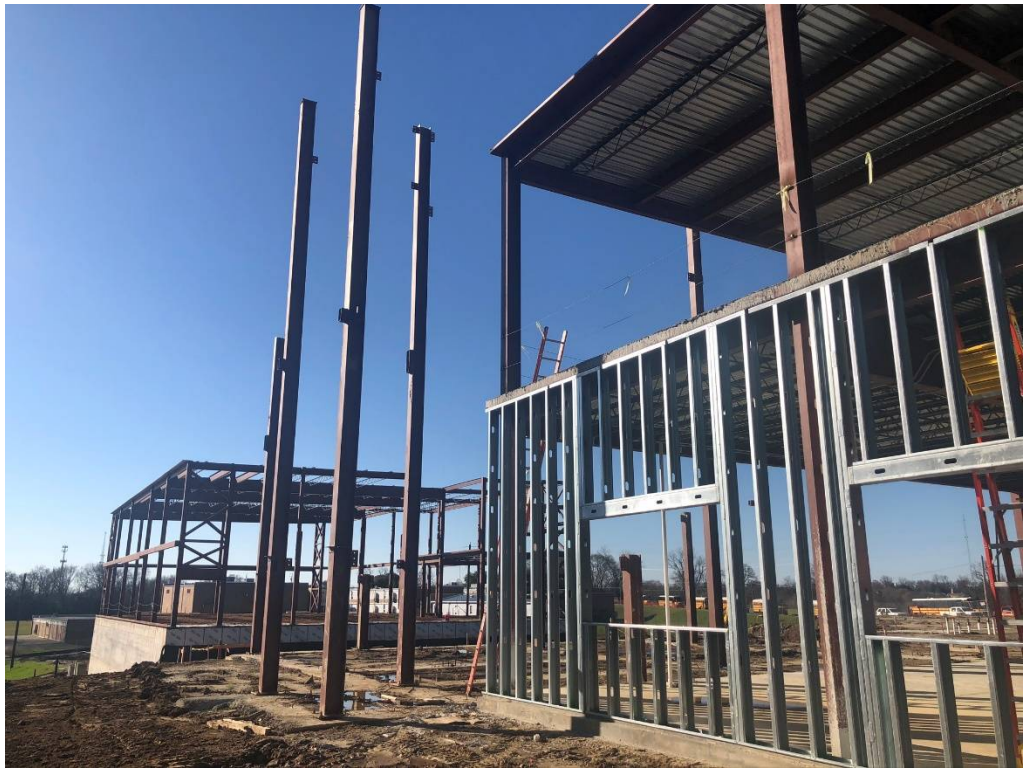
Figure 5 – New Steel at Connection Between Previously Erected Steel
