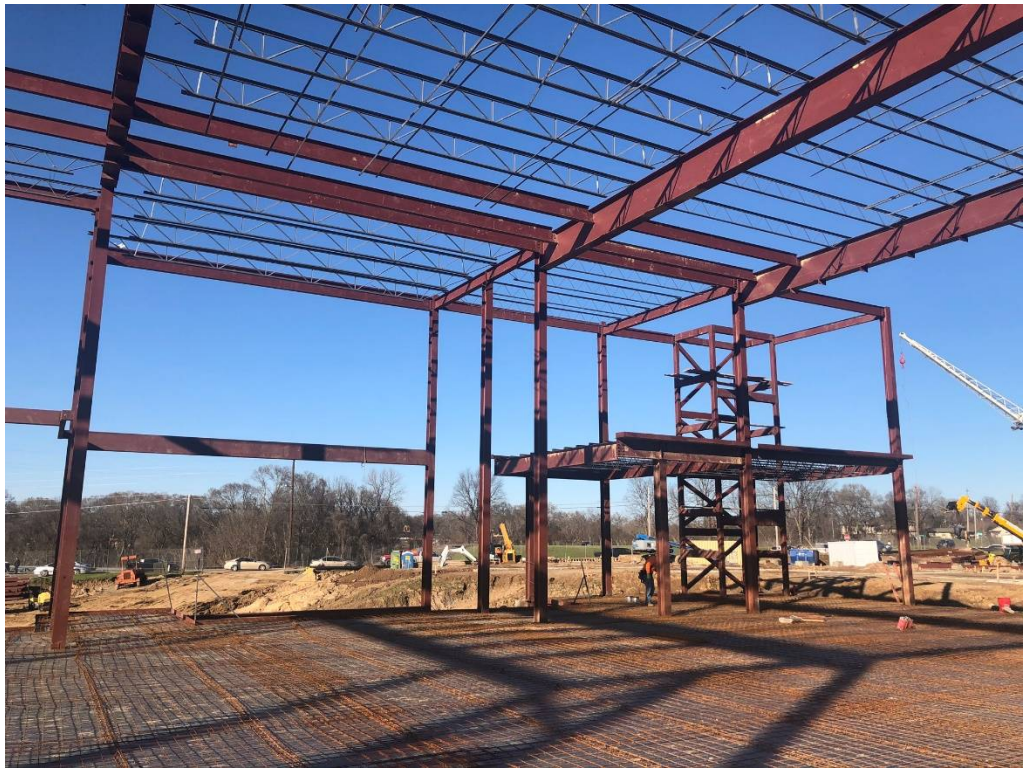
Figure 21 – South side of West Structure Looking North
