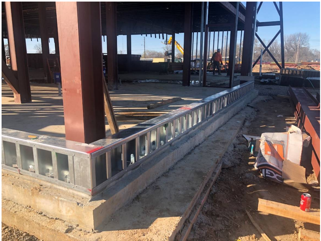
Figure 2 – Light Gauge Framing Started
