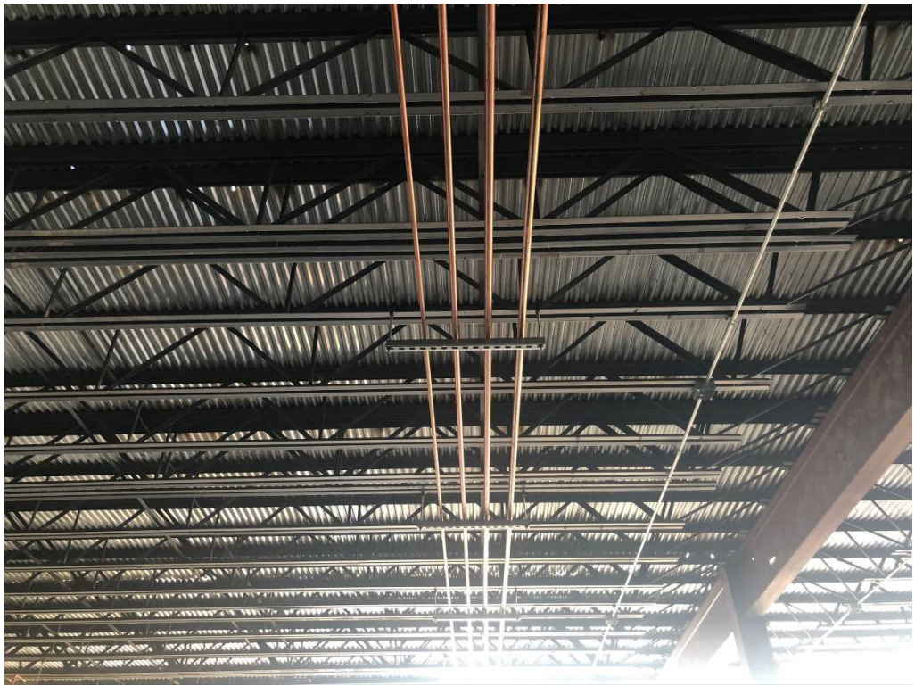
Figure 15 – Plumbing Rough-In Ongoing in West Structure
