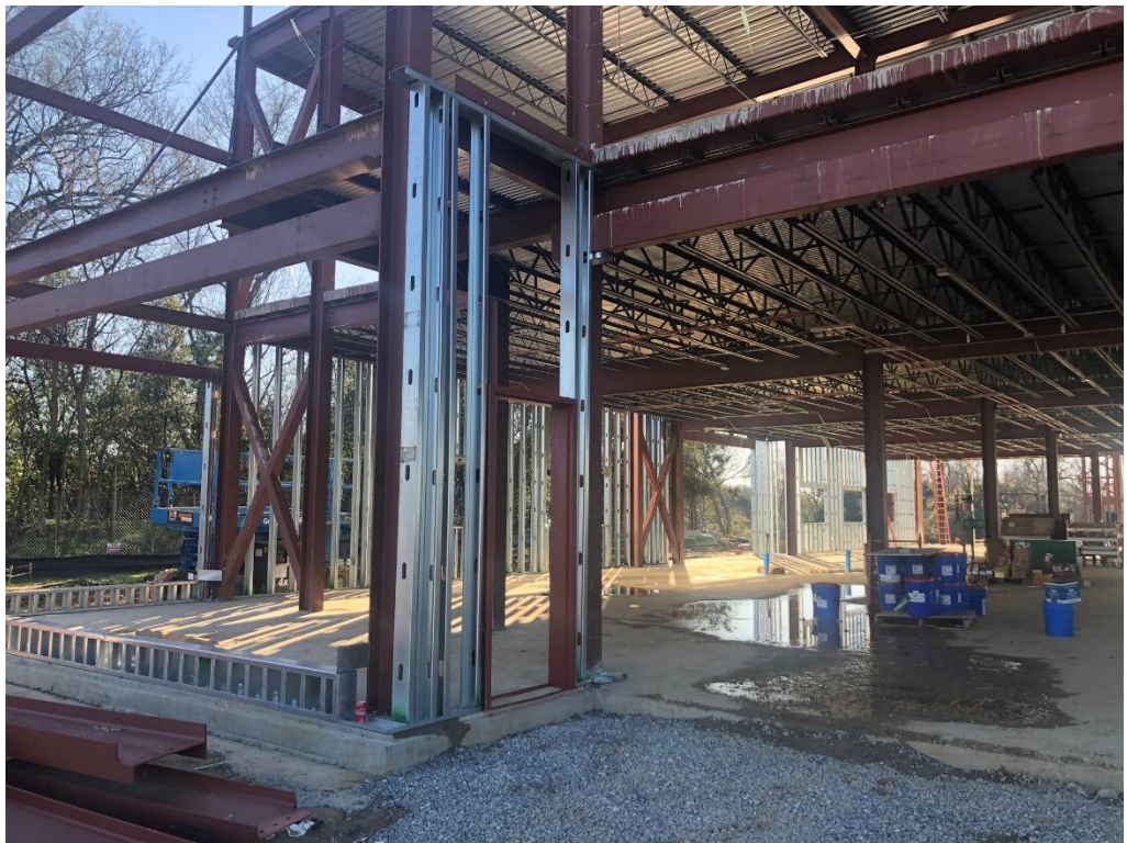
Figure 22 – East Building Door Set in Place
