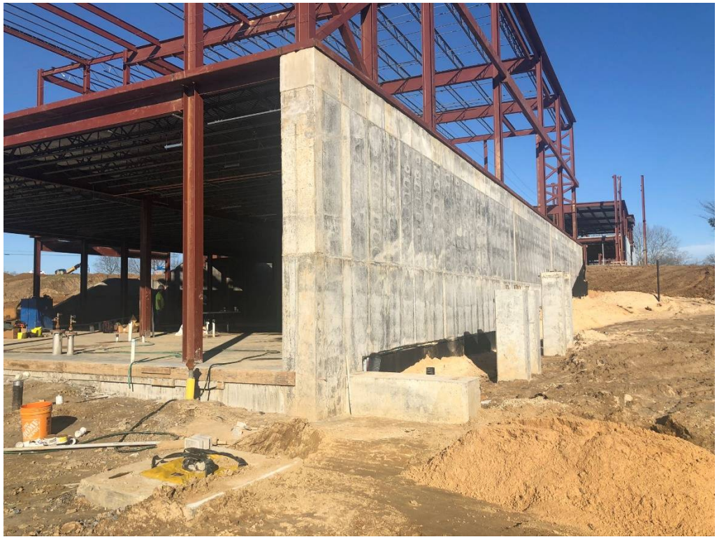
Figure 17 – Southwest Corner of Building
