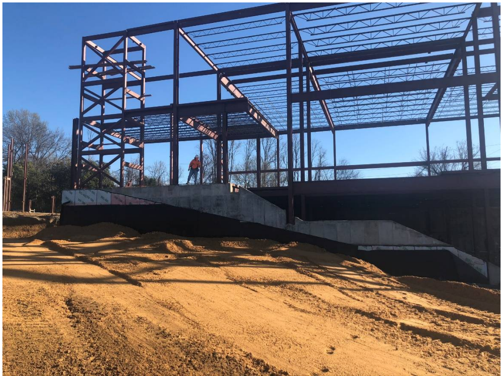
Figure 12 – West Structure Backfill Continued
