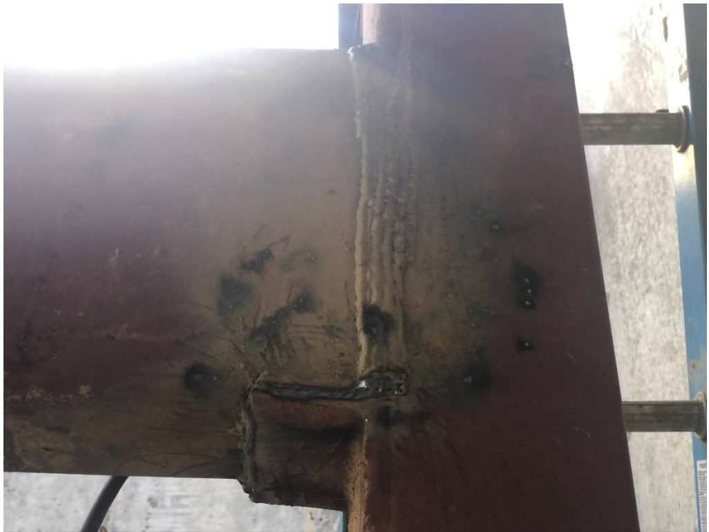
Figure 14 – Welding @ Elevator Shaft Structure
