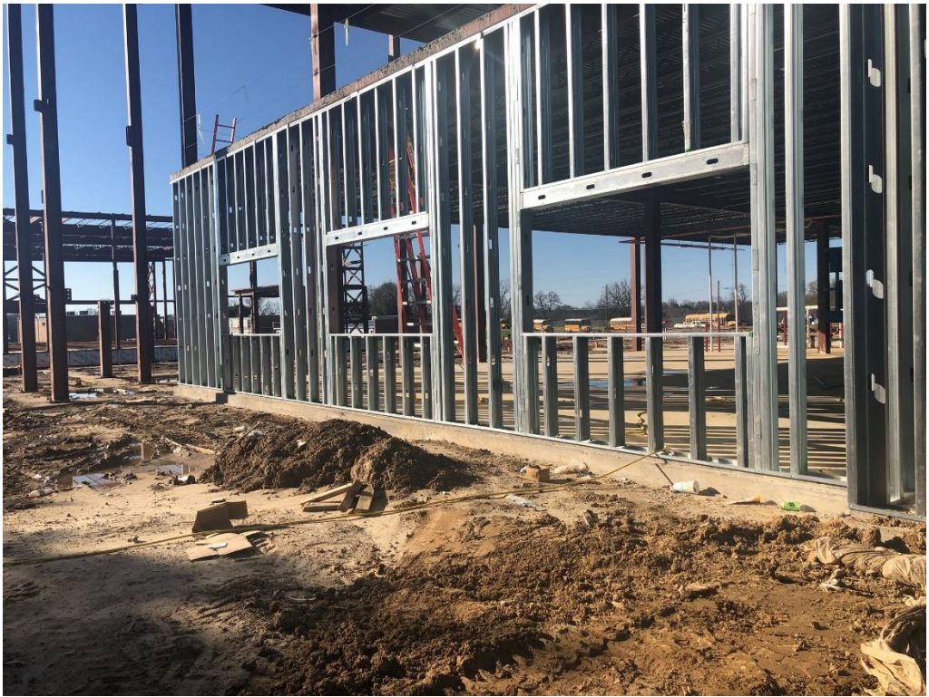
Figure 3 – Light Gauge Framing
