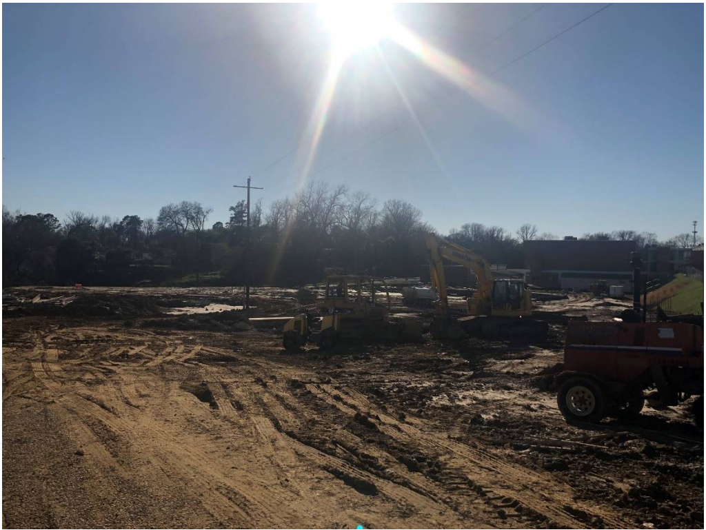
Figure 9 – North Entry Looking WSW
