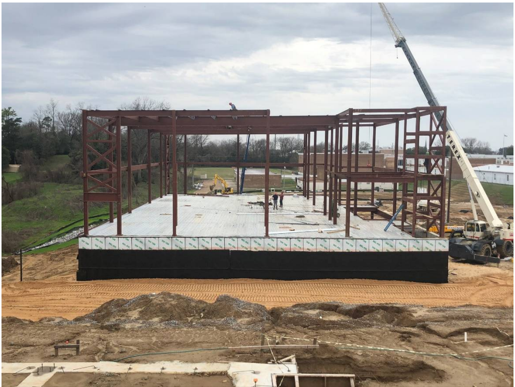
Figure 6 – West Building Progress
