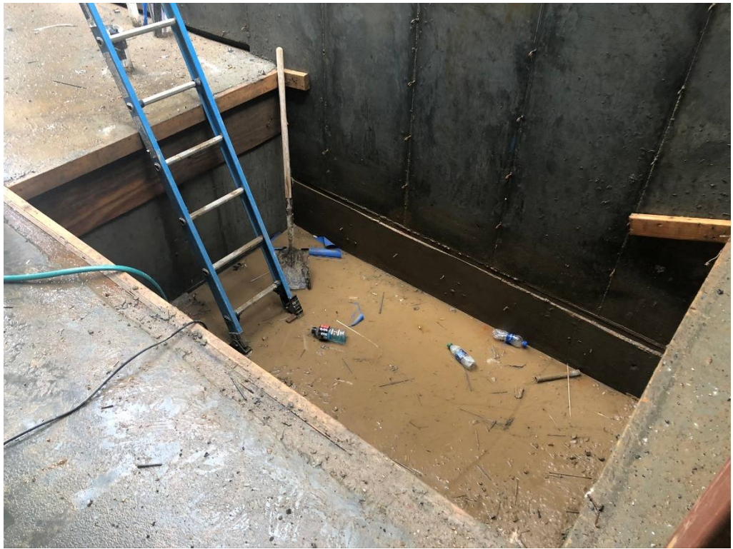
Figure 11 – Elevator Pit Drained
