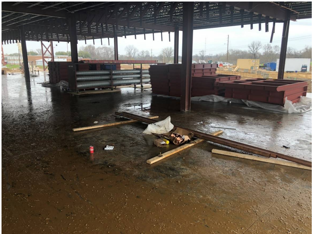
Figure 4 – Spiral Duct On Site
