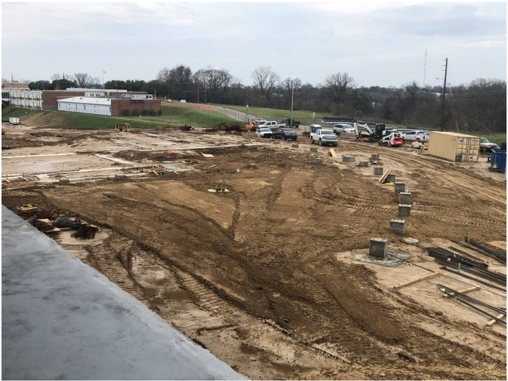
Figure 5 – Concrete Piers at North Curvature
