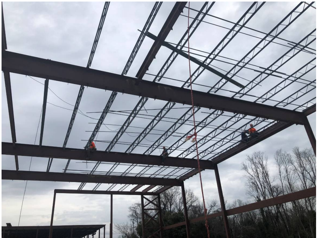
Figure 8 – Roof Joist Setting at West Building
