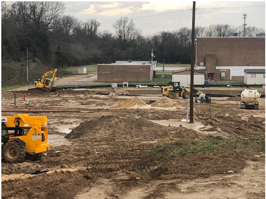
Figure 14 – Continued Sewer Work
