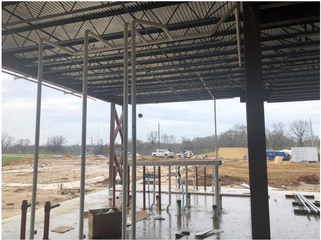
Figure 3 – Plumbing Rough-In Ongoing
