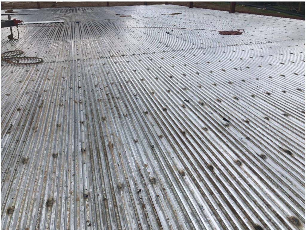
Figure 10 – Floor Steel Decking Prepped for Concrete
