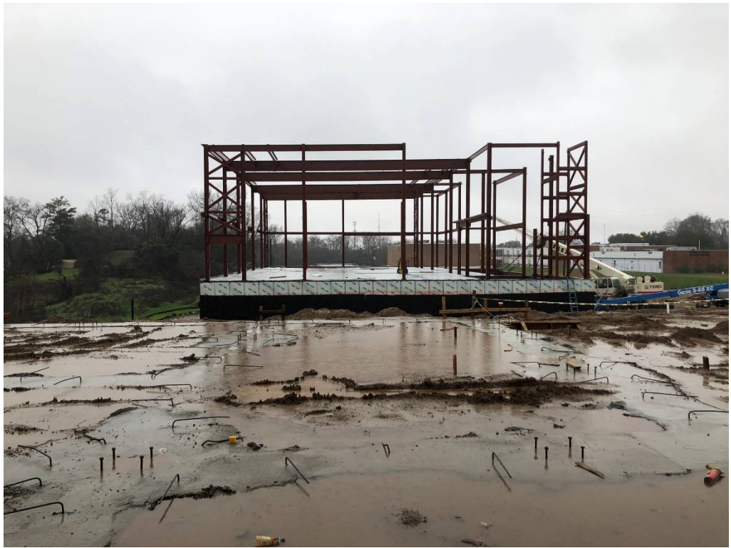
Figure 7 – West Building looking from West edge of East Structure
