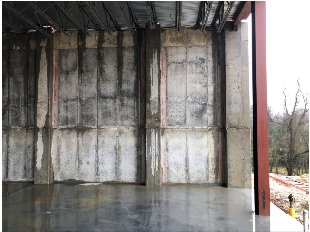
Figure 11 – South Wall in West Lower Building
