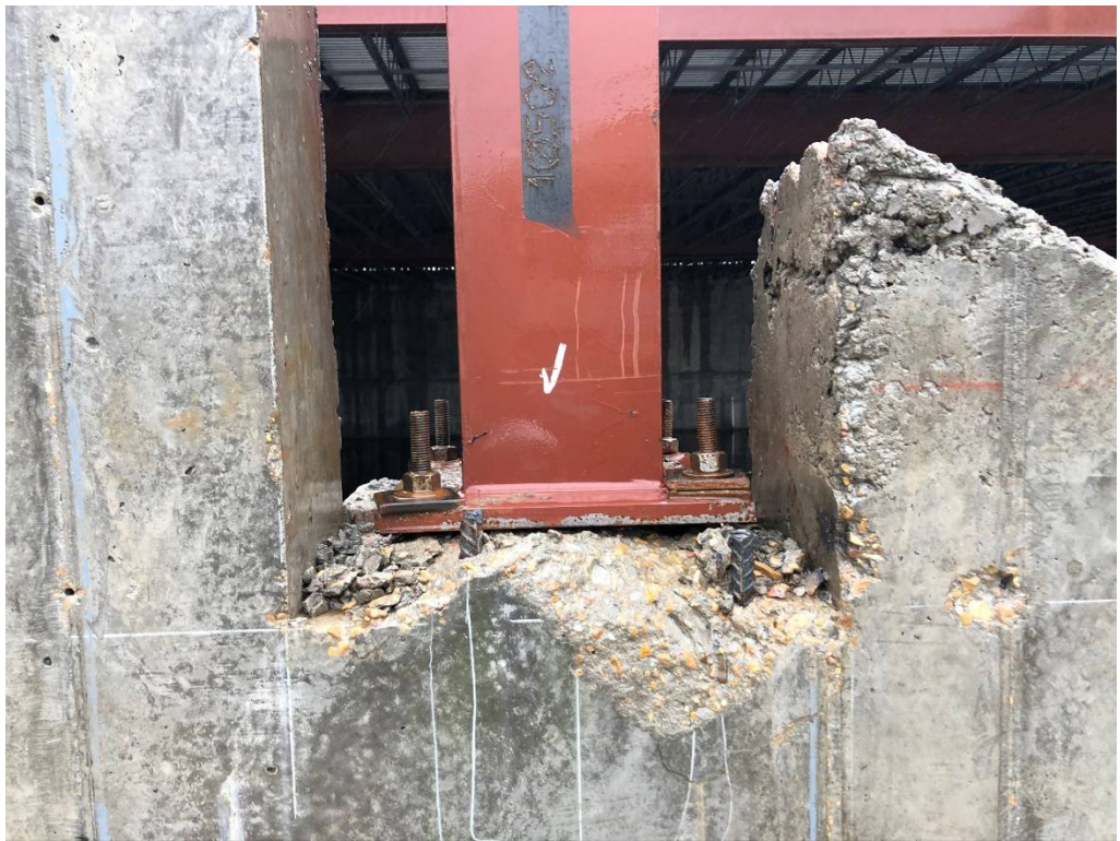
Figure 8 – Structural Connection @ West Building (North Center)
