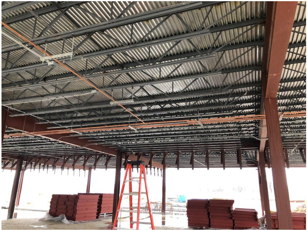
Figure 3 – Plumbing & Electrical Rough-In Ongoing
