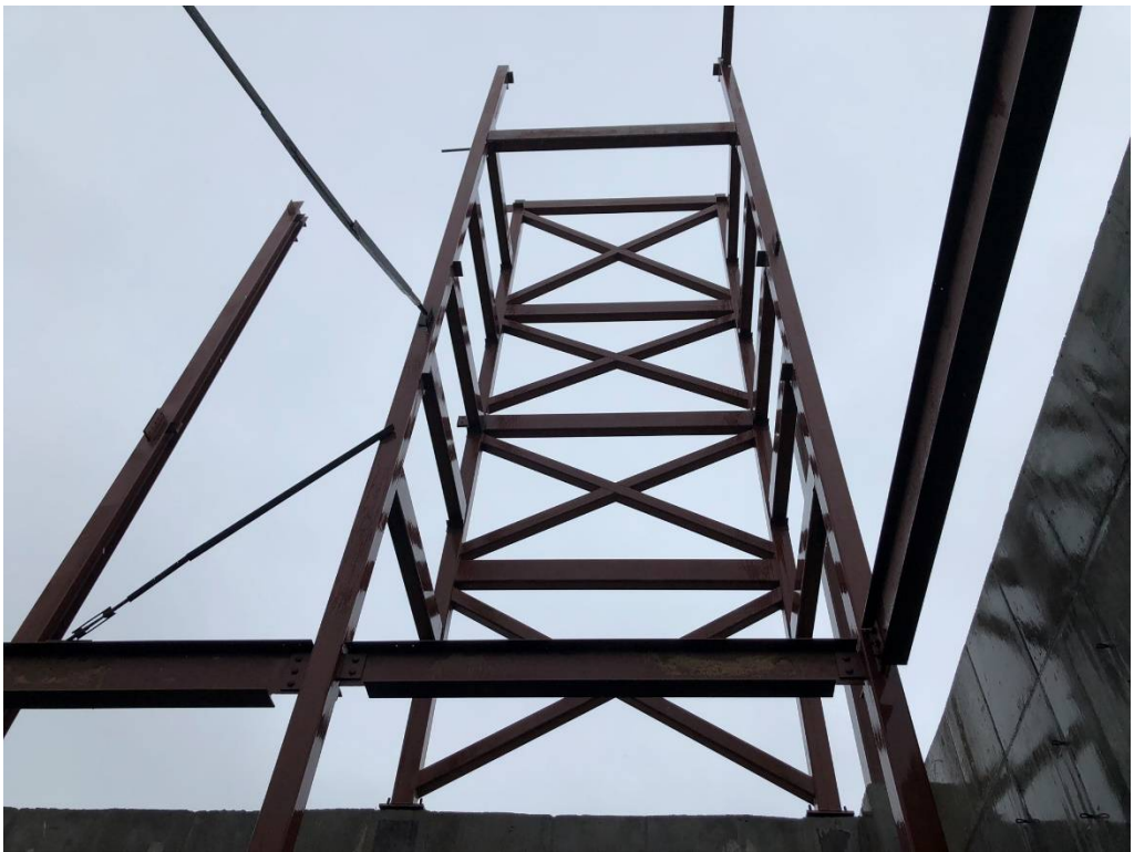
Figure 14 – Elevator Framework
