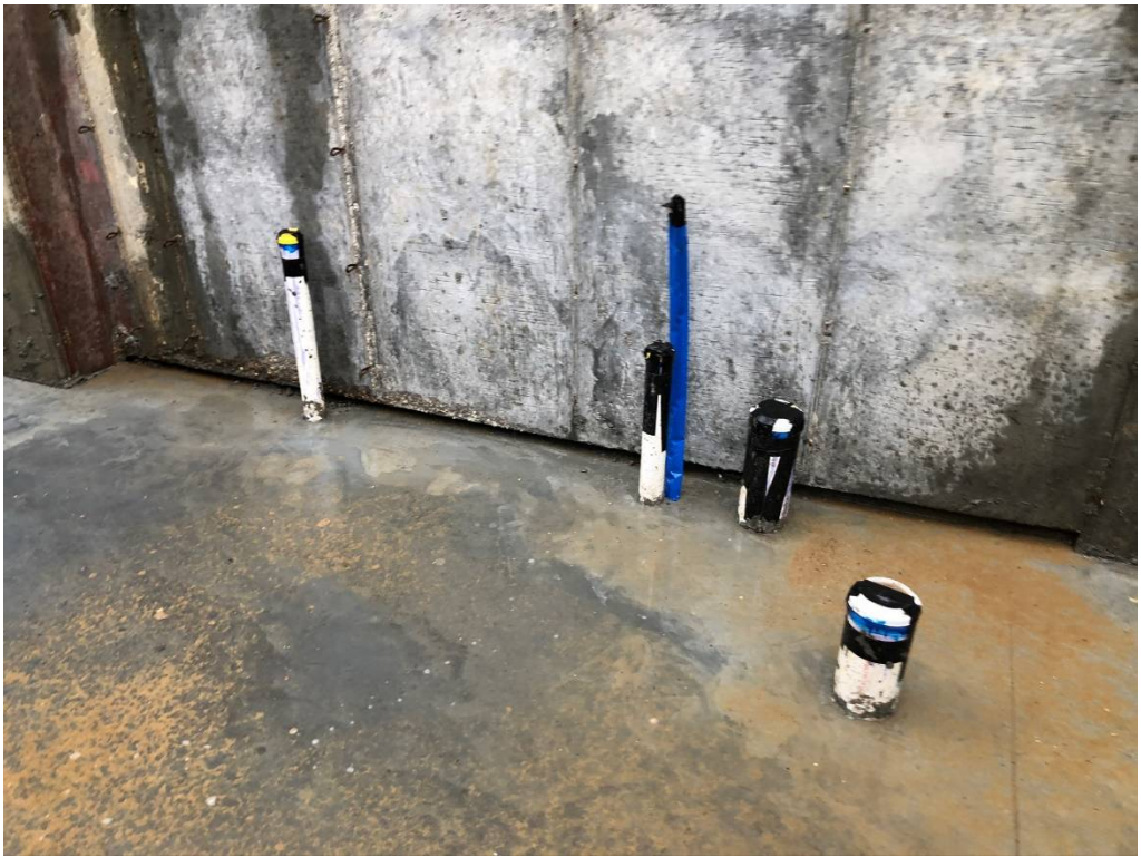
Figure 13 – Thru-Slab Penetrations
