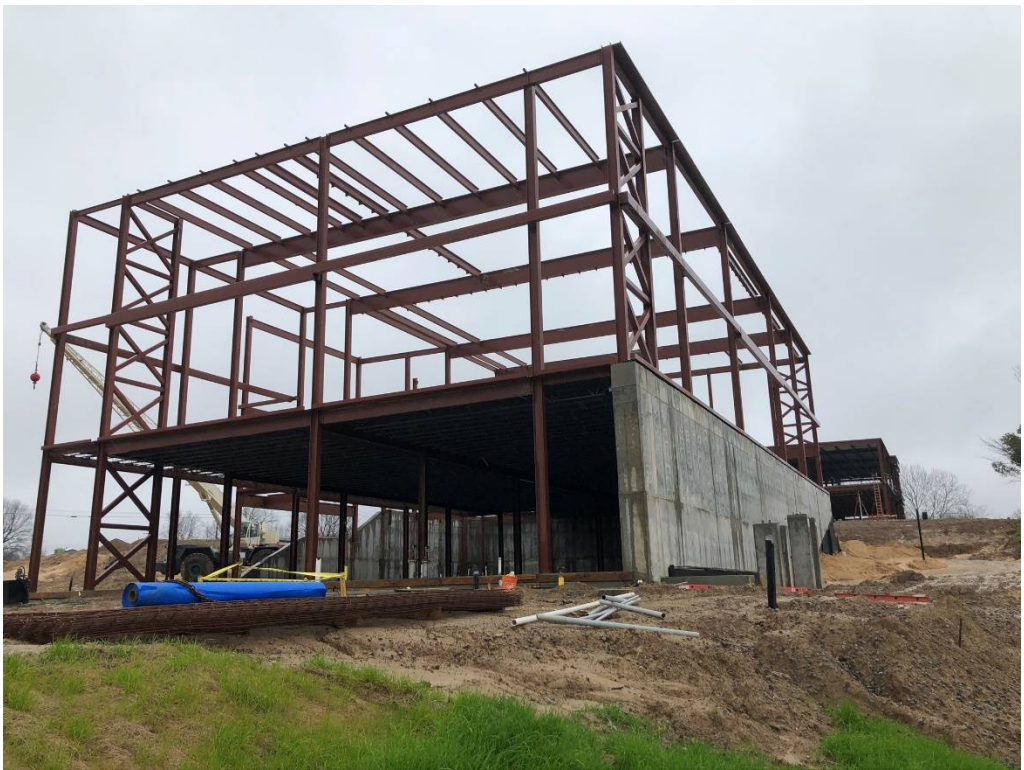
Figure 16 – West Structure from Southwest Vantage
