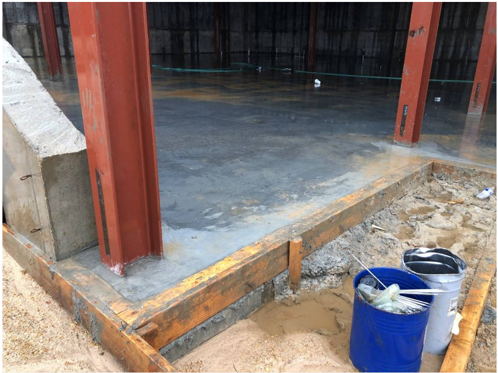
Figure 9 – Newly Poured Slab @ West Lower Level
