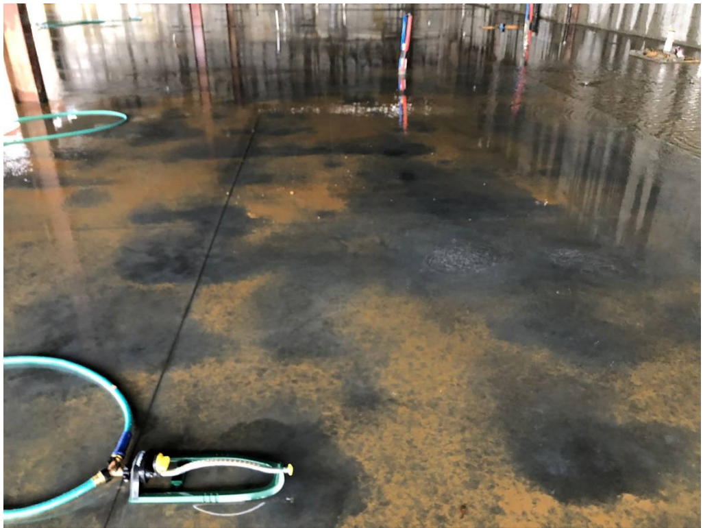
Figure 10 – Evidence that Slab has been kept Sprinkled (4 th Day Since Pour)
