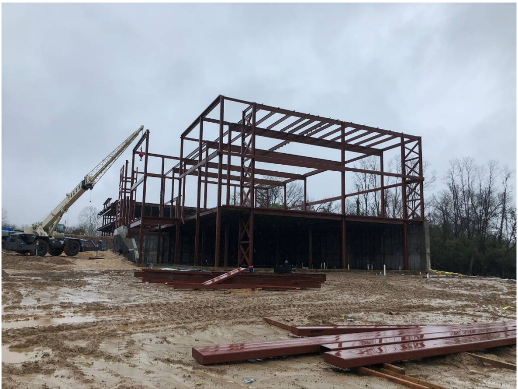
Figure 18 – West Structure from Northwest Vantage
