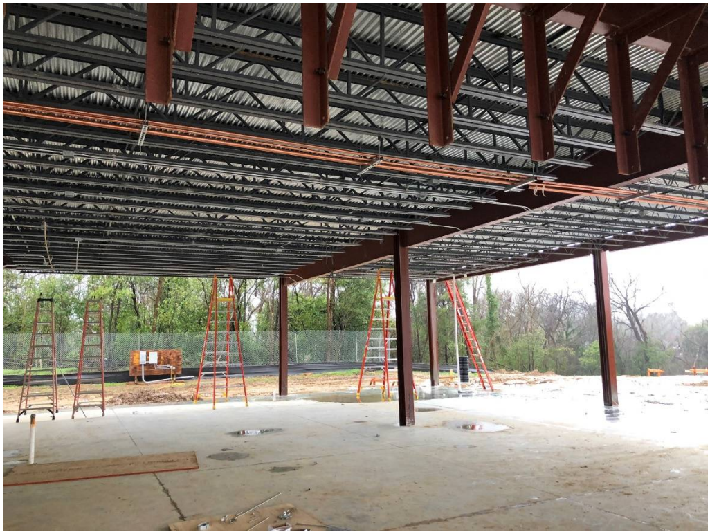
Figure 5 – Plumbing Rough-In Ongoing
