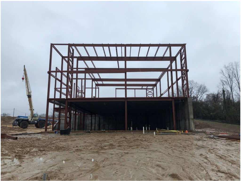
Figure 17 – West Structure from West Vantage
