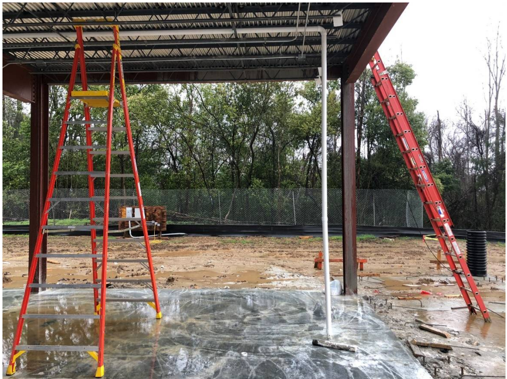
Figure 6 – Plumbing Rough-In Ongoing
