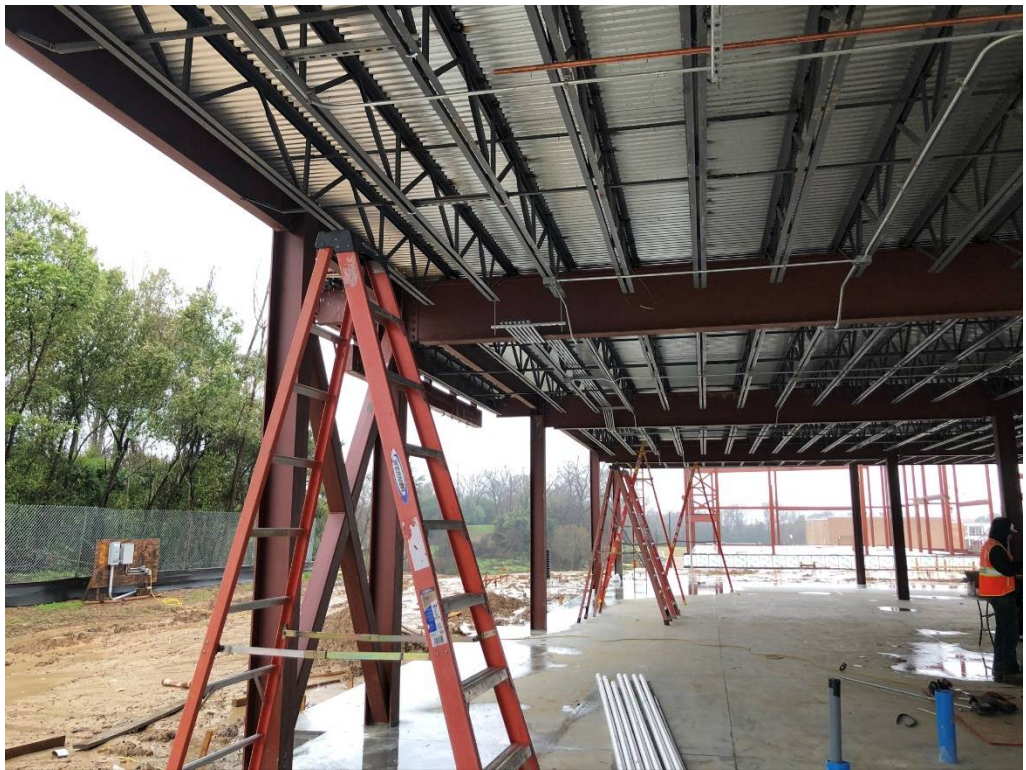
Figure 2 – Plumbing Rough-In Ongoing
