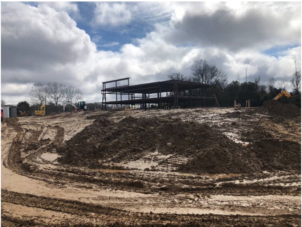
Figure 8 – North Entry Looking ESE
