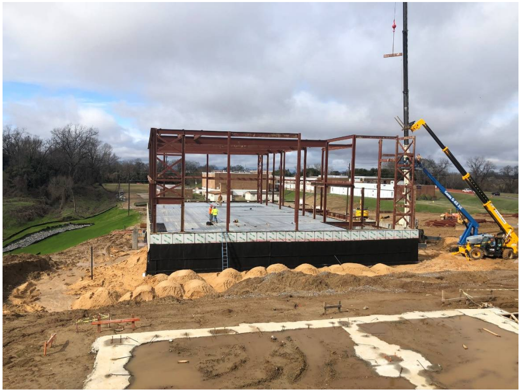
Figure 5 – West Building Platform
