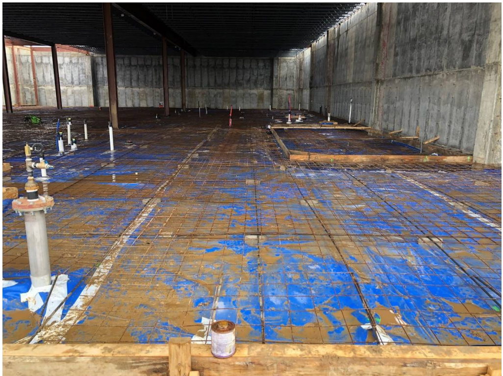
Figure 10 – Rebar @ West Bottom Floor
