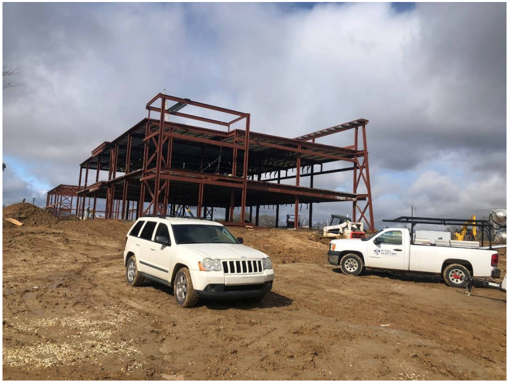
Figure 1 – East Building Erected
