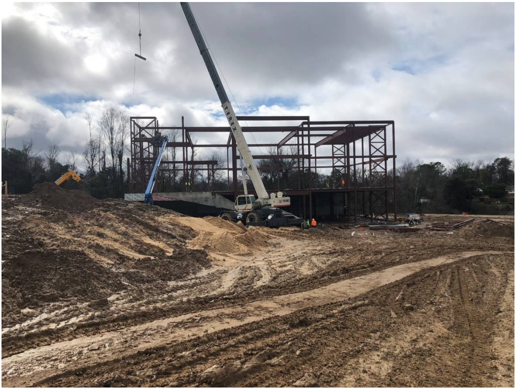
Figure 7 – North Entry Looking S
