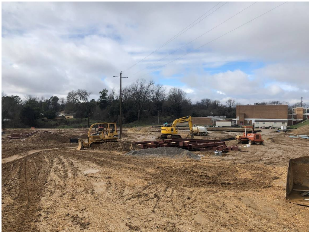
Figure 6 – North Entry Looking WSW
