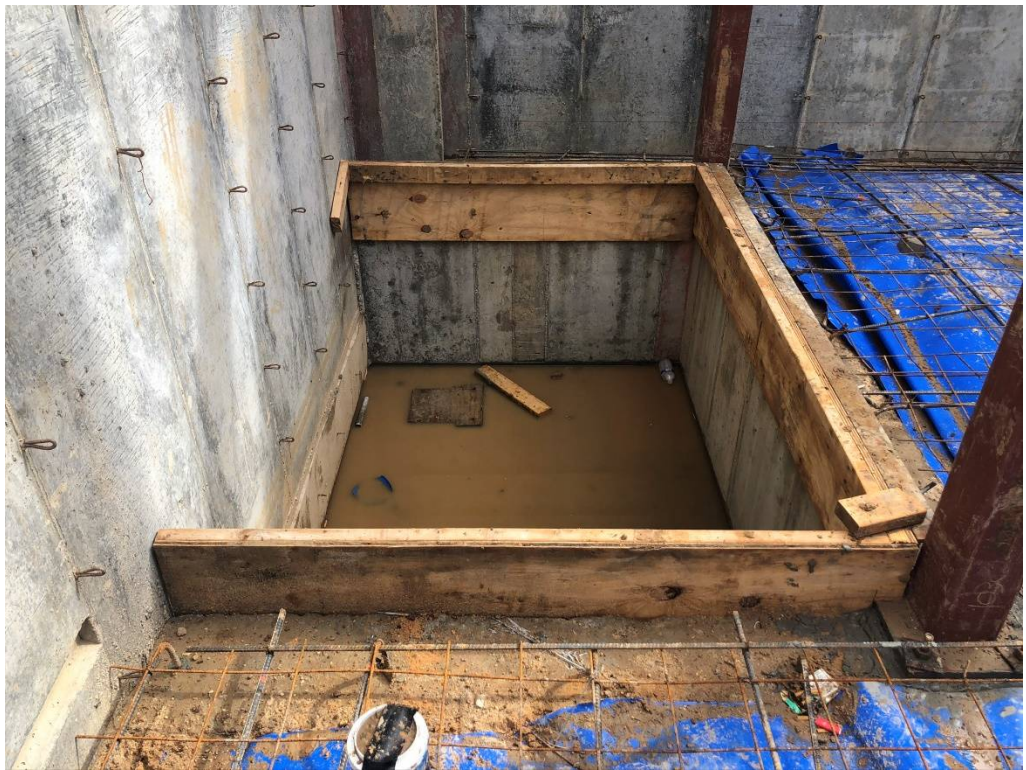
Figure 14 – Elevator Pit
