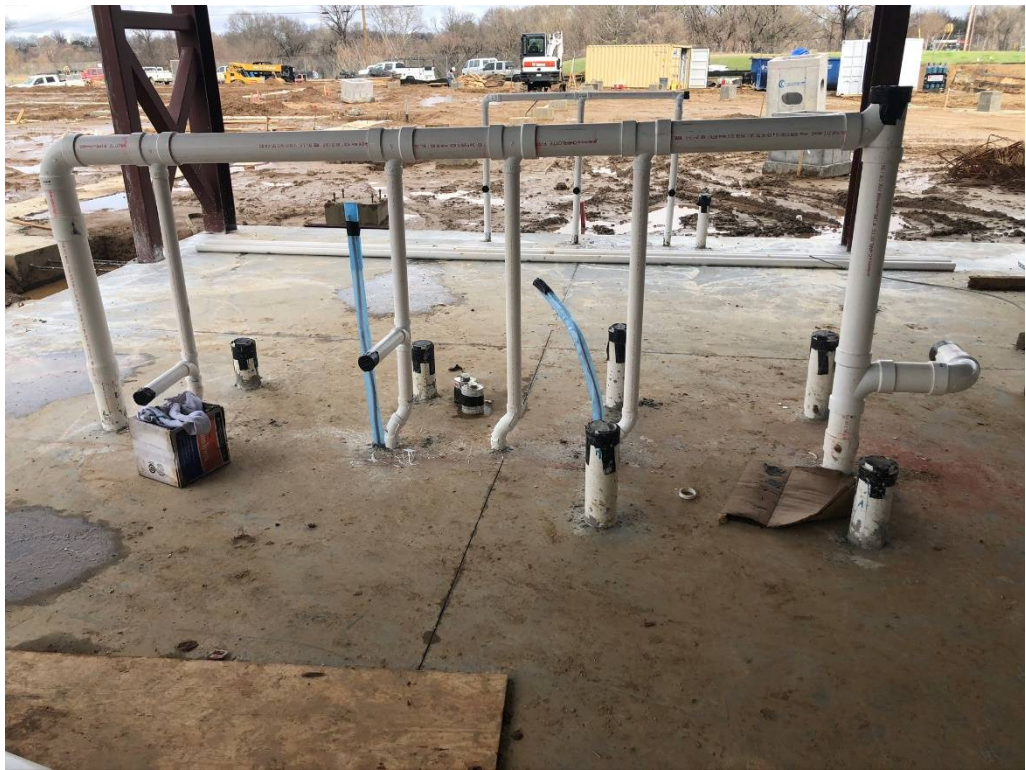
Figure 4 – Plumbing Rough-In Ongoing
