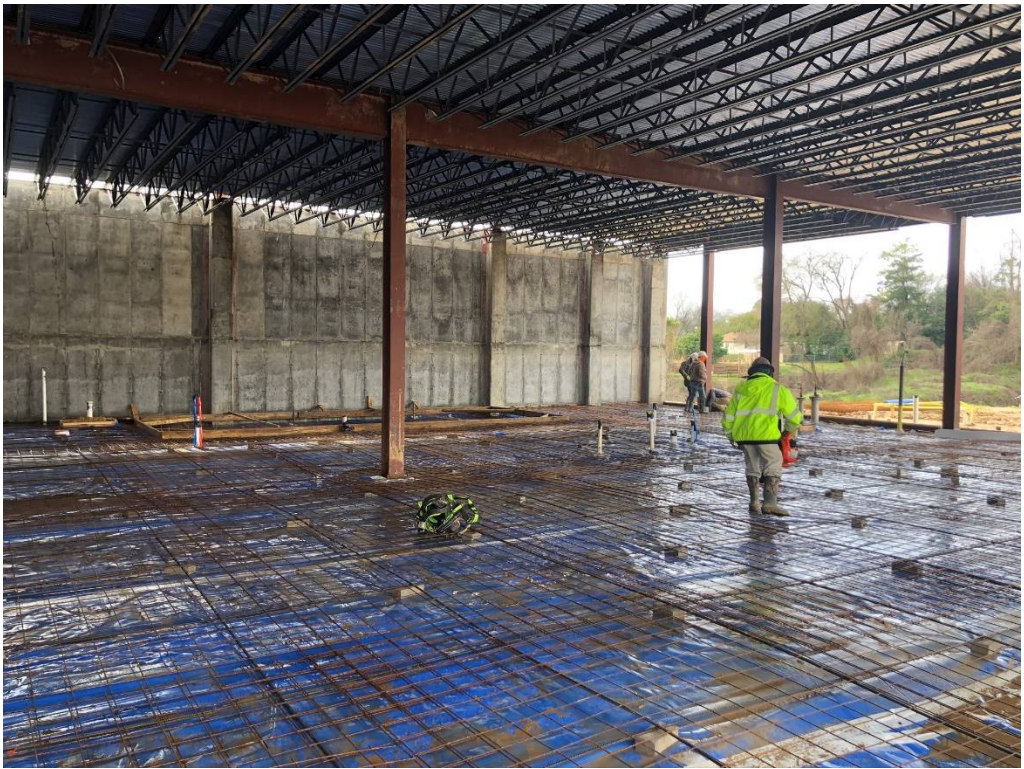
Figure 15 – Rebar at Lower Level
