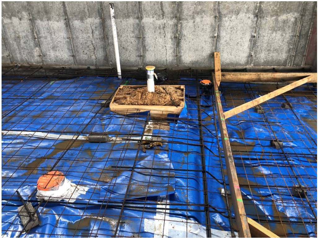
Figure 11 – Rebar and Form @ South Wall in West Lower Building
