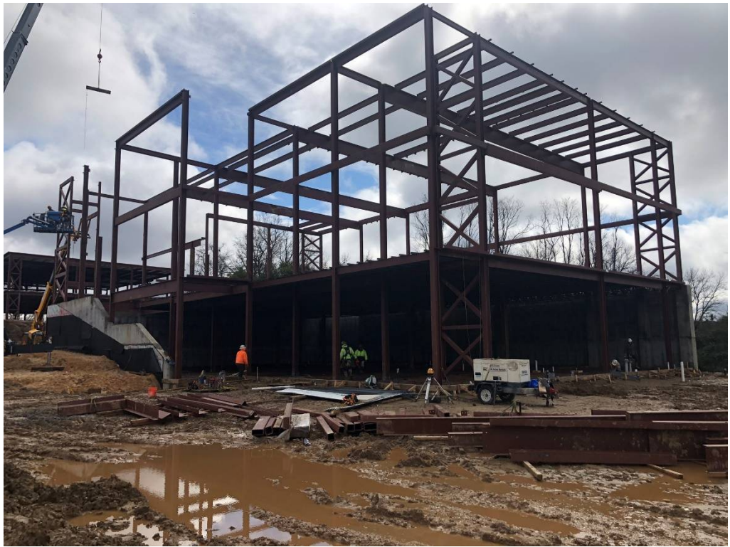
Figure 9 – NW Corner of West Building Looking SE
