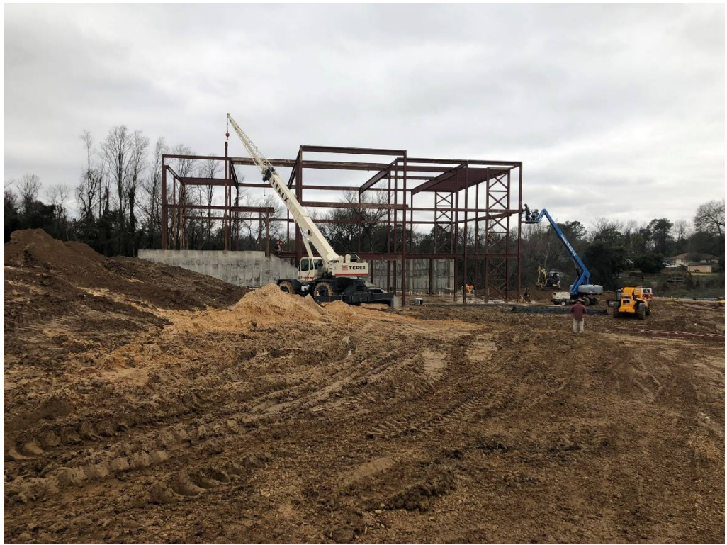
Figure 21 – North Entry Looking S
