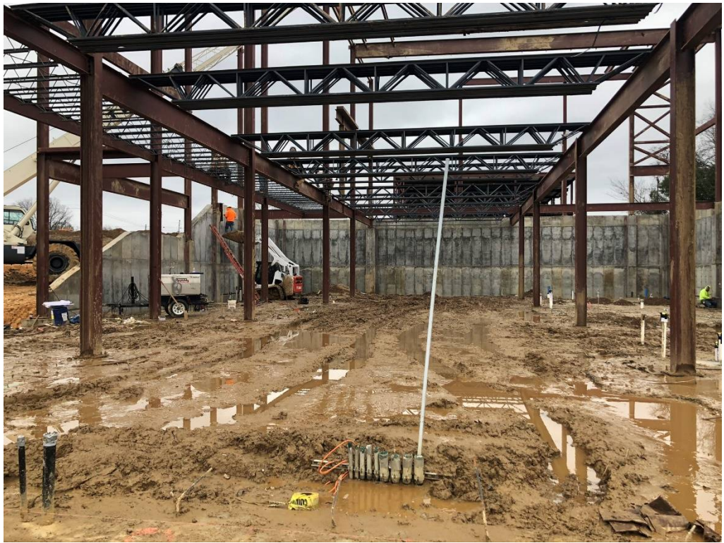
Figure 13 – Lower West Section of Building Looking East
