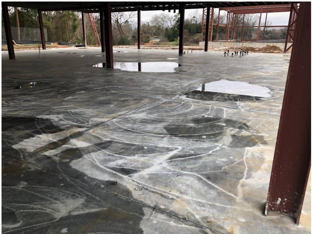
Figure 2 – Lower Slab Day 7
