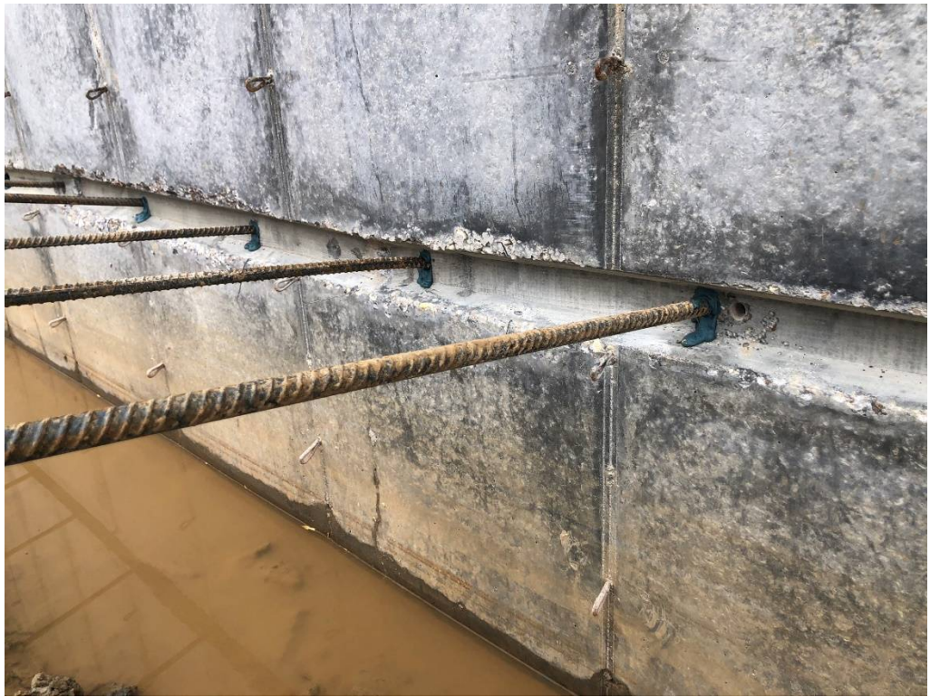
Figure 15 – Rebar Installed with Epoxy at Lower Level
