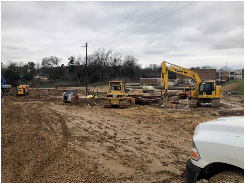
Figure 20 – North Entry Looking WSW
