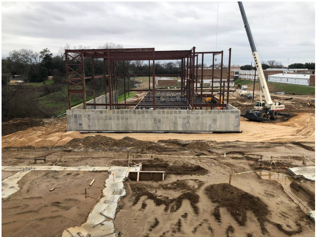
Figure 6 – West Building Steel Erection Progress
