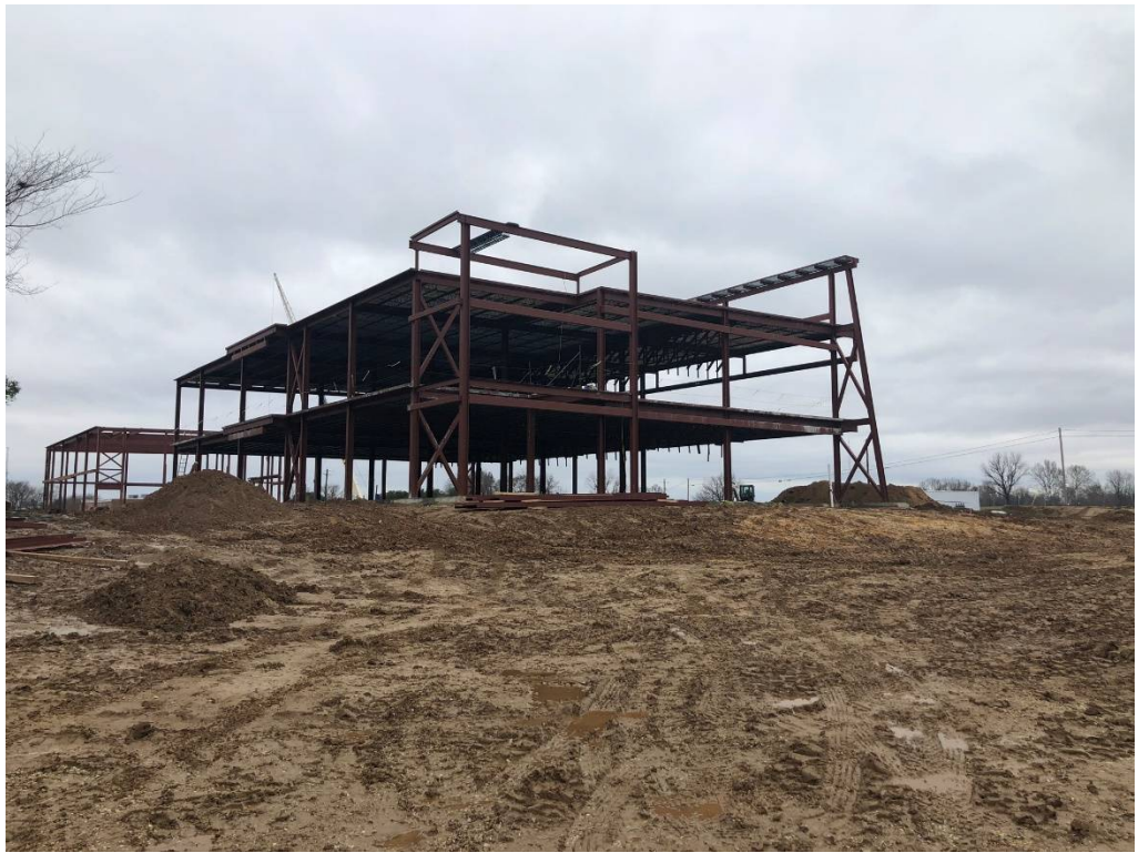
Figure 1 – East Building Erected
