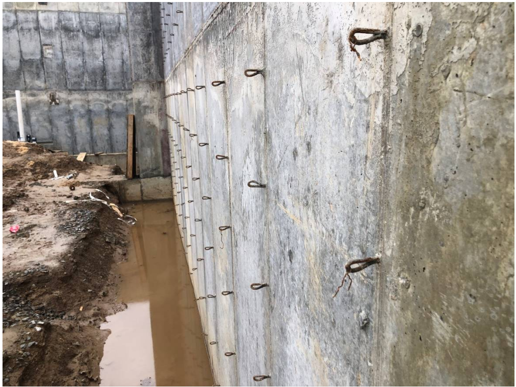
Figure 17 – Concrete Work and Mechanical Attachments at Foundation Wall
