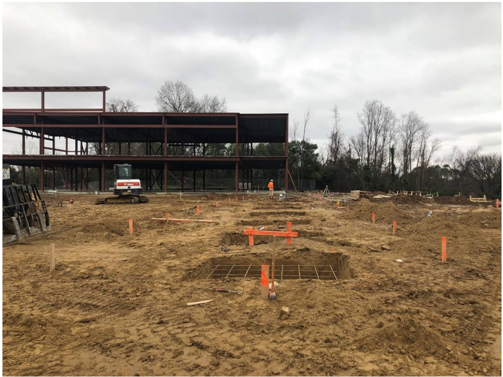
Figure 23 – Out Stretch of Structure from North Perspective
