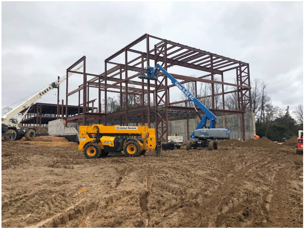
Figure 11 – Progress on Steel Erection from NW of Structure
