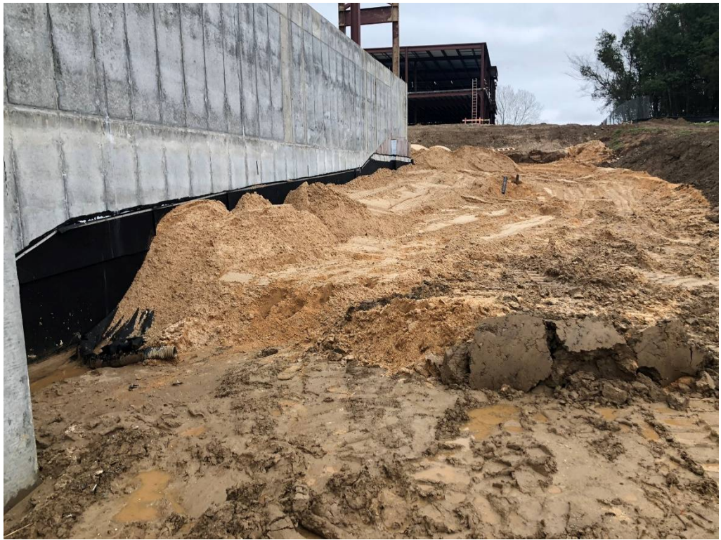
Figure 19 – Select Fill Installed at South Section of Lower West Building
