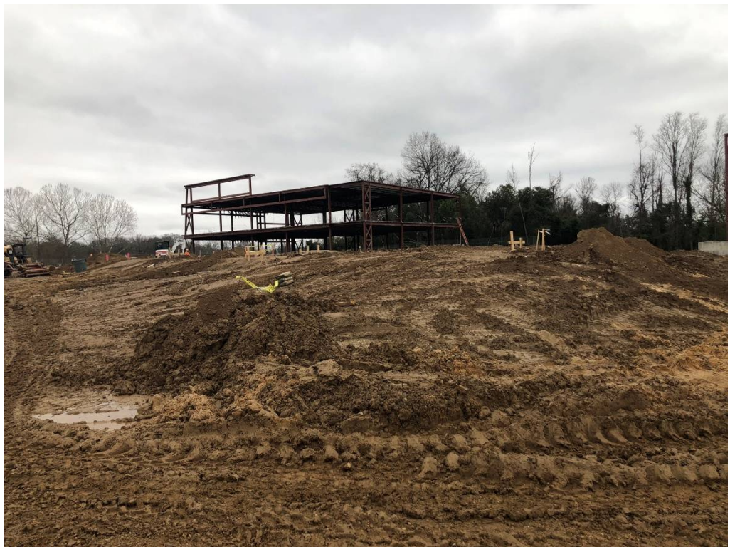
Figure 22 – North Entry Looking ESE
