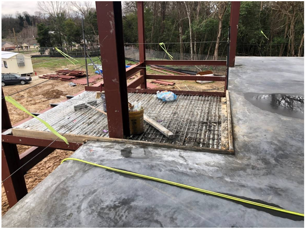
Figure 5 – Section Un-Finished (Awaiting Steel Egress Stair Installation)
