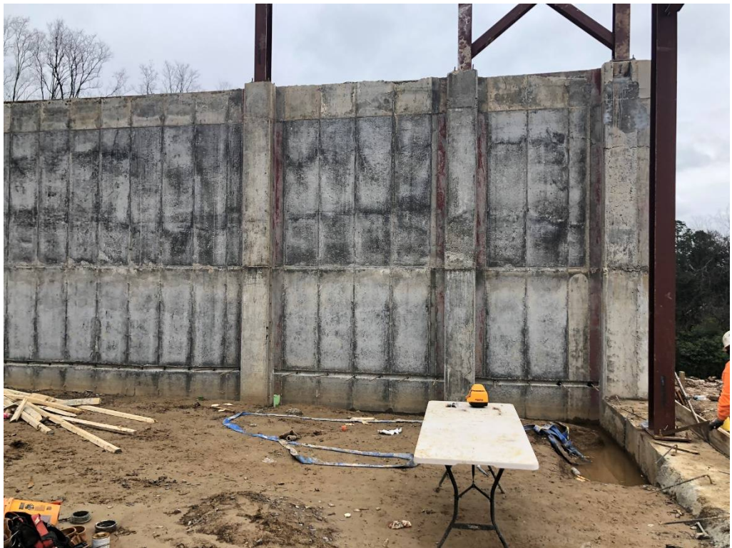
Figure 14 – Southwest Corner of Structure
