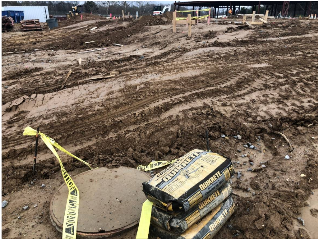
Figure 9 – Man Hole Installed at North Section of Site
