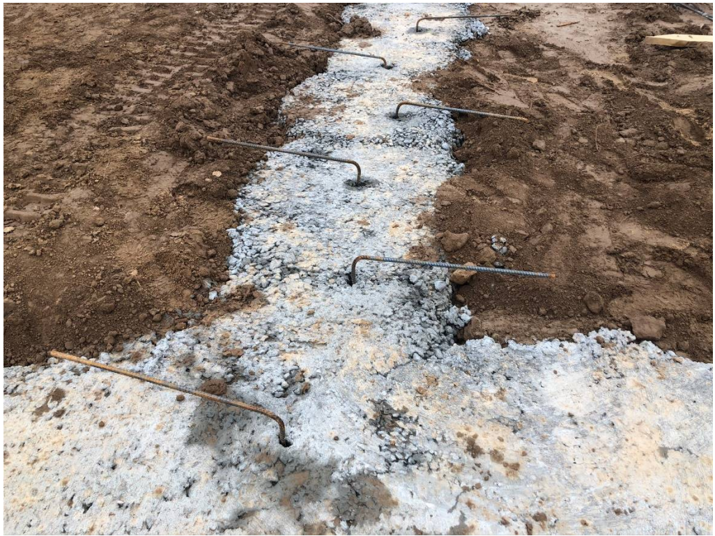
Figure 7 – New Footings Poured on North Central Section of Building
