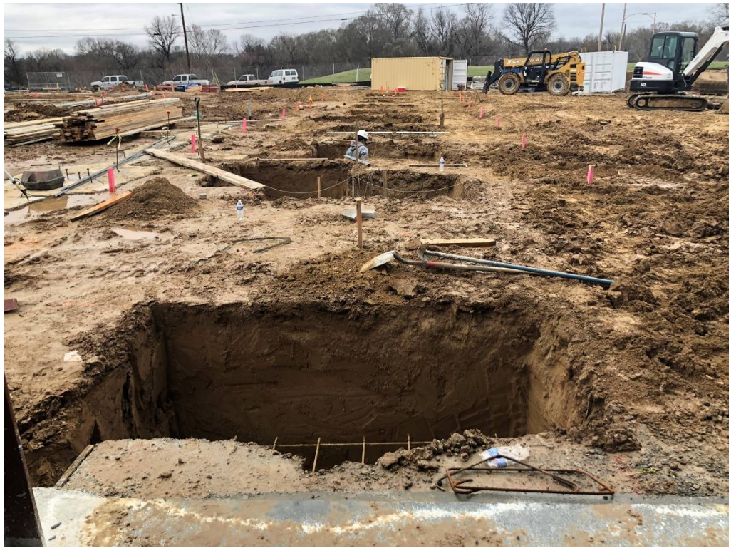
Figure 3 – Footing Dug for North Out Stretch of Buidling
