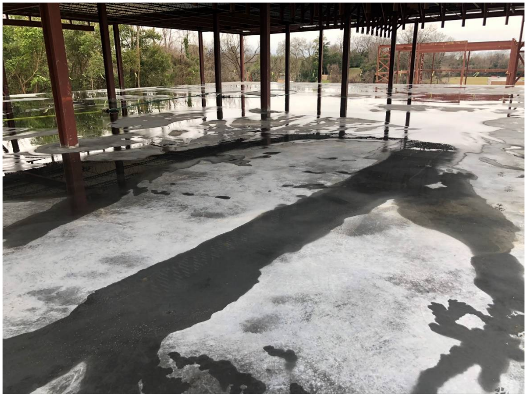
Figure 4 – Upper Slab Day 5
