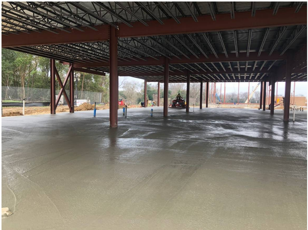
Figure 2 – Poured Slab, ready for Troweling (Wednesday)
