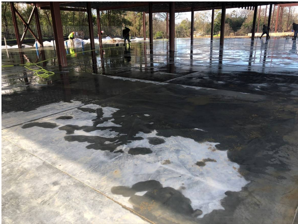
Figure 6 – Finished Slab @ Lower Level (Today)
