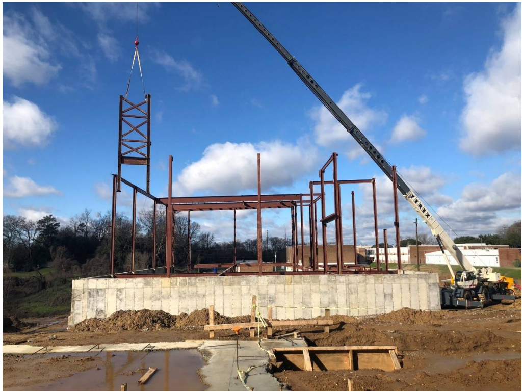
Figure 9 – Continued Steel Work @ Lower Level
