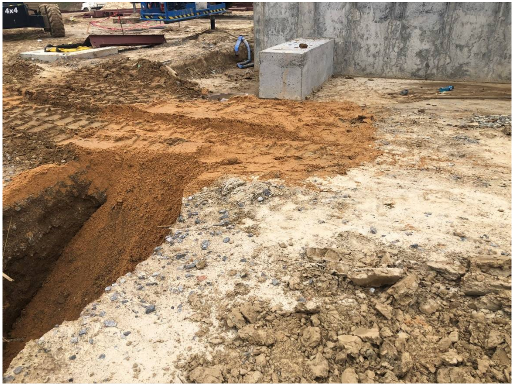
Figure 3 – Compacted Fill @ Southwest Corner (Wednesday)
