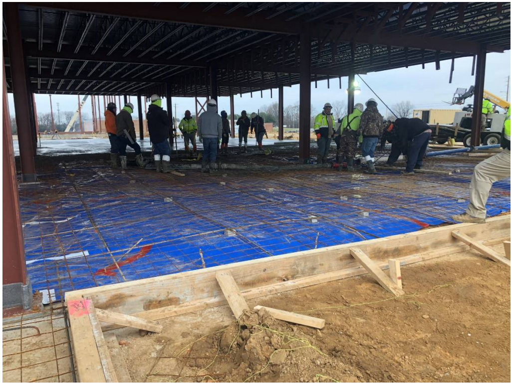
Figure 1 – Concrete work at Lower Level (Wednesday)
