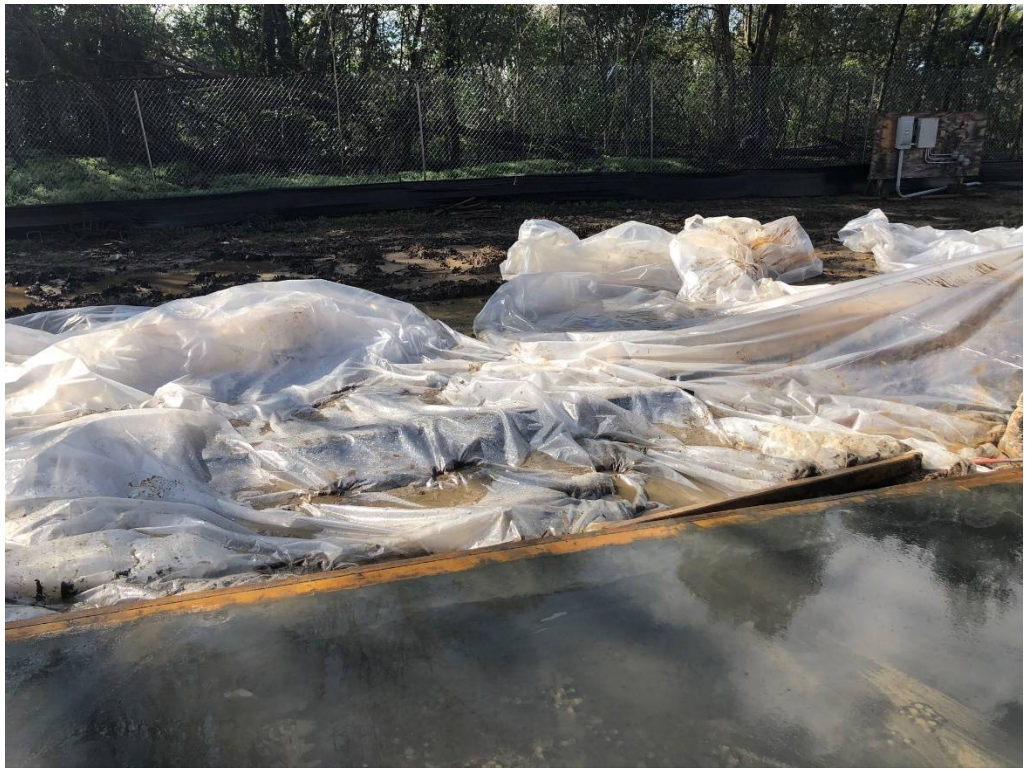
Figure 7 – Plastic Used to Cure Slab (Today)
