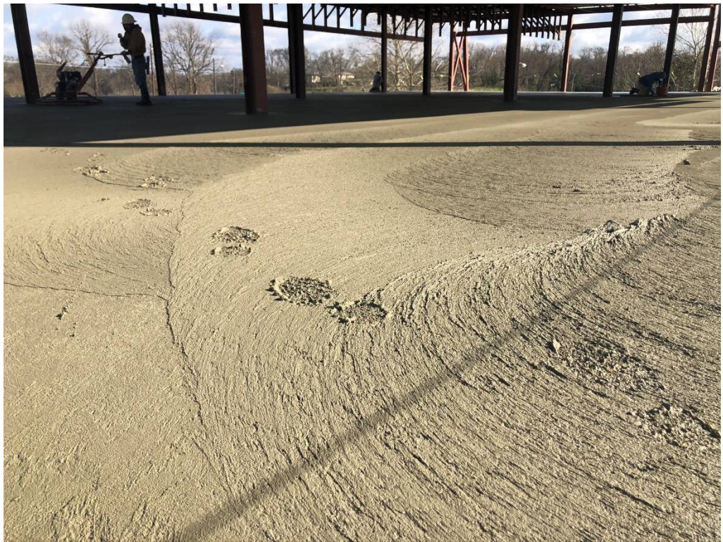
Figure 8 – Second Floor Slab, Ready for Troweling (Today)
