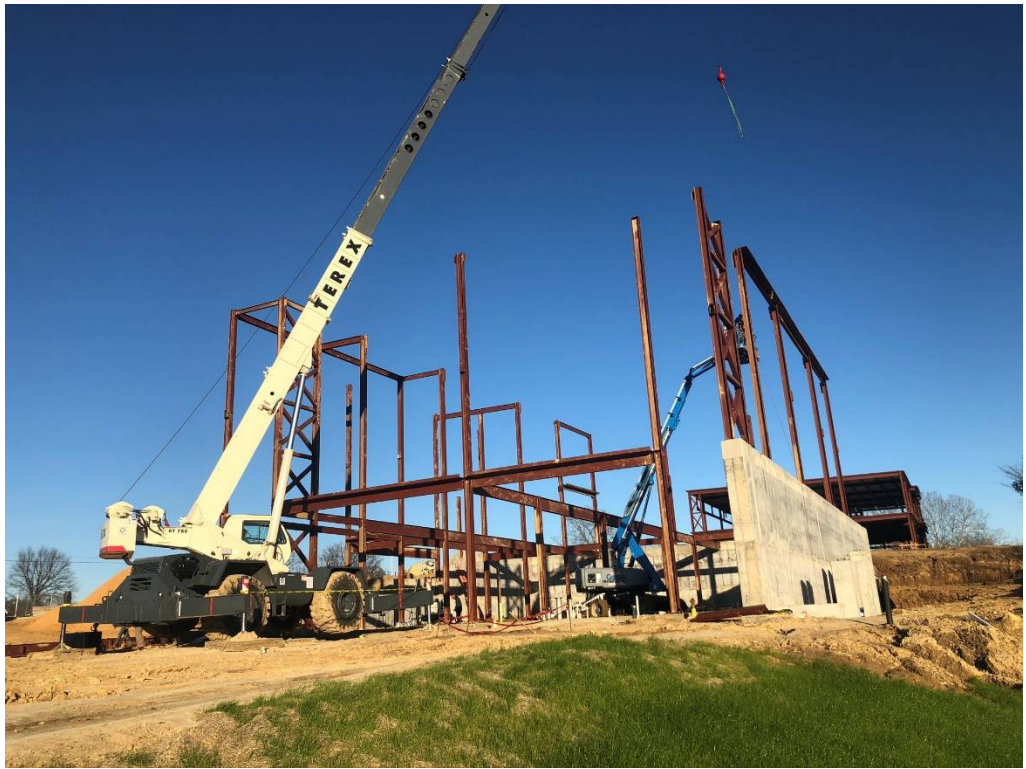
Figure 13 – Steel Erected; View From Southwest corner looking WNW
