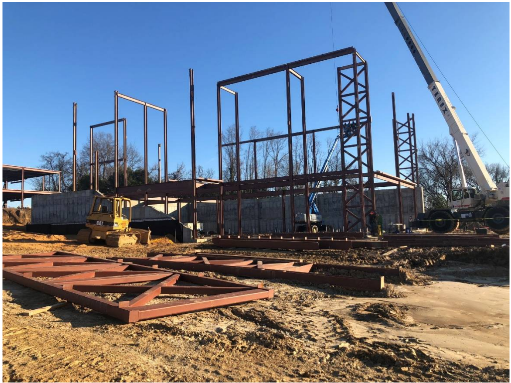
Figure 9 – Steel Erected; view from north west corner looking SSE
