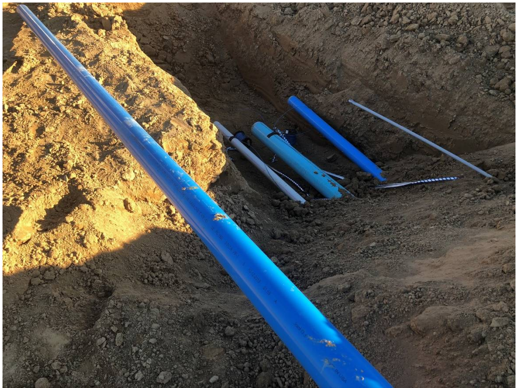
Figure 10 – Underground Utilities to west of lower structure
