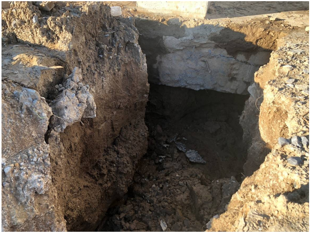
Figure 15 – Underside of footing exposed
