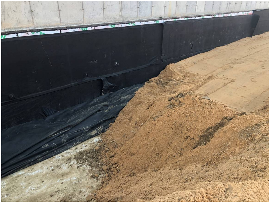
Figure 17 – Select Fill Installed at foundation wall
