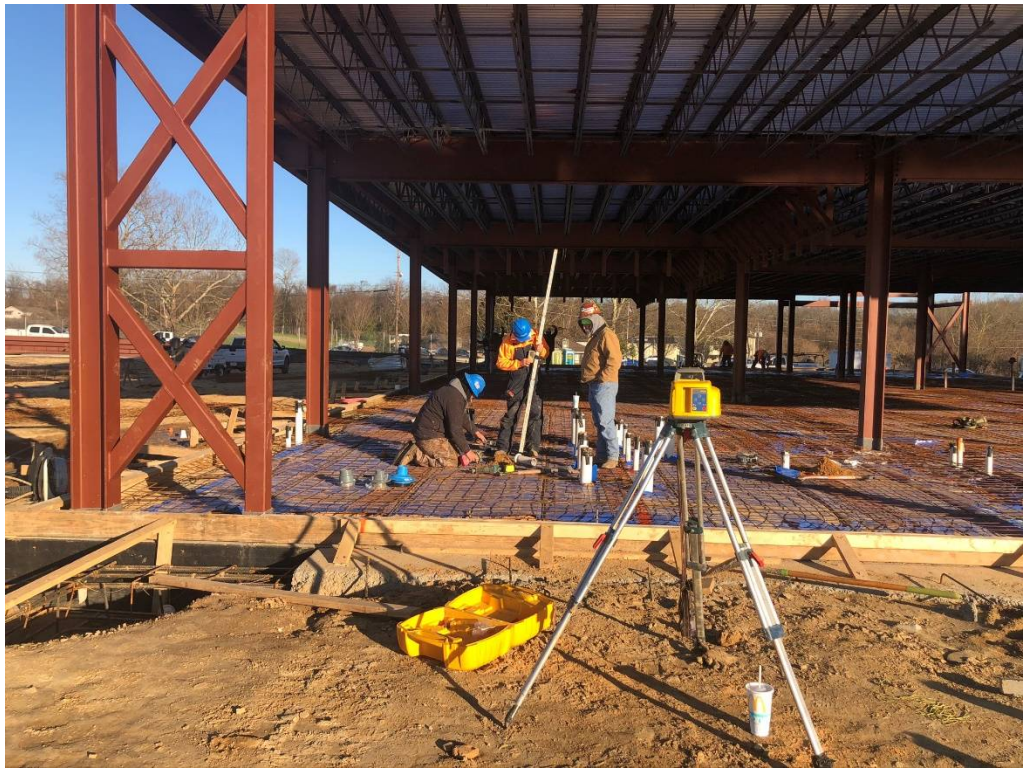
Figure 7 – Plumbers setting floor drains
