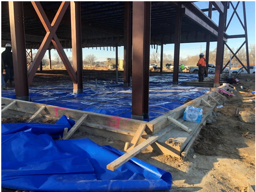
Figure 2 – Formwork in place
