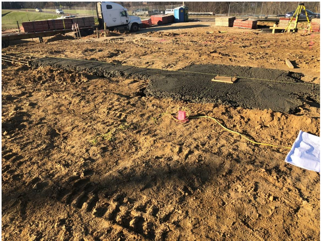
Figure 8 – Newly poured Concrete Footings
