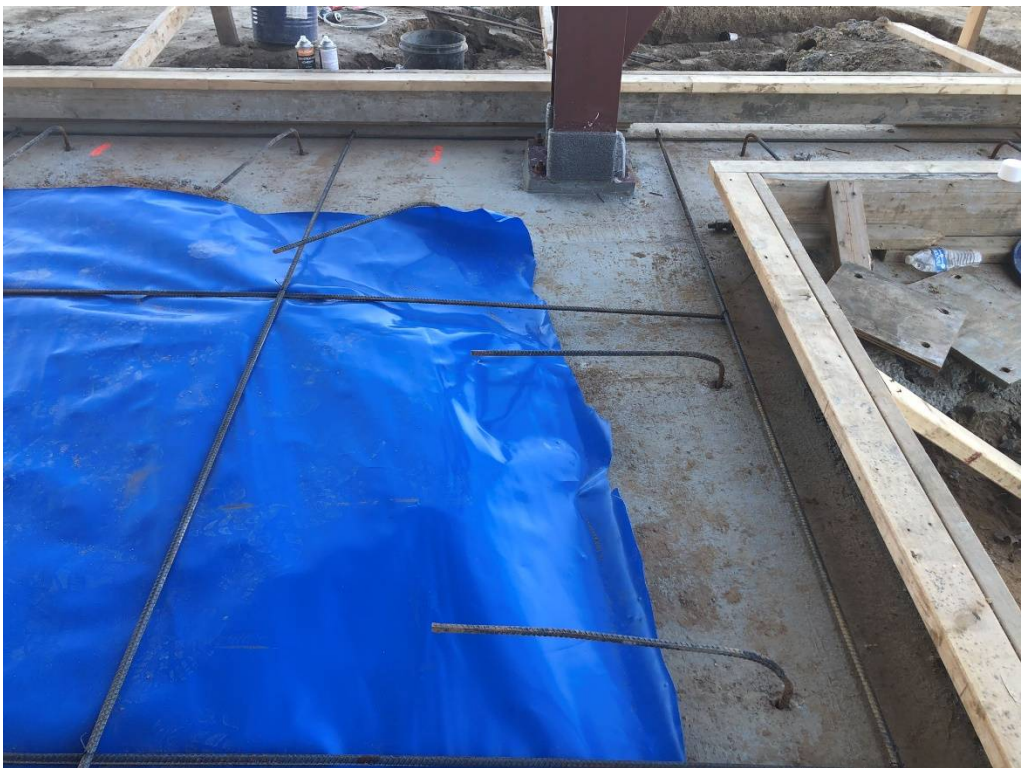
Figure 6 – North East corner of Upper Structure
