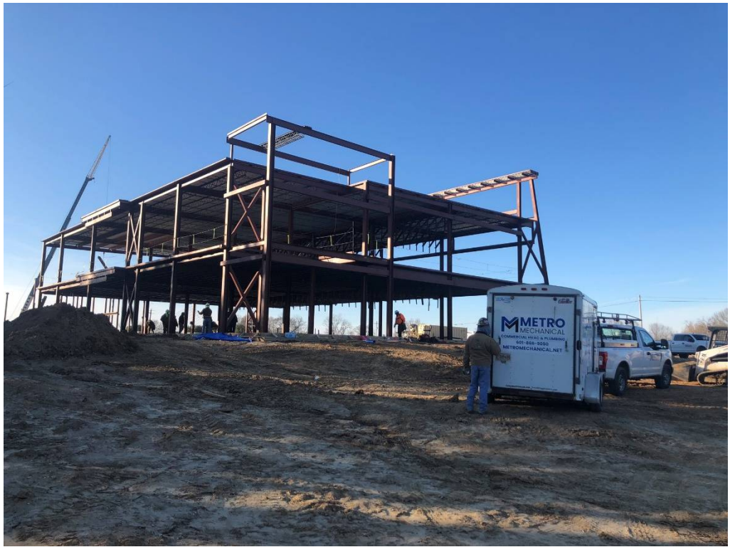
Figure 1 – Red Steel Erected
