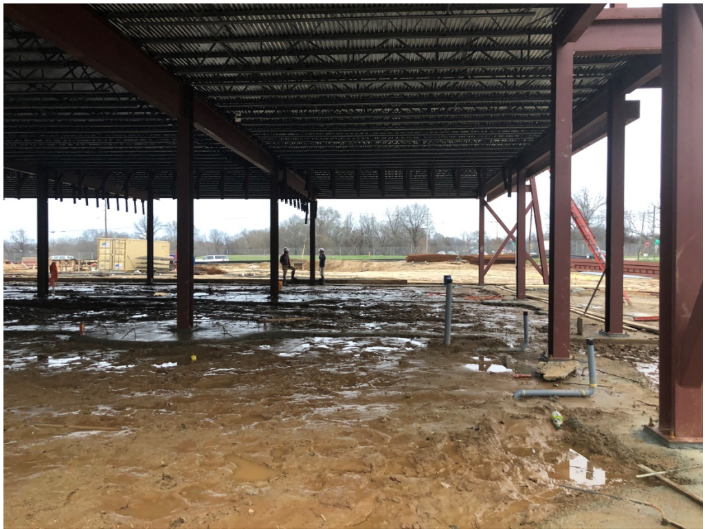
Figure 2 – Upper East Building Site Condition
