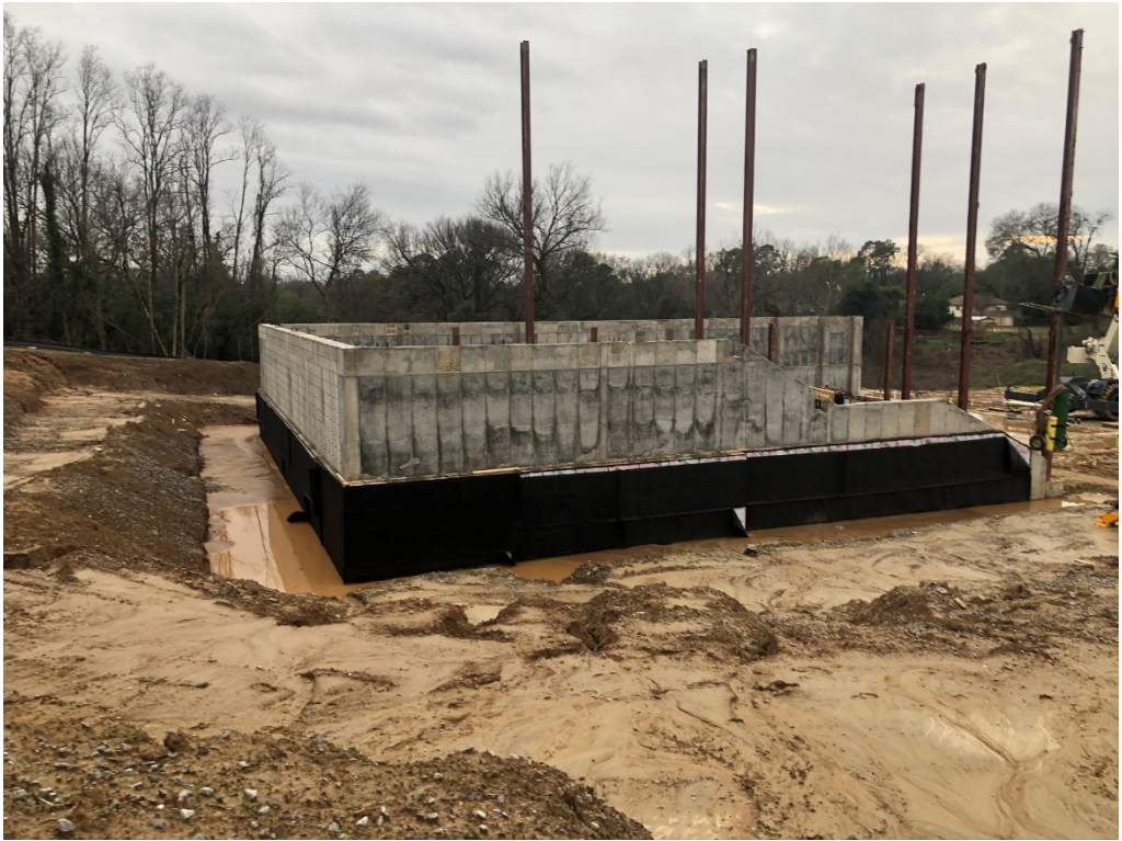
Figure 5 – Lower Level Progress, Steel Erected
