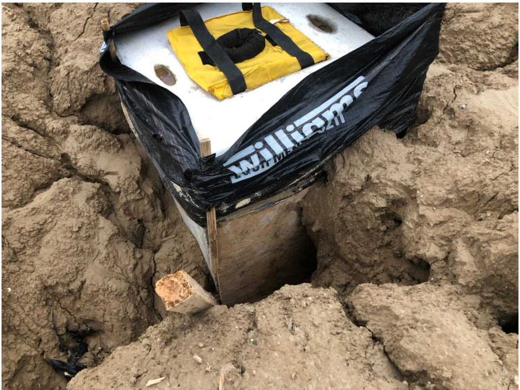
Figure 10 – Northeast Storm Sewer Set
