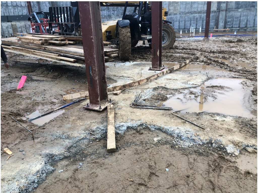
Figure 6 – Steel @ Lower Level Footings
