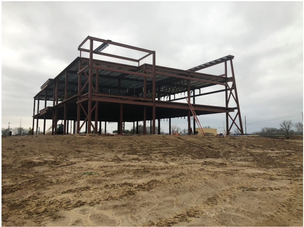
Figure 1 – Red Steel Erected
