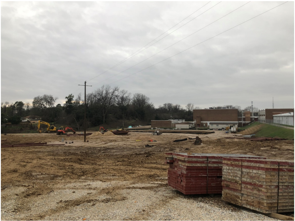
Figure 9 – North Entry Looking WSW
