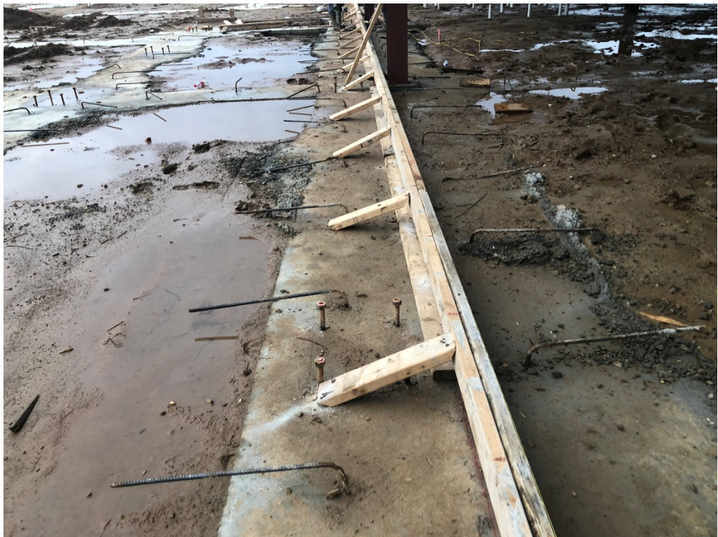
Figure 4 – Formwork @ Upper East Building for Topping Slab
