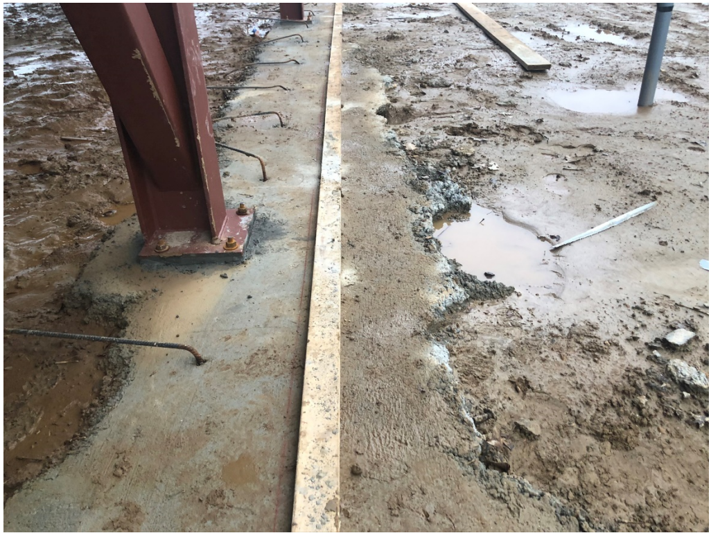
Figure 3 – Formwork Bracing @ Upper Building
