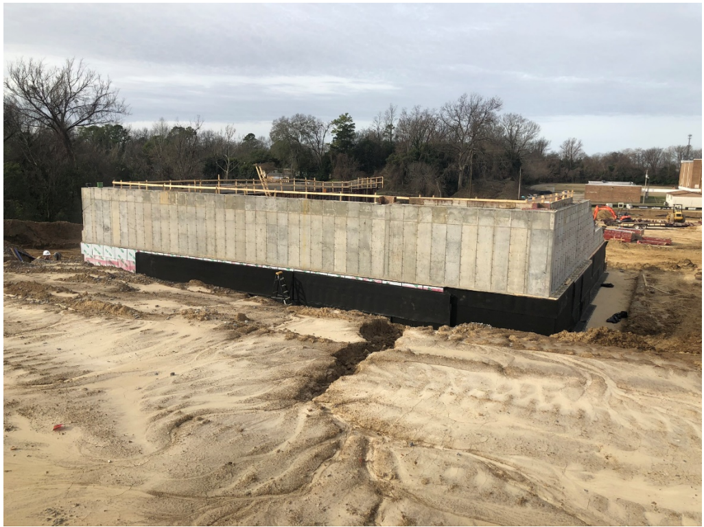
Figure 3 – Foundation (Dirt Side)
