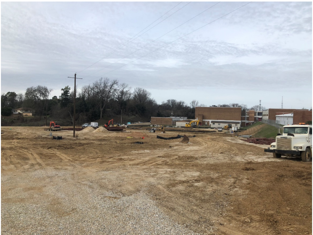
Figure 10 – North Entry Looking WSW
