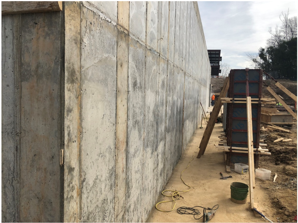
Figure 5 – Formwork Removed @ Exterior of Foundation Wall
