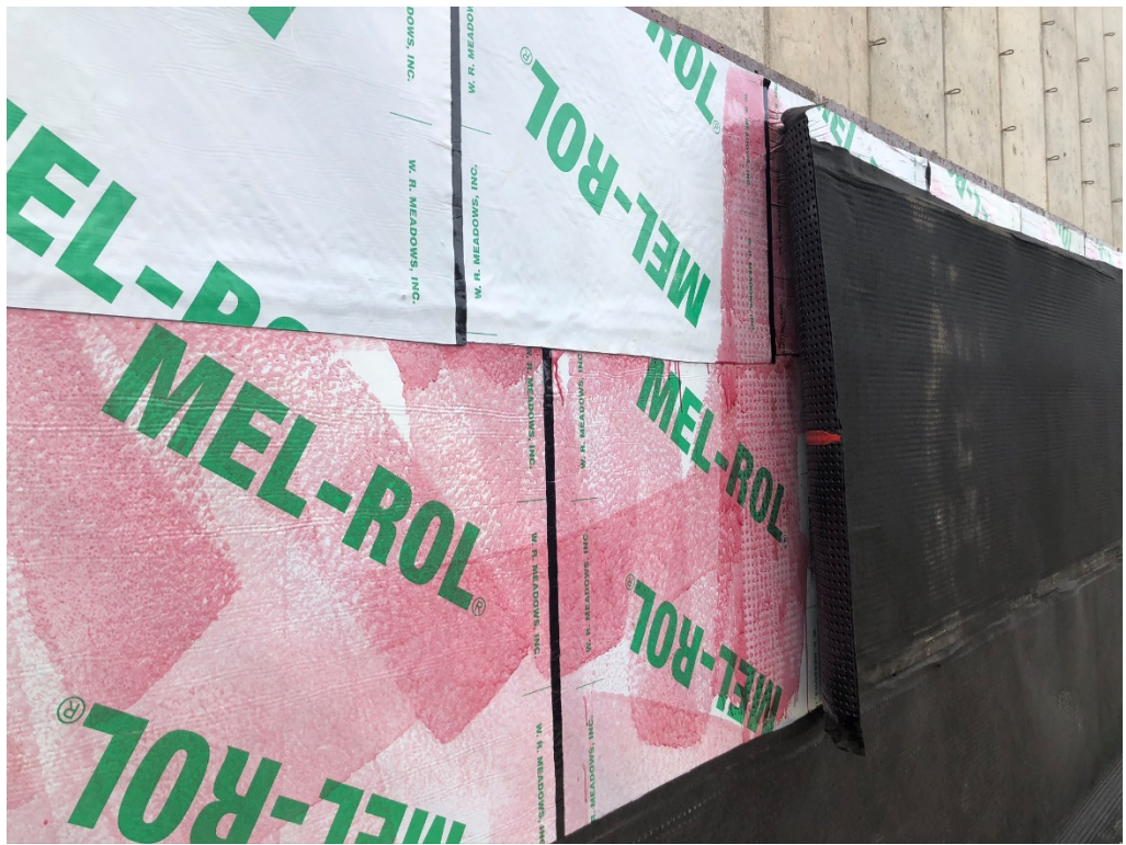
Figure 7 – Bitumen Self Adhering Sub Sheet with Fabric Drainage Plain in Place
