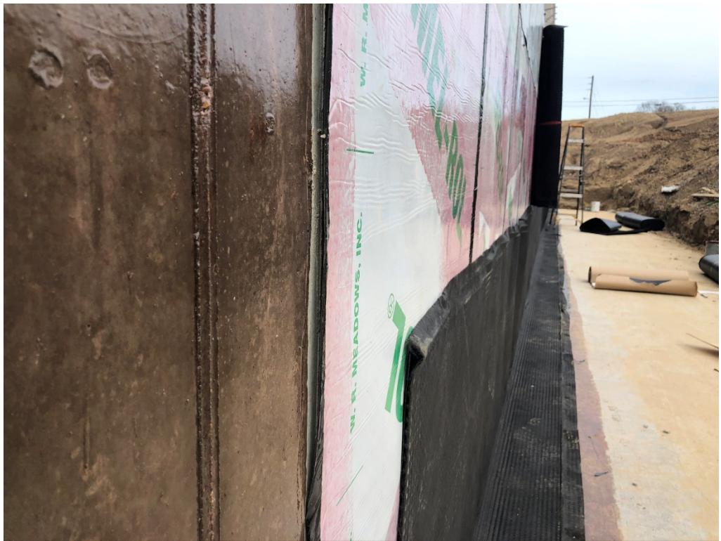
Figure 6 – Mel-Rol Sheet Drainage Assembly
