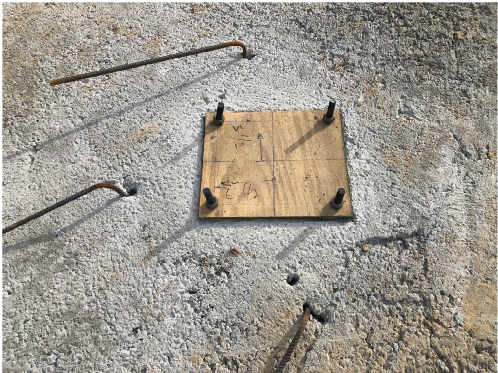
Figure 4 – Bolts for Steel Structure in Place @ Lower Level
