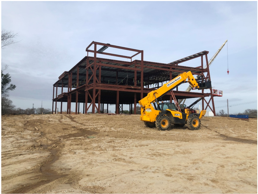
Figure 1 – Red Steel Erected
